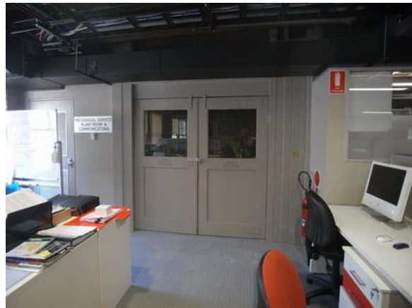
Figure 41: First floor, vertical timber lift enclosure
