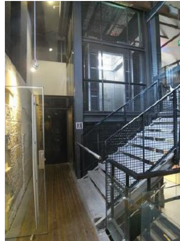
Figure 45: Steel frame stair and caged lift between second and third floors
