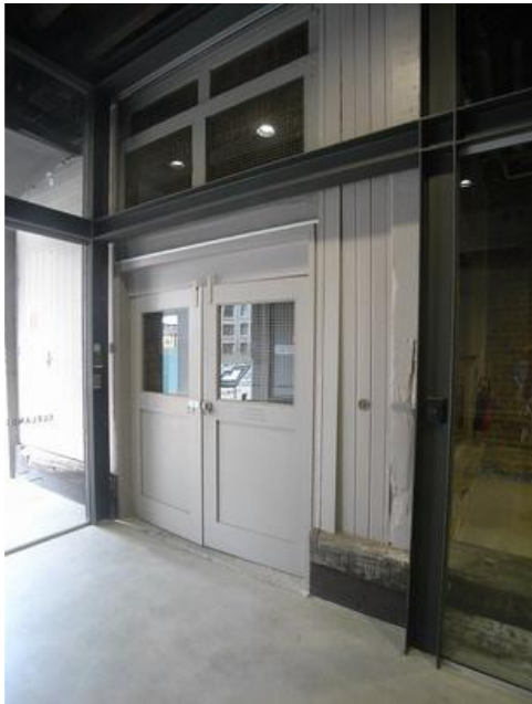
Figure 36: Ground floor, vertical timber lift enclosure
