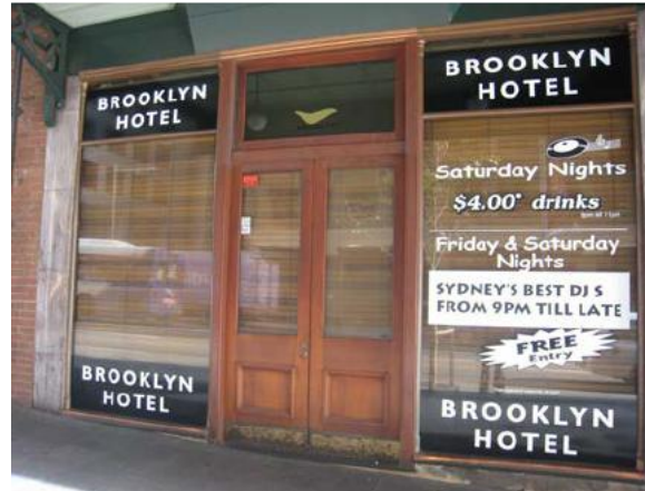
Figure 93 –The Commercial Building shopfront
