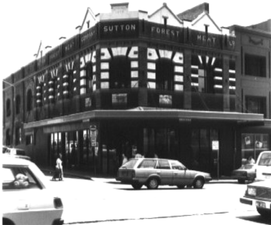
Figure 124– Sutton Forest Meat Building (former)/ 761-763 George Street. The two storey building is heavily influenced by Arts and Crafts
