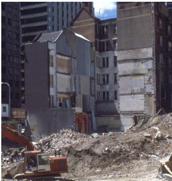
Figure 72 – View of the building group shown partially demolished (c.1983)
