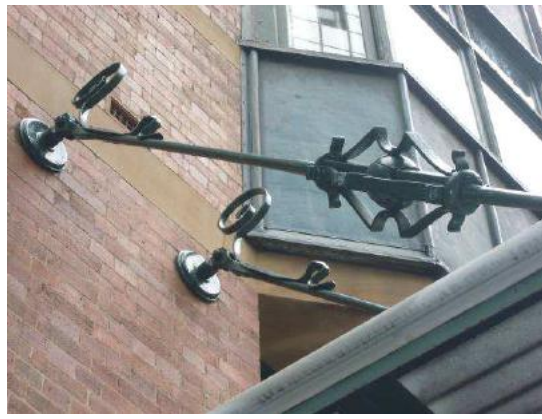
Detail of one of the tie-rods, as viewed from Grosvenor Street.
