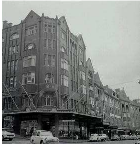
Figure 17– Johnson's Group 1963. Note the scale of the buildings along the western side of George Street.
