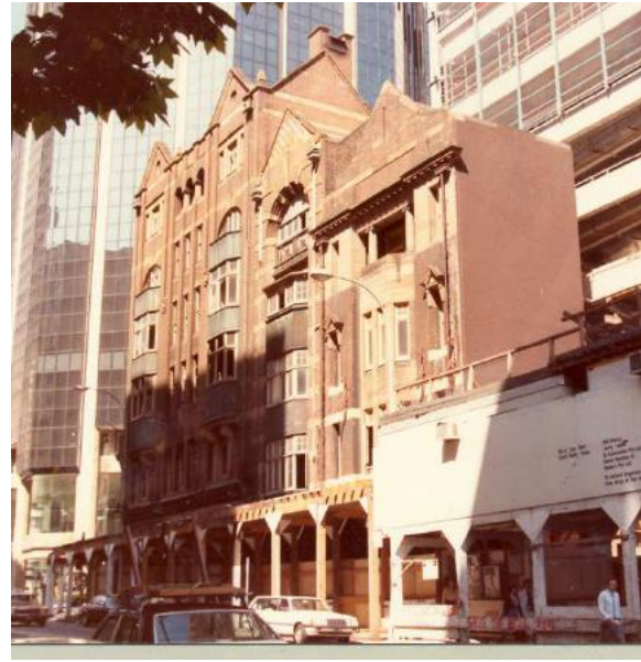
Figure 76 –The fire damaged Johnson's group as viewed from George Street (north)
