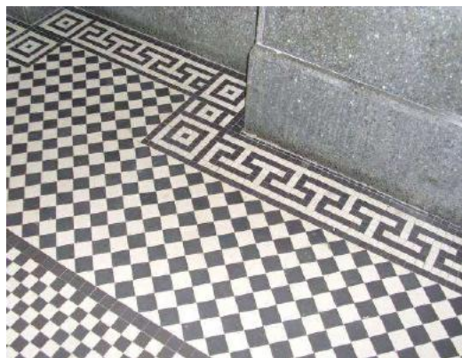
Detail of the classical geometric floor tiling.
