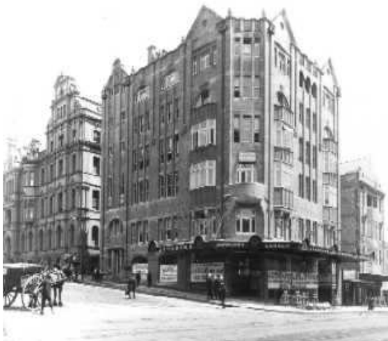
Figure 16 –Johnson's Group 1912 prior to the construction of the Commercial Building. The subject site is indicated.
