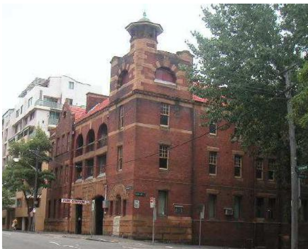
Figure 114 – Pyrmont fire station
