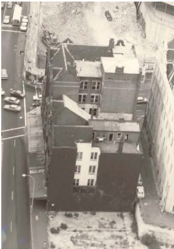
Figure 69 – Aerial view of the site prior to the demolition of the demolition of Royal Naval House (c.1980).
