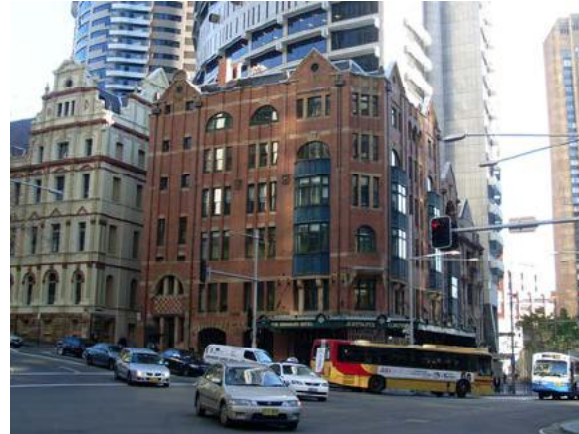
Figure 4 – The Johnson's buildings as viewed from the intersection of George and Bridge Streets.
