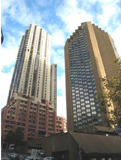
Figure 96 – View west along Essex Street from George, showing the Quay West (left) and Four Seasons Hotels.
