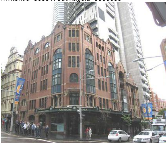
Figure 18 – Streetscape view from Bridge Street showing the Edwardian building group
