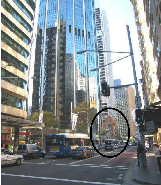
Figure 105– View north along George Street to the Johnson's group. Image taken from the intersection of George and Bond Streets. The Edwardian group creates an element of visual and architectural interest in the context of the surrounding contemporary high rise.
