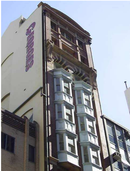
Figure 122– Detail of the upper levels of “Georges House”.
