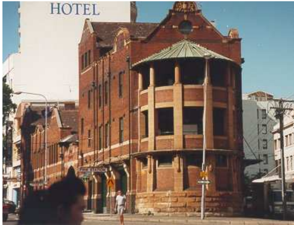
Figure 116 – Darlinghurst Fire Station designed by Vernon 1910-1912
