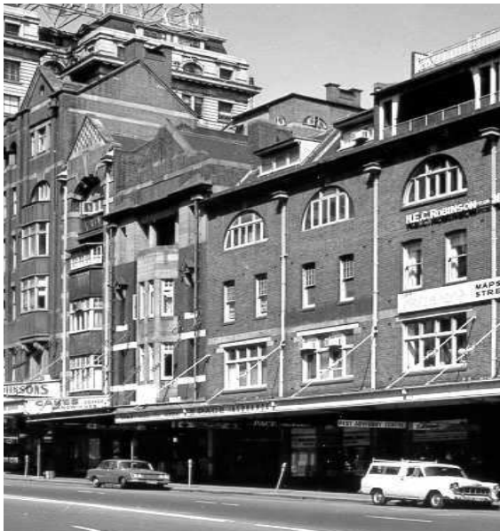
Figure 109– c. 1970 view of George Street west, showing partial view of the Johnson's group and the four storey commercial buildings designed by McRae adjacent.
