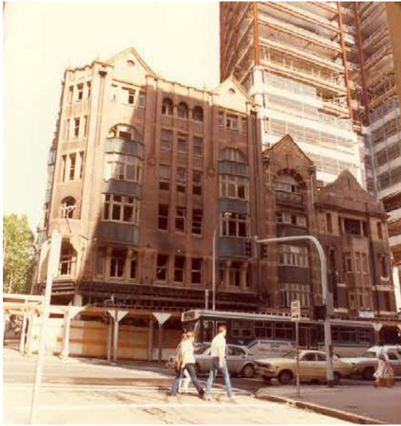
Figure 75 – The fire damaged Johnson's group as viewed from Dalley Street.
