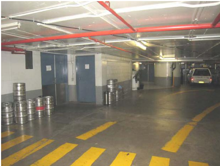
Figure 108 – Subfloor basement view
