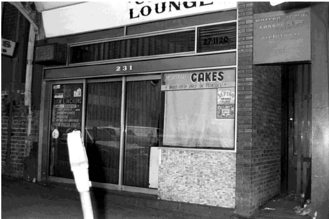
Figure 51 – The former Commercial Building shopfront (undated but likely c.1980).
