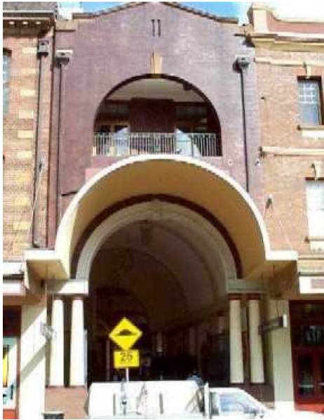
Figure 128– The altered façade of the three storey Federation building at 147 George Street, The Rocks (1914; photographed c.1985)
