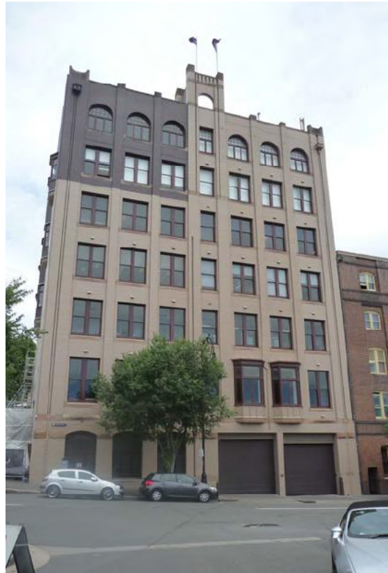
Figure 113 – Bushell's Place elevation, featuring irregular oriel window bays.
