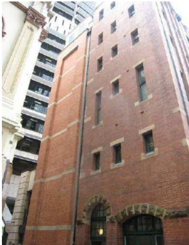
Figure 90 – Rear/ western elevation, showing the original and new sections, delineated by the differing brickwork
