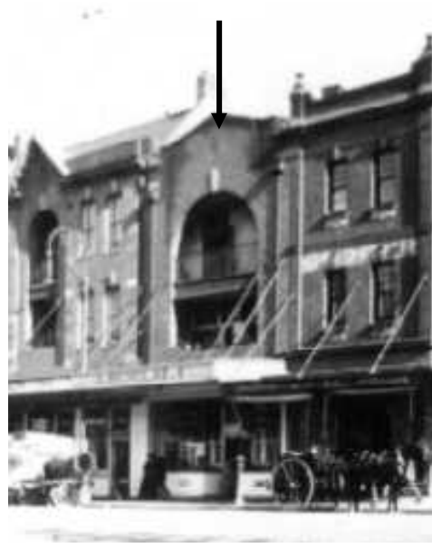
Figure 129– c.1930 view of the 147 George Street showing original shopfront, cantilevered awning and two storey recessed balcony to the upper levels.
