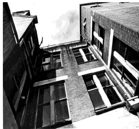
Figure 66 – The former Northern elevation (lightwell) – undated c.1980
