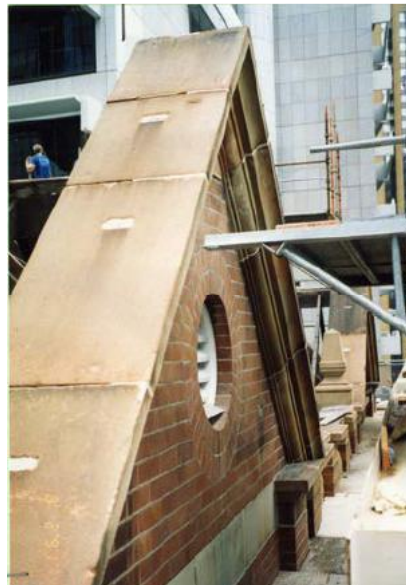
Figure 79– Scaffolding erected in front of the George Street gable (2/8/1991)
