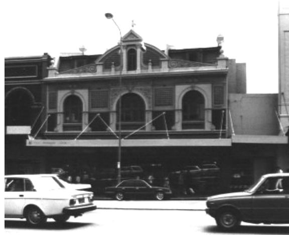
Figure 125– Federation Free Style Commercial Building/ 849-855 George Street (1905). Individualistic example of the style with Anglo-Dutch influences.
