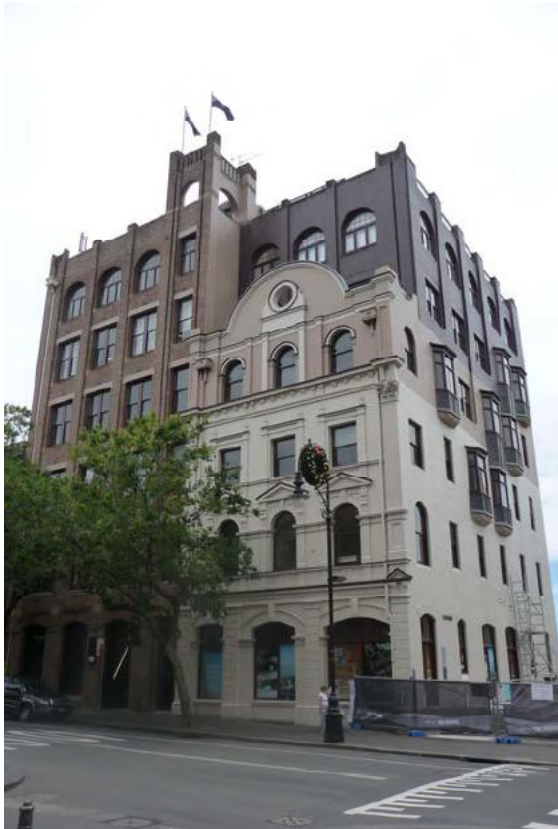
Figure 112 – George Street elevation of the remodelled Bushells building, showing the original Victorian building façade.
