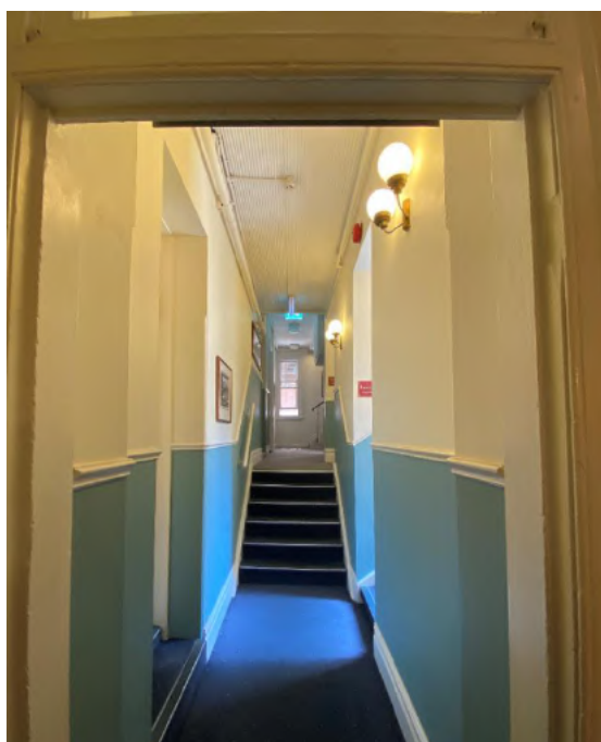
Figure 155: Hallway 1.07, looking west towards the new stair 1.01, was formed by enclosing an open verandah that originally provided access from the front (1887) wing of the building to the rooms of the rear (1913) addition and the rear stair. Most of the fabric dates from the mid 1980s and later, although there are some remaining Edwardian features. Source: TKD Architects 2020.
