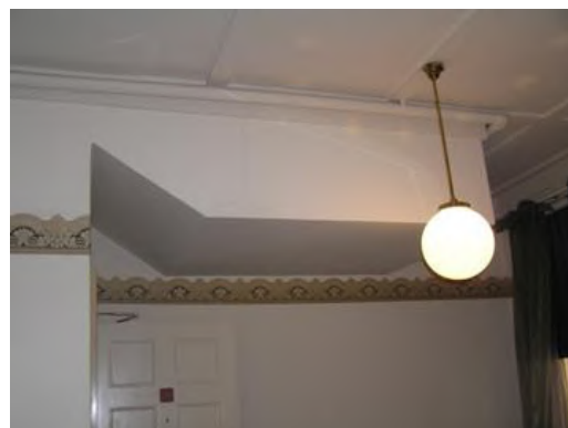
Figure 248: In Room 25 (1.41), the mid 1980s fire stair projects below ceiling level interrupting the original battened ceiling. Source: CMP 2013.
