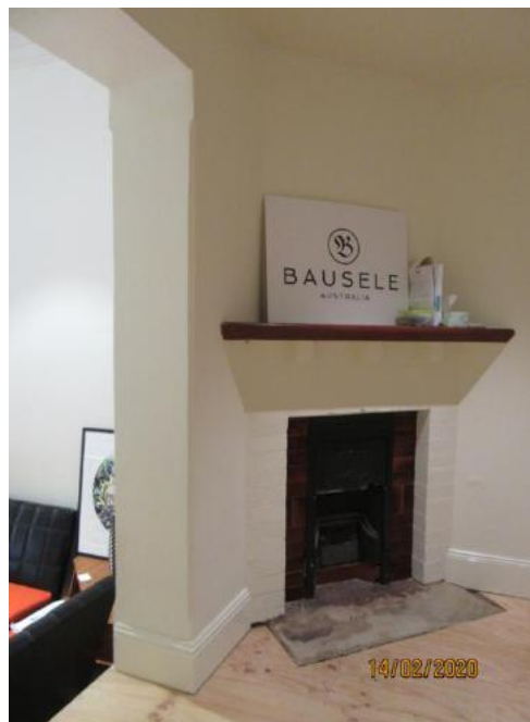
Figure 178: This chimney piece in 141 George Street (G.14) dates from c.1900. It is not original to the 1882 construction of the building but G.13, G.14 the fireplace opening is probably original. Source: TKD Architects 2020.
