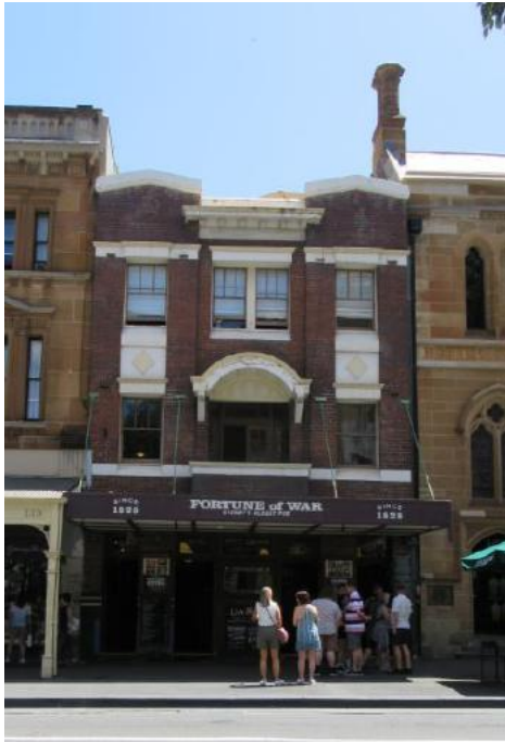
Figure 205: George Street façade of 137 George Street. The 1920s elevation is face brick in English bond with cement render decorative details (cornices, parapet ridge, window sills, lintels, spandrels and arched canopy to the central balcony) and timber windows with three paned upper sashes. Source: TKD Architects 2020.
