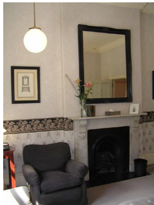
Figure 186: The original marble chimneypiece to Room 22 of The Russell Hotel (1.23) is one of the few surviving elements of early fabric in this area of the building. It is probably original. Some of the timber skirtings in this space are original, while others are modern reproductions. Source: CMP 2013.
