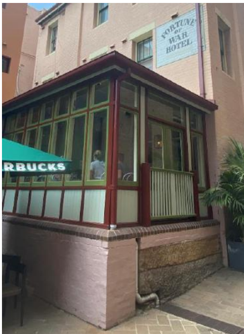
Figure 207: Part of the northern elevation of 137 George Street, showing original windows and the late 1980s verandah addition. The sandstone visible below the balustrade is part of a rock ridge on which the portable hospital once sat. Source: TKD Architects 2020.
