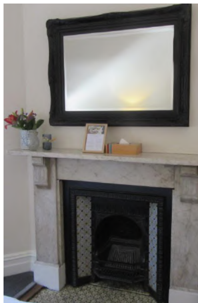
Figure 134: This white marble chimney piece to 1.16 (Room 1), and its cast iron fire place register grate, are original. Spaces 1.17 and have similar chimney pieces, while 2.18 (Room 10) has a painted timber chimney piece. The moulded timber skirtings are also original. Source: TKD Architects 2020.
