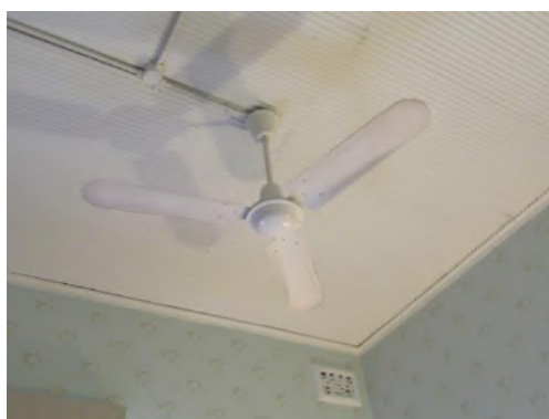
Figure 151: The original ripple iron ceiling, cast iron wall vents and timber cornice of space 1.05 (Room 5) are typical of the ceilings of the guest rooms in the 1913 rear wing of The Russell Hotel (1.05, 1.06, 1.09, 2.05, 2.06 and 2.09). Some of the electrical installation to this wing is original. Source: TKD Architects 2020.
