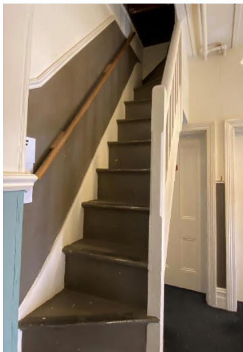
Figure 145: The steep timber stair leading to the attic from the second floor, space 2.02, is original. The set plaster wall finish is original, but the timber dado rail is a modern reproduction. The stair originally led to the hotel's rooftop laundry and drying area. Source: TKD Architects 2020.
