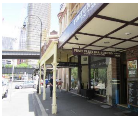
Figure 204: The battened fibre cement ceiling is a reconstruction of an original design feature. Source: TKD Architects 2020.
