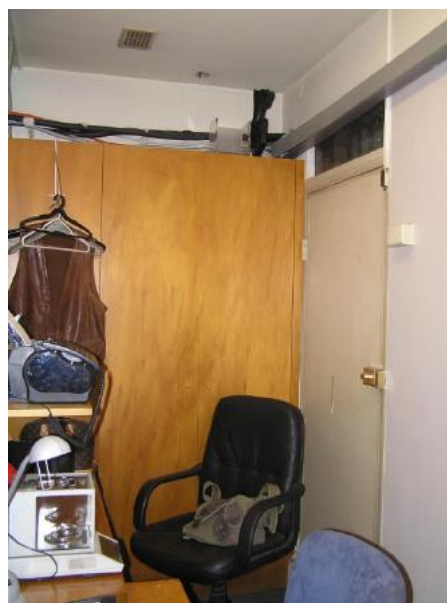
Figure 180: Comparison of the location of this door opening in the rear section of the shop at 141 George Street (G.15) with early plans suggests that it may have been an original window opening. Source: CMP 2013.
