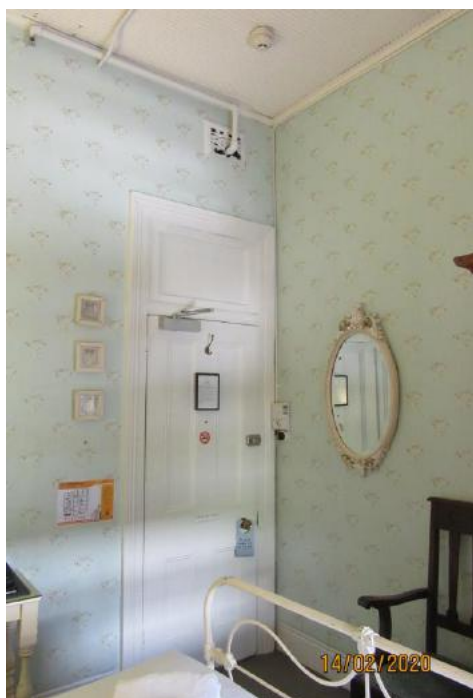
Figure 149: Door and fanlight (painted over) to space 1.05 (Room 5). This original door joinery is typical of the rooms to the 1913 rear wing of The Russell Hotel (1.05, 1.06, 1.09, 2.05, 2.06, 2.09). Source: TKD Architects 2020.
