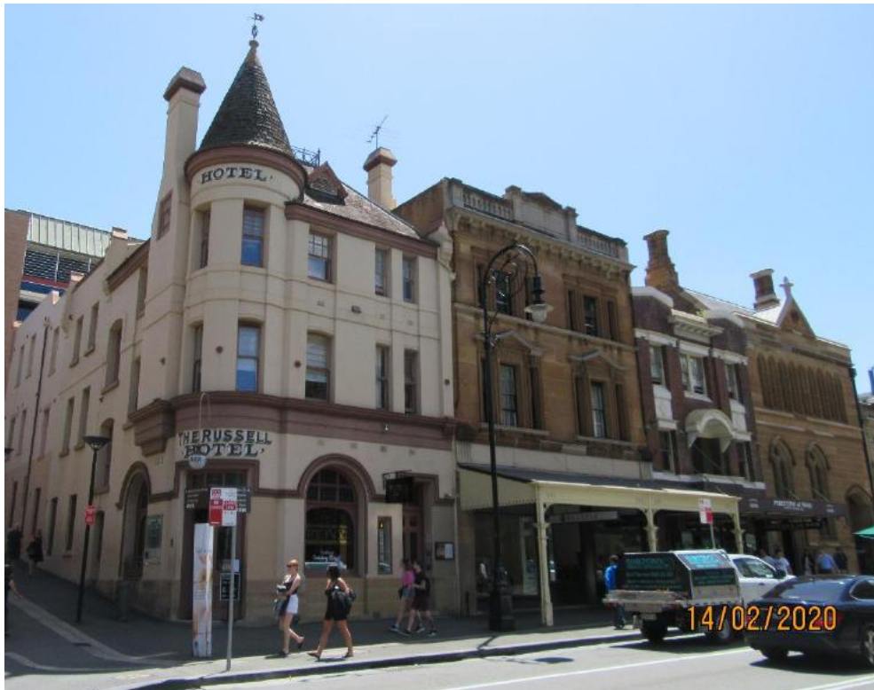
Figure 5: Eastern elevation on George Street of the study area. The façade of The Russell Hotel on the corner of George and Globe Streets is rendered and painted masonry, the shops at 139-141 George Street are of sandstone and The Fortune of War has a face brick façade. 139-141 George St has an awning supported by three timber posts, and The Fortune of War has a cantilevered steel awning over the footpath. Source: TKD Architects 2020.
