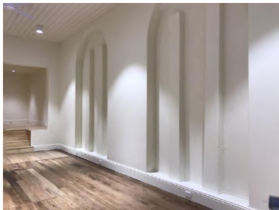
Figure 183: Painted brick party wall between 139 and 141 George Street (taken from G.18). The original structural brick arches are clearly visible. Source: PMNSW 2019
