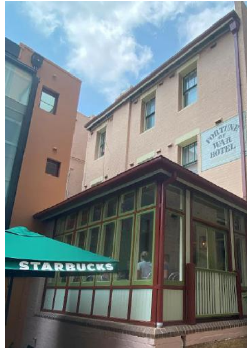
Figure 206: Painted brick rear (western) elevation of 137 George Street. The flat roof over the front section of the building is concealed from view by the roof level laundry structure. The roof of the rear section of the building is visible from Nurses Walk and has exposed eaves. Source: TKD Architects 2020.
