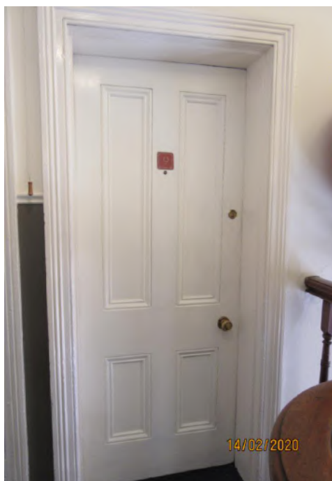
Figure 143: The door leading from space 2.02 to space 2.17 (Room 9). The four panel door joinery is typical of the original (1887) section of the building and the door leaf, architraves and skirtings are original. Source: TKD Architects 2020.
