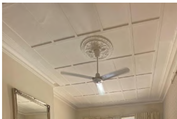
Figure 140: The battened ceiling to Room 2 (1.17) is typical of the ceiling finish to the original section of the building (1887) except for in the smaller guest rooms, which had timber boarded ceilings. Source: TKD Architects 2020.
