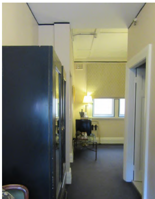
Figure 254: Space 2.34 (also in Room 27) has a relatively recent ceiling. An original section of battened ceiling can be seen in 2.33, at the rear. To the right of 2.34 is an en suite bathroom (2.35) added in the late 1980s. Source: TKD Architects 2020.
