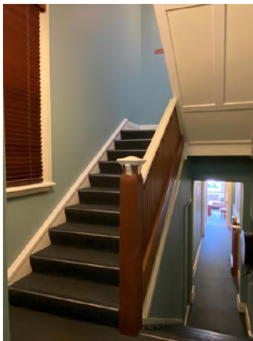
Figure 239: The stair (1.03) retains its original timber balustrades and handrails. Source: TKD Architects 2020.
