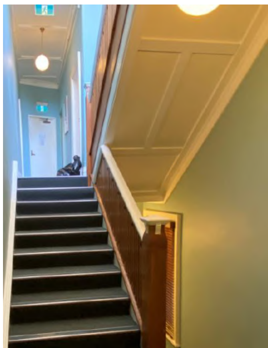
Figure 255: Original timber balustrade, handrail and newel post to stair 2.03. The battened soffit is also original. Source: TKD Architects 2020.
