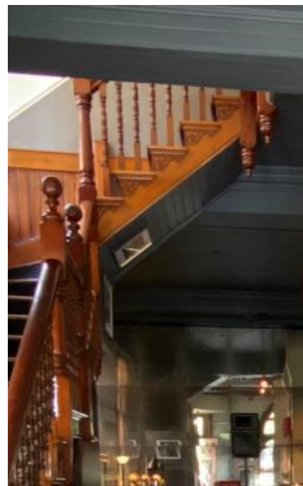
Figure 128: The Russell Wine bar, space G.11. The beams at ceiling level in this image and Figure 66 indicate the former locations of original internal walls. The wine bar fitout is recent. The timber boarded stair soffit is modern. Source: TKD Architects 2020.
