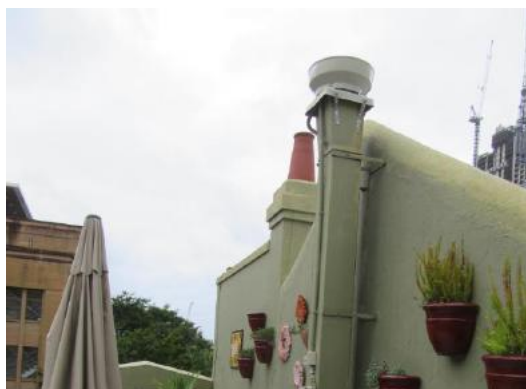
Figure 211: This rendered masonry gable on the southern side of the roof terrace at 137 George Street is probably the original southern wall of the original Fortune of War Hotel. Source: TKD Architects 2020.
