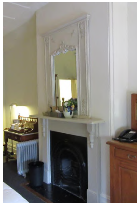
Figure 138: Room 19 (2.18) has a painted timber chimney piece. This is the only chimney piece of this type in the original section of the building and it is possible that it is a later replacement of the original. However, the Clive Lucas Stapleton CMP of 1999 notes it as being original. Source: TKD Architects 2020.
