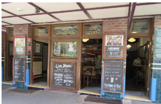
Figure 203: Original tiled dado, yellow terrazzo thresholds to the George Street elevation. The trachyte margins around the steel grilles to the keg drops are also visible. Source: TKD Architects 2020.
