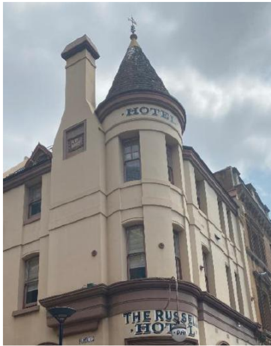
Figure 123: The corbelled chimney and distinctive conical tower of The Russell Hotel. The date plaque on the chimney reads 1887, the date of the construction of the original portion of the building. Source: TKD Architects 2020.
