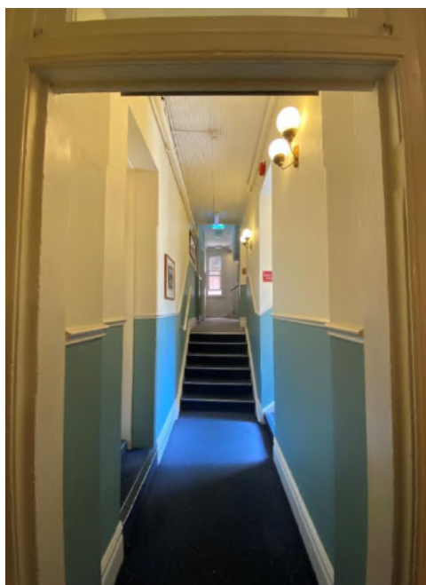
Figure 147: View from The Russell Hotel reception, space 1.13, looking west along hallway 1.07. The opening to 1.07 was made during the 1913 construction of the rear wing of the building. A similar opening directly above, on the second floor, was made at the same time. Source: TKD Architects 2020.
