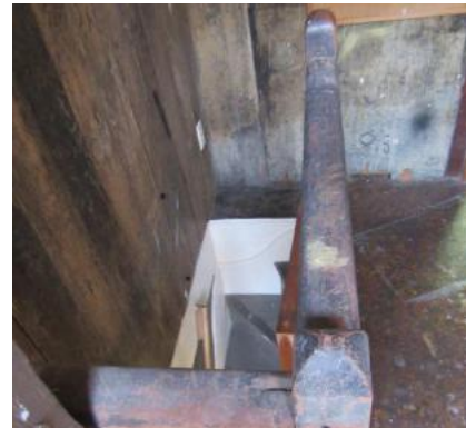
Figure 162: The top of the stair in space R02. The beaded timber lining boards on the wall adjacent to the stair are original. Source: TKD Architects 2020.
