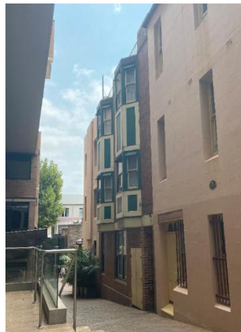
Figure 126: The door and window opening (bottom right) to the western elevation was created post 1913. The window directly above, originally to a guest room, now to stair 1.01, is original. To the left sit the rear elevations of 137–141 George Street. Source: TKD Architects 2020.
