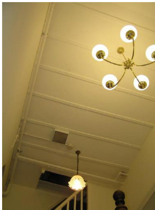
Figure 146: The batted ceiling of the stairhall, 2.02, showing the opening in the ceiling through which the attic is reached. The ceiling is lath and plaster and is 2.022 original, although the timber battens may be later, possibly Edwardian, additions. Source: TKD Architects 2020.
