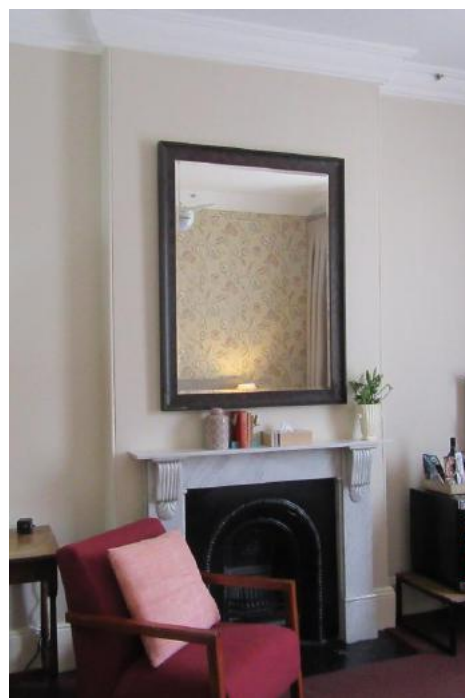
Figure 188: Room 21 of The Russell Hotel (1.28) showing the chimney piece which is original but has been restored. The remainder of the room contains very little original fabric. Source: TKD Architects 2020.
