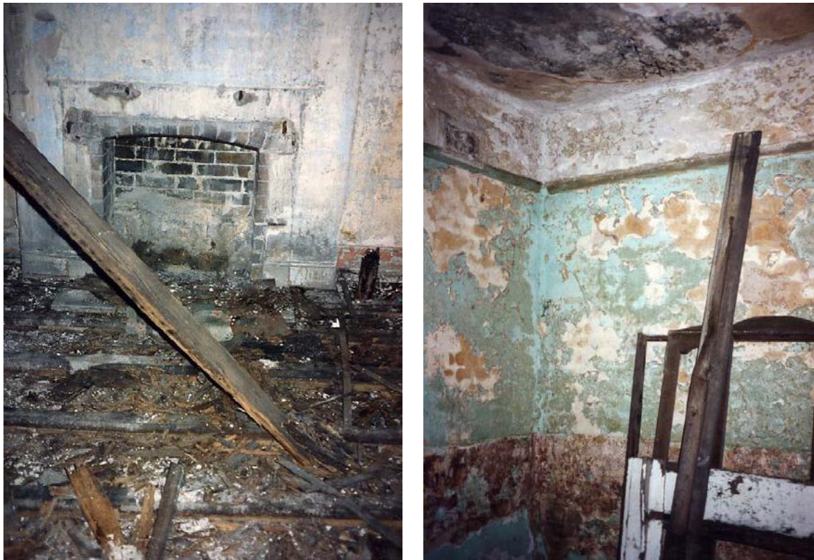
Figure 24: 117-117A Gloucester Street, Remains of interiors with fireplace, plaster ceiling and walls and paint scheme, c1993. Source: Sydney Harbour Foreshore Authority
