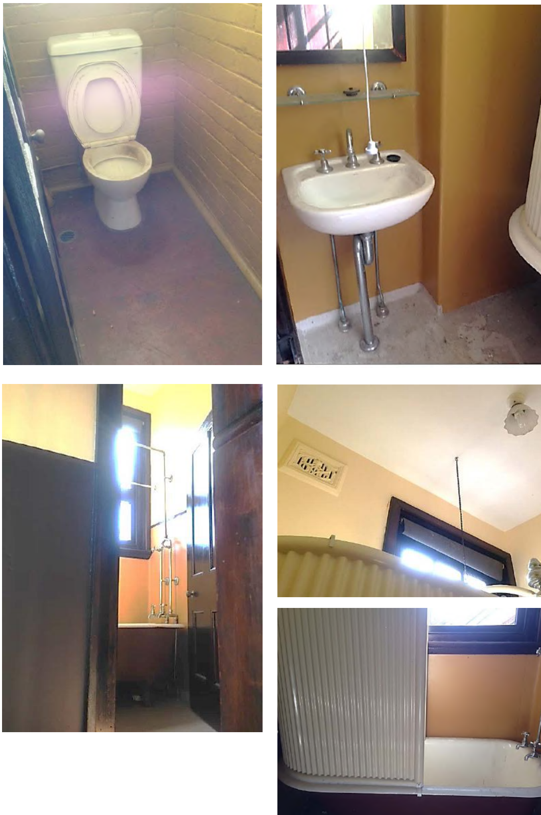
Figure 80: Toilet (A5) and Bath Room (A6) cast iron bath with ripple iron shower screen over, double hung sash window, air vent and light fitting, 117A Gloucester Street, 2016. Source: Sydney Harbour Foreshore Authority, M Stacy
