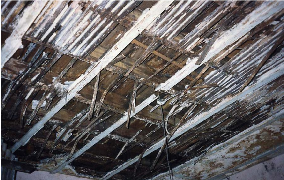
Figure 22: 117-117A Gloucester Street, Remains of lathe and plaster ceiling and underside floor joinery c1993. Source: Sydney Harbour Foreshore Authority
