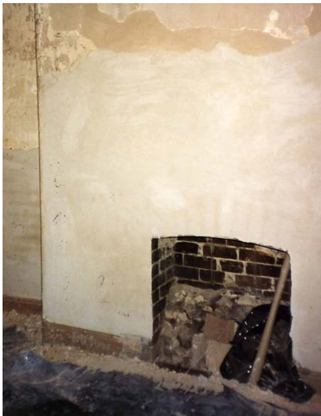
Figure 28: 117-117A Gloucester Street. Replastered walls and chimney breast and repaired door joinery, 1995. Source: Sydney Harbour Foreshore Authority
