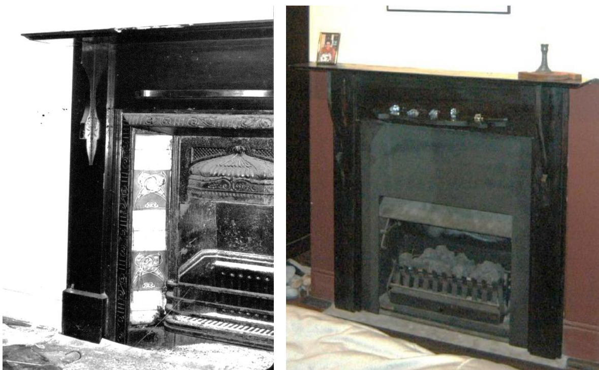
Figure 34: Typical fireplace in 117-117A Gloucester Street; (left) 1970s, (right) 2007. While the timber chimney pieces survive or were reconstructed as part of the conservation works in 1994, the tile firebox surrounds and iron grates have been removed and replaced. (Source: (left) Sydney Harbour Foreshore Authority 48991 GLM65, (right) Clive Lucas Stapleton & Partners).
