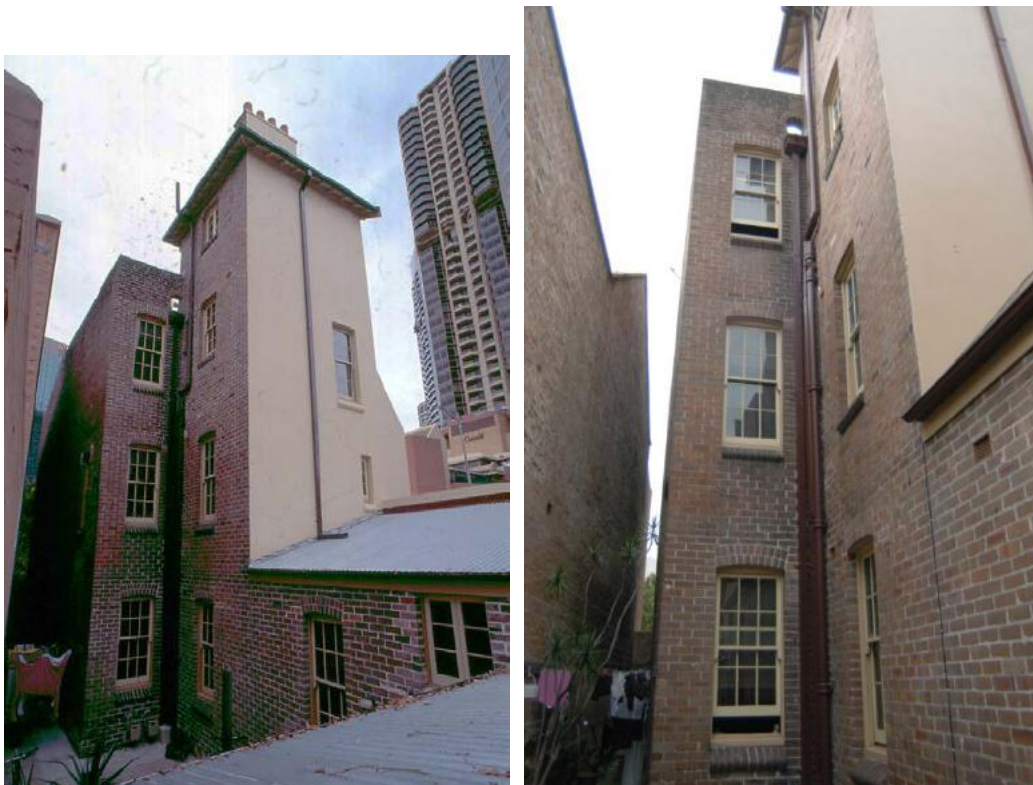
Figure 32: 117-117A Gloucester Street after conservation showing the restored window sashes in 1996 and 2007. Source: Sydney Harbour Foreshore Authority
