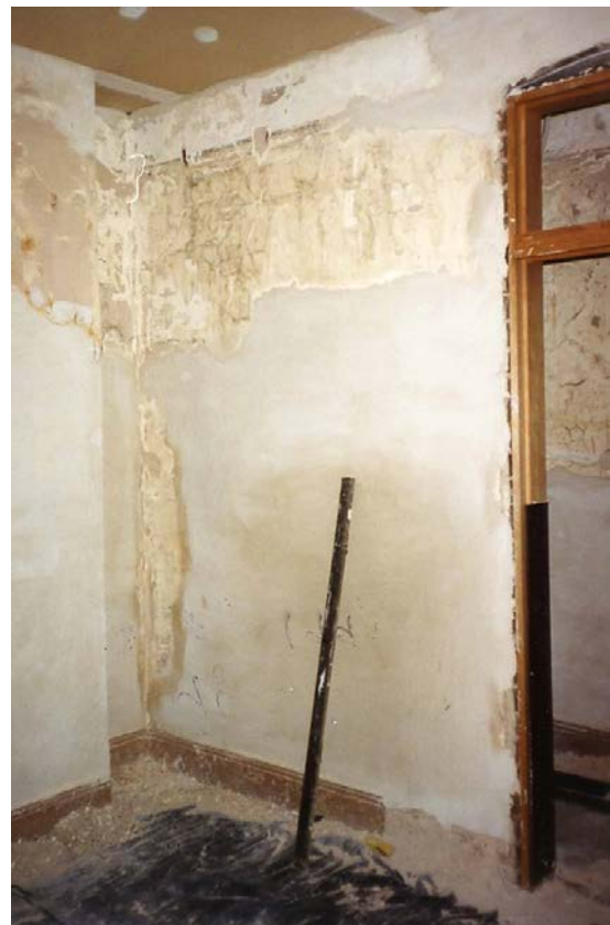
Figure 28: 117-117A Gloucester Street. Replastered walls and chimney breast and repaired door joinery, 1995. Source: Sydney Harbour Foreshore Authority
