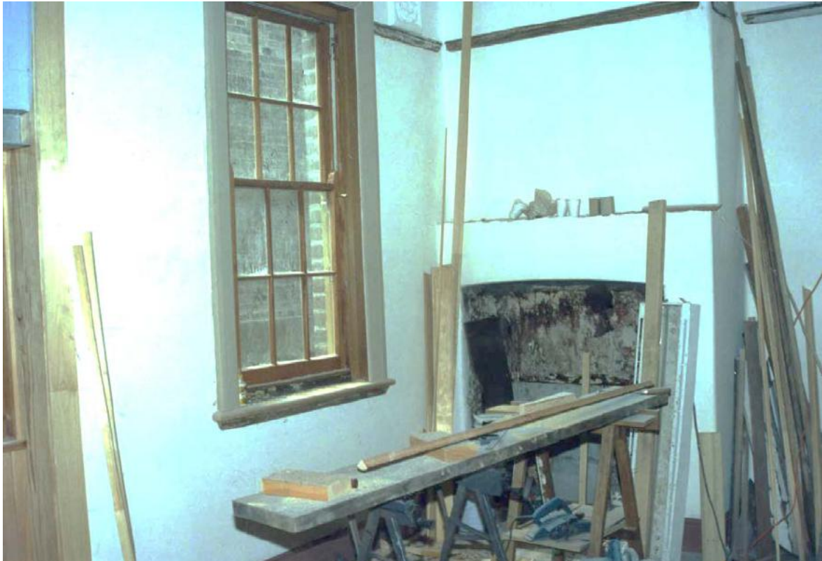
Figure 29: 117-117A Gloucester Street. Replastered walls and chimney breast and repaired window joinery, ground floor rear kitchen, 1995. Source: Sydney Harbour Foreshore Authority
