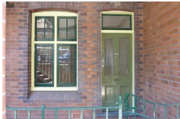
Figure 4.4 Detail of western elevation to Flat 46 at ground floor level, showing original casement windows and panel door with fanlight, slate threshold and contrasting brick arched heads and surrounds to openings. (Source: GML 2015)
