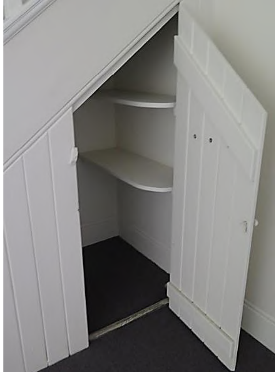
Figure 4.31 Cupboard under the stairs in living room (space 1.3) with original T&G boarding and ledged timber door—48A / 46–56 Gloucester Street. (Source: GML Heritage, May 2016)
