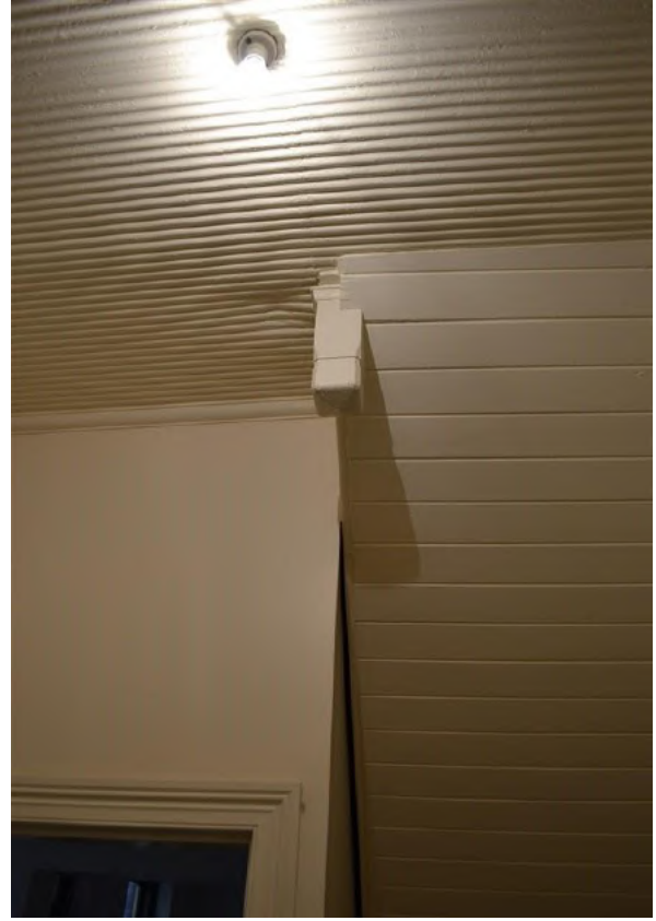
Figure 5.39 Laundry (space LG.3) showing the original ripple iron ceiling, T&G boarded timber stair soffit and newel post extending from ceiling above—50 / 46–56 Gloucester Street. (Source: GML Heritage, June 2016)
