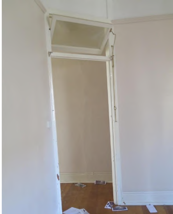
Figure 15.23 Living room (space G.3) showing new opening with the repurposed original fanlight of removed door to entry hall—56B / 46–56 Gloucester Street. (Source: GML Heritage, June 2016)
