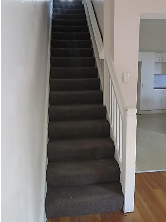
Figure 9.22 Stair with modern carpeting (space G.7) showing original timber handrail and modern T&G boarding—54 / 46–56 Gloucester Street. (Source: GML Heritage, July 2016)
