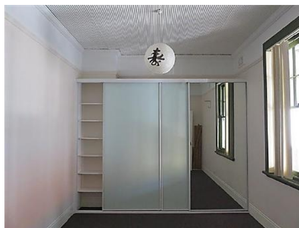
Figure 16.21 Front bedroom (space 1.2) showing the cement rendered skirting, moulded timber picture rail, timber cornice and ripple iron ceiling. The modern wardrobe is not significant—56C / 46–56 Gloucester Street. (Source: GML Heritage, July 2016)
