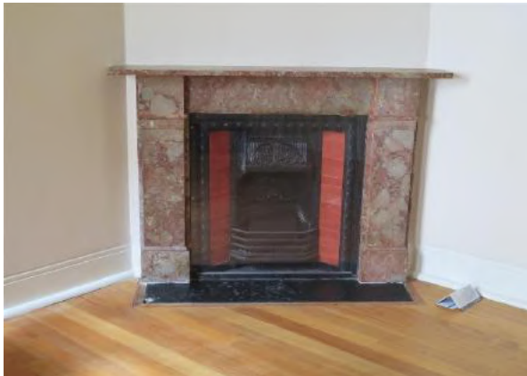
Figure 11.16 Marble chimney piece with cast-iron and tiled grate, and painted concrete hearth in the living room (space G.3)—54B / 46–56 Gloucester Street. (Source: GML Heritage, July 2016)
