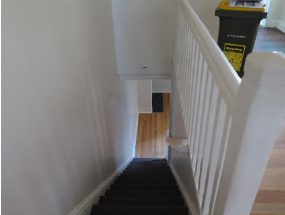
Figure 11.18 Timber balustrade and newel post, moulded handrail and stairs (space G.7) from living room (space G.3)—54B/ 46–56 Gloucester Street (Source: GML Heritage, July 2016)
