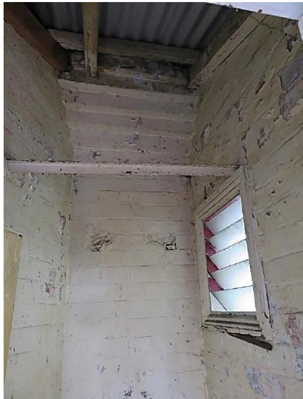
Figure 7.37 The interior of space E.3 showing the original fixed glass louvres in the window—52 / 46–56 Gloucester Street. (Source: GML Heritage, July 2016)
