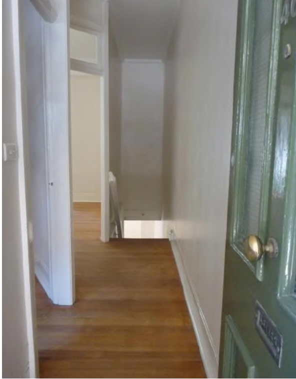
Figure 4.29 The front hallway (end flat, ground floor level, Flat 46) showing refinished wood floor, splayed coke-breeze partition and expressed door frame to the left of the stairs. (Source: GML 2015)
