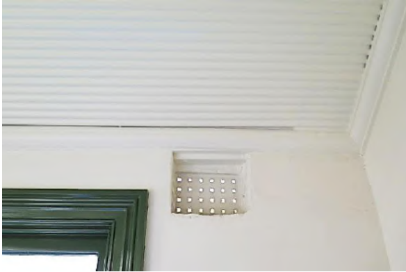
Figure 4.46 Later grille pattern wall vents and ripple iron ceiling with timber cornice in laundry (space 2.2)—48A / 46–56 Gloucester Street. (Source: GML Heritage, May 2016)
