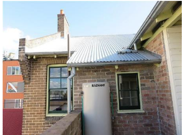
Figure 16.13 Rear elevation from roof terrace (space E.1) showing the corrugated metal roof, and the corbelled brick eaves to the party wall, and chimney stack with terracotta pots—56C / 46–56 Gloucester Street. (Source: GML Heritage, July 2016)
