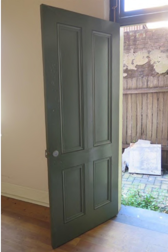
Figure 15.46 Lower ground-floor (LG.1) showing four panelled timber door with fanlight above—56B / 46–56 Gloucester Street. (Source: GML Heritage, July 2016)
