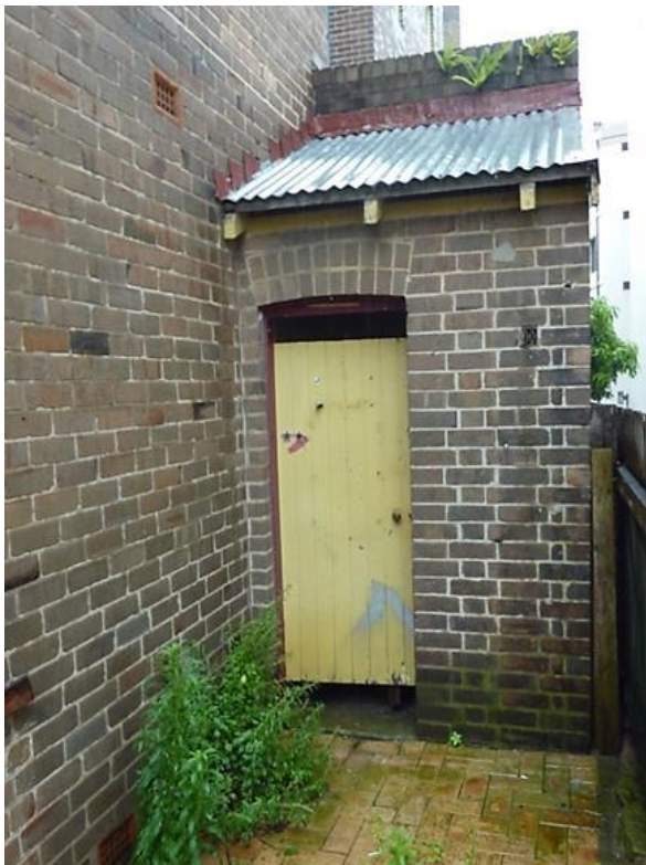
Figure 4.15 Detail of the outside toilet with skillion roof and timber-boarded door (Flat 54), and later paving to rear yard. (Source: GML 2015)
