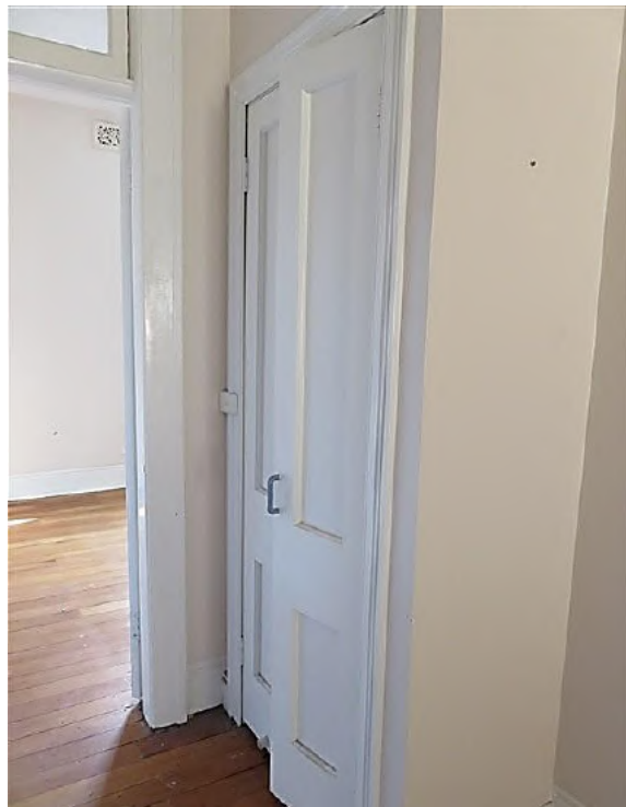
Figure 14.40 Built-in cupboard with panel doors is recent addition. It covers original door opening to space 2.3—56A / 46–56 Gloucester Street. (Source: GML Heritage, July 2016)
