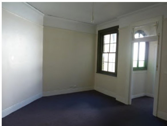
Figure 2.24 Living room (space 1.3) showing the original double hung window with four pane sashes, and original doorframe with fanlight above—46A/46–56 Gloucester Street.. (Source: GML Heritage, July 2016)
