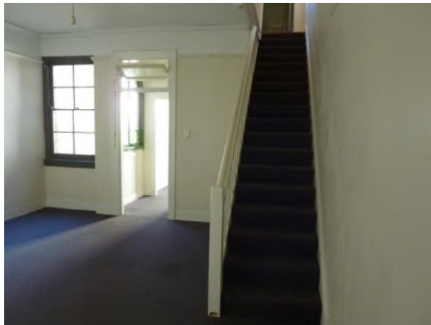
Figure 4.28 The main space on first floor level with stair (Flat 50A). Note the walls are rendered to the dado with rendered skirting, and timber picture rail and cornice to ripple iron ceiling. (Source: GML 2015)
