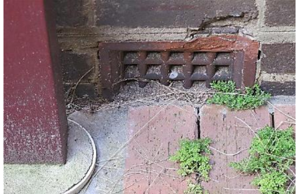
Figure 13.37 Original terracotta subfloor vent, partially covered by brick paving—56 / 46–56 Gloucester Street. (Source: GML Heritage, July 2016)
