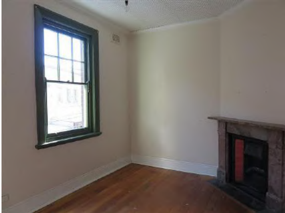
Figure 14.47 Front room on second floor (space 2.4) showing the original double hung window (complete with original architraves and sill board), ripple iron ceiling, timber cornice, timber floor and marble chimney piece to fireplace—56A / 46–56 Gloucester Street. (Source: GML Heritage, July 2016)
