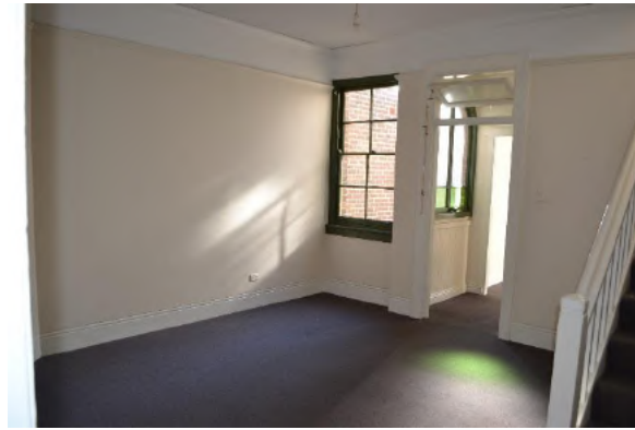
Figure 6.21 Living room (space 1.3)—50A / 48–56 Gloucester Street, showing cement rendered skirtings, timber picture rail, ripple iron ceiling and moulded timber cornice. Original sash window with original architraves. (Source: GML Heritage, July 2016)
