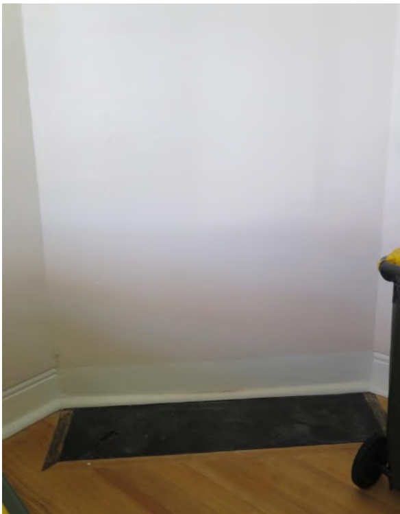
Figure 13.16 Original, now blocked off, corner fireplace (space G.2)—56 / 46-56 Gloucester Street. (Source: GML Heritage, July 2016)
