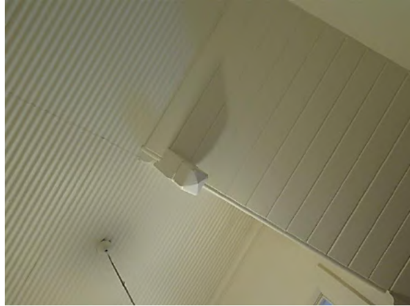
Figure 9.31 Laundry (space LG.3) showing boarded soffit to stair, newel pendant and ripple iron ceiling. (Source: GML Heritage, July 2016)
