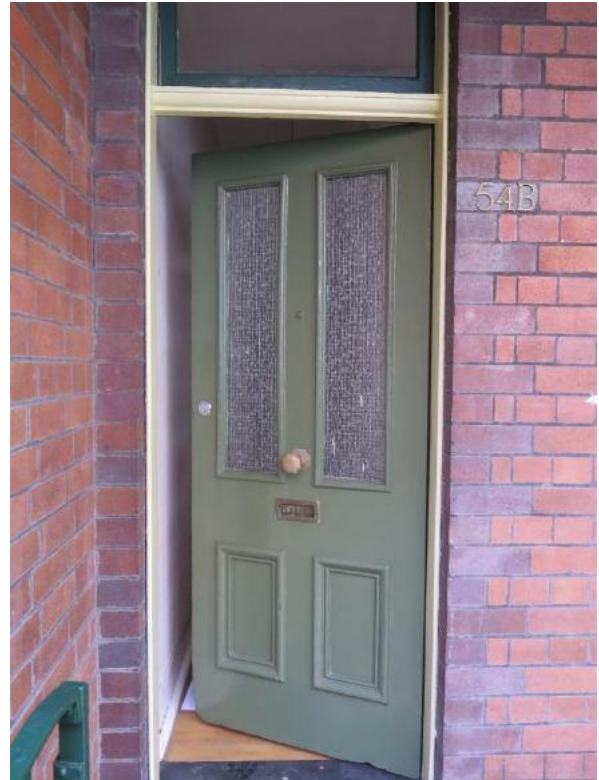
Figure 11.7 The four-panel front door with bolection moulds to bottom panels and wired glass to top panels, fanlight above, dark brick surround, number plate and slate threshold—54B / 46-56 Gloucester Street. (Source: GML Heritage, July 2016)
