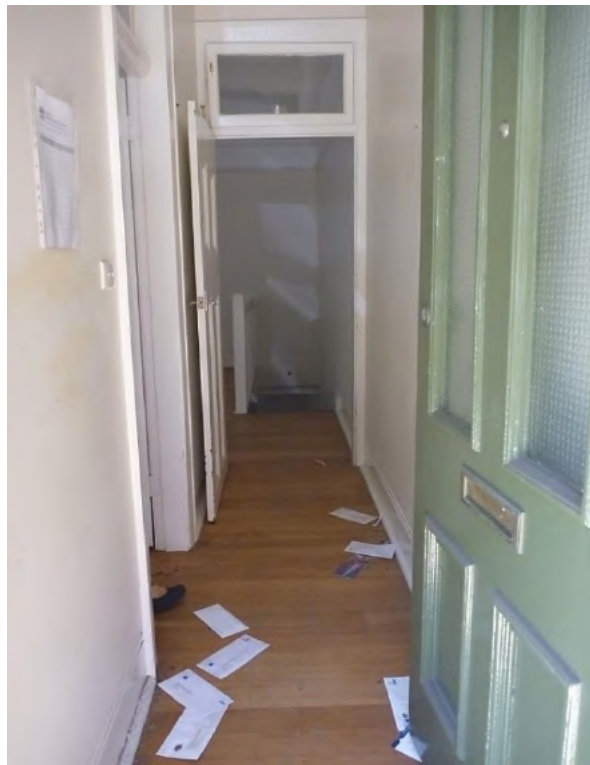
Figure 5.13 The entry (space G.1) showing the timber floor, cement run skirting and timber door frame with fanlight above to front bedroom (space G.2) and living room (space G.3)—50 / 46–56 Gloucester Street. (Source: GML Heritage, November 2015)
