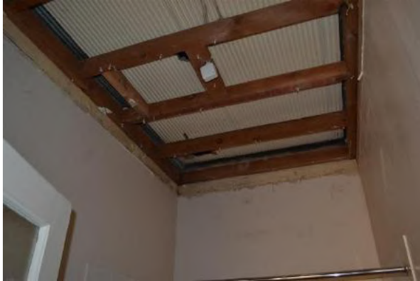
Figure 1.30 Bathroom (space G.5). The plasterboard ceiling has been removed—46/46–56 Gloucester Street. (Source: GML Heritage, July 2016)
