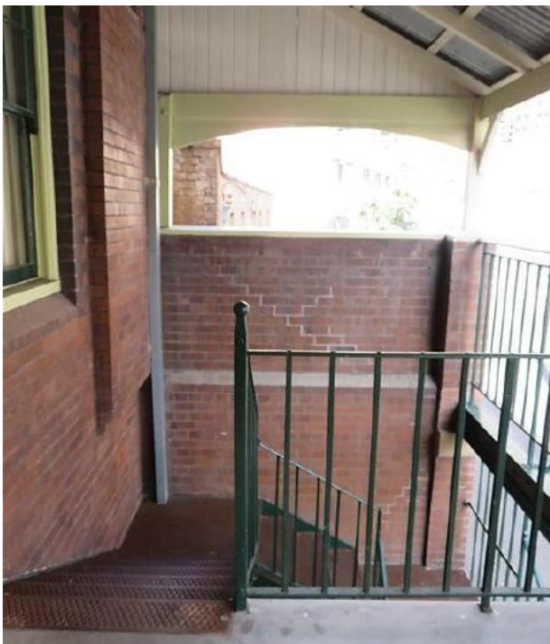
Figure 16.8 Detail of exterior staircase to ground floor at the southern end of the building. The brickwork corbels out over the stair to the south of the front window of Flat 56C—56C / 46–56 Gloucester Street. (Source: GML Heritage, July 2016)
