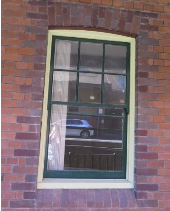
Figure 3.10 Double-hung window with chamfered brick sill, twenty-first century glass in the lower sash, and dark brick surrounds—48 / 46–56 Gloucester Street. (Source: GML Heritage, May 2016)
