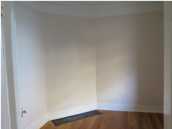
Figure 11.12 Front bedroom (space G.2) showing timber floors, rendered wall finishes, fireplace blocked up with cement rendered skirting over and original concrete hearth—54B / 46–56 Gloucester Street. (Source: GML Heritage, July 2016)
