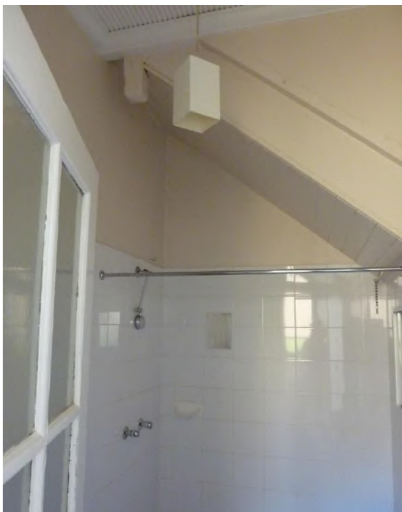
Figure 2.33 Bathroom (space 1.5) showing modern fit out, v-jointed timber stair soffit with ripple iron to ceiling—46A/46–56 Gloucester Street. (Source: GML Heritage, July 2016)
