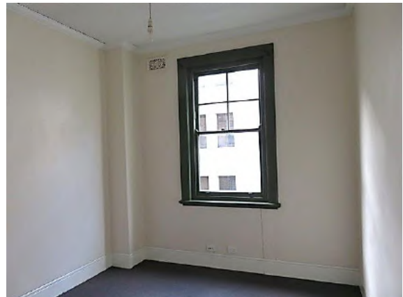
Figure 12.33 Rear bedroom (space 1.6) showing the original double hung sash window, cement run skirting, ripple iron ceiling and moulded timber cornice. A chimney flue rises up through the northeast corner of the room—54C / 46–56 Gloucester Street. (Source: GML Heritage, July 2016)
