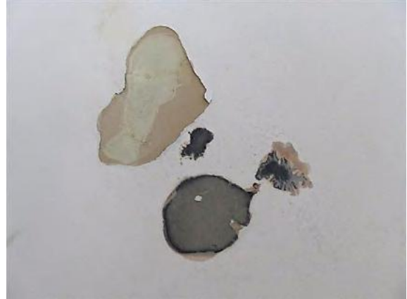
Figure 12.47 Paint scrapes above the stair reveal a dark painted dado and a lighter colour on the wall above—54C / 46–56 Gloucester Street. (Source: GML Heritage, July 2016)
