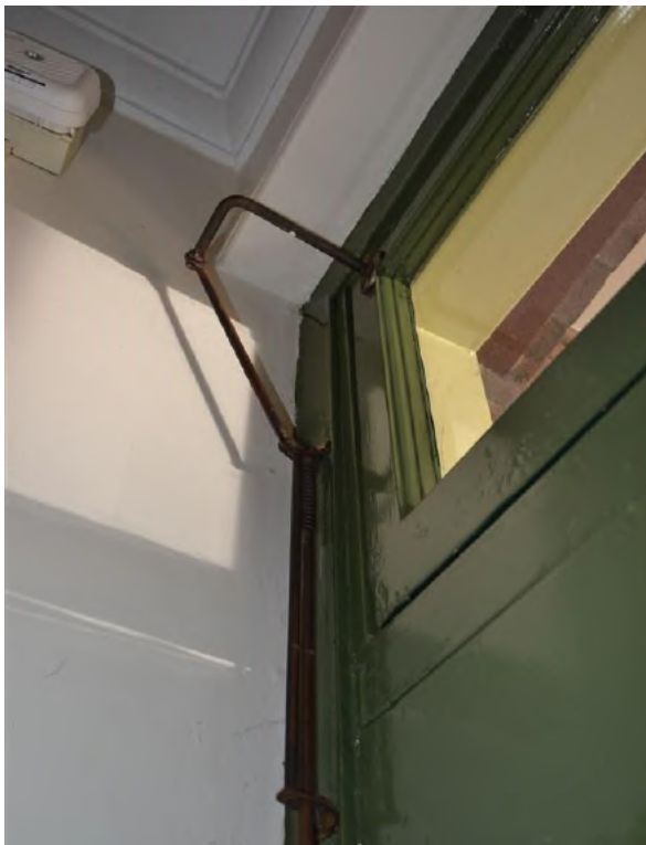
Figure 5.12 Original (?) mechanism to the pivot fanlight over the front door—50 / 46–56 Gloucester Street. (Source: GML Heritage, June 2016)
