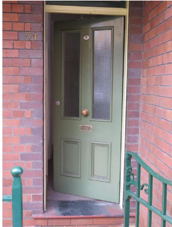
Figure 9.7 The four-panel front door with bolelection moulds to bottom panels and wired glass to top panels, fanlight above, dark brick surround and slate threshold—54 / 46–56 Gloucester Street. (Source: GML Heritage, July 2016)
