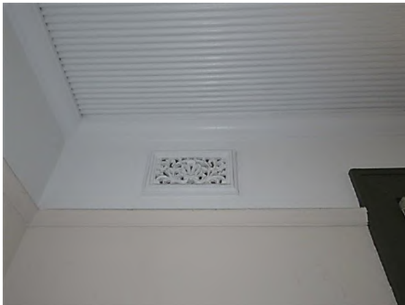
Figure 8.36 Decorative plaster wall vent, ripple iron ceiling, timber cornice and picture rail in the rear bedroom (space 1.6)—52A / 46–56 Gloucester Street. (Source: GML Heritage, July 2016)
