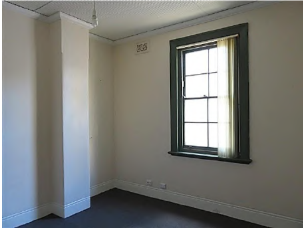
Figure 16.34 Rear bedroom (space 1.6) showing original double-hung window, complete with original architrave, sill board and moulding, chimney flue against north wall, decorative plaster wall vent and ripple iron ceiling with timber cornice—56C / 46–56 Gloucester Street. (Source: GML Heritage, July 2016)
