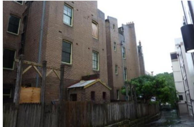
Figure 3.8 Eastern elevation of the building at 46–56 Gloucester Street, facing Cambridge Street, showing exterior WCs, timber-framed laundry hoists within the rear yards and a mango tree at rear of Flat 52. (Source: GML 2015)
