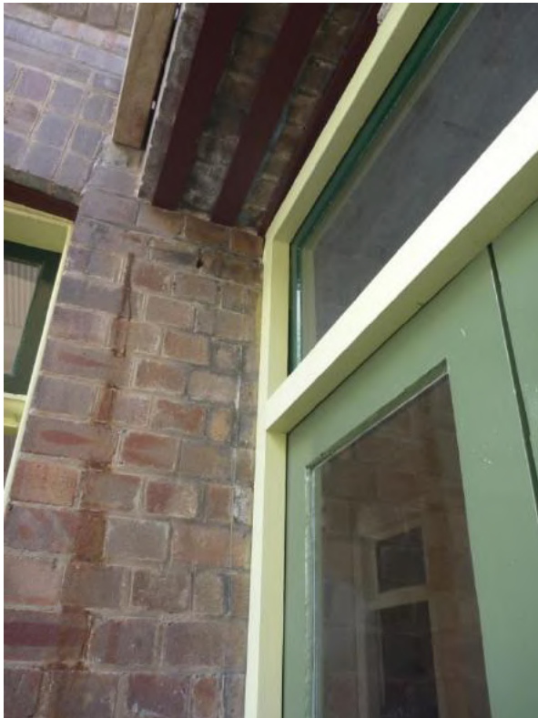
Figure 1.48 Fanlight and arch bars above exterior door—46/46–56 Gloucester Street. (Source: GML Heritage, July 2016)
