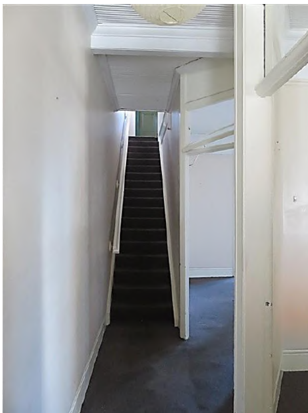
Figure 16.18 Entrance hall (space 1.1) showing stair (space 1.7), ripple iron ceiling and beam over where walls are splayed—entrances to spaces 1.2 and 1.3 on right—56C / 46–56 Gloucester Street. (Source: GML Heritage, July 2016)
