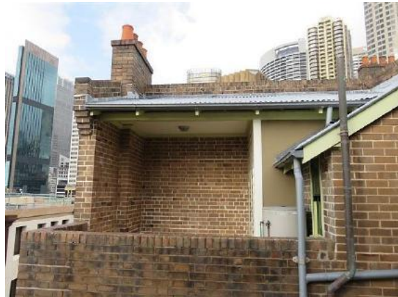
Figure 14.13 Roof terrace viewed from Flat 54C, showing area covered by skillion roof, chimney over rear wing and brick balustrade to roof terrace—56A / 46–56 Gloucester Street. (Source: GML Heritage, July 2016)
