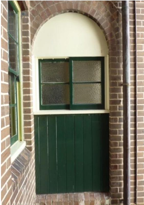
Figure 3.54 Round-arched window of the former rear porch on the southern elevation showing modern infill. Also original brick round arch and chamfered window sill—48 / 46–56 Gloucester Street. (Source: GML Heritage, May 2016)
