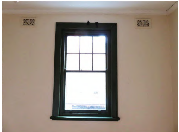
Figure 10.47 Timber double hung sash window to dining room (space 2.4)—54A / 46–56 Gloucester Street. (Source: GML Heritage, July 2016)
