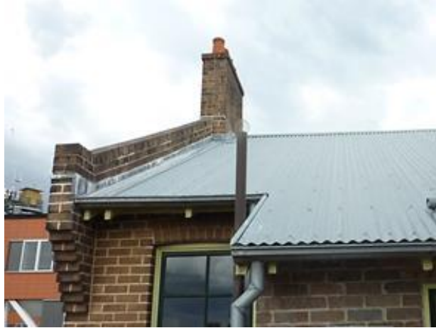
Figure 4.18 Common brick chimney stacks (Flat 56C). (Source: GML 2015)
