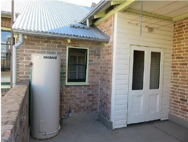
Figure 16.14 Rear wall of the flat opening onto the roof terrace (space E.1), showing recent weatherboard wall and pair of half glazed doors opening onto terrace and exposed rafters to eaves—56C / 46–56 Gloucester Street. (source: GML Heritage, July 2016)
