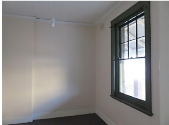
Figure 12.21 Front bedroom (space 1.2) showing timber double hung sash window with six pane upper sash and single pane lower sash, cement run skirting, ripple iron ceiling and moulded timber cornice. There is a chimney flue running up the southern wall—54C / 46–56 Gloucester Street. (Source: GML Heritage, July 2016)
