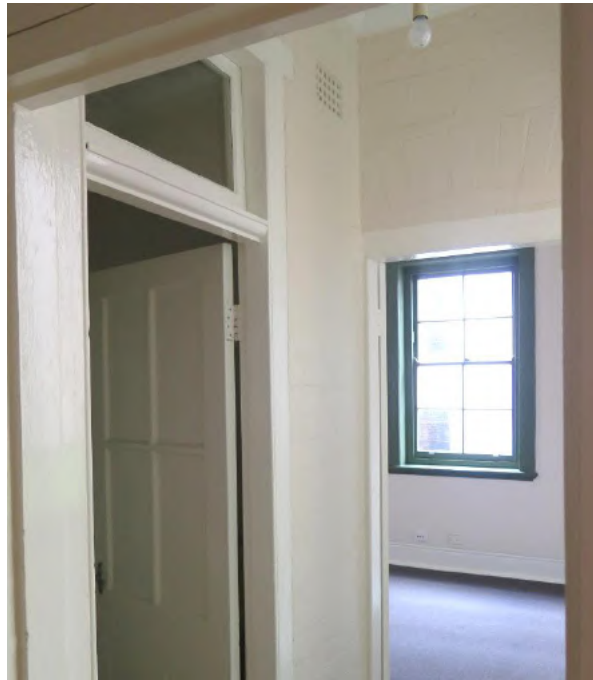
Figure 11.21 Infilled former rear porch opening (space G.4), with unrendered brick walls, timber door with fanlight to bathroom—54B / 46–56 Gloucester Street (Source: GML Heritage, July 2016)
