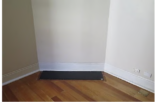
Figure 3.23 The original corner fireplace with concrete hearth is blocked in the living room (space G.3). Note original cement run skirtings have been replicated across new section—48 / 46–56 Gloucester Street. (Source: GML Heritage, May 2016)
