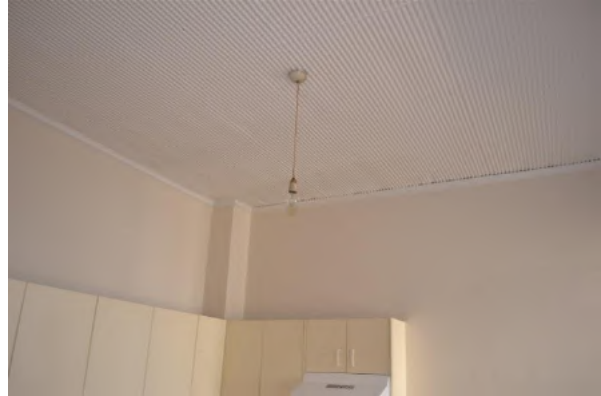
Figure 1.43 Original ripple iron ceiling in the kitchen (space LG.2)—46/46–56 Gloucester Street. (Source: GML Heritage, July 2016)
