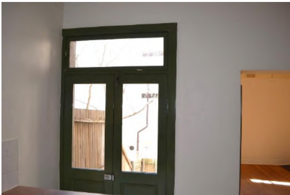
Figure 1.44 Half-glazed timber door with fanlight above from kitchen (space LG.2) to rear yard (space E.2)—46/46–56 Gloucester Street. (Source: GML Heritage, July 2016)
