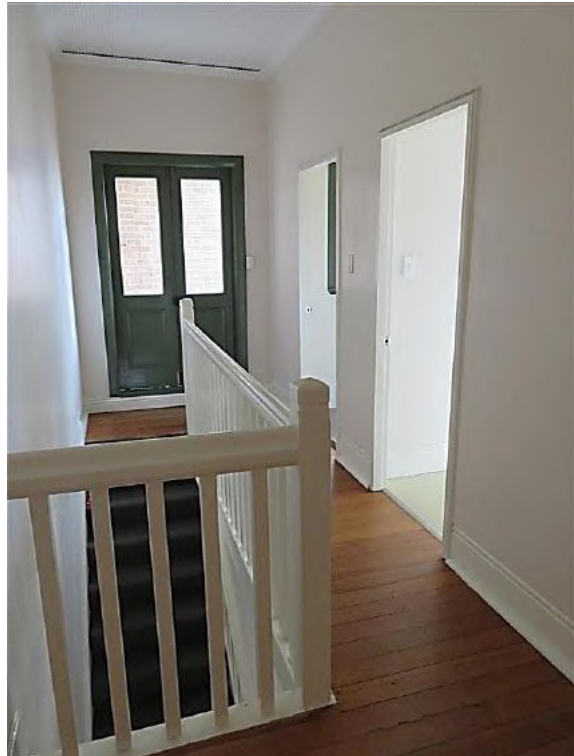
Figure 12.37 Second floor landing (space 2.1) looking east, showing timber balustrade around stair with moulded handrail, square balusters and chamfered newel posts, cement rendered skirting to the wall. The half glazed timber doors to the roof terrace are late twentieth century—54C / 46–56 Gloucester Street. (Source: GML Heritage, July 2016)
