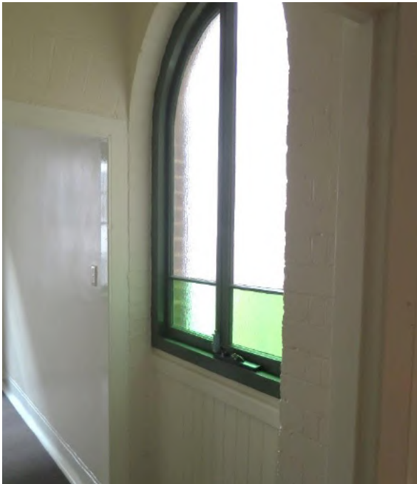
Figure 11.20 Infilled former rear porch opening (space G.4), with unrendered brick walls, arched modern casement window and modern T&G boarding below—54B / 46–56 Gloucester Street (Source: GML Heritage, July 2016)
