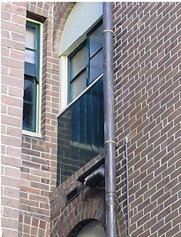
Figure 4.16 Round-arched opening and sliding sash window added to the former rear porch on the southern elevation. Also late 20th century copper plumbing additions—48A / 46–56 Gloucester Street. (Source: GML Heritage, May 2016)
