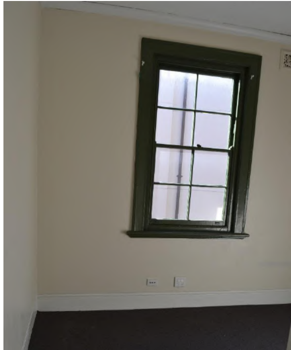
Figure 6.29 Rear bedroom (space 1.6) showing timber double hung sash window and cement run skirting—50A / 48–56 Gloucester Street. (Source: GML Heritage, July 2016)
