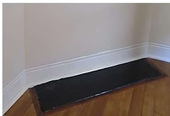
Figure 3.17 Timber floor and original corner fireplace, concrete hearth blocked off and rendered and skirted in the front bedroom (space G.2)—48 / 46–56 Gloucester Street. (Source: GML Heritage, May 2016)
