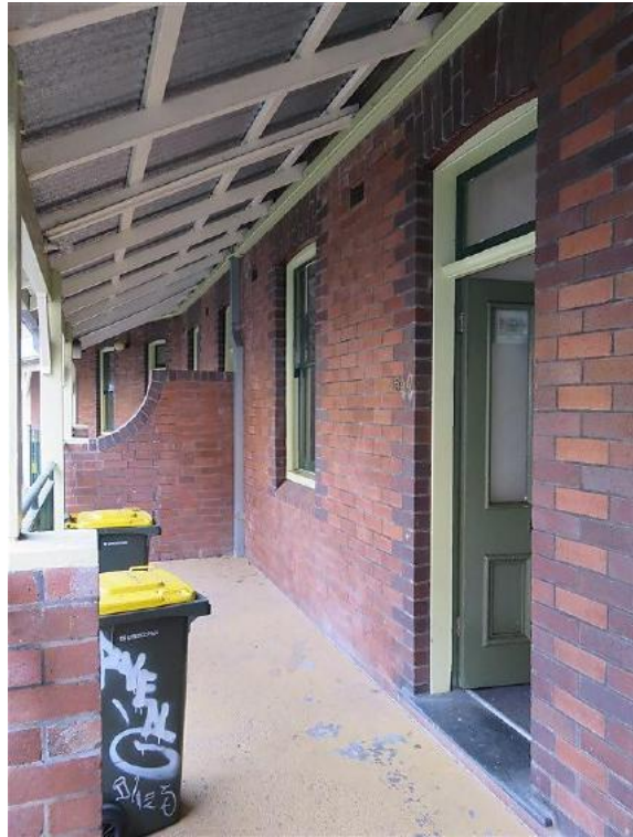
Figure 10.7 Front façade of flat 54A showing facebrick external wall with contrasting brick surround to window and door openings—54A / 46–56 Gloucester Street. (Source: GML Heritage, July 2016)
