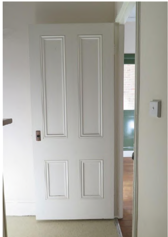
Figure 4.32 Replica four-panel internal door as used in the 1988 renovations (second floor level, Flat 54A). (Source: GML 2016)
