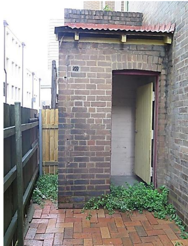
Figure 9.37 External WC (space E.3) with skillion roof, timber boarded door and brick parapet—54 / 46–56 Gloucester Street. (Source: GML Heritage, July 2016)
