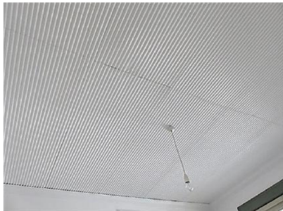
Figure 14.32 Ripple iron ceiling in the rear bedroom with moulded timber cornice (space 1.6)—56A / 46–56 Gloucester Street. (Source: GML Heritage, July 2016)
