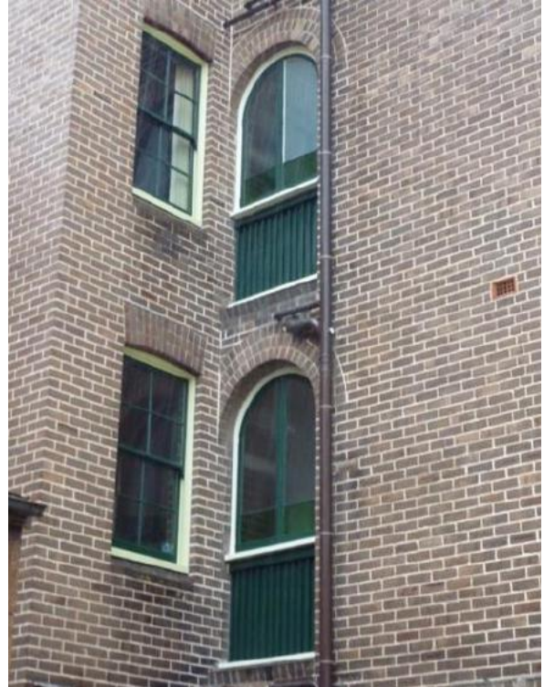
Figure 4.14 Arched openings to former porches in the rear wings with infill balustrades and windows c1988 (Flat 54B, first floor level). Note the triple brick arched heads to openings. (Source: GML 2015)
