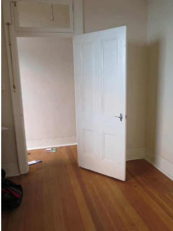
Figure 11.14 Four-panel timber door with fanlight above and reproduction mechanism between front bedroom (space G.2) and entry (space G.1)—54B / 46–56 Gloucester Street (Source: GML Heritage, July 2016)
