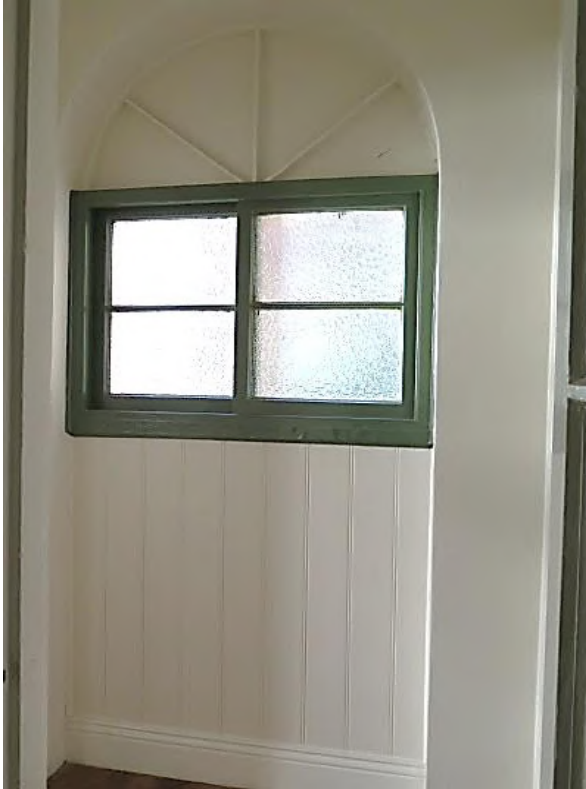
Figure 4.34 Infilled former rear porch opening (space 1.4), with modern horizontal sliding sash window and T&G boarding and modern skirting below—48A / 46–56 Gloucester Street. (Source: GML Heritage, May 2016)
