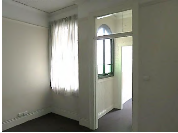
Figure 10.25 Living room (space 1.3) showing the original opening through to space 1.4. The frame and architrave are original. The door is missing and the fanlight has been replaced with fixed glazing—54A / 46–56 Gloucester Street. (Source: GML Heritage, July 2016)
