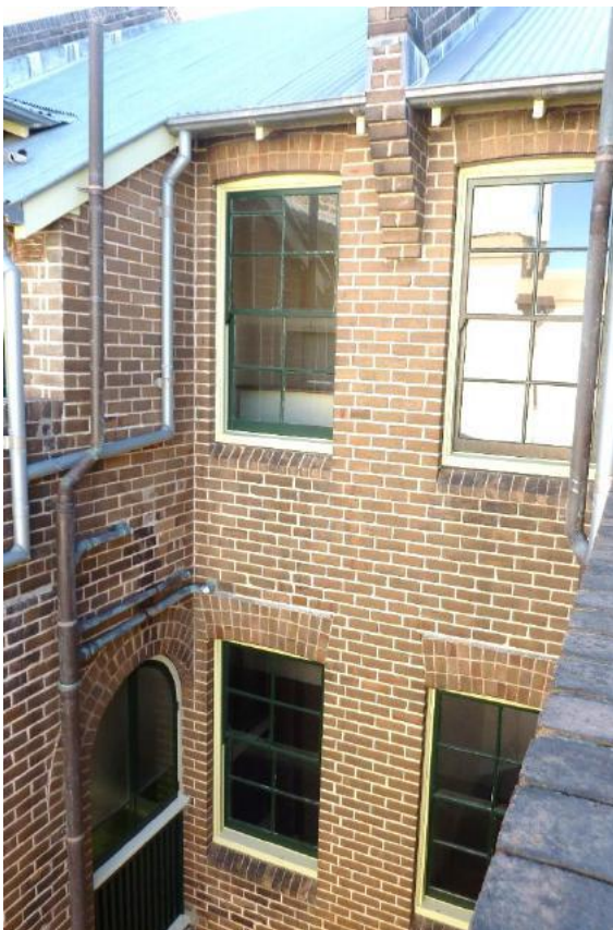
Figure 6.12 Brick rear wing (first and second floor levels), and typical segmental brick arched heads over openings—50A / 48–56 Gloucester Street. (Source: GML Heritage, July 2016)
