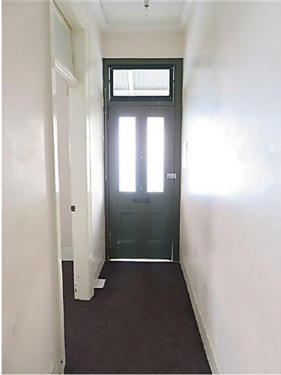
Figure 12.18 Entrance hall (space 1.1), looking towards front door, showing the ripple iron ceiling, moulded timber cornice and cement run skirting—54C / 46–56 Gloucester Street. (Source: GML Heritage, July 2016)
