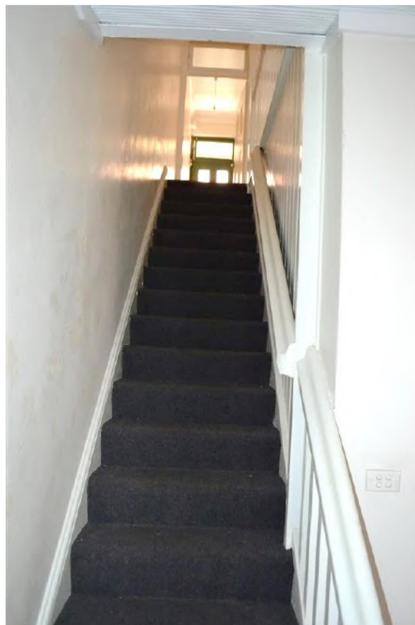
Figure 5.31 The stair (space G.7) showing the original timber handrail and timber boarded wall—50 / 46–56 Gloucester Street. (Source: GML Heritage, June 2016)
