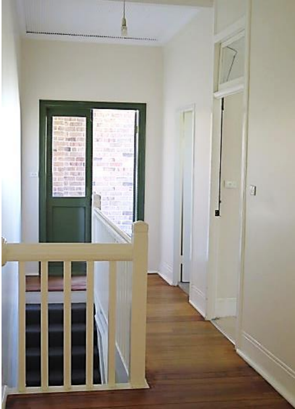
Figure 4.42 Hall (space 2.1) showing timber balustrade and modern French door to terrace (space E.1) and original cement run skirtings—48A / 46–56 Gloucester Street. (Source: GML Heritage, November 2015)
