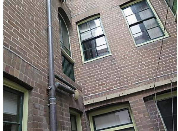
Figure 9.35 Rear wing and rear façade showing copper service pipes and later porch opening infill—54 / 46–56 Gloucester Street. (Source: GML Heritage, July 2016)
