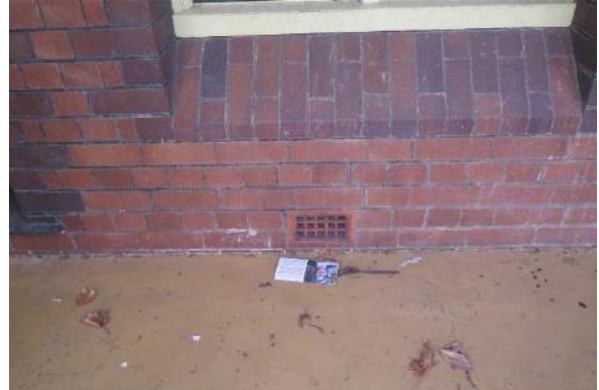
Figure 15.11 The front yard (space E.1) showing the chamfered brick sill to the window, terracotta wall vent as typical in all external spaces and concrete yard paving—56B / 46–56 Gloucester Street. (Source: GML Heritage, July 2016)
