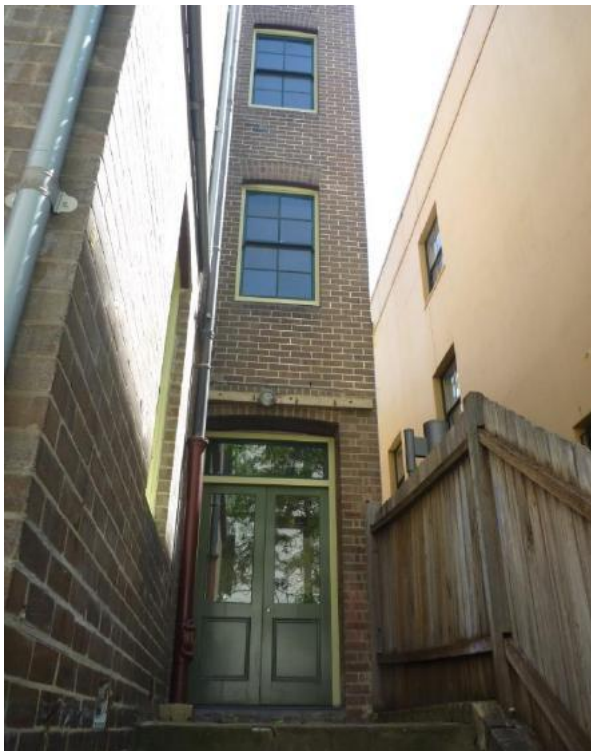
Figure 1.56 Rear façade, showing the northern timber fence, window to living room (space G.3) and half-glazed timber double doors to the kitchen (space LG.2)—46/46–56 Gloucester Street. (Source: GML Heritage, July 2016)
