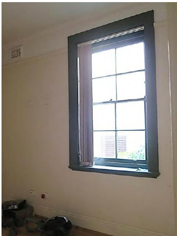
Figure 7.22 The rear bedroom (space G.6) showing timber floor and original cement run skirtings, decorative plaster wall vent, picture rail and timber double-hung sash window with its original architrave and sill board—52 / 46–56 Gloucester Street. (Source: GML Heritage, July 2016)
