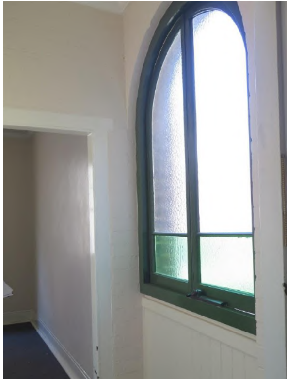
Figure 15.25 Infilled former rear porch opening (space G.4). The original arched opening has been infilled with vertical boarding and casement windows—56B / 46–56 Gloucester Street. (Source: GML Heritage, July 2016)
