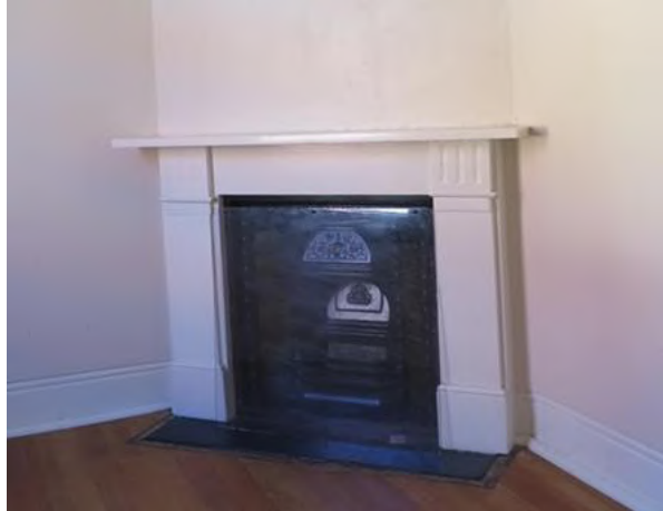
Figure 4.50 The overpainted stone surround (second floor level, Flat 54A). (Source: GML 2016)
