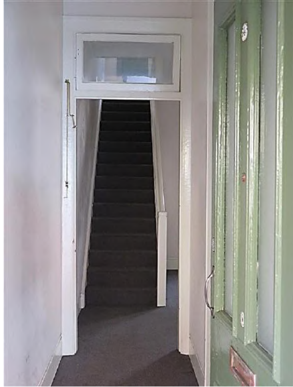
Figure 12.19 View of entrance hall (space 1.1) from front door, showing original door frame, with fanlight above, leading to the living room (space 1.3) and stair (space 1.7). The door is missing—54C / 46–56 Gloucester Street. (Source: GML Heritage, July 2016)
