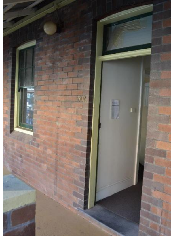
Figure 6.7 Door and fanlight—50A / 48–56 Gloucester Street, showing the contrasting brick surround and segmental arch (supported on a metal arch bar) to the opening. (Source: GML Heritage, July 2016)
