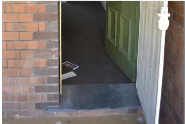
Figure 2.11 Original slate threshold to front door—46A/46–56 Gloucester Street. (Source: GML Heritage, July 2016)
