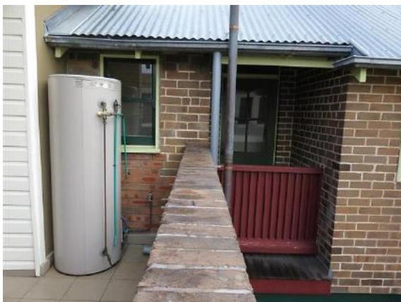
Figure 10.14 Rear elevation of flat 54A showing the recessed balcony off the kitchen (space 2.3) and new brickwork and window to the laundry (space 2.2)—54A / 46–56 Gloucester Street. (Source: GML Heritage, July 2016)
