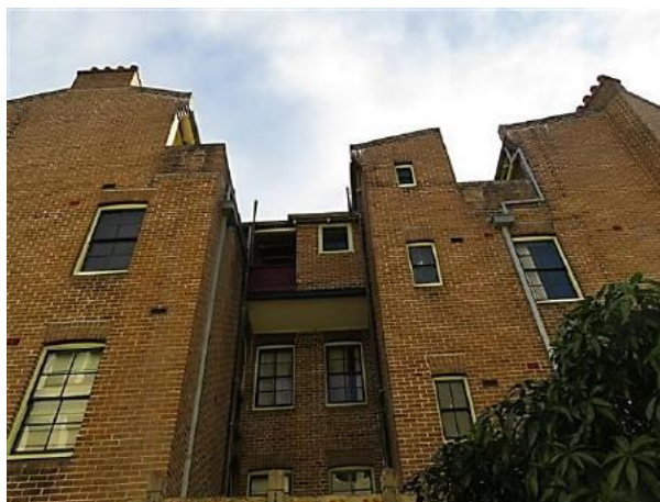
Figure 8.11 Rear elevation of flat 54A (left) and 52A (right) showing common brick walls, projecting landing bay with ripple iron cladding to underside, original double hung sash windows and skillion roofed sections of roof terrace—46 / 56 Gloucester Street. (Source: GML Heritage, July 2016)
