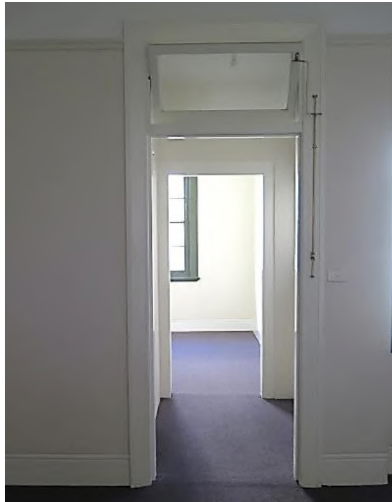
Figure 4.33 Doorway with original transom light above and reproduction mechanism between the living room (space 1.3) and the former rear porch (space 1.4)—48A / 46–56 Gloucester Street. Note original door is missing. (Source: GML Heritage, May 2016).
