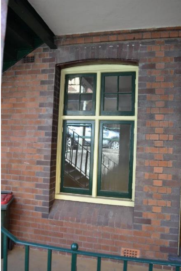
Figure 1.10 Detail of western elevation to Flat 46 at ground-floor level, showing original casement window with—46/46–56 Gloucester Street. (Source: GML Heritage, July 2016)
