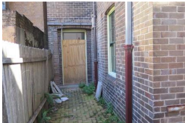
Figure 15.49 Rear yard with brick paving (space E.2), timber fencing and boarded up double doors—56B / 46–56 Gloucester Street. (Source: GML Heritage, July 2016)
