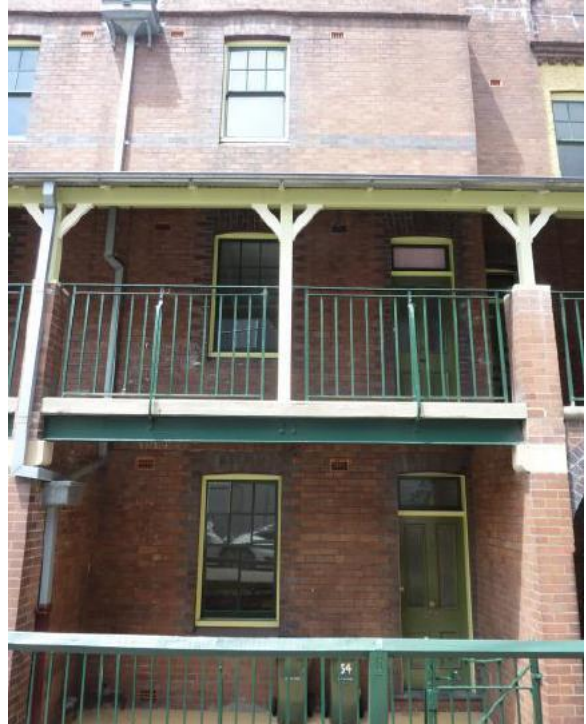
Figure 4.6 Detail of the first floor verandahs with steel beams spanning between brick piers, concrete slab floor, square timber posts and brackets, steel balustrades and stays and exposed rafters to the eaves. Note original double-hung windows with six-pane upper sashes to the Gloucester Street facade. (Source: GML 2015)
