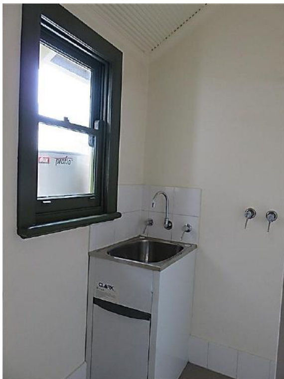
Figure 12.40 Laundry (space 2.2) showing modern refit and timber double hung window—54C / 46–56 Gloucester Street. (Source: GML Heritage, July 2016)
