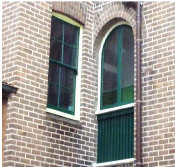
Figure 5.45 Round arched window of the infilled former rear porch—50 / 46–56 Gloucester Street. (Source: GML Heritage, July 2016).
