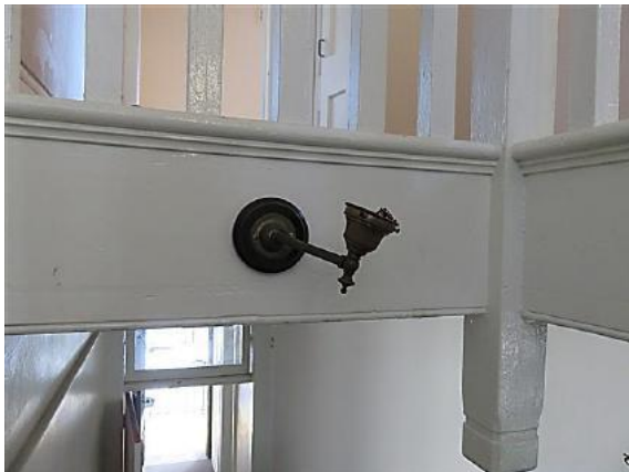
Figure 14.35 Early gaslight fitting over stair (space 1.7) and detail of bottom of newel post—56A / 46–56 Gloucester Street. (Source: GML Heritage, July 2016)
