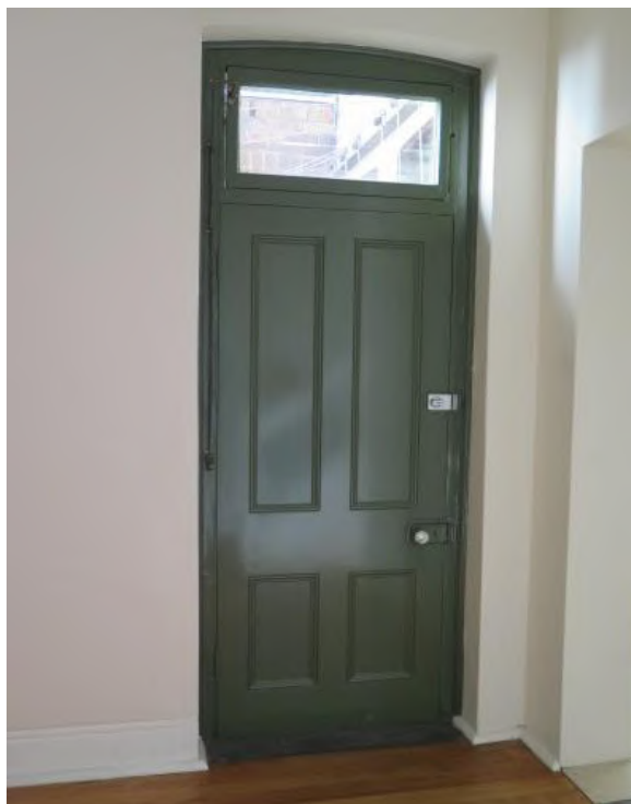
Figure 3.39 Four-panel bolection moulded timber external door with fanlight in the dining room (space LG.1)—48 / 46–56 Gloucester Street. (Source: GML Heritage, May 2016)
