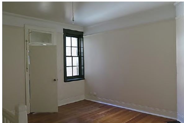
Figure 3.21 The living room (space G.3) showing cement run skirtings, timber cornice, timber double-hung sash window—48 / 46–56 Gloucester Street. (Source: GML Heritage, May 2016)
