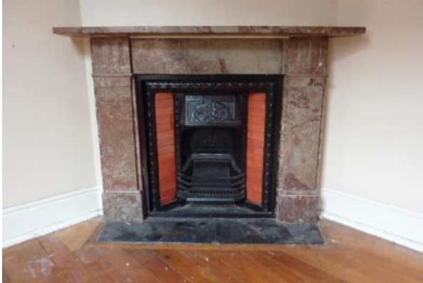
Figure 4.49 A marble chimney piece with cast-iron and tiled grate, and painted concrete hearth (second floor level, Flat 56A). (Source: GML 2015)
