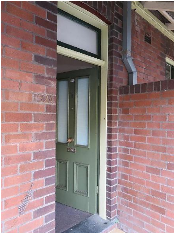
Figure 8.8 Four panel entrance door with bolection moulds, wired glass to upper panels, fanlight over and slate threshold—52A / 46–56 Gloucester Street. (Source: GML Heritage July 2016)
