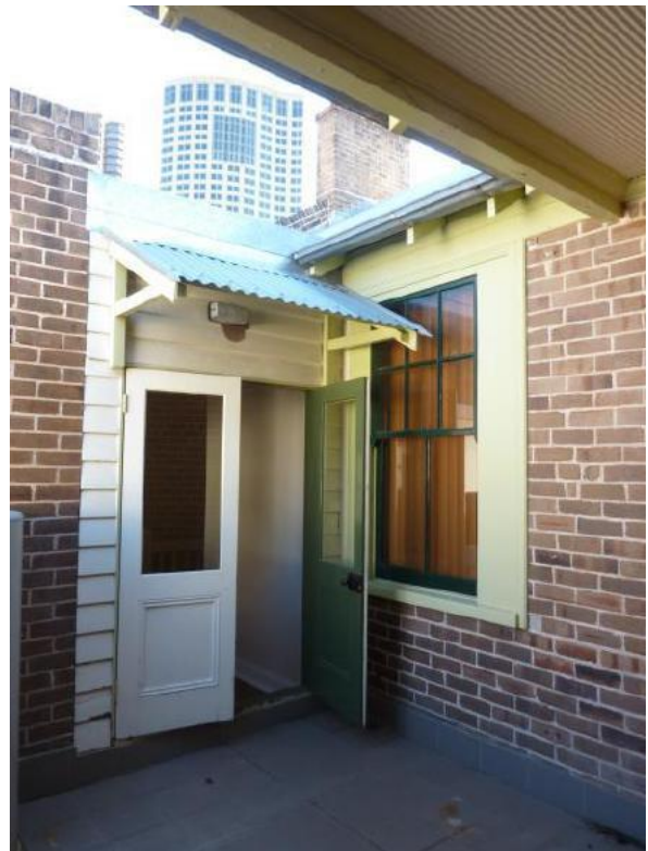
Figure 4.16 Weatherboard enclosure to the former roof top balcony with awning c1988 and six-over-two sash window (window matches the detail of the front ground-floor window of Flat 56) (Flat 52A). (Source: GML 2015)
