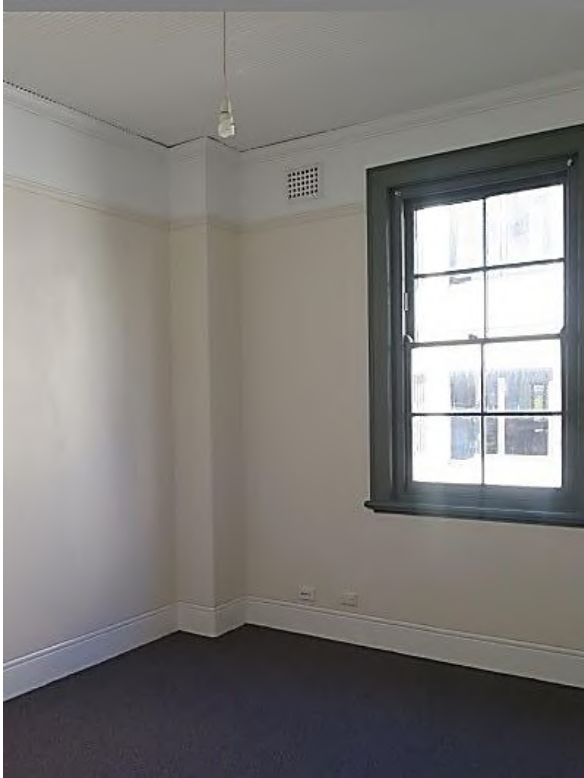
Figure 4.38 Rear bedroom (space 1.6), showing modern carpeted floor (over original timber), original skirtings, ripple iron ceiling, cornice, picture rail, wall vent and timber double-hung sash window—48A / 46–56 Gloucester Street. (Source: GML Heritage, May 2016)
