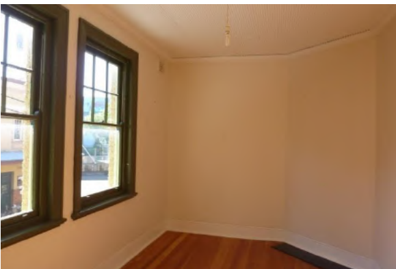
Figure 2.47 Front room on second floor (space 2.4) showing the original double hung window, ripple iron ceiling and timber floor)—46A / 46–56 Gloucester Street. (Source: GML Heritage, July 2016)
