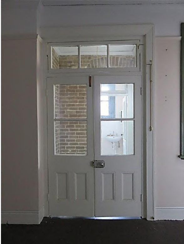
Figure 8.30 Half glazed panel doors with fanlight over, leading from the living room (space 1.3) to the rear porch (space 1.4)—52A / 46–56 Gloucester Street. (Source: GML Heritage, July 2016).
