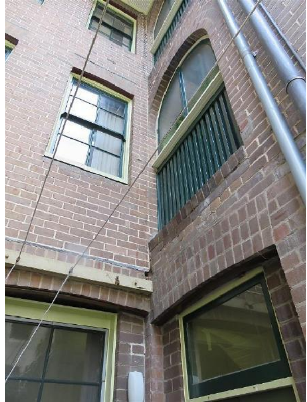
Figure 7.39 Brick arch and iron lintel bar over the rear door fanlight, also showing laundry hoist fixings above the window and brick arched head—52/46–56 Gloucester Street. (Source: GML Heritage, June 2016)
