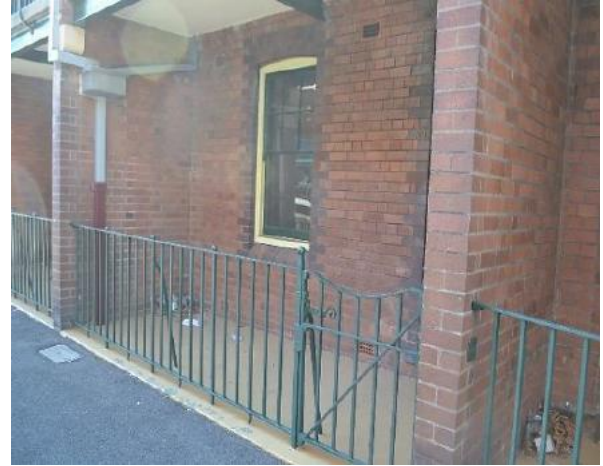
Figure 5.7 The front façade—50 / 46–56 Gloucester Street, showing external walls, projecting party walls with sandstone bolsters, wrought iron fence with square pales, wrought iron gates and the front yard (space E.1) (Source: GML Heritage, November 2015)
