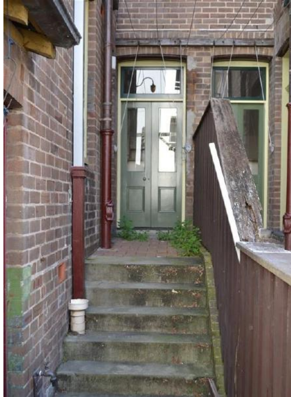
Figure 5.43 Exterior walls of the rear wing showing concrete steps, original cast iron and modern stainless and copper downpipes, and terracotta wall vents (space E.2)—50 / 46–56 Gloucester Street. (Source: GML Heritage, June 2016)
