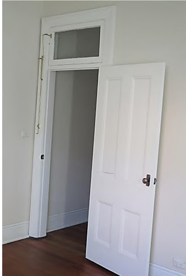
Figure 4.55 Original four-panel sunk moulded timber door to dining room (space 2.4), with original fanlight above—48A / 46–56 Gloucester Street. (Source: GML Heritage, May 2016)
