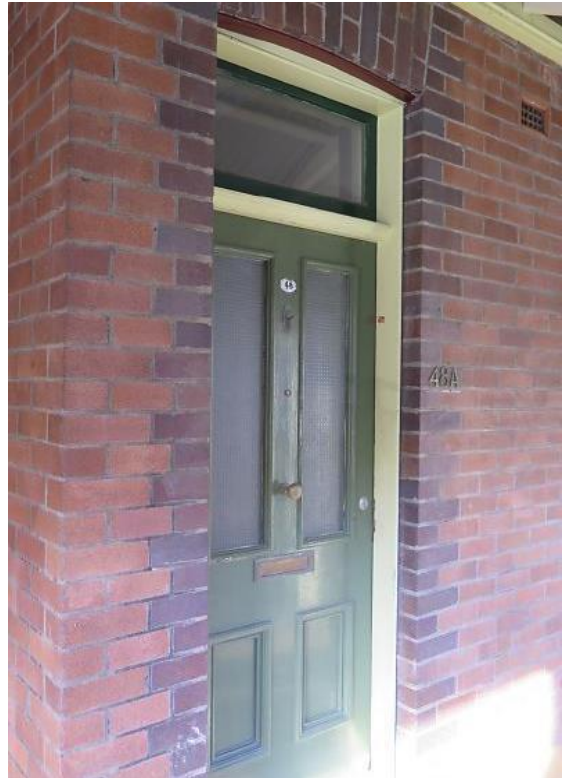
Figure 4.9 Four-panel front door with bolection moulds to bottom panels and textured and wired glass to upper panels, dark brick surrounds, arched head and enamelled number plate—48A / 46–56 Gloucester Street. (Source: GML Heritage, May 2016)
