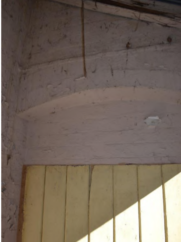
Figure 1.54 External store (space E.3) showing the ledgered and sheeted timber door and arched detail brick on the internal wall—46/46–56 Gloucester Street. (Source: GML Heritage, July 2016)
