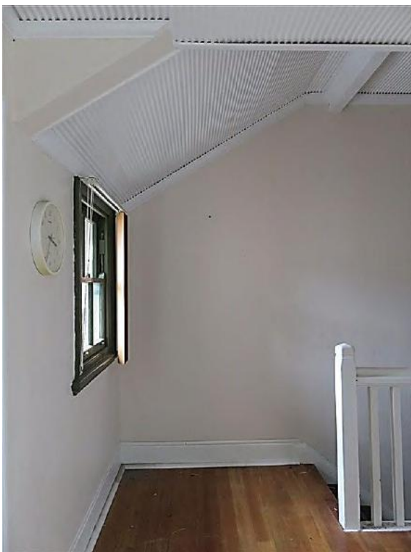
Figure 8.40 Second floor landing (space 2.1) showing the raked ripple iron ceiling, cross beam, timber floor and cement skirtings to the projecting landing space, with original timber double hung window—52A / 46–56 Gloucester Street. (Source: GML Heritage, July 2016)
