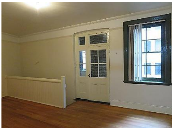
Figure 7.14 Living room (space G.3) showing timber flooring, cement run skirtings and picture rail. The timber stair with its boarded and newel post runs along the eastern wall. The half-glazed door with its side light and fanlights, and the timber double-hung sash window are original—52 / 46–56 Gloucester Street. (Source: GML Heritage, July 2016)
