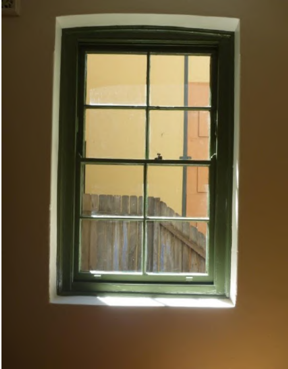
Figure 4.33 Lower ground floor level timber double-hung sash window with rendered reveals (lower ground floor level, Flat 46). (Source: GML 2015)
