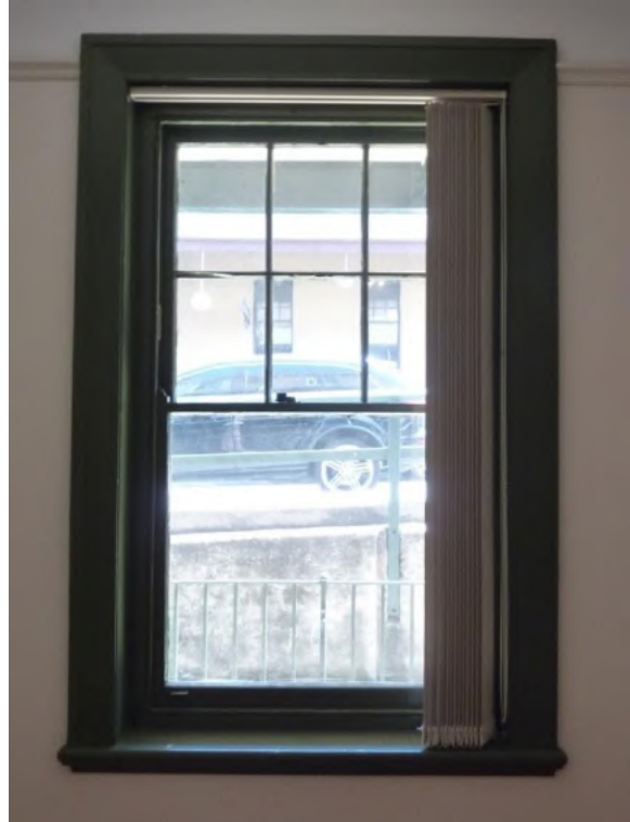
Figure 4.34 Typical double-hung window in the western elevation, with original timber architrave, sill board and moulding (ground floor level, Flat 48). (Source: GML 2015)
