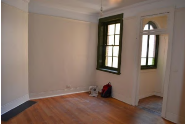
Figure 1.22 Living room (space G.3) showing timber floors, cement run skirting, moulded timber picture rail and plasterboard ceiling and cement hearth to the original fireplace (blocked up)—46/46–56 Gloucester Street. (Source: GML Heritage, July 2016)
