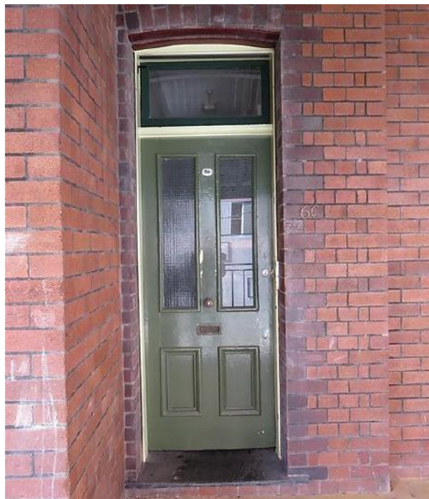
Figure 16.9 Four-panel entrance door with bolelection moulds, wired glass to upper panels and fanlight over, slate threshold and contrasting brick trim—56C / 46–56 Gloucester Street. (Source: GML Heritage, July 2016)
