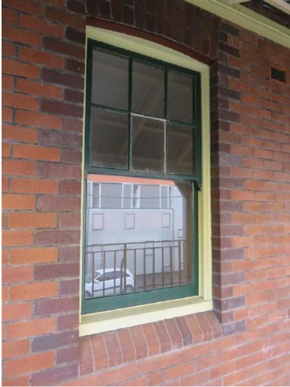
Figure 12.10 Original double hung sash window with chamfered brick sill—54C / 46–56 Gloucester Street. (Source: GML Heritage, July 2016)
