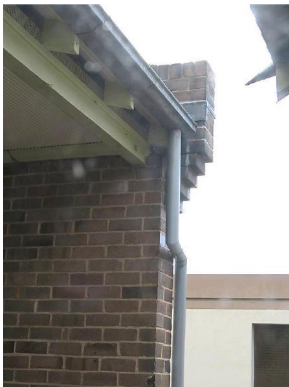
Figure 8.13 Skillion roof over the roof terrace (space E.1) with corbelled brick gable parapet detail, ripple iron ceiling, timber cornice, exposed rafters and modern guttering—52A / 46–56 Gloucester Street. (Source: GML Heritage, July 2016)
