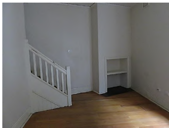
Figure 7.25 Original stair at lower ground-floor level with closed string, simple square balusters and newel post and moulded handrail. Later shelving in the original fireplace—52 / 46–56 Gloucester Street. (Source: GML Heritage, July 2016)
