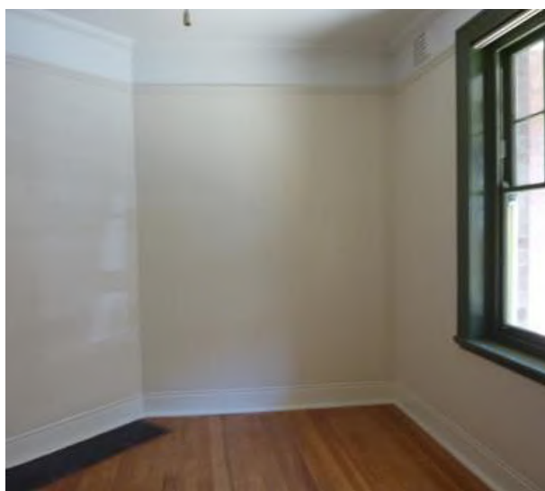
Figure 4.64 The front bedroom (second floor level, Flat 54) showing the concrete hearth of blocked up fireplace, rendered wall finishes to the dado level with set plaster above, rendered cement skirting, timber picture rail, cornice and double-hung sash window. (Source: GML 2015)
