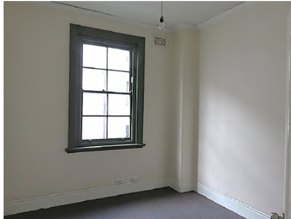
Figure 10.35 Rear bedroom (space 1.6) showing the original timber double hung window with original architraves, sill board and moulding, ripple iron ceiling and decorative plaster wall vent—54A / 46–56 Gloucester Street. (Source: GML Heritage, July 2016)
