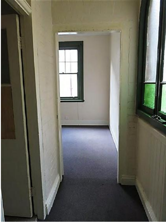
Figure 12.26 Space 1.4 (former rear porch) looking through to space 1.5 (rear bedroom). The floor has been raised and the timber skirting is recent—54C / 46–56 Gloucester Street. (Source: GML Heritage, July 2016)
