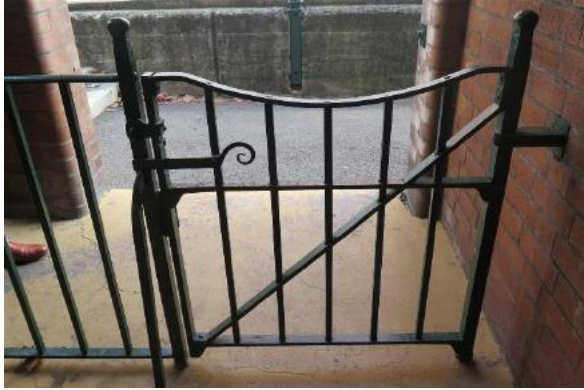
Figure 15.10 Detail of the wrought iron gate with original gate latch—56B / 46–56 Gloucester Street. (Source: GML Heritage, July 2016)
