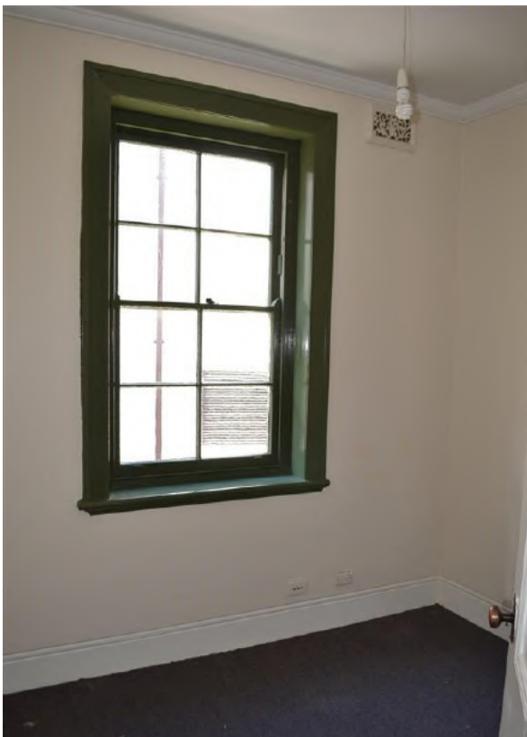
Figure 5.28 Rear bedroom (space G.6) showing the timber double hung window, cement render skirting and decorative plaster wall vent—50 / 46–56 Gloucester Street. (Source: GML Heritage, June 2016)
