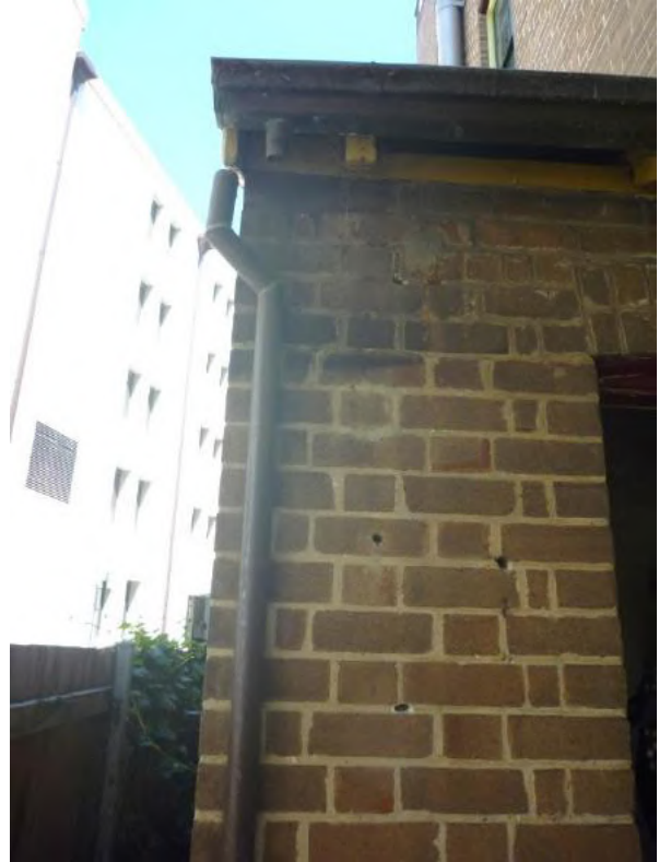
Figure 1.55 Failed guttering and down pipe to the roof of the external store (space E.3)—46/46–56 Gloucester Street. (Source: GML Heritage, July 2016)
