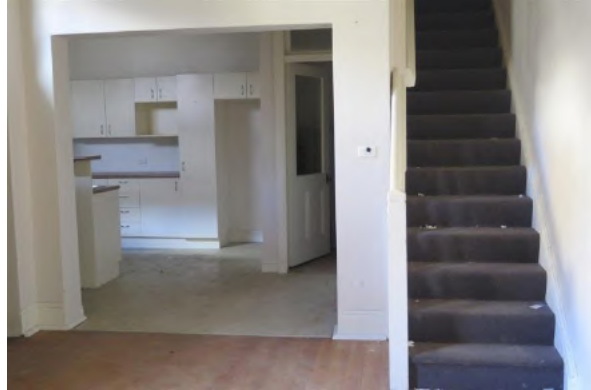
Figure 15.39 Lower ground-floor level showing original timber stair, large opening cut through to kitchen (space LG.2) and enclosure to create laundry under stairs c1988 (space LG.3)—56B / 46–56 Gloucester Street. (Source: GML Heritage, July 2016)
