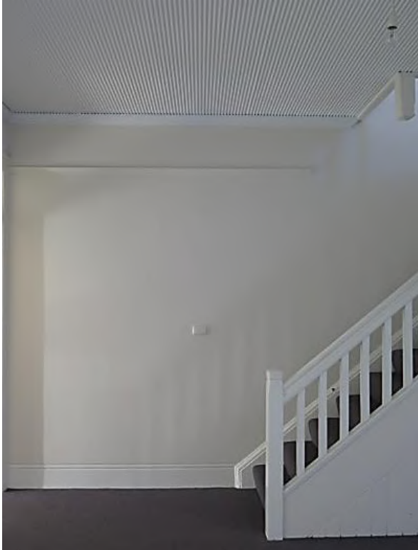
Figure 4.30 Living room (space 1.3) showing half picture rail, T&G timber boards to staircase and ripple iron ceiling. Walls with painted set plaster above dado, cement render below dado—48A / 46–56 Gloucester Street. (Source: GML Heritage, May 2016)
