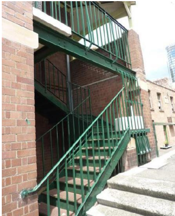
Figure 4.7 Detail of the exterior steel staircase to the first floor at the southern end of the building, with original handrail and iron balustrade, and cast-iron treads and risers. Note sandstone bolsters supporting the steelwork. (Source: GML 2015)
