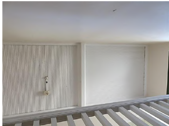
Figure 14.36 Second floor landing ceiling (space 2.1) showing the ripple iron ceiling laid in different directions on either side of beam—56A / 46–56 Gloucester Street. (Source: GML Heritage, July 2016)
