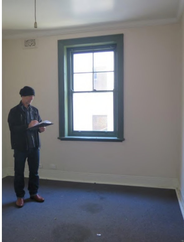
Figure 15.31 Rear bedroom (space G.6) showing timber double hung sash window, modern carpet over original timber floor boards, cement rendered skirting and decorated wall vent—56B / 46–56 Gloucester Street. (Source: GML Heritage, July 2016)
