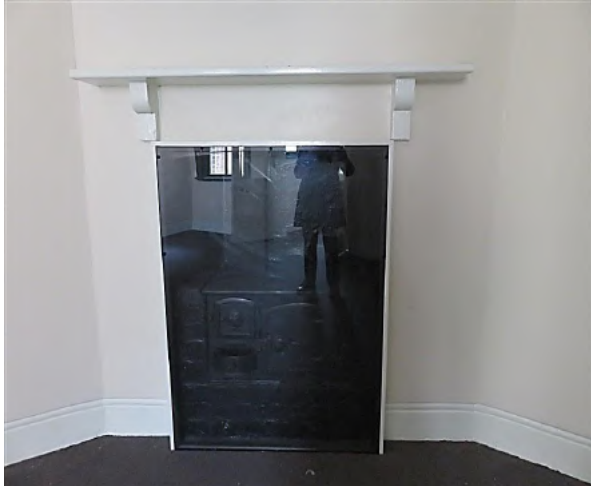
Figure 8.26 Original mantel shelf over fireplace in space 1.3 supported on corbelled brick brackets. A cast iron range is set within the fireplace behind the Perspex screen (see Figure 8.27 )—52A / 46–56 Gloucester Street. (Source: GML Heritage, July 2016)
