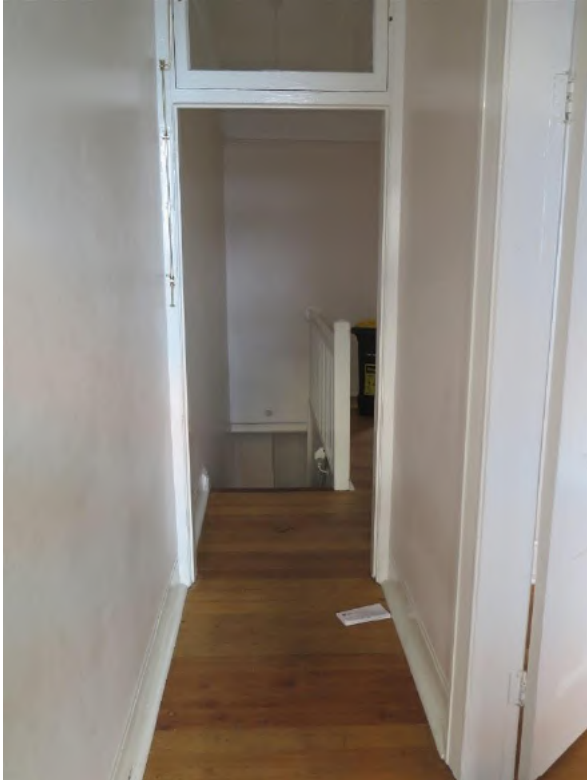
Figure 11.10 Entry (space G.1 showing timber floor, cement run skirtings, and timber door frame with fanlight to the living room—54B / 46–56 Gloucester Street. (Source: GML Heritage, July 2016)
