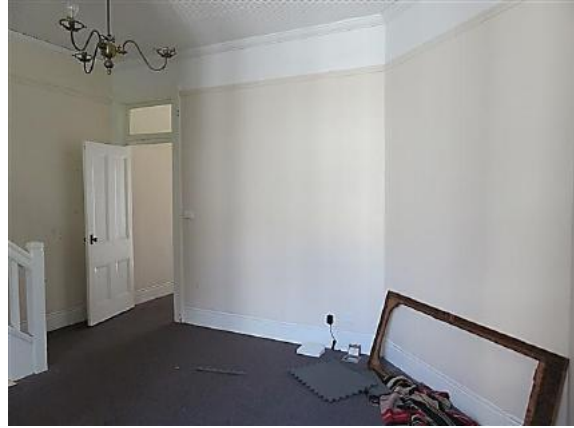
Figure 14.21 Living room (space 1.3) showing cement rendered skirtings, timber picture rail, ripple iron ceiling and moulded timber cornice. Original door and fanlight with original architraves—56A / 46–56 Gloucester Street. (Source: GML Heritage, July 2016)
