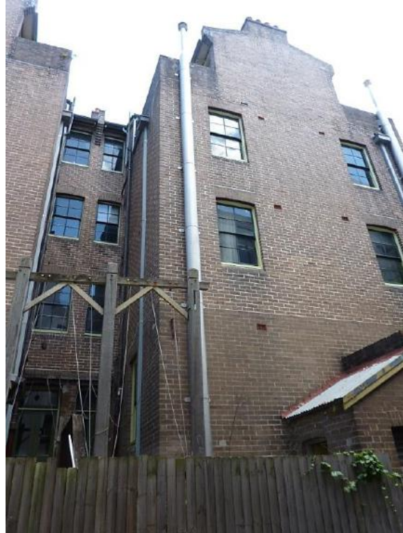
Figure 4.15 Exterior walls of the rear wing in common brick, showing reconstructed garbage chute and roof terrace parapet, shared chimney, skillion roof and steel downpipes—48A / 46–56 Gloucester Street. (Source: GML Heritage, May 2016)
