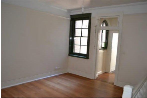
Figure 5.18 The living room (space G.3) showing cement run skirtings, timber cornice, timber double-hung sash window—50 / 46–56 Gloucester Street. (Source: GML Heritage, June 2016)
