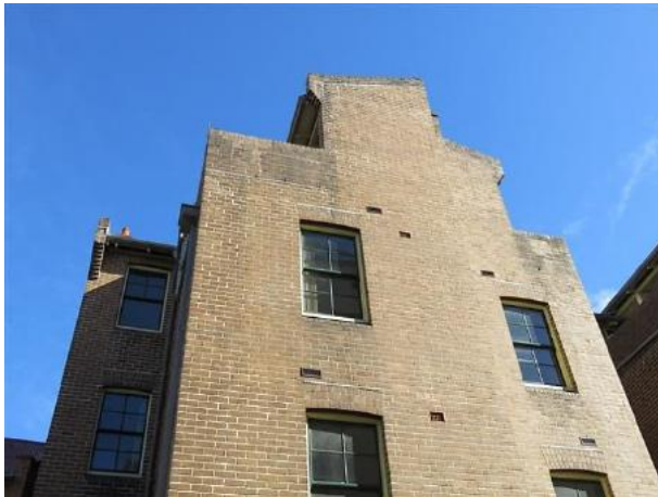
Figure 16.12 Rear elevation of Flat 56C (left) and 56A (right), showing arched brick heads to window openings and wall enclosing roofed over area of roof terrace—56C / 46–56 Gloucester Street. (Source: GML Heritage, July 2016)
