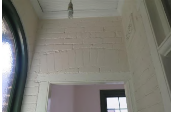
Figure 4.42 Painted unrendered brick walls to enclosed porch (first floor level, Flat 54A). (Source: GML 2016)
