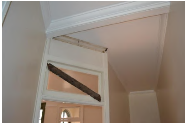
Figure 1.21 Ceiling of entry hall (space G.1) showing beaded timber beam and cornices, lightweight concrete wall, fanlight and architrave—46/46–56 Gloucester Street. (Source: GML Heritage, July 2016)
