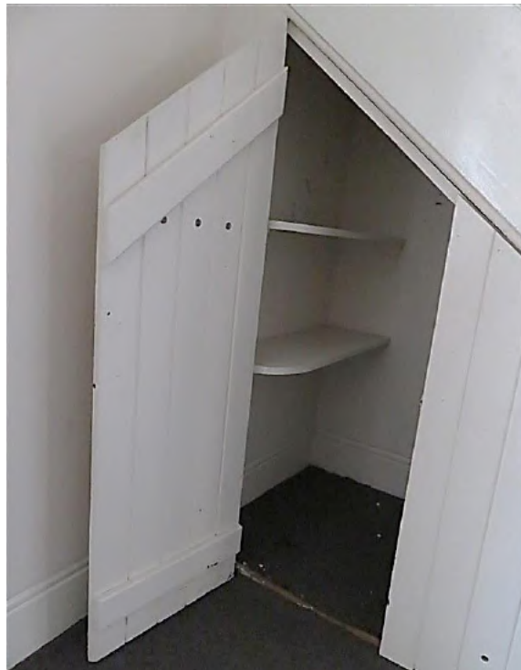
Figure 10.27 Cupboard under the stair (space 1.3) with v-jointed boarding, ledged and sheeted timber door and timber shelves—54A / 46–56 Gloucester Street. (Source: GML Heritage, July 2016)
