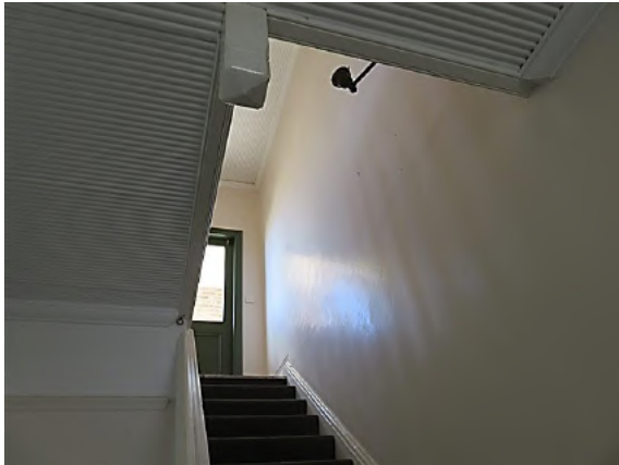
Figure 14.33 Living room (space 1.3) showing the ripple iron ceiling and newel post projecting below stair—56A / 46–56 Gloucester Street. (Source: GML Heritage, July 2016)
