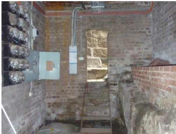
Figure 4.23 View of the south end of service tunnel, showing a non-original steel stair leading up to the original access opening in the south wall. (Source: GML 2015)
