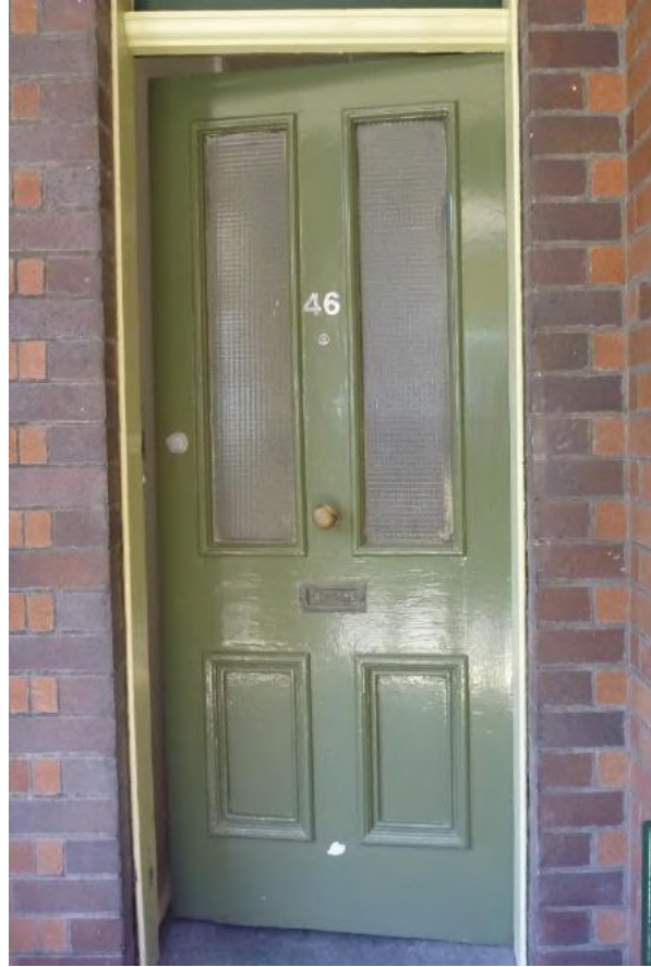
Figure 1.11 Timber four panel bolection moulded door with wired glass to the upper panels—46/46–56 Gloucester Street. (Source: GML Heritage, July 2016)
