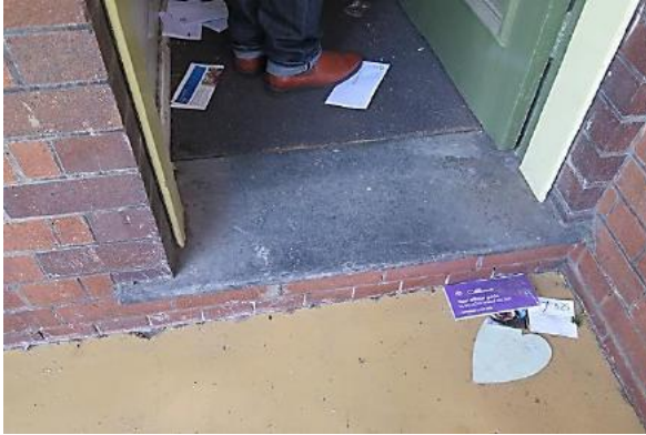
Figure 13.10 Original slate threshold to front door—56 / 46–56 Gloucester Street. (Source: GML Heritage, May 2016)
