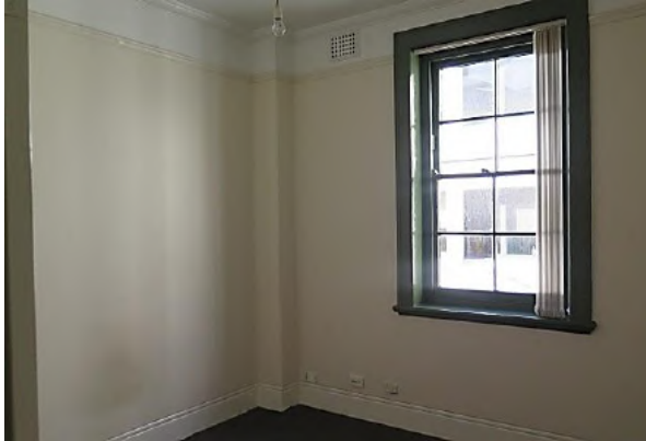
Figure 3.30 The rear bedroom (space G.6) showing carpeted floor, and original cement run skirtings, grille pattern wall vent, picture rail and timber double-hung sash window—48 / 46–56 Gloucester Street. (Source: GML Heritage, April 2016)
