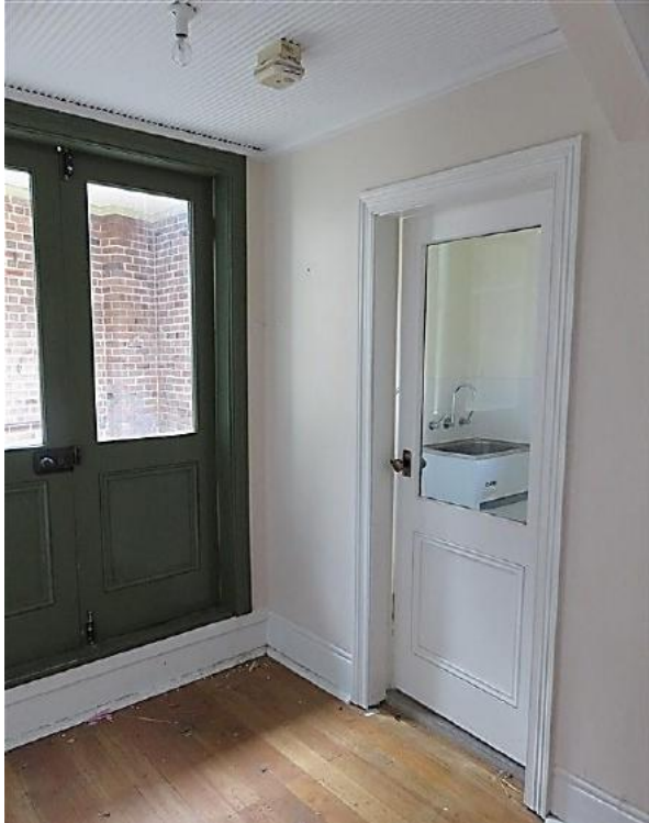
Figure 8.42 Second floor landing (space 2.1) showing the cement rendered skirting and later half glazed doors to the roof terrace and laundry—52A / 46–56 Gloucester Street. (Source: GML Heritage, July 2016)
