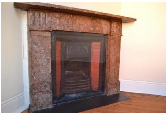
Figure 6.45 Fireplace (space 2.4) with early cast iron grate with tiled sides, and red marble chimney piece—50A / 48–56 Gloucester Street. (Source: GML Heritage, July 2016)
