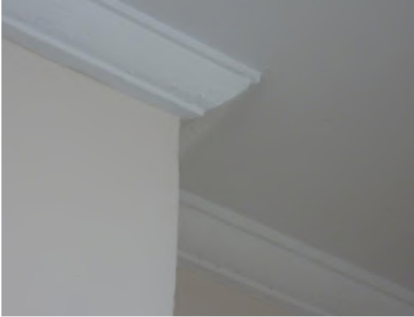
Figure 4.57 Flat ceiling and timber cornice detail, typical of ground floor level spaces (Flat 56B). (Source: GML 2015)
