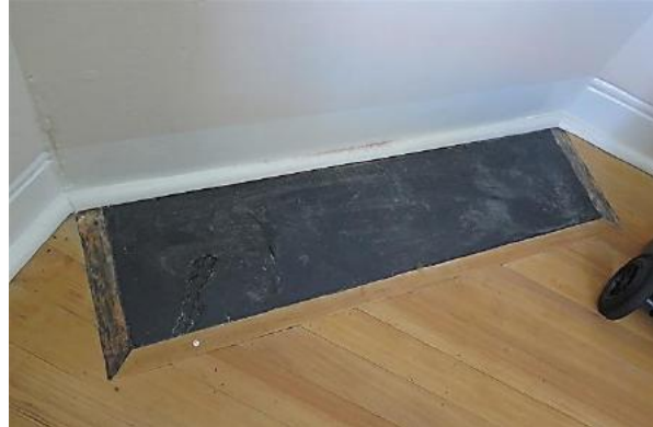
Figure 13.15 Original corner fireplace blocked up with concrete hearth (space G.2). Note skirtings have not been continued across fireplace wall—56 / 46-56 Gloucester Street. (Source: GML Heritage, July 2016)
