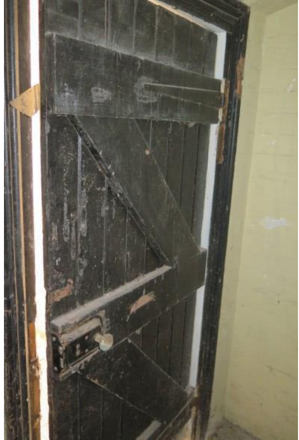
Figure 3.47 Original ledged/braced timber boarded door (space E.3)—48 / 46–56 Gloucester Street. (Source: GML Heritage, May 2016)
