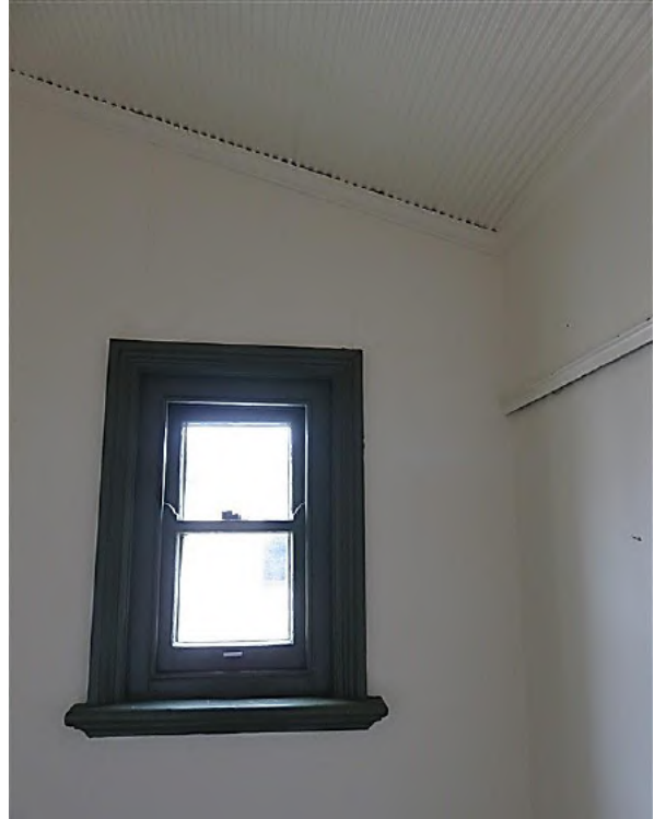
Figure 8.43 Laundry (space 2.2) showing original raked ripple iron ceiling and modern sash window—52A / 46–56 Gloucester Street. (Source: GML Heritage, July 2016)
