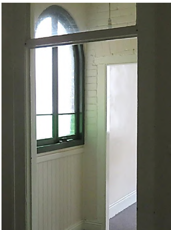
Figure 10.30 Casement windows and v-jointed vertical boarded panel below are late twentieth century infill to the original arched opening of the former rear porch—54A / 46–56 Gloucester Street. (Source: GML Heritage, July 2016)
