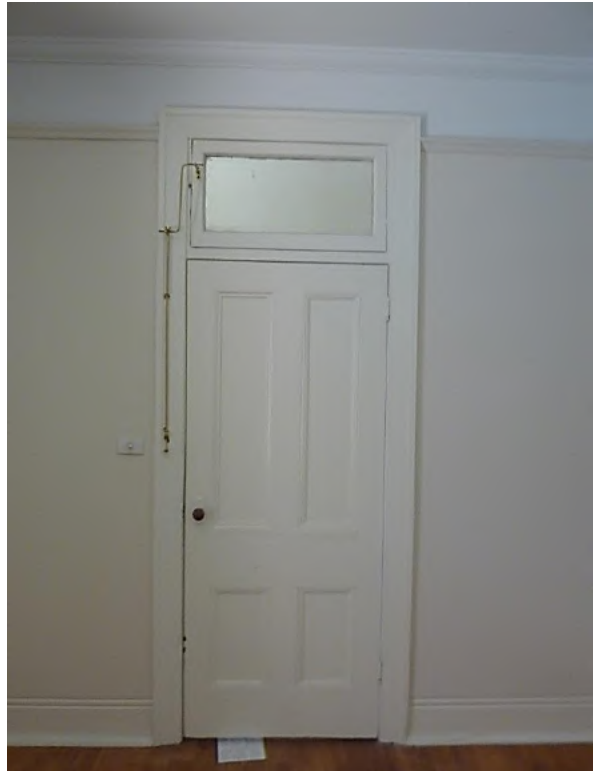
Figure 3.19 Run cement skirtings, four-panel timber door with fanlight above and reproduction mechanism between the front bedroom (space G.2) and entry (space G.1)—48 / 46–56 Gloucester Street. (Source: GML Heritage, November 2015)
