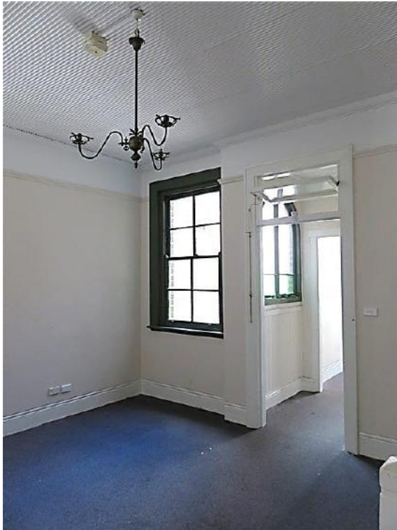
Figure 14.25 View from space 1.3 into space 1.4 showing floor of space 1.4 raised to same level as floors in surrounding rooms and timber skirting under arched window in north wall of space 1.4—56A / 46–56 Gloucester Street (Source: GML Heritage, July 2016)
