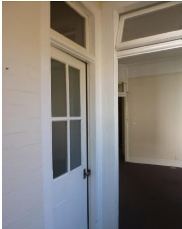
Figure 2.32 Modern half-glazed door to the bathroom (space 1.5)—46A / 46–56 Gloucester Street. (Source: GML Heritage, November 2015)
