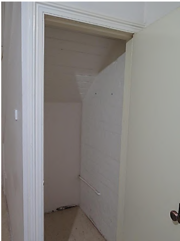
Figure 7.32 Enclosed space below the stairs, showing unrendered painted brick wall—52 / 46–56 Gloucester Street. (Source: GML Heritage, July 2016)
