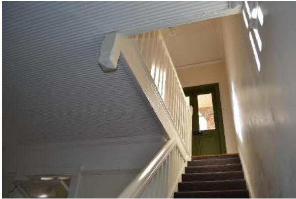
Figure 6.32 Stair (space 1.7)—50A / 48–56 Gloucester Street, showing the original ripple iron ceiling, timber balustrade and handrail and newel post projecting below stair (Source: GML Heritage, July 2016)
