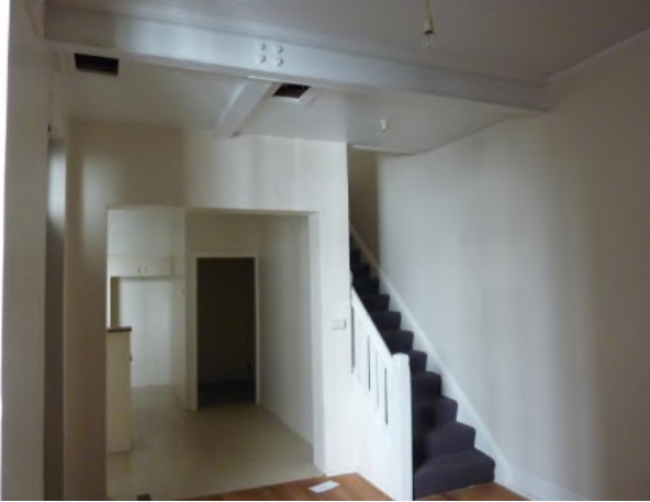
Figure 4.25 The lower ground floor level (Flat 48) showing the original timber stair . Note the large opening cut through to the kitchen and enclosure to create the laundry under stairs c1988. (Source: GML 2015)
