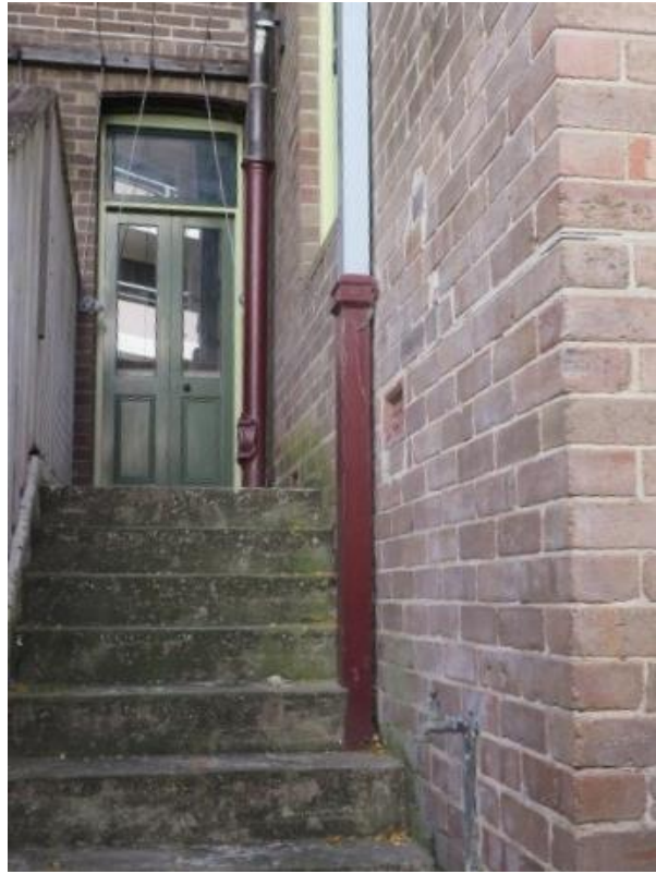
Figure 3.55 Half-glazed French doors with fanlights, with original segmental headed opening, accessing the rear yard from the kitchen. Also shows concrete steps leading up from the rear yard (space E.2) — 48 / 46–56 Gloucester Street. (Source: GML Heritage, May 2016)
