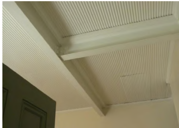
Figure 4.60 Original steel beams supporting walls above (lower ground floor level, flat 46) and ripple iron ceiling. (Source: GML 2015)
