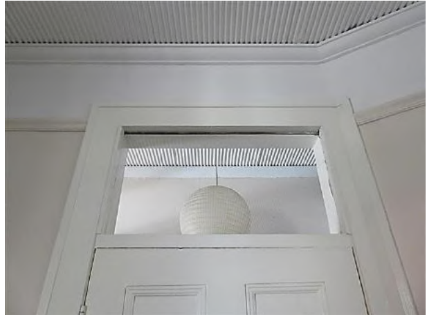
Figure 16.23 Original architrave, picture rail and cornice details. Pivot fanlight sash missing from above front bedroom door (space 1.2)—56C / 46–56 Gloucester Street. (Source: GML Heritage, July 2016)
