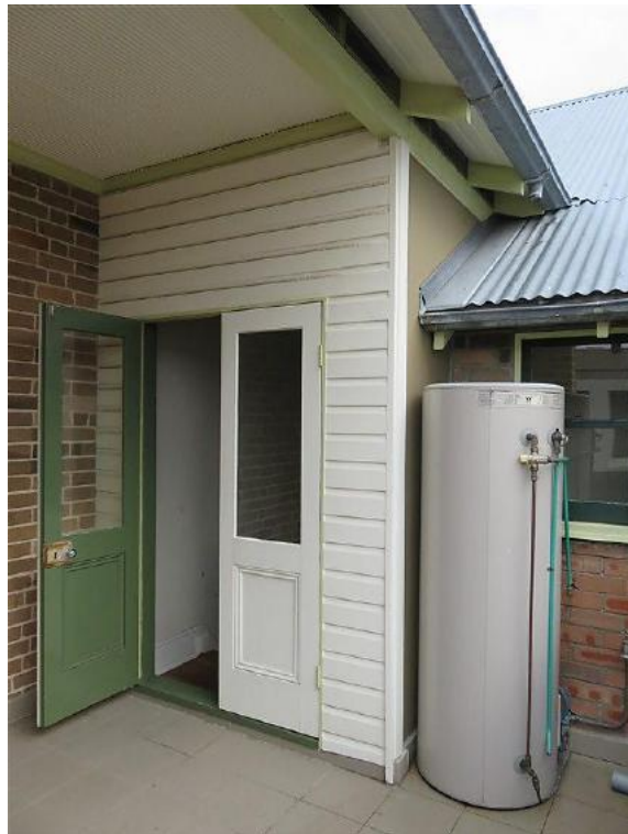
Figure 10.19 Rear wall of the flat opening onto the roof terrace (space E.1), showing recent weatherboard wall, pair of half glazed doors and rendered finish to stair hall wall. The window is also recent, replacing a previous door—54A / 46–56 Gloucester Street. (Source: GML Heritage, July 2016)
