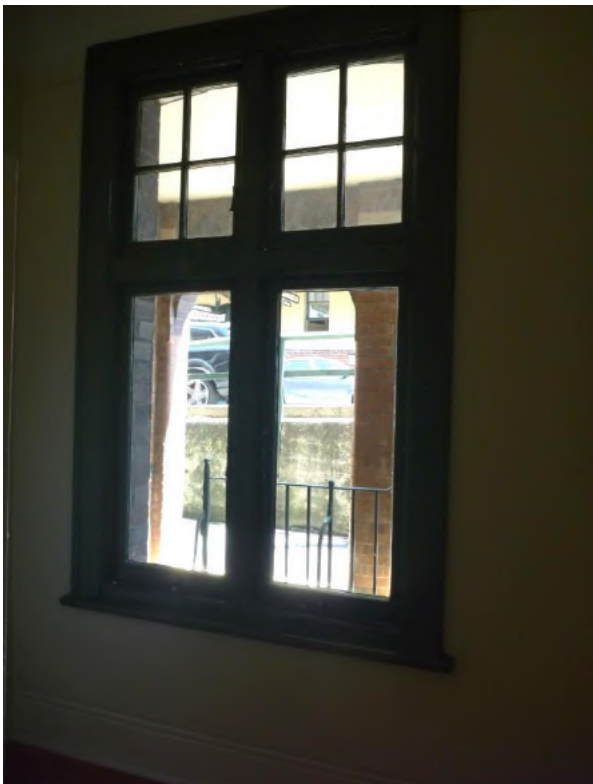
Figure 4.35 Timber casement window in the western elevation with original timber architrave, sill board and moulding (ground floor level, Flat 46). (Source: GML 2015)
