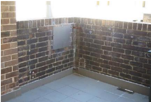
Figure 4.12 Terrace (space E.2) showing the original garbage shoot blocked up and brick balustrade—48A/46–56 Gloucester Street. (Source: GML Heritage, May 2016)
