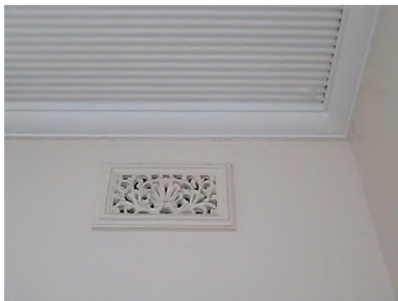
Figure 12.23 Detail of the decorative plaster wall vent, timber cornice and ripple iron ceiling typical to flat 54A (space 1.2)—54C / 46–56 Gloucester Street. (Source: GML Heritage, July 2016)
