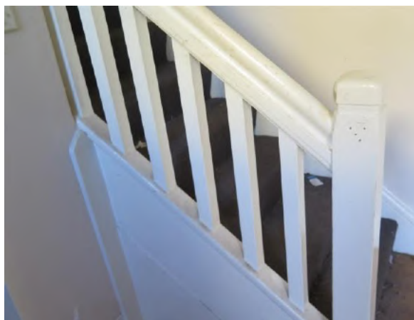
Figure 15.37 Original stair (space LG.1) with closed string, simple square balusters and newel posts, and moulded handrail—56B / 46–56 Gloucester Street. (Source: GML Heritage, July 2016)
