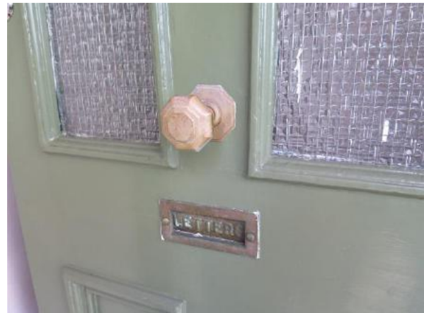
Figure 11.9 Original door knob(?) and letter slot on front door—54B / 46-56 Gloucester Street (Source: GML Heritage, June 2016)
