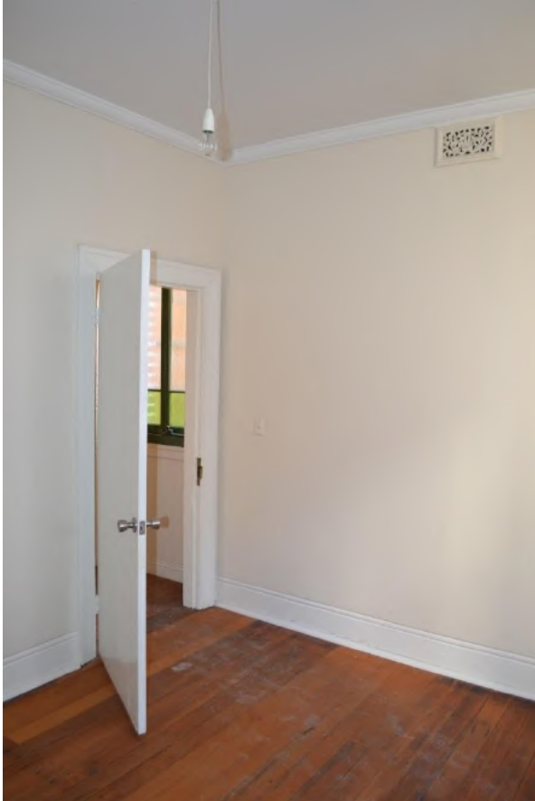
Figure 1.34 Rear bedroom (space G.6) showing the plaster board ceiling, cement rendered skirting and modern door—46/46–56 Gloucester Street. (Source: GML Heritage, July 2016)
