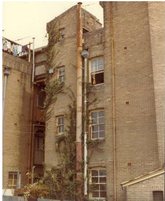
Figure 2.10 Rear (eastern) elevation (Flats 50 and 50A) showing the balustrade across the opening of rear porches, the garbage chute and building's condition in 1984. (Source: SHFA, Image 49763 CEM 31)
