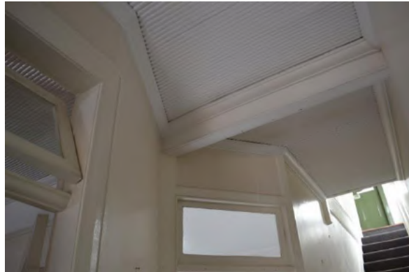
Figure 2.20 Typical detail of original internal fanlight, ripple iron ceiling and moulded timber cornice—door between spaces 1.1 and 1.3—46A / 46–56 Gloucester Street. (Source: GML Heritage, July 2016)
