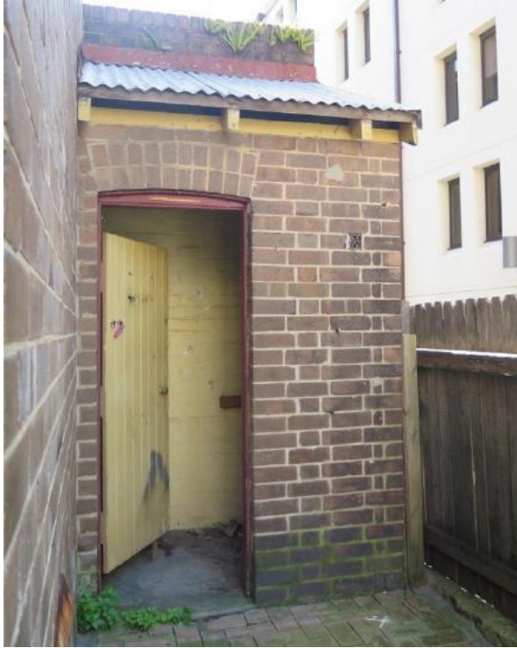
Figure 15.50 External WC or store in common brick (space E.3) with skillion roof and timber door with brick arch above—56B / 46–56 Gloucester Street. (Source: GML Heritage, July 2016)
