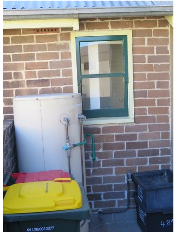
Figure 4.11 Rear wall of terrace (space E.2) showing modern spiral balance timber sash window and repaired brickwork to laundry—48A / 46–56 Gloucester Street. (Source: GML Heritage, May 2016)
