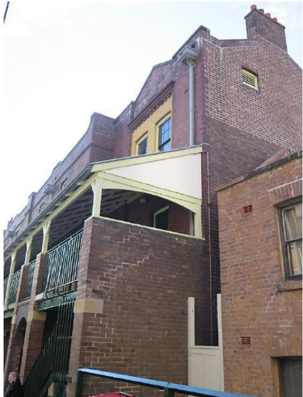
Figure 16.7 Southern elevation (partially concealed behind the neighbouring building) showing timber louvre to roof space and brick chimney stack with terra cotta pots—56C / 46–56 Gloucester Street. (Source: GML Heritage, July 2016)
