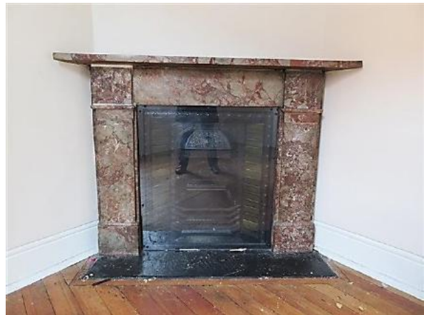
Figure 8.49 Fireplace in the front room on second floor (space 2.4) with early cast iron grate with tiled sides (covered with perspex), and red marble chimney piece—52A / 46–56 Gloucester Street. (Source: GML Heritage, July 2016)
