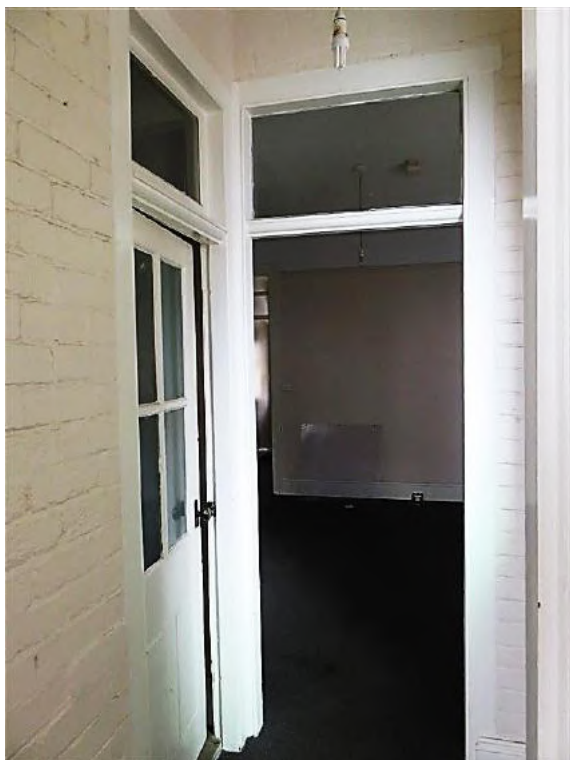
Figure 10.28 Former porch (space 1.4), showing original door frames. The door to the bathroom (space 1.5) has its original half glazed door and fanlight—54A / 46–56 Gloucester Street. (Source: GML Heritage, July 2016)
