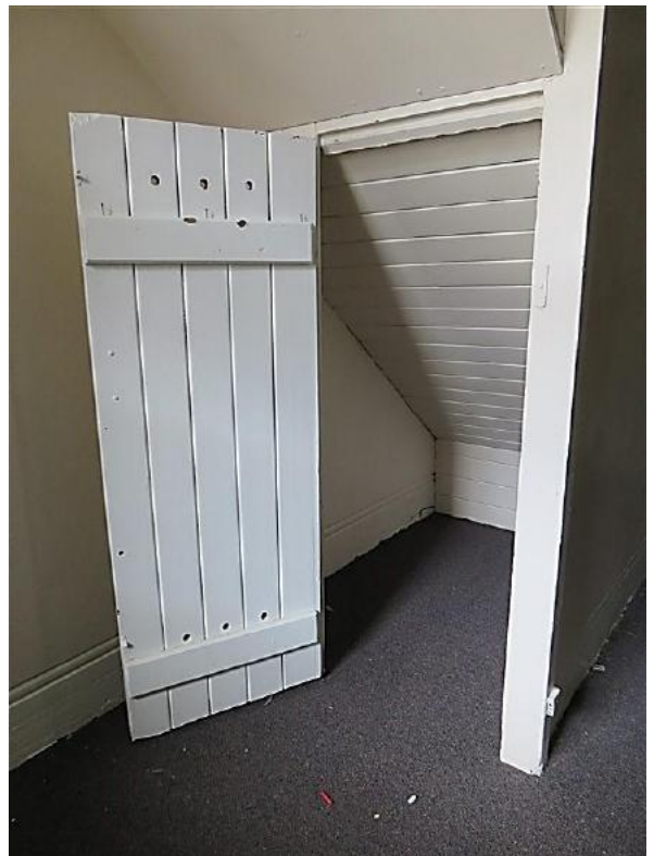
Figure 8.29 Cupboard under the stairs (space 1.3) showing the v-jointed timber stair soffit and ledged and sheeted timber door—52A / 46–56 Gloucester Street. (Source: GML Heritage, July 2016)
