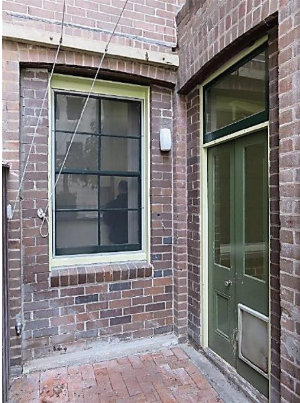
Figure 7.38 Original opening to rear elevation (Kitchen) with modern brick infill and replacement sash window—52/46–56 Gloucester Street (Source: GML Heritage, June 2016)
