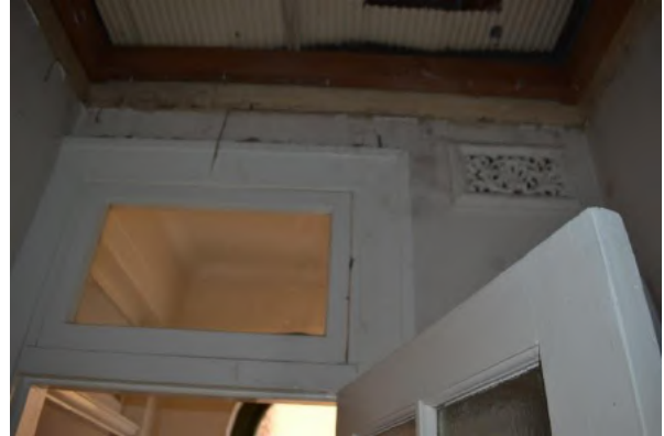
Figure 1.31 Bathroom (space G.5) showing the original fanlight and decorative plaster wall vent—46/46–56 Gloucester Street. (Source: GML Heritage, July 2016)
