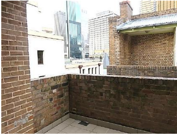
Figure 12.14 Roof terrace (space E.1) showing tiled floor and evidence of the original garbage chute (blocked up)—54C / 46–56 Gloucester Street—54C / 46–56 Gloucester Street. (Source: GML Heritage, July 2016)
