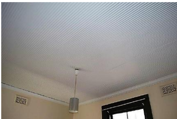
Figure 2.35 Ripple iron ceiling in the rear bedroom with moulded timber cornice (space 1.6) showing the decorative plaster wall vents—46A/46–56 Gloucester Street. (Source: GML Heritage, July 2016)
