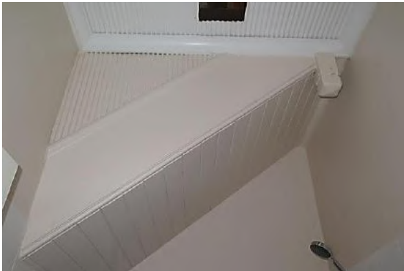
Figure 4.36 Bathroom (space 1.5) showing boarded soffit to stair, pendant newel to stair, and ripple iron ceiling, with section of ripple iron over stringer—48A / 46–56 Gloucester Street. (Source: GML Heritage, May 2016)
