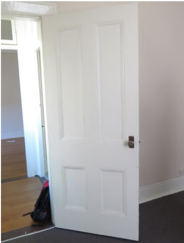
Figure 15.32 Original four-panel sunk moulded timber door in the rear bedroom (space G.6)—56B / 46–56 Gloucester Street. (Source: GML Heritage, July 2016)
