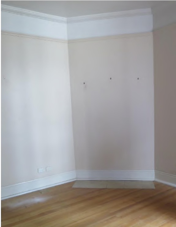
Figure 13.18 Living room showing blocked off fireplace, skirting, picture rail and cornice (space G.3)—56 / 46–56 Gloucester Street. (Source: GML Heritage, July 2016)
