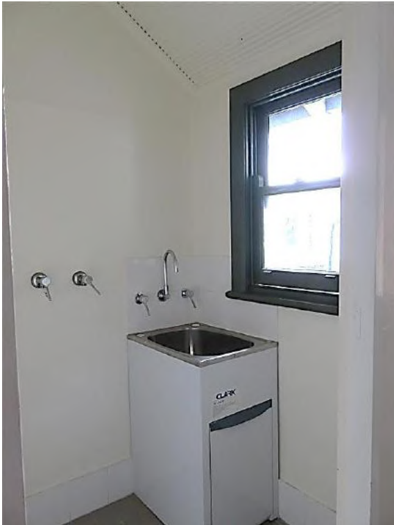
Figure 10.42 Laundry (space 2.2) showing modern laundry tub unit and original raked ripple iron ceiling. The window is late 20 th century—54A / 46–56 Gloucester Street. (Source: GML Heritage, July 2016)
