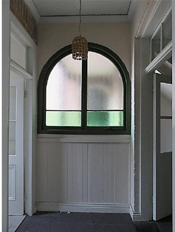
Figure 8.31 Original opening to rear porch (space 1.4), infilled with a casement window—52A / 46–56 Gloucester Street. (Source: GML Heritage, July 2016).
