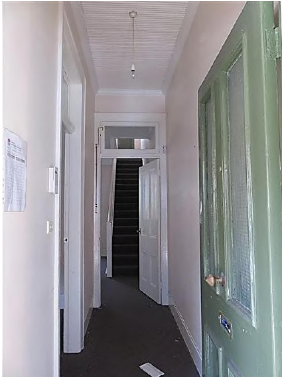
Figure 14.16 Entrance hall (space 1.1) showing the ripple iron ceiling, moulded timber cornice and cement rendered skirting—56A / 46–56 Gloucester Street. (Source: GML Heritage, July 2016)
