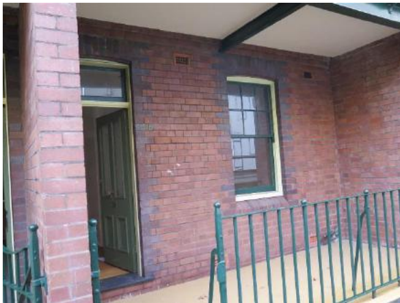
Figure 11.8 Front porch (space E.1) showing external brick walls, timber entry door with fanlight, wrought iron fence and gate, double-hung window with chamfered brick sill—54B / 46-56 Gloucester Street. (Source: GML Heritage, July 2016)
