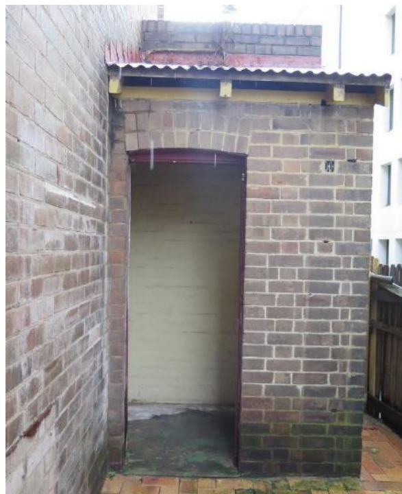
Figure 11.39 External WC (space E.3) with skillion roof, brick parapet. Boarded timber door is missing—54B / 46–56 Gloucester Street. (Source: GML Heritage, July 2016)
