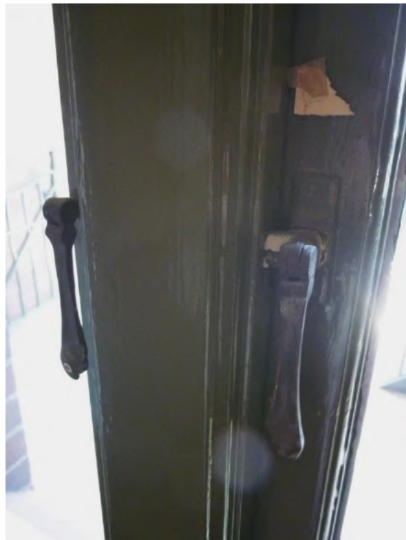
Figure 4.36 Original casement window fixtures (Flat 46). (Source: GML 2015)
