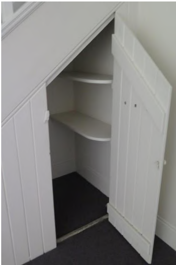
Figure 4.47 Original ledged and sheeted cupboard door to area below the stairs (first floor level, Flat 48A). (Source: GML Heritage 2015)
