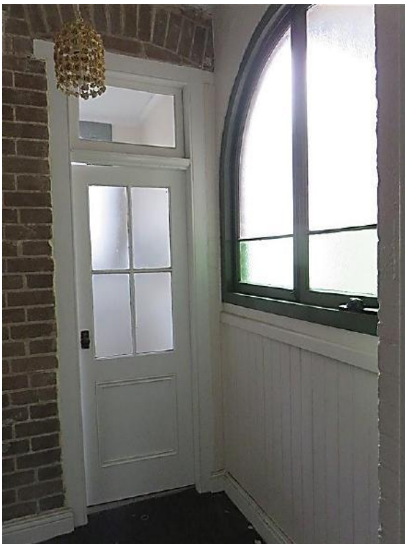
Figure 8.32 Half glazed door to bathroom (space 1.4) with original door frame, fanlight, unpainted brickwork and arched door head—52A / 46–56 Gloucester Street. (Source: GML Heritage, July 2016).
