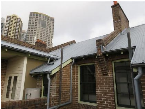
Figure 14.12 Rear elevation of Flat 56A showing corrugated metal roof, party walls and chimneys—56A / 46–56 Gloucester Street. (Source: GML Heritage, July 2016)
