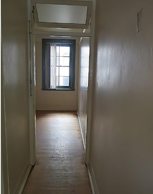
Figure 7.10 Entry (space G.1) showing timber floor, cement run skirtings, with quad mould, and timber door frame with fanlight over to the living room (space G.3)—52 / 46–56 Gloucester Street (Source: GML Heritage, July 2016)
