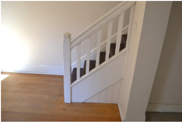
Figure 1.36 Original stair (space LG.1) with closed string, square balusters and newel posts, and moulded timber handrail—46/46–56 Gloucester Street. (Source: GML Heritage, July 2016)
