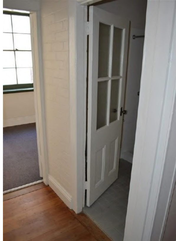
Figure 5.23 Infilled former rear porch opening, showing the cement skirting and half-glazed timber panel door to the bathroom—50 / 46-56 Gloucester Street. (Source: GML Heritage, June 2016)
