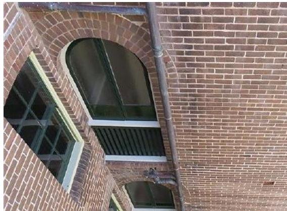
Figure 12.12 Original brick arched opening to former porch in rear wing (first floor level), now infilled with window and solid balustrade). Typical triple brick to window head and arched opening—54C / 46–56 Gloucester Street. (Source: GML Heritage, July 2016)
