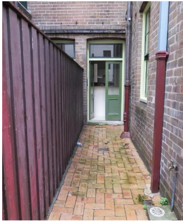
Figure 11.37 Exterior walls of the rear wing showing original cast iron and modern stainless and copper downpipes and paved yard area (space E.2)—54B / 46–56 Gloucester Street. (Source: GML Heritage, July 2016)
