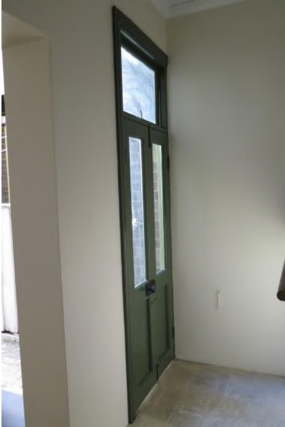
Figure 3.42 Modern half-glazed double French doors from the kitchen (space LG.2) to the rear yard—48 / 46–56 Gloucester Street. (Source: GML Heritage, May 2016)
