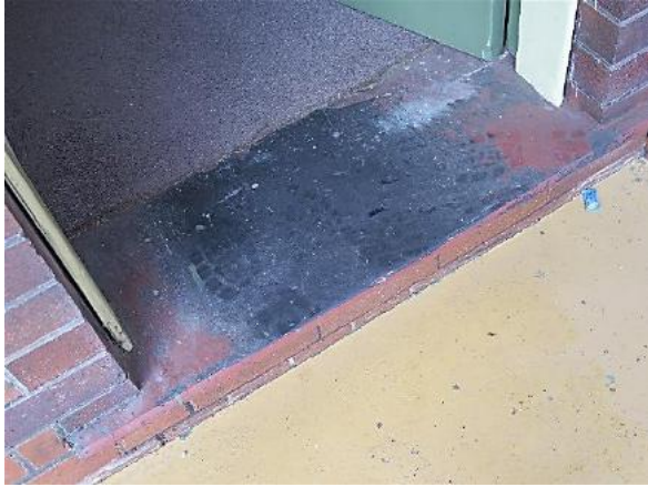
Figure 9.10 Slate threshold—54 / 46–56 Gloucester Street. (Source: GML Heritage, November 2015)
