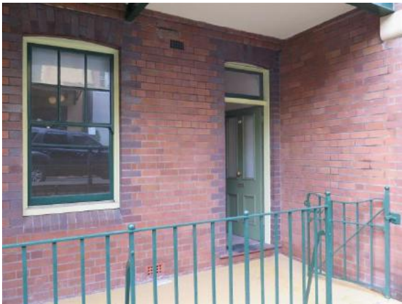
Figure 9.8 Front porch (space E.1) showing external brick walls, timber entry door with fanlight, wrought iron fence and gate, double-hung window with chamfered brick sill—54 / 46–56 Gloucester Street. (Source: GML Heritage, July 2016)
