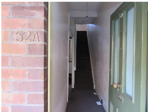
Figure 8.18 Entrance hall (space 1.1) showing cement rendered skirtings and carpeted floors—52A / 46–56 Gloucester Street. (Source: GML Heritage, July 2016)
