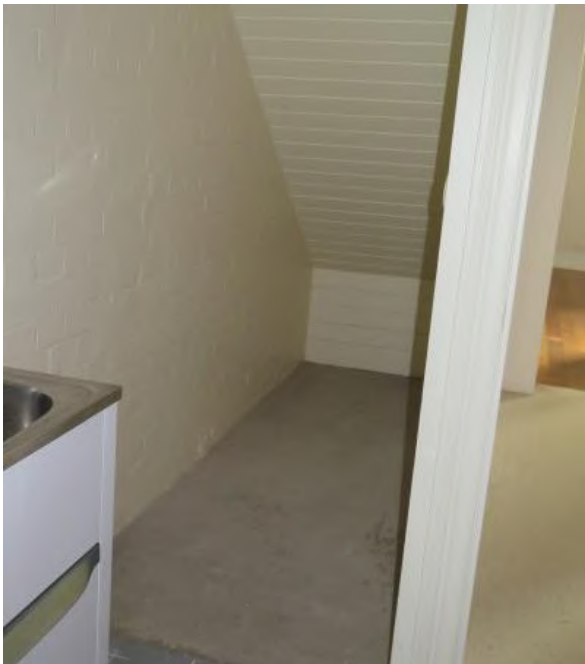
Figure 3.44 The enclosed laundry below the boarded stairs, showing unrendered painted brick (space LG.3)—48 / 46–56 Gloucester Street. (Source: GML Heritage, May 2016)
