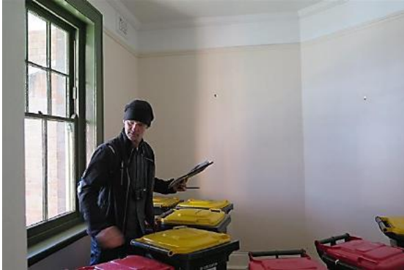
Figure 13.14 Front bedroom (space G.2)—56 / 46-56 Gloucester Street, showing fibrous plaster cornice, timber picture rail, decorative plaster wall vent and blocked up fireplace to far right of image. (Source: GML Heritage, July 2016)
