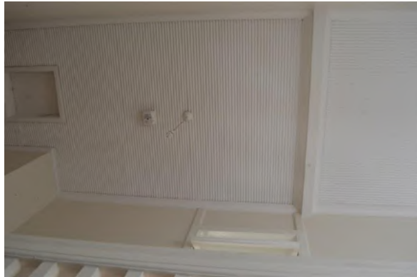
Figure 2.38 Ceiling of second floor landing (space 2.1) showing the ripple iron ceiling running in opposite directions—46A/46–56 Gloucester Street. (Source: GML Heritage, July 2016)
