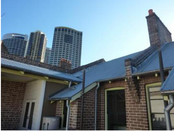
Figure 4.17 Brick party walls with corbelled brickwork at the eaves. The weatherboard wall and French doors onto the roof top terrace are c1988 (Flat 54C). (Source: GML 2015)
