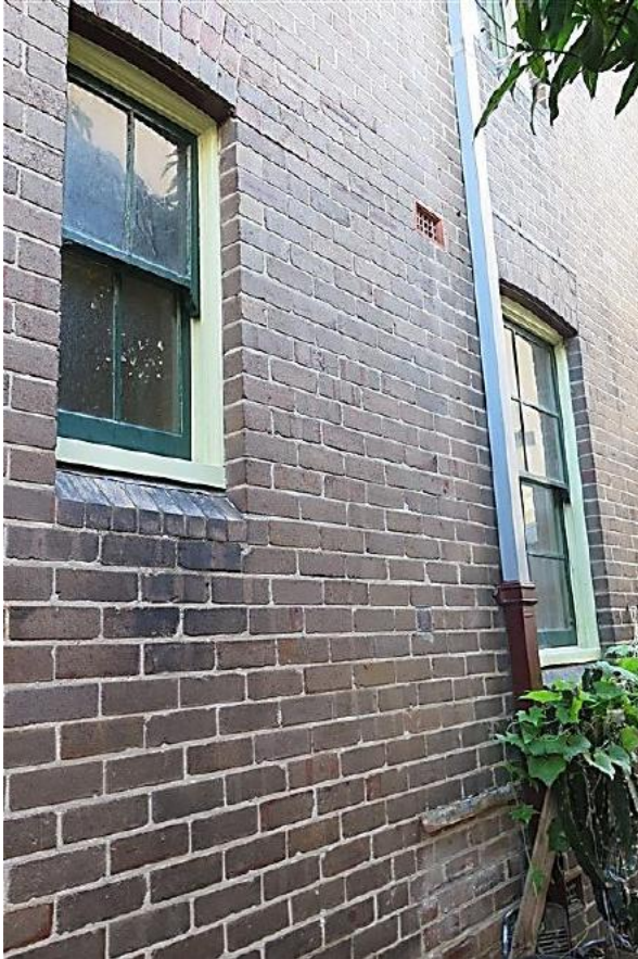
Figure 7.42 Triple brick arched head and chamfered sill details to windows in rear elevation (typical detail to the 46-56 Gloucester Street flats)—52/46-56 Gloucester Street. (Source: GML Heritage, March 2016)
