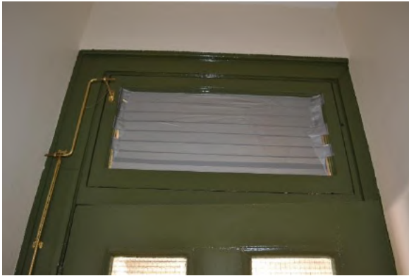
Figure 6.18 Original pivot internal fanlight to main entry door, reproduction mechanism and moulded timber cornice. Space 1.1—50A / 48–56 Gloucester Street. (Source: GML Heritage, July 2016)
