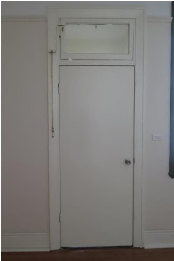
Figure 3.24 Modern hollow core door with original transom light above and reproduction mechanism between the living room (space G.3) and the former rear porch (space G.4)—48 / 46–56 Gloucester Street. (Source: GML Heritage, May 2016)
