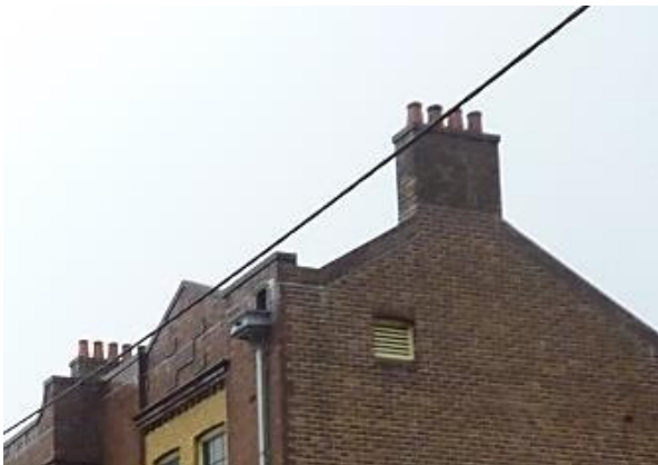
Figure 4.3 Detail of the timber louvre for ventilation of the roof space over flat 56A, and original chimney stack with terracotta chimney pots. (Source: GML Heritage, July 2016)
