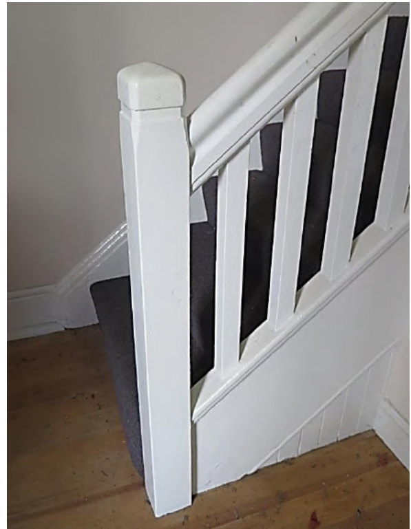
Figure 13.27 Dining area (space LG.1). Original timber balustrade to stair consisting of square newel post, and balusters and moulded timber handrail. The stair has closed strings—56 / 46—56 Gloucester Street. (Source: GML Heritage, July 2016)
