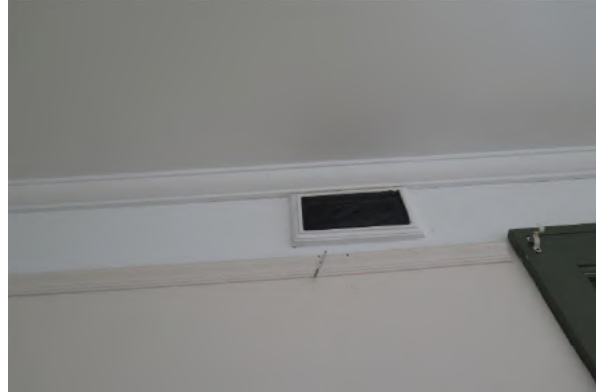
Figure 15.19 Front bedroom (space G.2) showing the moulded timber picture rail, plasterboard ceiling and wall vent with fly wire cover—56B / 46–56 Gloucester Street. (Source: GML Heritage, July 2016)
