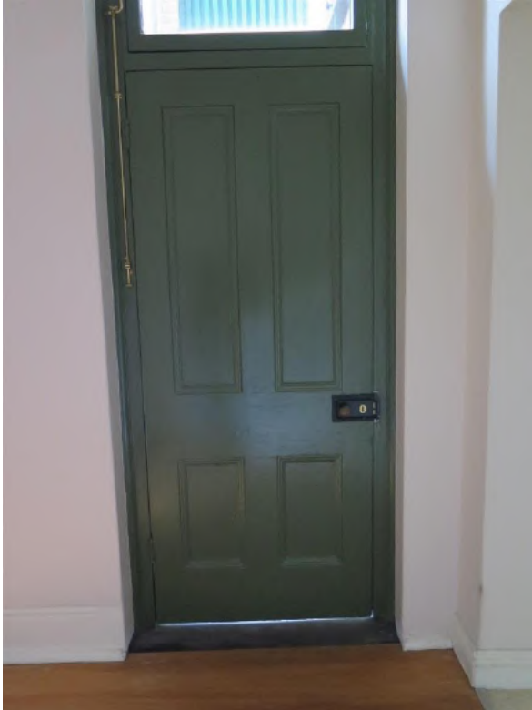
Figure 11.26 Four-panel bolection moulded timber external door with fanlight (space LG.1) —54B / 46–56 Gloucester Street. (Source: GML, July 2016).
