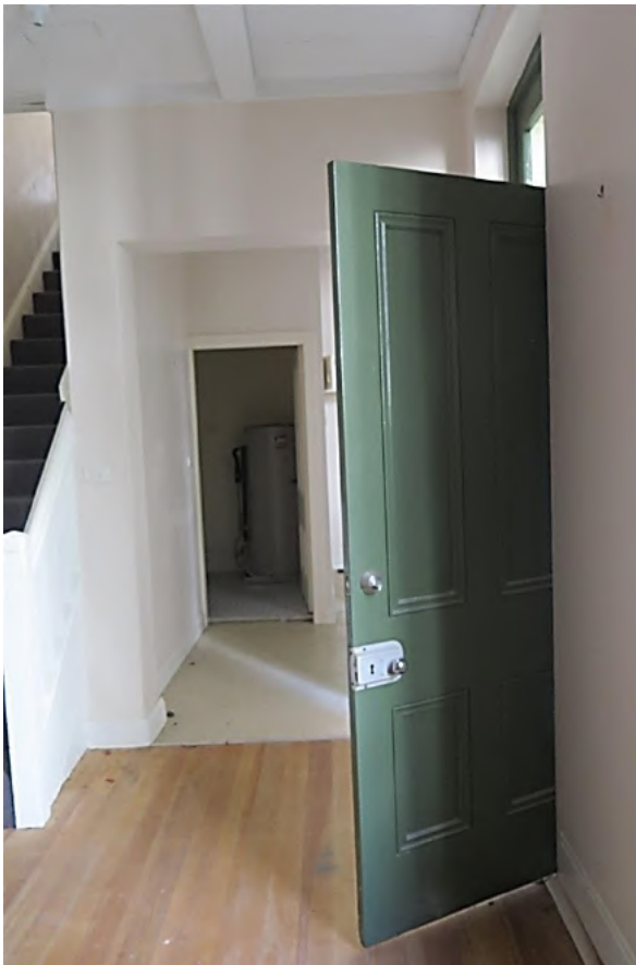
Figure 13.30 Four panel sunk-moulded external door (space LG.1). Large opening through to kitchen (space LG.2 is late 20 th century). (Source: GML Heritage, July 2016)
