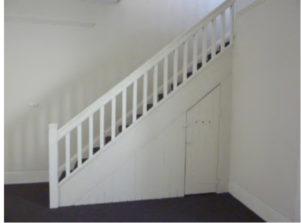
Figure 4.46 The timber-boarded wall and ledged and braced door to the area below the stair (first-floor level, Flat 48A). (Source GML 2015)
