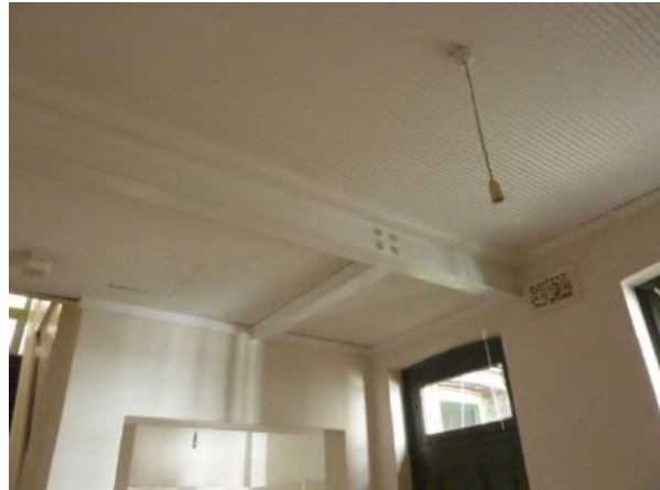
Figure 5.35 Dining room (space LG.1) showing the ripple iron ceiling, decorative plaster wall vent and fanlight above door to rear yard—50 / 46–56 Gloucester Street. (Source: GML Heritage, June 2016)
