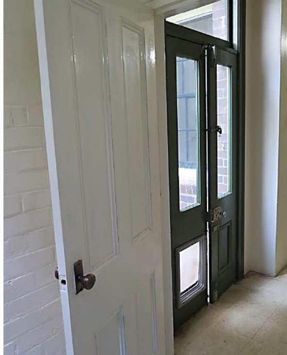
Figure 7.35 Four panel timber door as viewed from interior of laundry (space LG.5). Modern French doors to rear yard. (Source: GML Heritage, July 2016)
