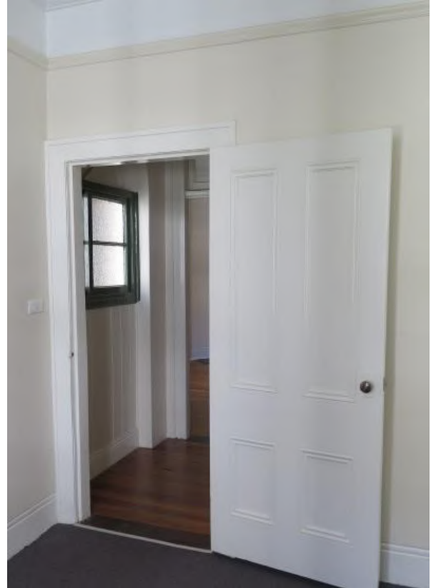
Figure 3.31 Original/reproduction four-panel sunk moulded timber door, original timber picture rail and timber cornice in the rear bedroom (space G.6)—48 / 46–56 Gloucester Street. (Source: GML Heritage, May 2016)
