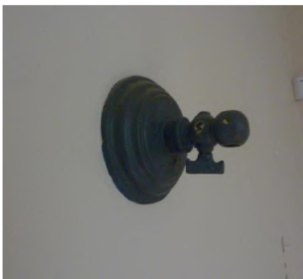
Figure 4.63 A gas light fitting (Flat 56B). (Source: GML 2015)
