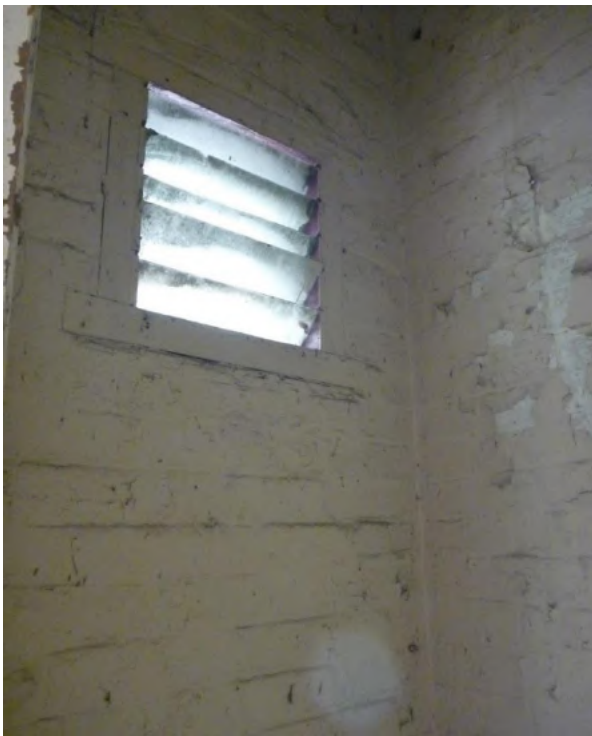
Figure 1.52 External store (space E.3) showing the original painted bricks and louvred glass window with brick arch above—46/46–56 Gloucester Street. (Source: GML Heritage, July 2016)
