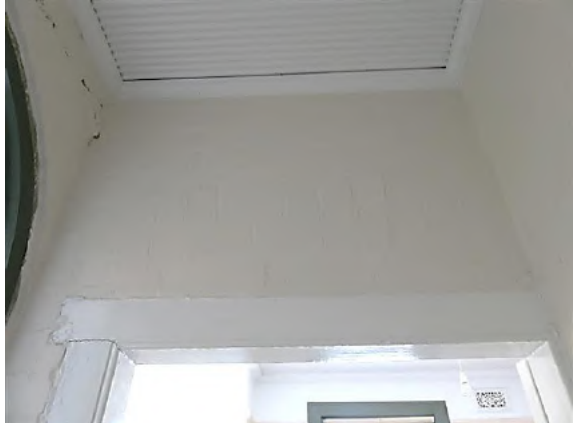
Figure 14.28 Original brick arched head above doorway opening to former porch (space 1.4) and ripple iron ceiling—56A / 46–56 Gloucester Street. (Source: GML Heritage, July 2016)
