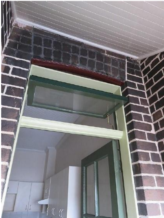
Figure 10.46 Detail of original door onto balcony from kitchen (space 2.3) with arched brick head and fanlight over—54A / 46–56 Gloucester Street. (Source: GML Heritage, July 2016)
