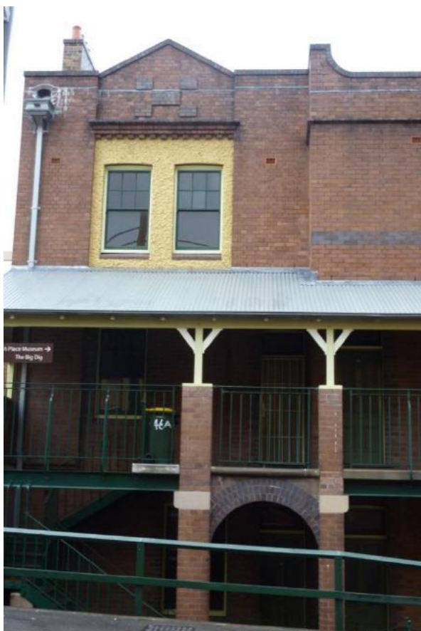
Figure 2.6 Western façade of flat 46A as viewed from Gloucester Street, showing pebble dash render to central portion of second floor wall, and decorative brick cornice and checkerboard pattern panel to triangular parapet, cast metal rainwater head and downpipe. (Source: GML Heritage, July 2016)
