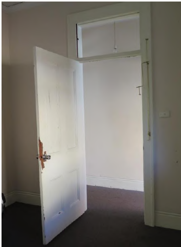
Figure 4.31 Damaged four-panel internal door with later door hardware (first floor level, Flat 54A). (Source: GML 2016)
