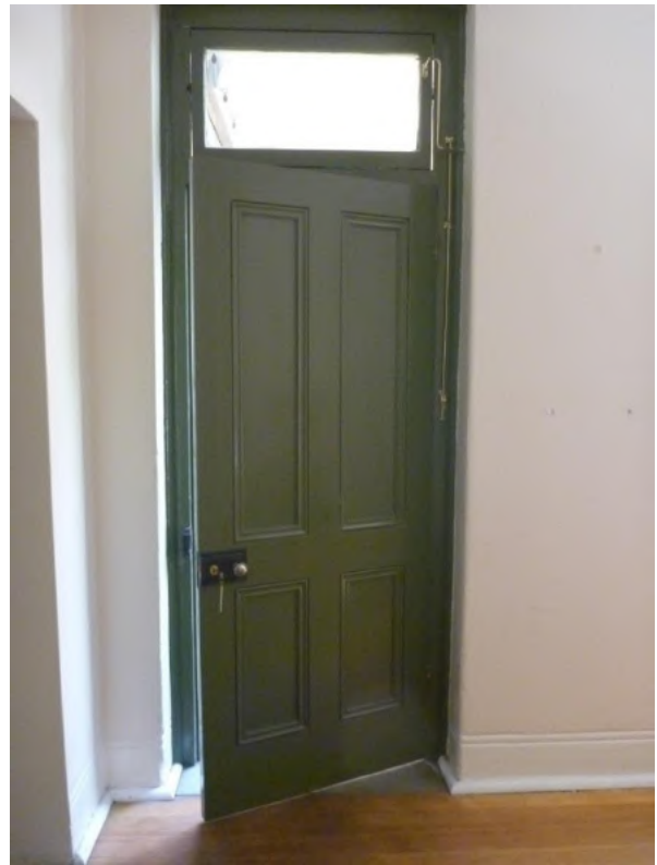
Figure 1.41 timber four panel door with bolelection mouldings and fanlight to rear yard (space E.2)—46/46–56 Gloucester Street. (Source: GML Heritage, July 2016)
