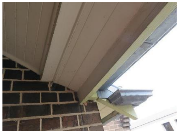
Figure 10.15 Painted V-jointed timber boarding to ceiling of the recessed balcony (space 2.3)—54A / 46–56 Gloucester Street. (Source: GML Heritage, July 2016)
