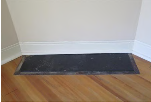
Figure 15.22 Living area (space G.3) showing blocked up fireplace with original concrete hearth—56B / 46–56 Gloucester Street, Source: GML Heritage, June 2016)
