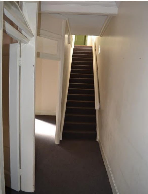
Figure 2.19 Entrance hall (space 1.1) showing the ripple iron ceiling, moulded timber cornice and fanlights to front bedroom (space 1.2) and living room (space 1.2)—46A/46–56 Gloucester Street. (Source: GML Heritage, July 2016)
