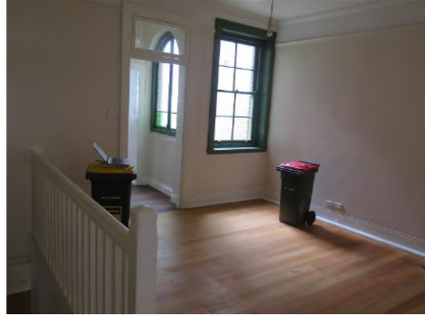
Figure 11.15 Living room (space G.3) showing cement run skirtings, timber flooring, picture rail, timber balustrade and newel post and timber double-hung sash window—54B / 46–56 Gloucester Street. (Source: GML Heritage, July 2016)
