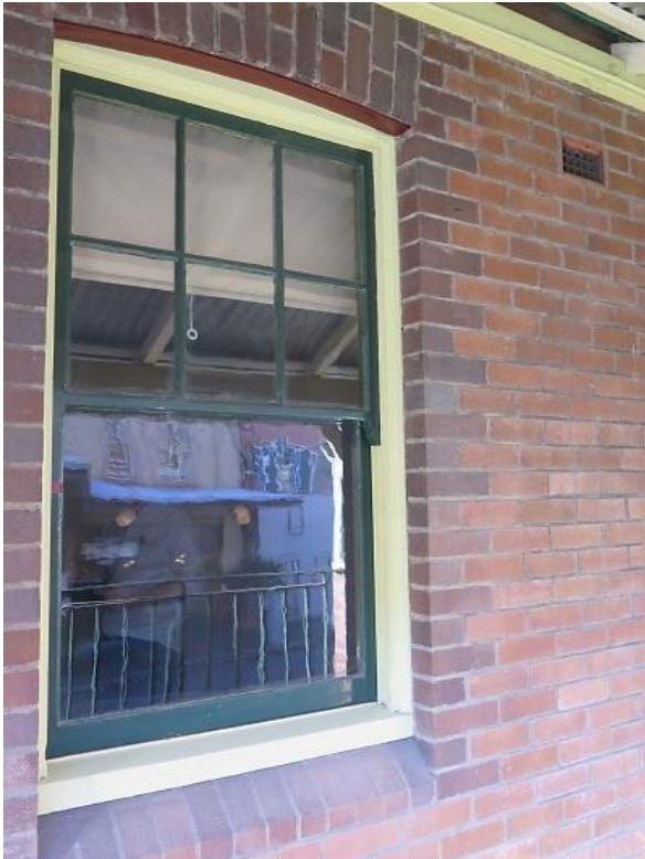
Figure 4.8 Double hung sash window with arched brick head and chamfered brick sill, terracotta vent and dark brick surround—48A / 46–56 Gloucester Street. (Source: GML Heritage, May 2016)
