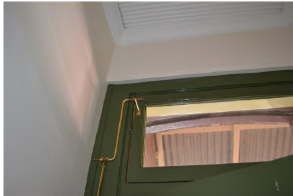
Figure 2.13 Fanlight and mechanism above front door—46A/46–56 Gloucester Street. (Source: GML Heritage, July 2016)
