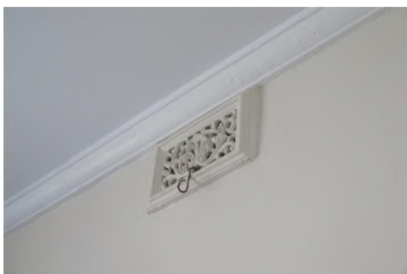
Figure 15.28 Bathroom (space G.5) showing the plasterboard ceiling and decorative plaster wall vent as typical to the flat—56B / 46–56 Gloucester Street. (Source: GML Heritage, July 2016)
