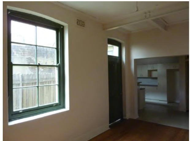
Figure 4.24 Lower ground floor room (Flat 56B) with original window and four-panelled door with external beaded panels, with a fanlight over. Note the large opening cut through to kitchen c1988. (Source: GML 2015)
