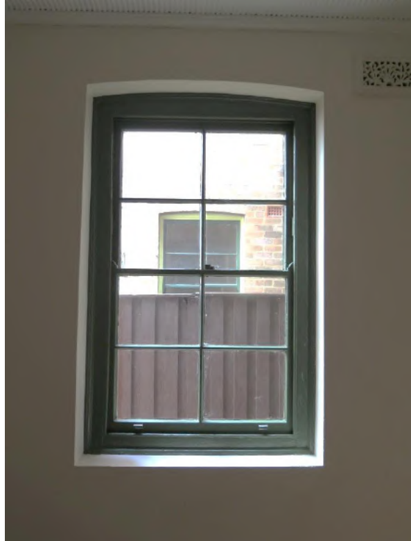
Figure 11.27 Timber double hung sash window, frame and brick sill (Space LG.1) —54B / 46–56 Gloucester Street. (Source: GML Heritage, July 2016).
