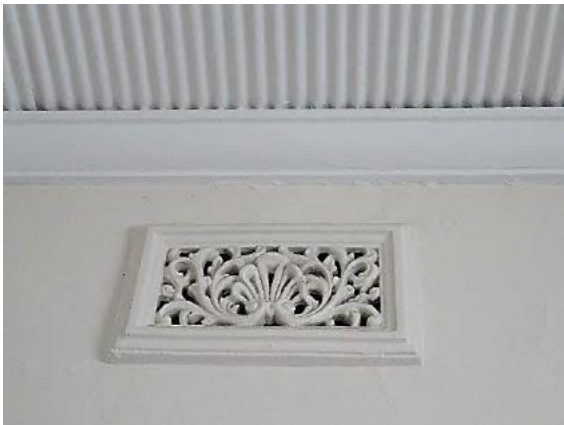
Figure 10.50 Detail of decorative plaster wall vent in space 2.4—54A / 46–56 Gloucester Street. (Source: GML Heritage, July 2016)
