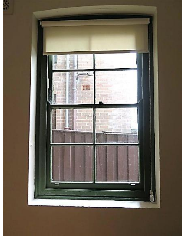
Figure 9.27 Lower ground-floor level timber double hung sash window with rendered reveals (space LG.1)—54 / 46–56 Gloucester Street. (Source: GML Heritage, July 2016)
