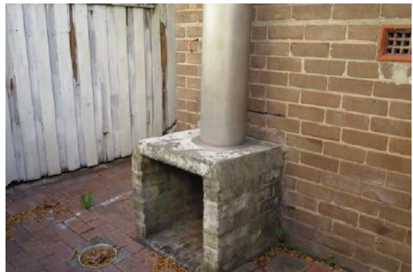
Figure 3.49 The original brick/concrete garbage chute surround and terracotta wall vents (space E.2)—48 / 46–56 Gloucester Street. (Source: GML Heritage, May 2016)
