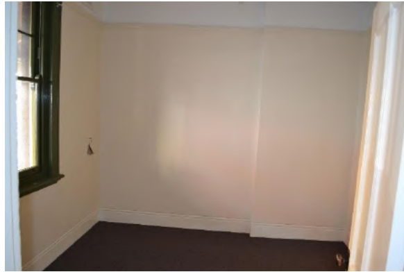
Figure 6.19 Front bedroom (space 1.2)—50A / 48–56 Gloucester Street, showing timber double hung sash window, moulded timber picture rail, run cement skirtings, flue and ripple iron ceiling with moulded timber cornice. (Source: GML Heritage, July 2016)
