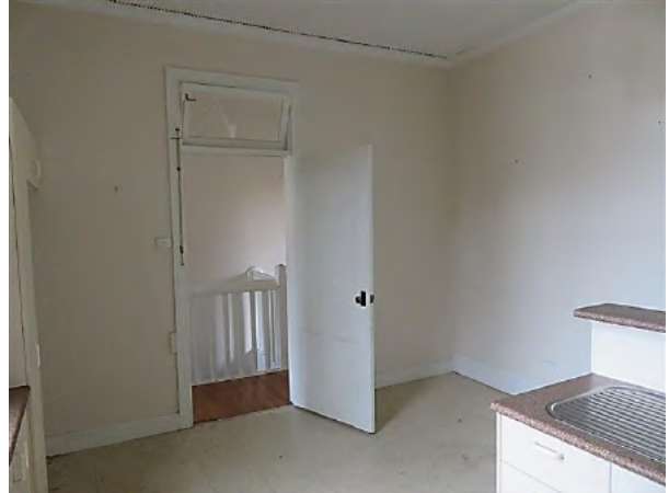
Figure 8.47 Kitchen (space 2.3) showing original four panel door, with architraves and fanlight above, original floor with later lino tiles and original cement skirtings—52A / 46–56 Gloucester Street. (Source: GML Heritage, July 2016)
