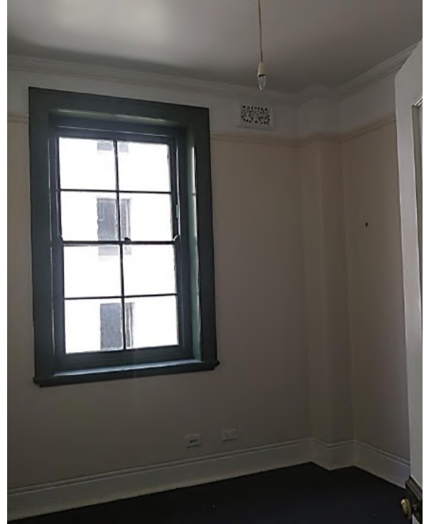
Figure 13.25 Rear bedroom (space G.6) showing carpeted floor, original cement run skirtings, timber picture rail, plaster cornice (not original) and decorative plaster wall vent. The timber double-hung sash window is original and retains its original architrave, sill board and moulding. A chimney flue rises in the southeast corner—56 / 46—56 Gloucester Street. (Source: GML Heritage, July 2016)
