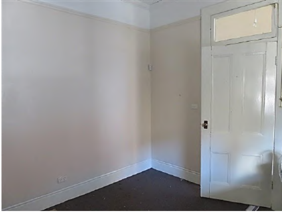
Figure 14.20 Front bedroom (space 1.2) with cement rendered skirting, picture rail and original four panel timber door with sunk moulds, original architrave and fanlight over—56A / 46–56 Gloucester Street. (Source: GML Heritage, July 2016)
