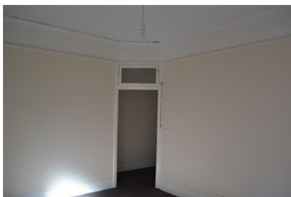
Figure 2.28 Living room (space 1.3) showing the original doorframe, with fanlight, to the entry hall (space 1.1), moulded timber picture rail and ripple iron ceiling—46A/46–56 Gloucester Street. (Source: GML Heritage, July 2016)
