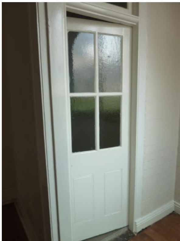
Figure 4.38 The original half-glazed door to the bathroom opening off the former porch (Flat 56B). The porch has painted brick walls, timber skirting and plain flat archtraves to the doors. (Source: GML 2015)
