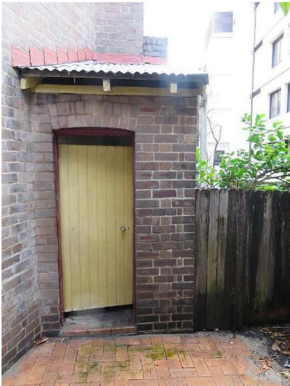
Figure 7.36 The rear yard (space E.2) and store in former external WC (space E.3) showing corrugated iron roof, exposed rafters at eaves, brick parapet and walls, brick arched head over doorway and timber ledged and sheeted door—52 / 46–56 Gloucester Street. (Source: GML Heritage, July 2016)
