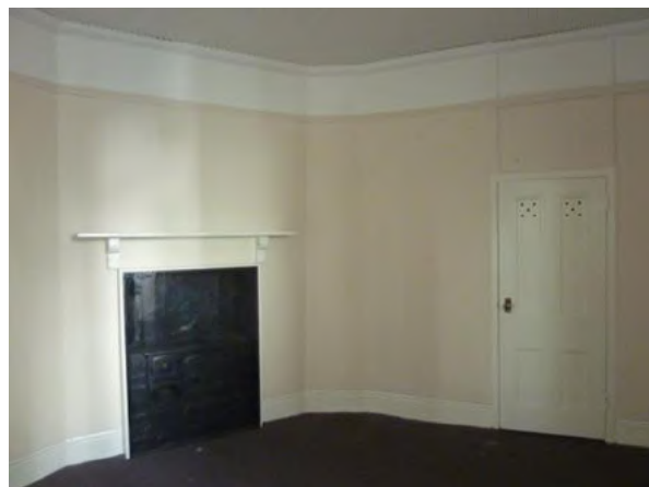
Figure 4.54 The cast-iron range and stone (?) mantel shelf in Flat 52A (the former kitchen, first floor level). (Source: GML 2015)
