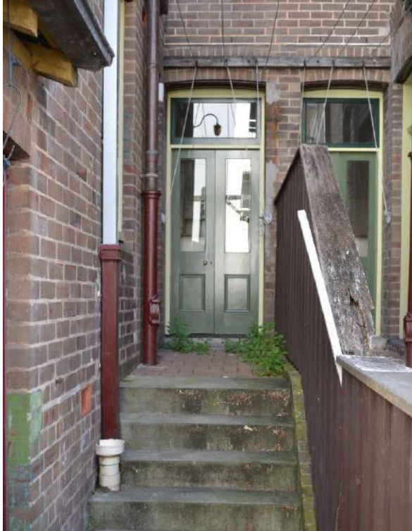
Figure 4.13 Rear of flat 50 showing copper and cast iron down pipes and modern steel downpipes. (Source: GML Heritage, July 2016)
