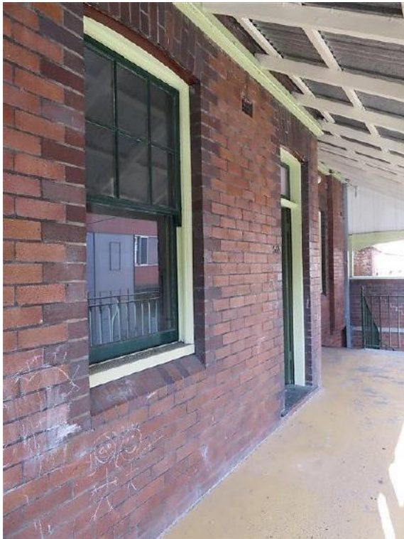
Figure 14.8 Front façade of flat 56A showing face brick external wall with contrasting brick surround to window and door openings and chamfered brick window sill—56A / 46–56 Gloucester Street. (Source: GML Heritage, July 2016)
