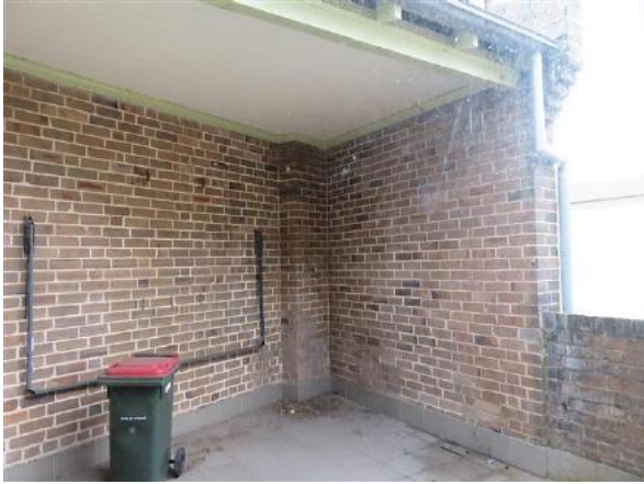
Figure 8.14 Roof terrace (space E.1) showing enclosed area with skillion roof, brick flue and ripple iron ceiling—52A/46–56 Gloucester Street. (Source: GML Heritage, July 2016)
