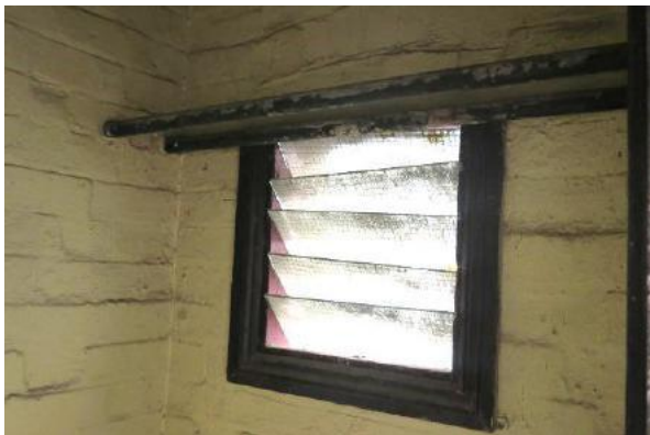
Figure 3.48 The store (space E.3) showing original timber fixed louvre window with early and later glass—48 / 46–56 Gloucester Street. (Source: GML Heritage, May)
