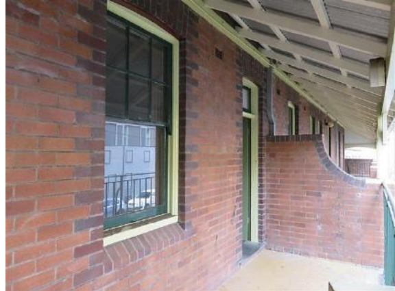
Figure 8.7 Front façade of flat 52A / 46–56 Gloucester Street showing face brick external wall with contrasting brick surround to window and door openings, chamfered brick window sill and dividing wall of the shared verandah (Source: GML Heritage, July 2016).
