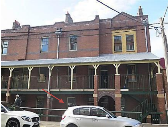
Figure 13.6 Overall façade of 46–56 Gloucester Street, showing front verandah (common property), shared guttering and downpipe on the boundary between 54C and 56, and flat 56 Gloucester Street marked with an arrow (Source: GML Heritage, July 2016)
