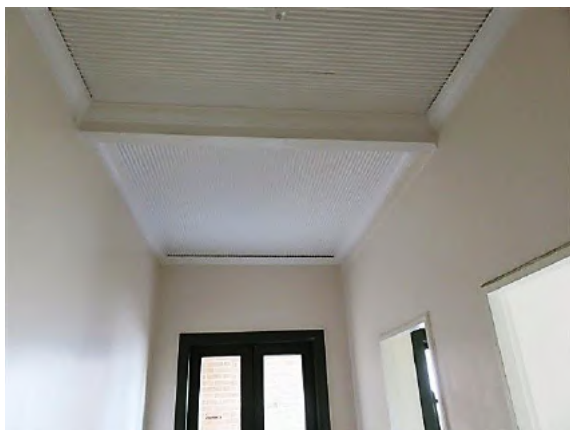
Figure 12.38 Second floor landing ceiling (space 2.1) showing the ripple iron ceiling running in two different directions either side of the beam—54C / 46–56 Gloucester Street. (Source: GML Heritage, July 2016)
