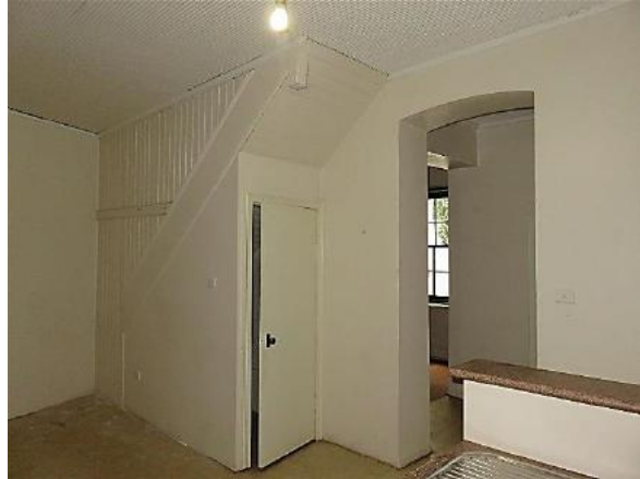
Figure 7.27 Kitchen (Space LG.2), showing original timber boarding to stair and later stair cupboard addition—52 / 46–56 Gloucester Street. (Source: GML Heritage, July 2016)
