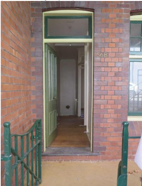
Figure 15.8 Front entry porch showing wrought iron gate with original gate latch, entry door with fanlight, slate threshold, brick arched heads over—56B / 46–56 Gloucester Street. (Source: GML Heritage, July 2016)
