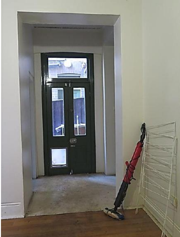
Figure 7.26 Timber floor in dining room (space LG.1) and vinyl floor in former porch. The half-glazed doors and fanlight are late 20 th century—52 / 46–56 Gloucester Street. (Source: GML Heritage, July 2016)
