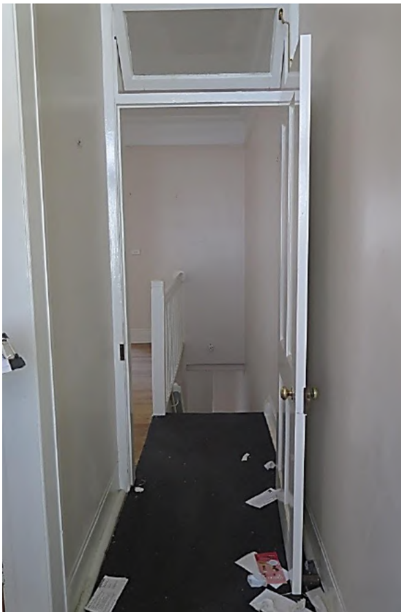
Figure 13.12 Entry (space G.1) of 56 / 46–56 Gloucester Street, showing carpeting over timber floor, cement run skirtings, and timber door frame with fanlight to the living room (space G.3). (Source: GML Heritage, June 2016)
