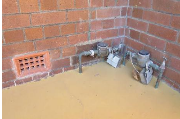
Figure 3.11 The front yard (space E.1) showing terracotta wall vents as typical in all external spaces, concrete yard paving and twentieth century water meters—48 / 46–56 Gloucester Street. (Source: GML Heritage, May 2016)
