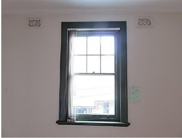
Figure 8.50 Original double hung timber window in the front room (space 2.4) flanked by a pair of decorative plaster wall vents—52A / 46–56 Gloucester Street. (Source: GML Heritage, July 2016)
