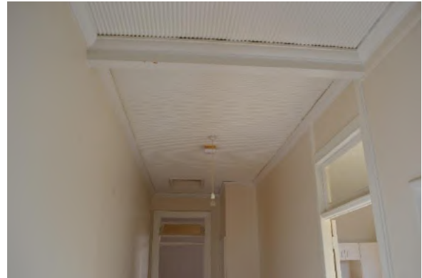
Figure 6.35 Second floor landing ceiling (space 2.1)—50A / 46–56 Gloucester Street, showing the ripple iron ceiling laid in different directions on either side of the transverse I-beam. (Source: GML Heritage, July 2016)
