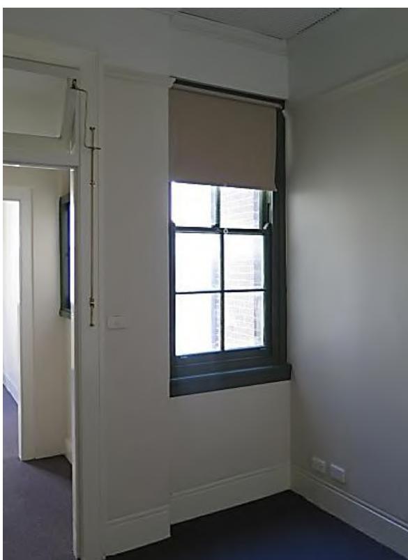
Figure 4.28 Timber double-hung sash window in living room (space 1.3), also showing the original run skirting, picture rail and timber cornice—48A / 46–56 Gloucester Street. (Source: GML Heritage, May 2016)
