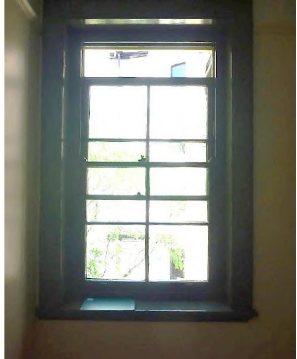
Figure 1.23 Original timber double-hung window to the living room (space G.3)—46/46–56 Gloucester Street. (Source: GML Heritage, July 2016)
