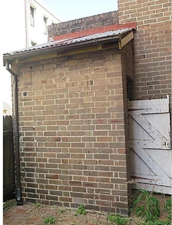
Figure 13.41 External WC (space E.3) with skillion roof, timber ledged and sheeted door, brick parapet and copper rainwater goods—56 / 46–56 Gloucester Street. (Source: GML Heritage, July 2016)
