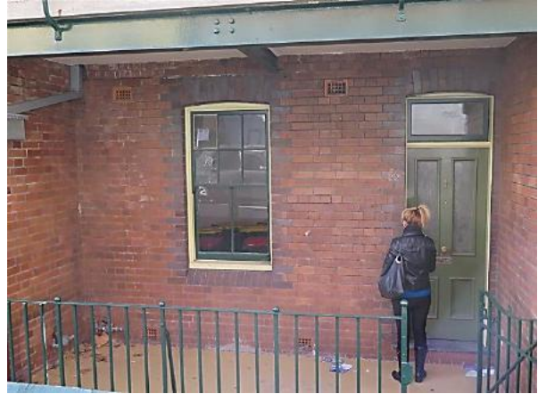
Figure 13.7 Front porch of western façade showing original casement window and timber panel door with fanlight. The steel beam supports the verandah above—56 / 46–56 Gloucester Street. (Source: GML Heritage, July 2016)
