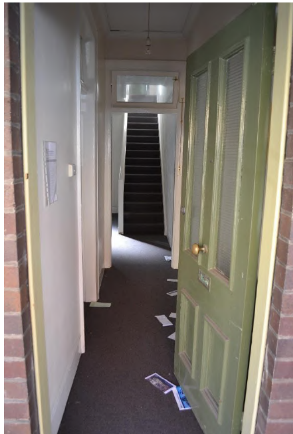
Figure 6.17 Entrance hall (space 1.1)—50A / 48–56 Gloucester Street, showing the ripple iron ceiling, cement run skirtings, moulded timber cornice and carpeted timber floor. (Source: GML Heritage, July 2016)
