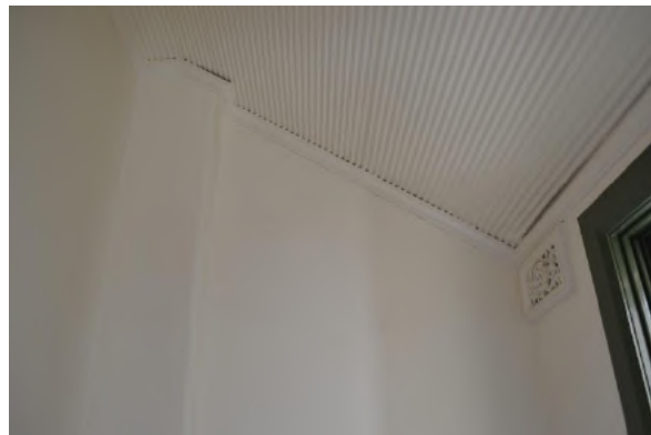
Figure 6.39 Laundry (space 2.2) showing original raked ripple iron ceiling, decorative wall vent and timber cornice—50A / 48–56 Gloucester Street. (Source: GML Heritage, July 2016)
