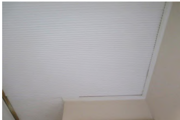
Figure 15.41 Kitchen ceiling (space LG.2) showing the original ripple iron ceiling and timber cornice—56B / 46–56 Gloucester Street. (Source: GML Heritage, July 2016)
