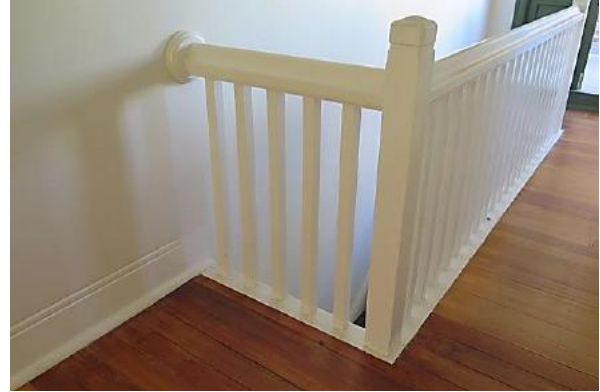
Figure 4.43 Hall (space 2.1) showing timber balustrade, newel post and handrail, original cement run skirtings and quad mould and timber floor—48A / 46–56 Gloucester Street. (Source: GML Heritage, May 2016)
