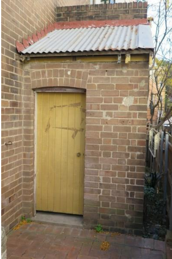
Figure 3.46 The rear yard (space E.2) and store in former external WC (space E.3) showing corrugated iron roof, exposed rafter eaves, brick parapet and walls, brick arched doorway and timber boarded door—48 / 46–56 Gloucester Street. (Source: GML Heritage, May 2016)
