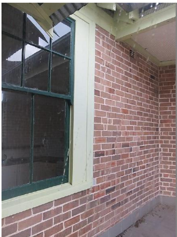
Figure 8.12 Roof terrace (space E.1) showing the double hung timber window to the kitchen, common brickwork and the tiled floor—52A / 46–56 Gloucester Street. (Source: GML Heritage, July 2016)
