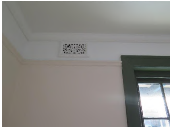
Figure 11.13 Front bedroom (space G.2) showing decorative wall vent, timber picture rail and timber cornice—54B / 46–56 Gloucester Street. (Source: GML Heritage, July 2016)
