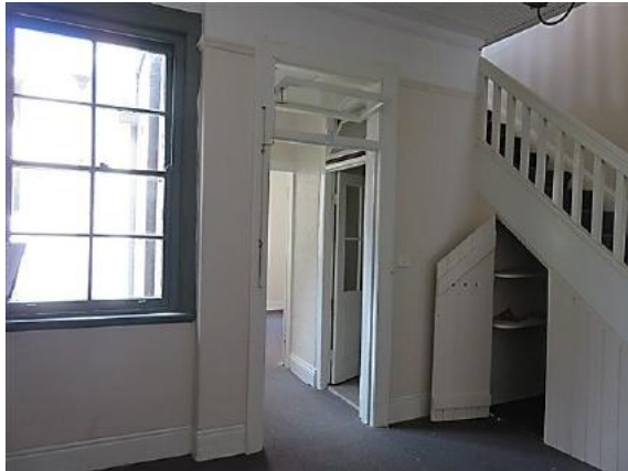
Figure 14.22 Living room (space 1.3) showing the original double hung window with four pane sashes, and original doorframe with fanlight above—56A / 46–56 Gloucester Street. (Source: GML Heritage, July 2016)
