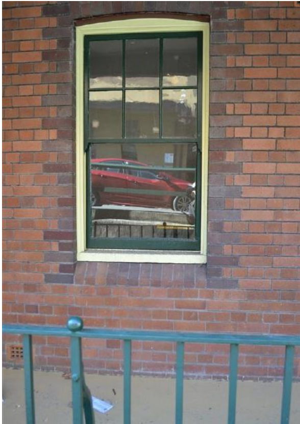
Figure 5.10 Double-hung window with chamfered brick sill, twenty-first century glass (lower sash) and dark brick surround—50 / 46–56 Gloucester Street (Source: GML Heritage, June 2016)
