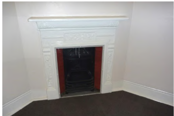
Figure 4.48 An original cast-iron chimney piece and grate (second floor level, Flat 54). The skirting is run in the wall render. (Source: GML 2015)
