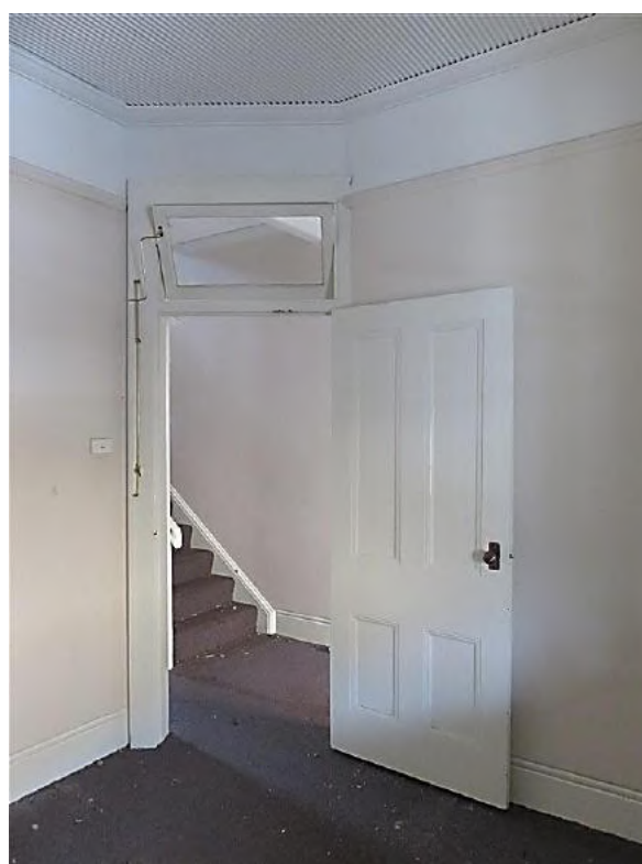
Figure 8.21 Front bedroom (space 1.2) showing the four panel sunk moulded timber door, ripple iron ceiling, reproduction mechanism, timber picture rail and moulded timber cornice—52A / 46–56 Gloucester Street. (Source: GML Heritage, July 2016)
