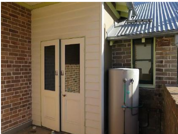
Figure 14.14 Rear wall of the flat opening onto the roof terrace (space E.1), showing recent weatherboard wall, pair of half glazed doors and rendered finish to stair hall wall. The window is also recent, replacing a previous door—56A / 46–56 Gloucester Street. (Source: GML Heritage, July 2016)
