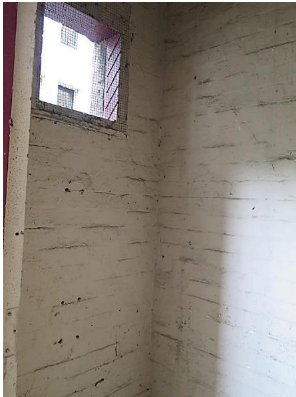
Figure 9.39 Interior of WC showing rendered painted brick (space E.3)—54 / 46–56 Gloucester Street. (Source: GML Heritage, July 2016)
