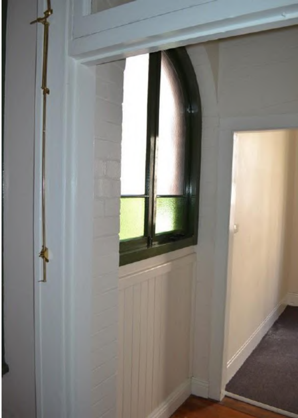
Figure 5.22 Infilled former rear porch opening (space G.4), with casement window and modern T&G boarding below—50 / 46-56 Gloucester Street. (Source: GML Heritage, June 2016)
