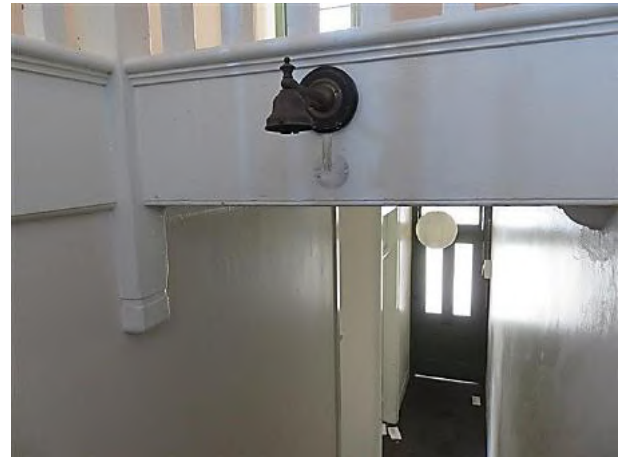
Figure 16.37 Original gas light fixture over the stairs (space 1.7). Bottom of stair newel post extends down stair hall wall below ceiling—56C / 46–56 Gloucester Street. (Source: GML Heritage, July 2016)
