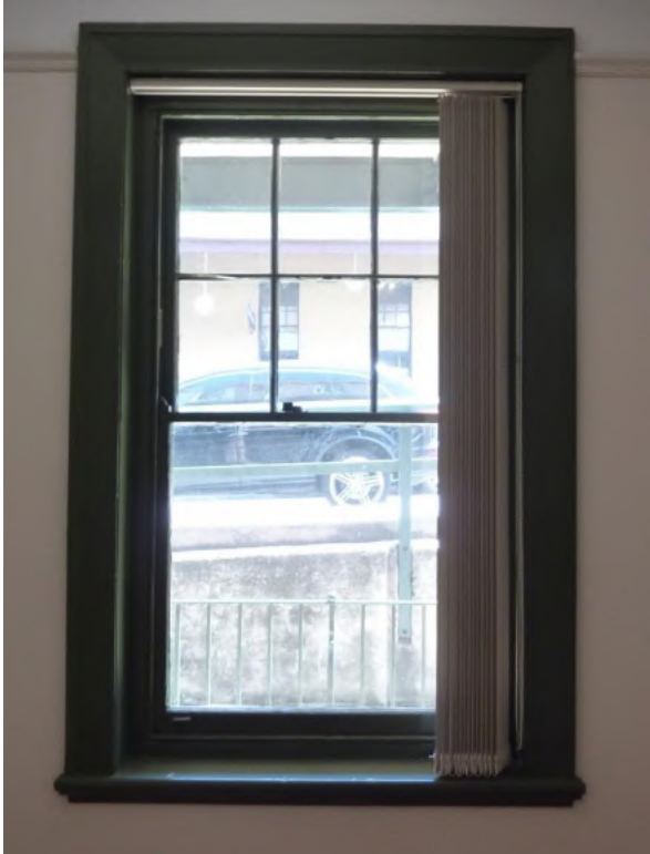
Figure 3.18 Timber double-hung sash window, architrave and sill board in the front bedroom (space G.2)—48 / 46–56 Gloucester Street. (Source: GML Heritage, November 2015)
