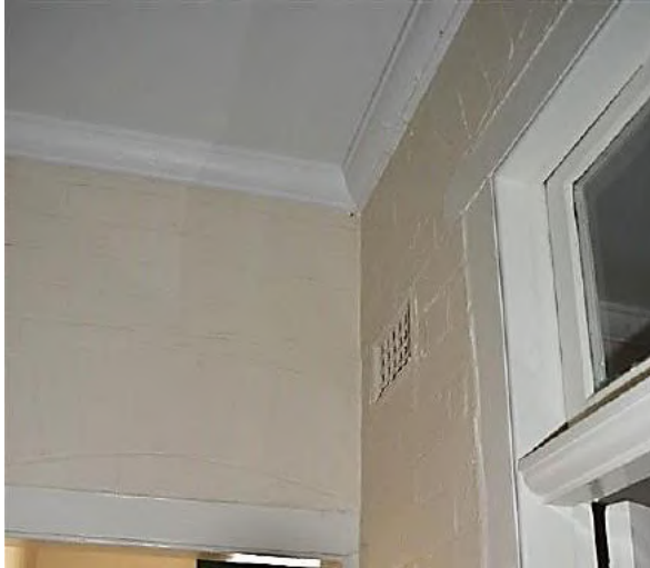
Figure 9.18 Former infilled porch (space G.4) showing the plaster ceiling and brick arches above the doorways—54 / 46–56 Gloucester Street. (Source: GML Heritage, July 2016)
