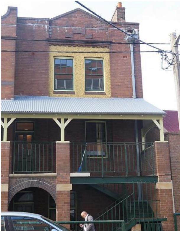
Figure 16.6 Western (front) façade of 56C Gloucester Street, showing western verandah and stair access (common property), pebble dash render to central portion of second floor wall, and decorative brick cornice and checkerboard pattern panel to triangular parapet. A cast metal rainwater head and downpipe extend down the face of the wall. (Source: GML Heritage, July 2016)
