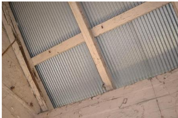
Figure 1.53 Ceiling of the external store (space E.3) formed by the underside of the corrugated metal roof—46/46–56 Gloucester Street. (Source: GML Heritage, July 2016)
