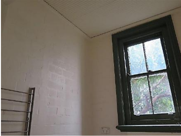
Figure 7.34 Interior of laundry showing timber double hung sash window, painted brick walls and original ripple iron ceiling. (Source: GML Heritage, July 2016)
