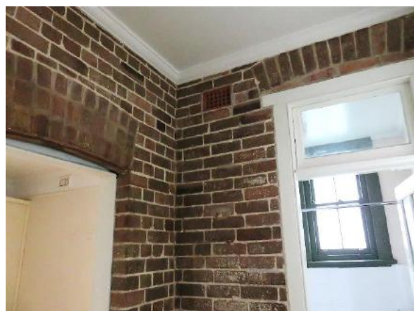
Figure 7.17 Former rear porch (space G.4) showing the brick arched heads above the doors to the rear bedroom (space G.6) and bathroom (space G.5). the latter appears to have been altered—52 / 46–56 Gloucester Street. (Source: GML Heritage, July 2016)
