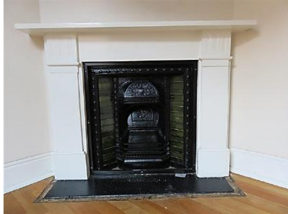
Figure 10.49 Fireplace in space 2.4 with early chimney piece, cast iron grate with tiled sides, and concrete hearth—54A / 46–56 Gloucester Street. (Source: GML Heritage, July 2016)
