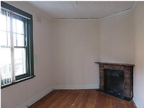
Figure 8.48 Front room on second floor (space 2.4) showing the original double hung window, ripple iron ceiling, cement skirtings, timber floor and marble chimney piece to fireplace—52A / 46–56 Gloucester Street. (Source: GML Heritage, July 2016)
