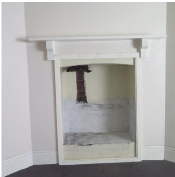
Figure 4.53 The cast-iron range has been removed from Flat 54A (first floor level). (Source: GML 2016)
