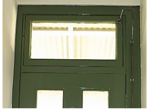
Figure 4.19 Pivot fanlight over the front door with original mechanism (space 1.1)—48A / 46–56 Gloucester Street. (Source: GML Heritage, May 2016)
