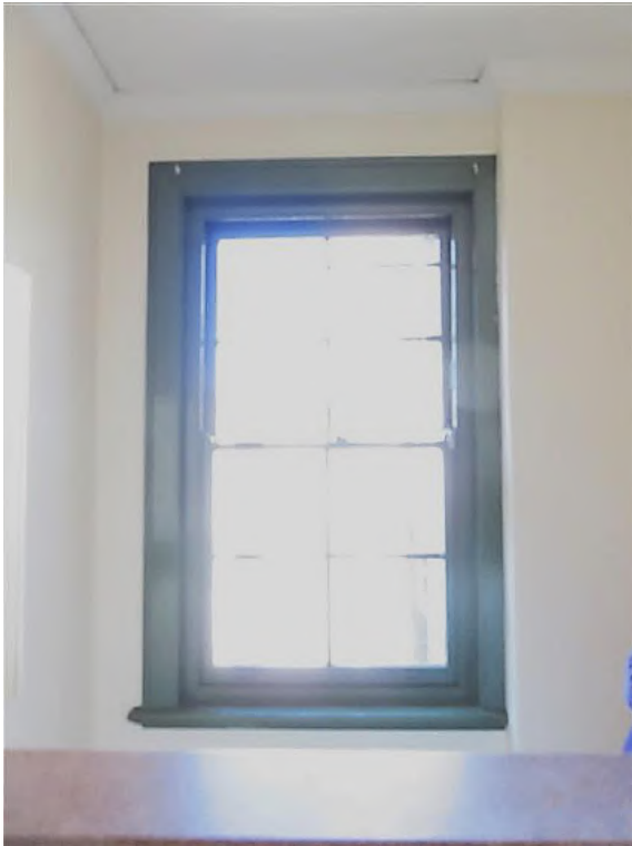
Figure 14.45 Original double hung sash window in the kitchen (space 2.3) with original architraves and sill board—56A / 46–56 Gloucester Street. (Source: GML Heritage, July 2016)
