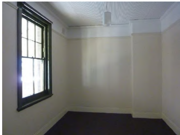
Figure 2.22 Front bedroom (space 1.2) showing timber double hung sash window, moulded timber picture rail and ripple iron ceiling with moulded timber cornice—46A / 46–56 Gloucester Street. (Source: GML Heritage, July 2016)
