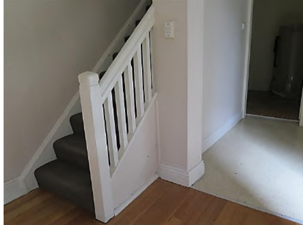
Figure 9.23 Original stair at lower ground-floor level with closed string, simple square balusters and newel post and moulded handrail (space G.7/ LG.1)—54 / 46–56 Gloucester Street. (Source: GML Heritage, July 2016)
