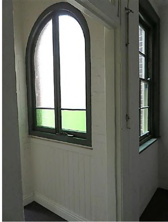
Figure 12.27 Infill to original arched opening of former porch in rear wing (space 1.4) consists of a pair of casement windows and vertical boarded panel below. The timber skirting is late twentieth century. (Source: GML Heritage, July 2016)
