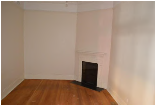
Figure 1.16 Front bedroom (space G.2) showing the timber floors, cement run skirting and fireplace—46/46–56 Gloucester Street. (Source: GML Heritage, July 2016)
