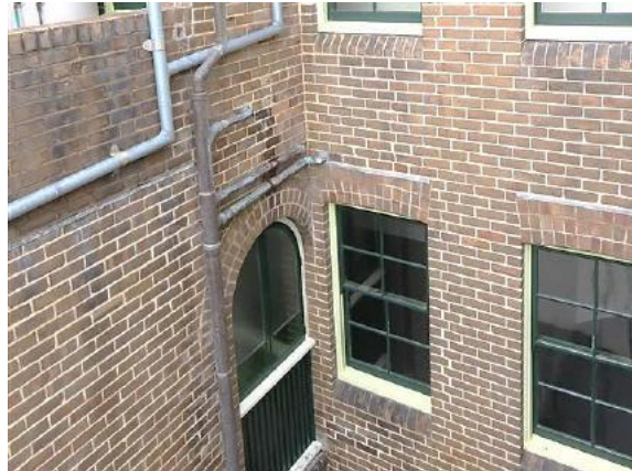
Figure 14.11 Original brick arched opening to former porch in rear wing (first floor level, now infilled with window and solid balustrade) and typical triple brick arched head over rear window opening—56A / 46–56 Gloucester Street. (Source: GML Heritage, July 2016)
