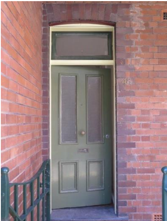
Figure 3.12 The four-panel front door with bolection moulds to bottom panels and wired glass to top panels, dark brick surround, arched head and slate threshold—48 / 46–56 Gloucester Street. (Source: GML Heritage, May 2016)
