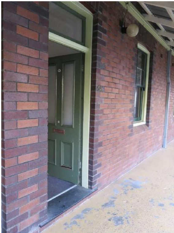
Figure 12.8 Front elevation of flat 54C from verandah showing original front door with slate threshold and fanlight over—54C / 46–56 Gloucester Street. (Source: GML Heritage, July 2016)
