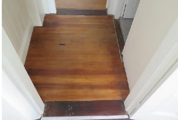
Figure 3.27 The raised timber floor of the former rear porch (space G.4) with original timber thresholds and nosings to steps—48 / 46–56 Gloucester Street. (Source: GML Heritage, May 2016)
