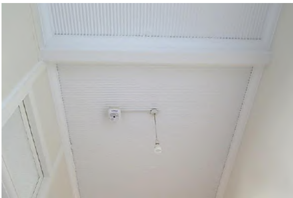
Figure 4.44 Original ripple iron ceilings with original cornice and exposed steel transverse I-beam in hall (space 2.1)—48A / 46–56 Gloucester Street. (Source: GML Heritage, May 2016)
