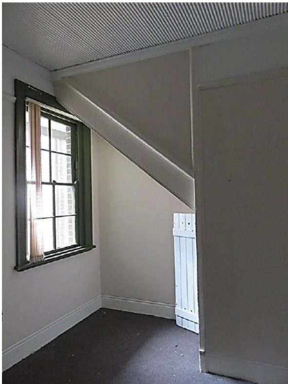
Figure 8.28 Living room (space 1.3) showing the timber double hung sash window and closed string staircase, with stair partition (possibly coke-breeze) on the right—52A / 46–56 Gloucester Street. (Source: GML Heritage, July 2016)
