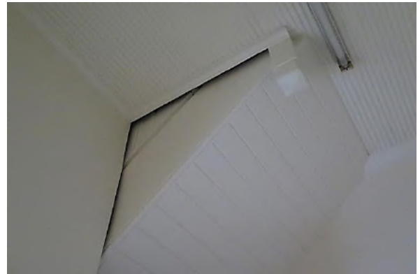
Figure 13.35 Laundry (space LG.3) showing boarded soffit to stair, with bottom of newel post extending down through ceiling. The ceiling is ripple iron—56 / 46–56 Gloucester Street. (Source: GML Heritage, July 2016)
