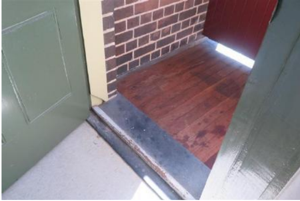
Figure 4.41 The rear balcony to Flat 54A showing the slate threshold and original timber boarded floor (second floor level). (Source: GML 2016)
