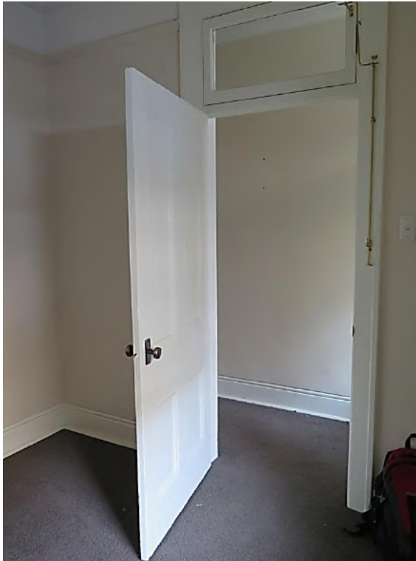
Figure 9.12 Four-panel timber door with fanlight above and reproduction mechanism between the front bedroom (space G.2) and entry (space G.1)—54 / 46–56 Gloucester Street. (Source: GML Heritage, July 2016)
