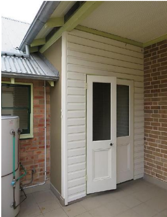
Figure 12.16 Rear wall of the flat opening onto the roof terrace (space E.1), showing recent weatherboard wall, pair of half glazed doors and rendered finish to stair hall wall. The window is also recent, replacing a previous door—54C / 46–56 Gloucester Street. (Source: GML Heritage, July 2016)
