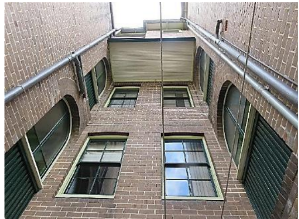
Figure 7.41 Round-arched window of the former rear porch on the southern elevation showing modern infill. Also original brick arched head to and chamfered window sill to the window of space G.3—52 / 46–56 Gloucester Street. (Source: GML Heritage, July 2015)
