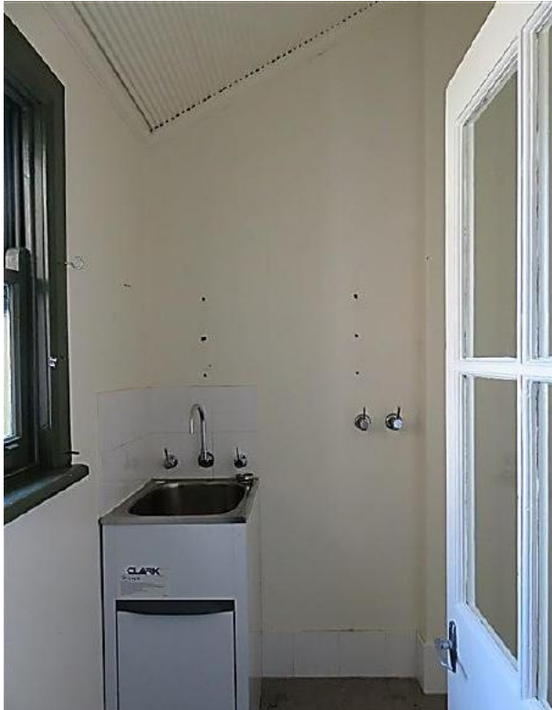
Figure 16.42 Laundry (space 2.2) showing the original raked ripple iron ceiling and modern fitout—56C / 46–56 Gloucester Street. (Source: GML Heritage, July 2016)
