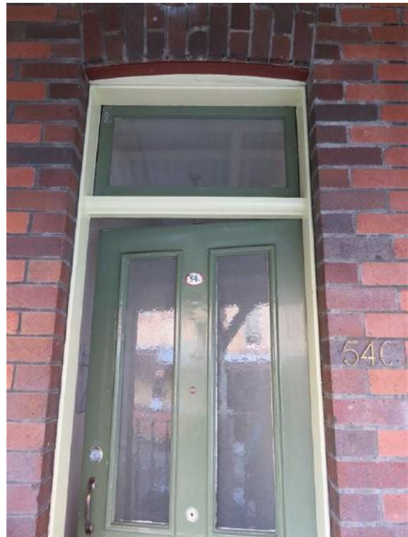
Figure 12.9 Four panel entrance door with bolection moulds, obscured glass to upper panels and fanlight over. The door has an early enamelled number plate—54C / 46–56 Gloucester Street. (Source: GML Heritage July 2016)
