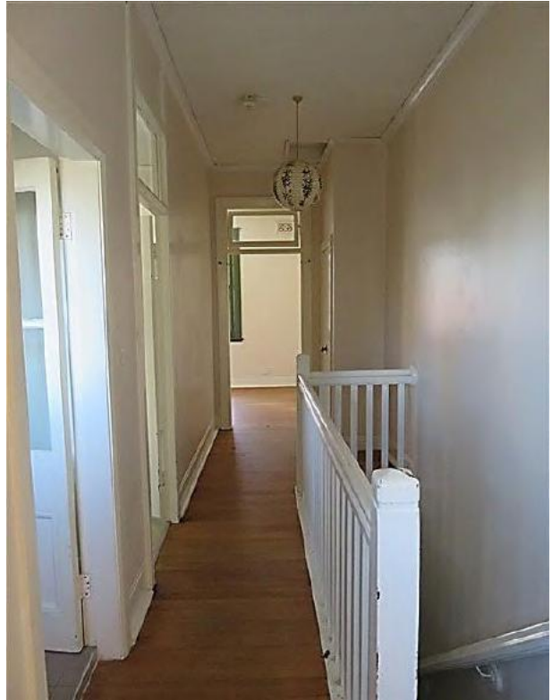
Figure 16.39 Second floor landing (space 2.1) looking west, showing the timber balustrade with moulded handrail, square balusters and chamfered top to newel post, cement rendered skirting with quad moulding—56C / 46–56 Gloucester Street. (Source: GML Heritage, July 2016)
