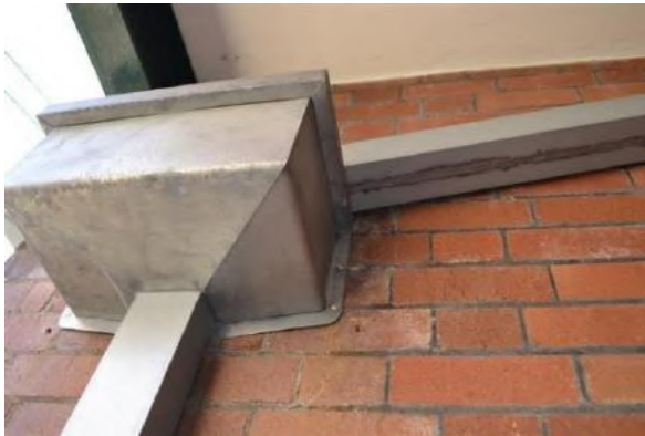
Figure 5.8 updated rain water collection system on the front porch (space E.1)—50 / 46–56 Gloucester Street. (Source: GML Heritage, June 2016)
