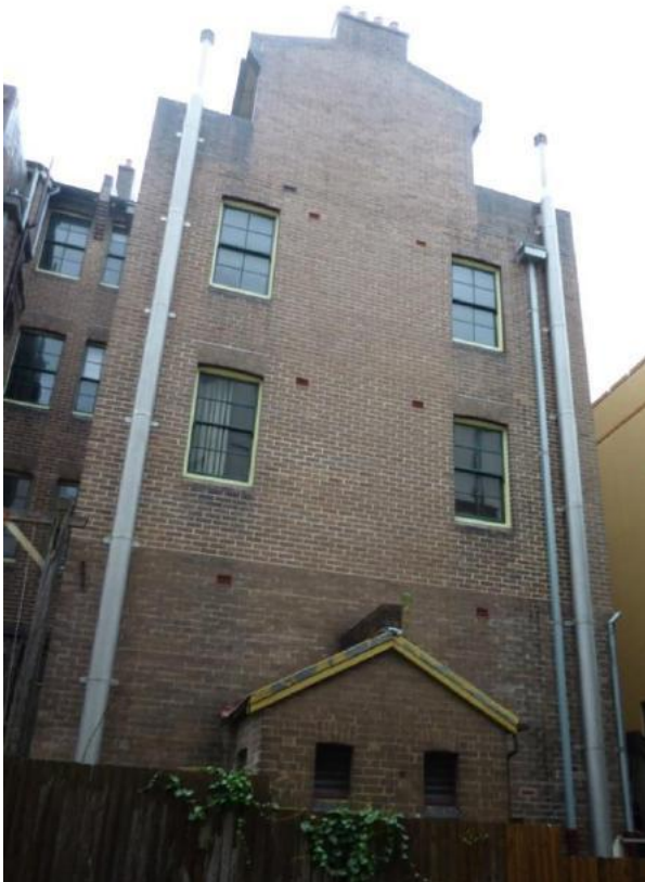
Figure 4.11 Eastern end of rear wing (Flats 46A and 48A) showing former external WCs attached to rear wall, solid brick balustrades to roof-top terraces, corbelled brickwork to the ends of eaves and reconstructed garbage chutes. (Source: GML 2015)
