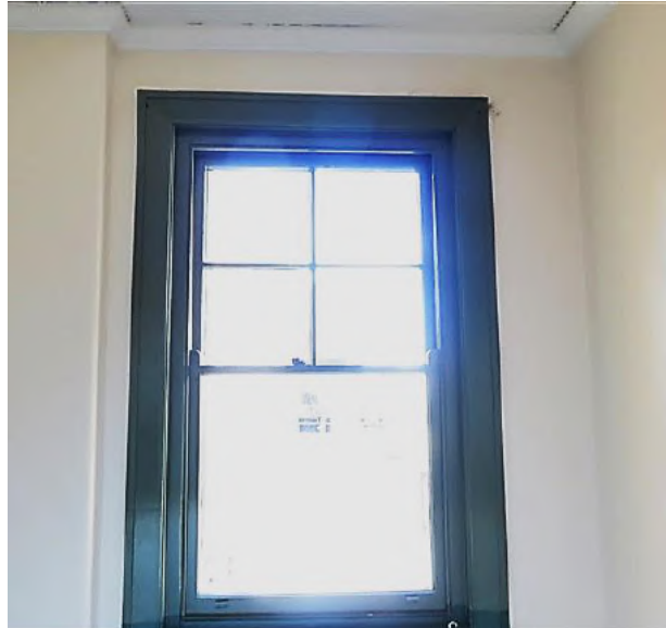
Figure 16.47 Original double hung window with four-pane upper sash (original) and single pane bottom sash (replaced), and original architrave—56C / 46–56 Gloucester Street. (Source: GML Heritage, July 2016)
