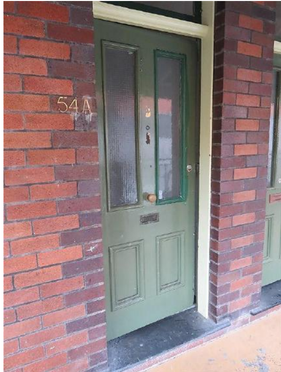
Figure 10.9 Four panel entrance door with bolecion moulds, wired glass to the upper panels and original slate threshold—54A / 46–56 Gloucester Street. (Source: GML Heritage, July 2016)
