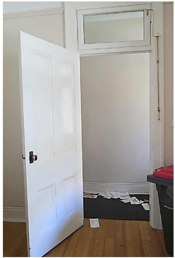
Figure 13.13 Four-panel timber door with fanlight above with reproduction mechanism—located between front bedroom (space G.2) and entry (space G.1). the cement run skirting and timber picture rail are also visible—56 / 46–56 Gloucester Street. (Source: GML Heritage, July 2016)
