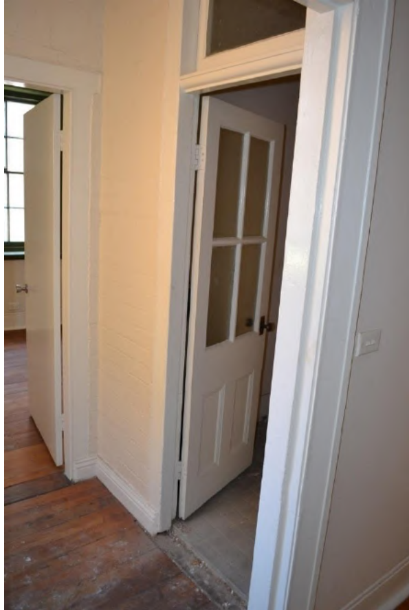
Figure 1.27 Infilled former rear porch opening (space G.4) showing half-glazed timber door to bathroom with original architraves—46/46–56 Gloucester Street. (Source: GML Heritage, July 2016)
