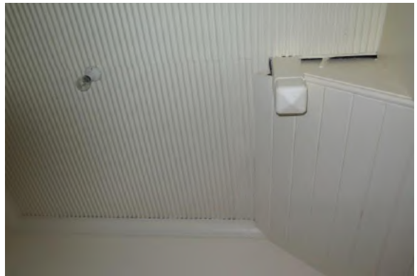
Figure 3.45 The laundry (space LG.3) showing original ripple iron ceilings and timber cornices, with boarded stairs and timber pendant newel post—48 / 46–56 Gloucester Street. (Source: GML Heritage, May 2016)
