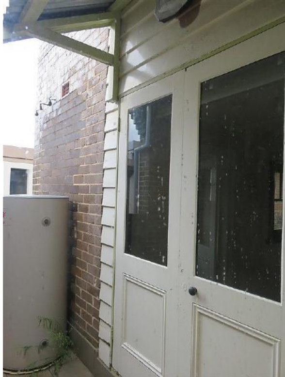
Figure 8.15 Half glazed doors leading from the roof terrace to the second floor landing. Note the later brickwork on the wall of the laundry where former door blocked up—52A / 46–56 Gloucester Street. (Source: GML Heritage, July 2016)
