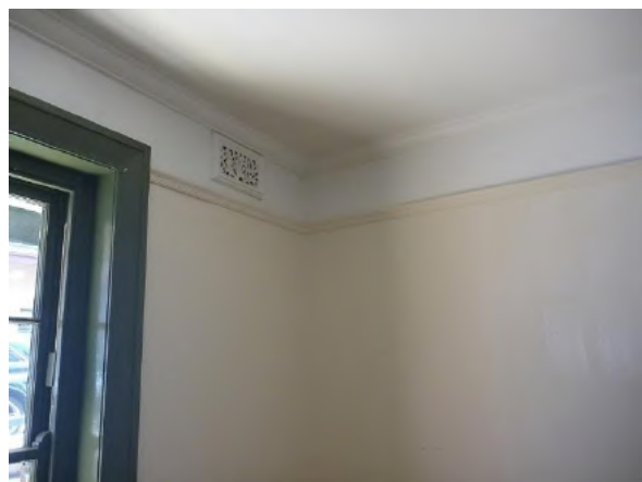
Figure 5.17 Front bedroom (space G.2) showing the moulded timber picture rail and cornice, decorative plaster wall vent and plaster board ceiling—50 / 46–56 Gloucester Street. (Source: GML Heritage, June 2016)
