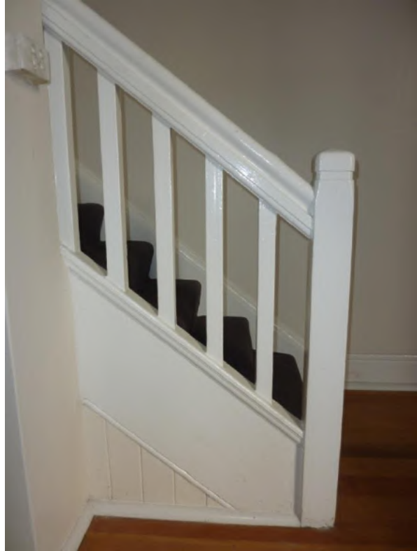
Figure 3.35 The stair (space G.7) showing original timber balustrade, newel post and stringer and original/refinished timber floor—48 / 46–56 Gloucester Street. (Source: GML Heritage, May 2016)
