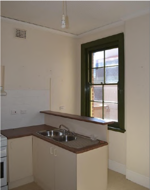
Figure 2.45 Kitchen (space 2.3) showing the original ripple iron ceiling, moulded timber cornice and original double hung window joinery. The fitout is modern—46A / 46–56 Gloucester Street. (Source: GML Heritage, July 2016)
