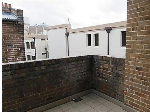
Figure 10.17 Roof terrace (space E.1) showing tiled floor and evidence of the original garbage chute (bricked up)—54A / 46–56 Gloucester Street. (Source: GML Heritage, July 2016)
