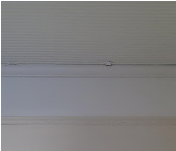
Figure 4.32 Original ripple iron ceiling, picture rail, timber cornice and early gas pipe/fitting in the ceiling of the living room (space 1.3)—48A / 46–56 Gloucester Street. (Source: GML Heritage, May 2016)
