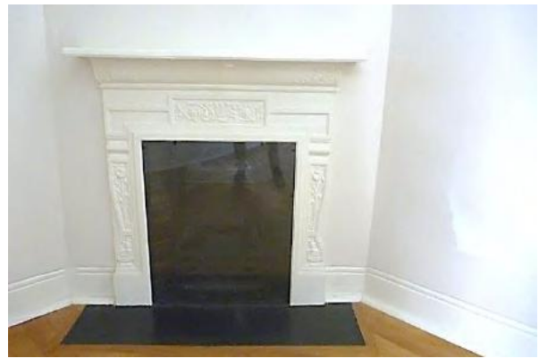
Figure 1.17 Original cast-iron chimney piece and grate (covered with Perspex) in the front bedroom (space G.2)—46/46–56 Gloucester Street. (Source: GML Heritage, July 2016)
