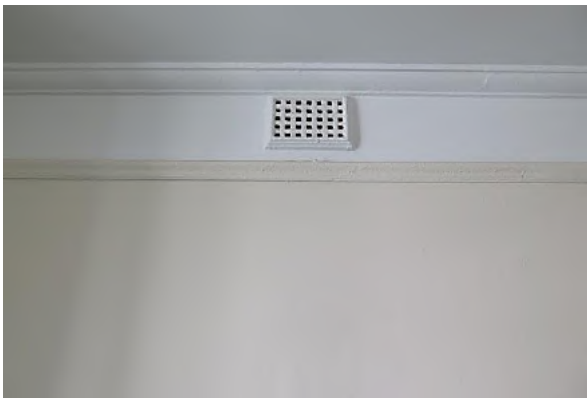
Figure 3.20 Grille pattern wall vents (common to interiors throughout 48 Gloucester Street) with original timber picture rail and timber cornice in the front bedroom (space G.2)—48 / 46–56 Gloucester Street. (Source: GML Heritage, May 2016)
