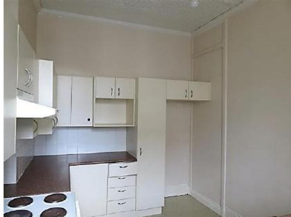
Figure 12.43 Kitchen (space 2.3) showing modern refit, ripple iron ceiling, timber cornice and cement run skirting. The original door frame survives in the wall at the northwest corner of the room—54C / 46–56 Gloucester Street. (Source: GML Heritage, July 2016)
