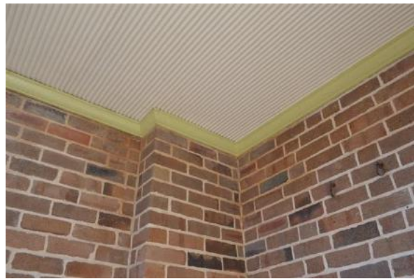
Figure 2.16 Original ripple iron ceiling and timber cornice to the terrace roof Rear roof slope and chimney and parapet (common property)—46A / 46–56 Gloucester Street. (Source: GML Heritage, May 2016)
