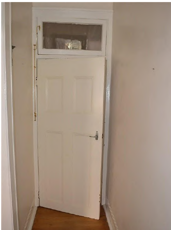
Figure 5.14 Four panel timber door, with fanlight above leading to the dining room (space G.3) from the entry hall (space G.1)—50 / 46–56 Gloucester Street. (Source: GML Heritage, June 2016)
