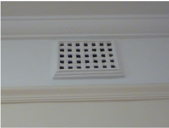
Figure 4.59 Plaster grid pattern vent and picture rail (Flat 48). (Source: GML 2015)
