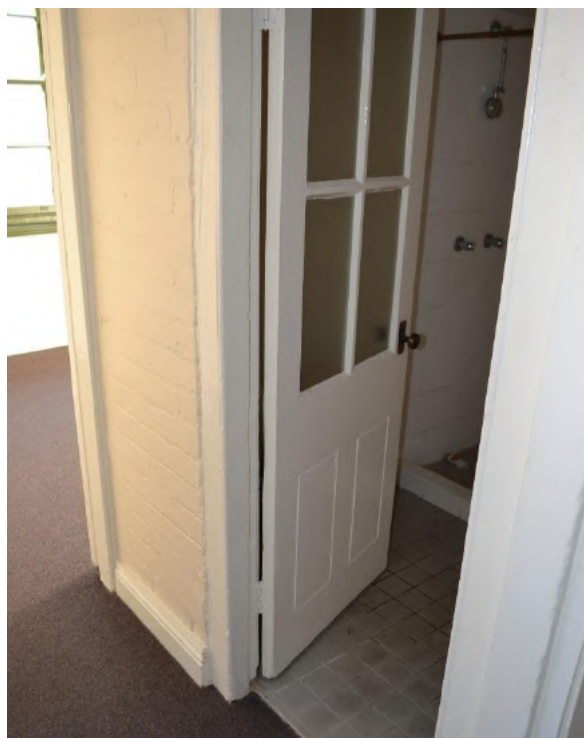
Figure 6.27 Original half-glazed door to the bathroom (space 1.5)—50A / 48–56 Gloucester Street. (Source: GML Heritage, July 2016)
