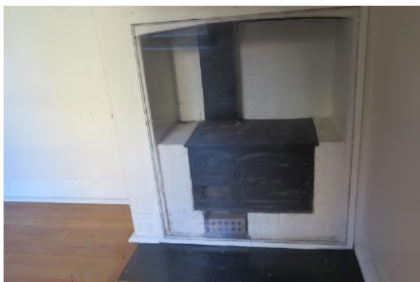
Figure 15.36 Cast-iron cooking range in fireplace (LG.1) (former kitchen). The range is covered by a perspex screen—56B/46–56 Gloucester Street—56B / 46–56 Gloucester Street. (Source: GML Heritage, July 2016)
