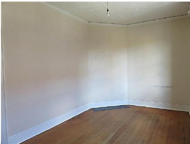
Figure 16.48 Front room on the second floor (space 2.4). The fireplace has been blocked up and chimney piece removed. Concrete hearth remains—56C / 46–56 Gloucester Street. (Source: GML Heritage, July 2016)
