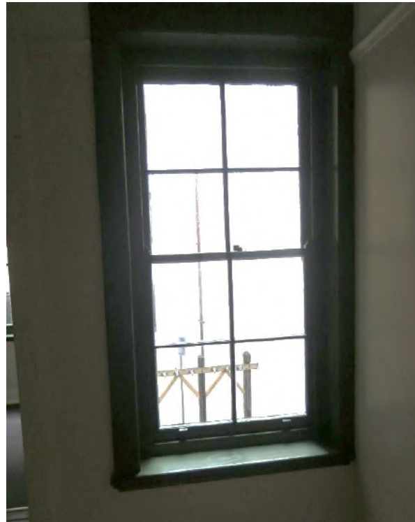
Figure 11.17 Double-hung sash window in the living room (space G.3)—54B / 46–56 Gloucester Street. (Source: GML Heritage, July 2016)
