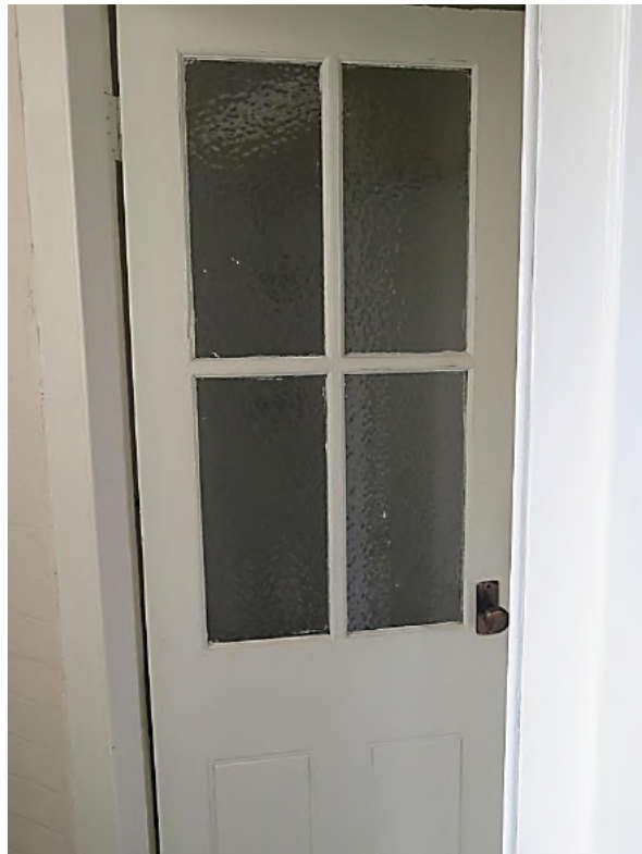
Figure 9.17 Half-glazed timber door to the bathroom (space G.5)—54 / 46–56 Gloucester Street. (Source: GML Heritage, July 2016)
