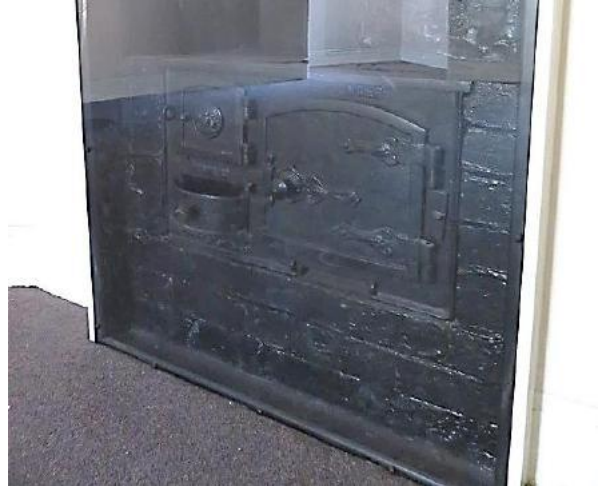
Figure 8.27 Original cast iron range in the living room (space 1.3)—52A / 46–56 Gloucester Street. (Source: GML Heritage, July 2016)
