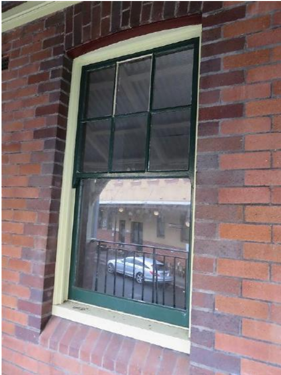
Figure 10.8 Double hung timber sash window, with six pane top sash and single pane bottom sash, contrasting brick surround and chamfered brick window sill—54A / 46–56 Gloucester Street. (Source: GML Heritage, July 2016)
