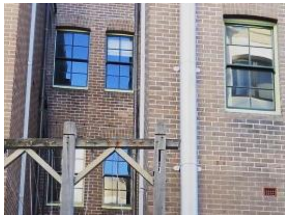
Figure 4.17 Rear façade of flat 48A showing double hung sash windows with arched brick heads—48A / 46–56 Gloucester Street. (Source: GML Heritage, May 2016)
