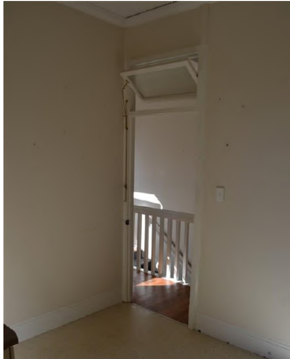
Figure 2.46 Fanlight with intact mechanism above the kitchen doorway (space 2.4) (Door is missing)—46A/46–56 Gloucester Street. (Source: GML Heritage, July 2016)
