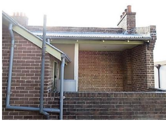
Figure 12.13 Roof terrace (space E.1) viewed from flat 56A, showing area covered by skillion roof chimney over the rear wing and brick balustrade to the roof terrace—54C / 46–56 Gloucester Street. (Source: GML Heritage, July 2016)
