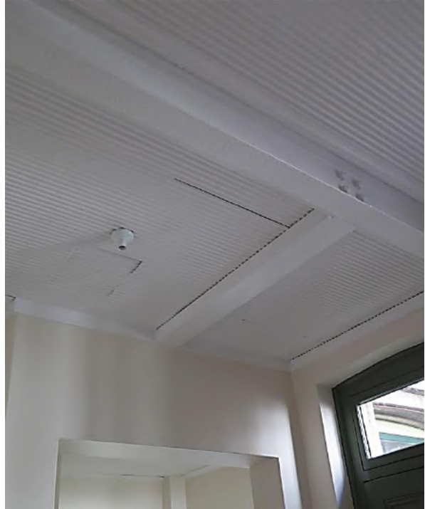
Figure 13.29 Original ripple iron ceiling and dropped ceiling over western portion of space LG.1—56 / 46–56 Gloucester Street. (Source: GML Heritage, June 2016)
