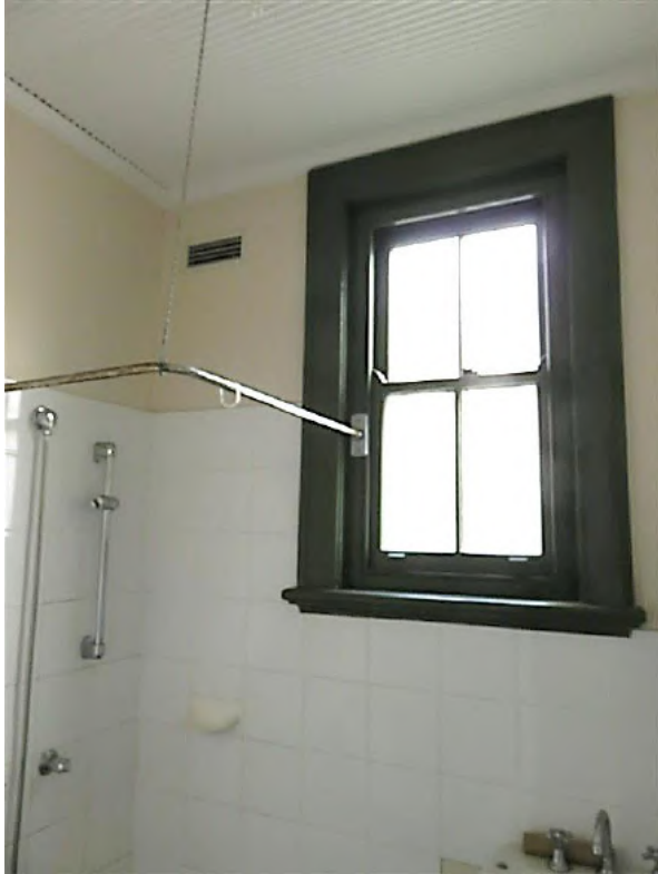
Figure 8.34 Bathroom (space 1.5) showing the ripple iron ceiling with moulded timber cornice and original timber double hung window—52A / 46–56 Gloucester Street. (Source: GML Heritage, July 2016)
