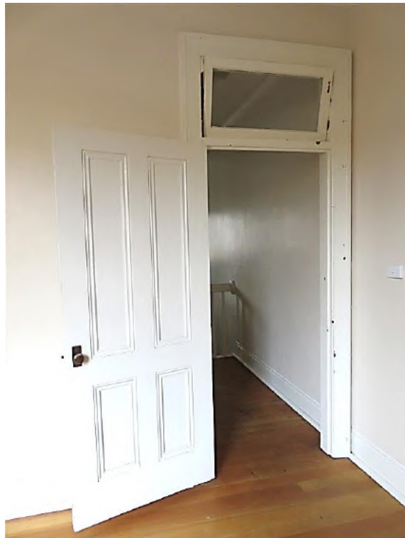
Figure 10.51 Front room on the second floor (space 2.4) showing the original four panel door with sunk moulds, set in original frame with original fanlight over and original architrave—54A / 46–56 Gloucester Street. (Source: GML Heritage, July 2016)
