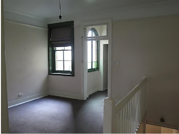
Figure 9.14 The living room (space G.3) showing cement run skirtings, timber cornice, picture rail and timber double-hung sash window—54 / 46–56 Gloucester Street. (Source: GML Heritage, June 2016)
