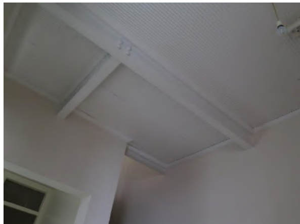
Figure 11.29 Steel beams supporting walls above and ripple iron ceiling (lower ground floor level of Flat 54B)—54B / 46–56 Gloucester Street. (Source: GML Heritage, July 2016)
