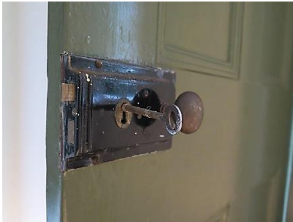
Figure 9.28 Original lock on lower ground-floor level door (space LG.1)—54 / 46–56 Gloucester Street. (Source: GML Heritage, July 2016).
