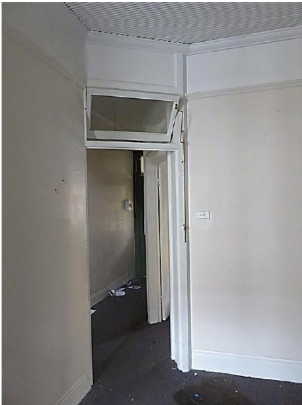
Figure 8.24 Living room (space 1.3) showing cement rendered skirtings, ripple iron ceiling and original expressed timber door frame with fanlight above— 52A / 46–56 Gloucester Street. (Source: GML Heritage, July 2016)
