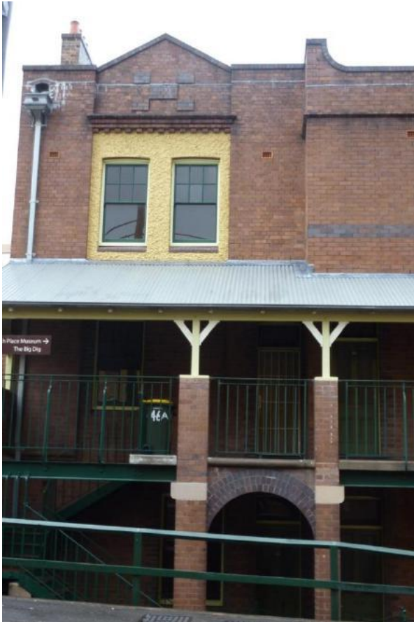
Figure 4.1 Detail of the main Gloucester Street facade, Flat 46 (ground level) and Flat 46A (first and second-floor levels), showing parapet with triangular pediment over roughcast panel, contrasting brick bands, moulded brick string courses and dentil detail, brick piers, stone bolsters and timber posts and brackets, brick arch to stair entry, corrugated skillion roof and wrought iron balustrades to the verandah. The decorative rainwater heads and rectangular downpipes are recent, but are appropriate to the building. (Source: GML 2015)
