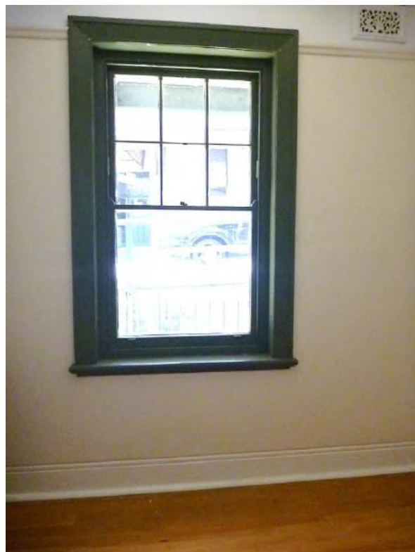
Figure 5.15 Front bedroom (space G.1) showing the timber double hung sash window, architraves, sill board and cement run skirting—50 / 46–56 Gloucester Street. (Source: GML Heritage, June 2015)
