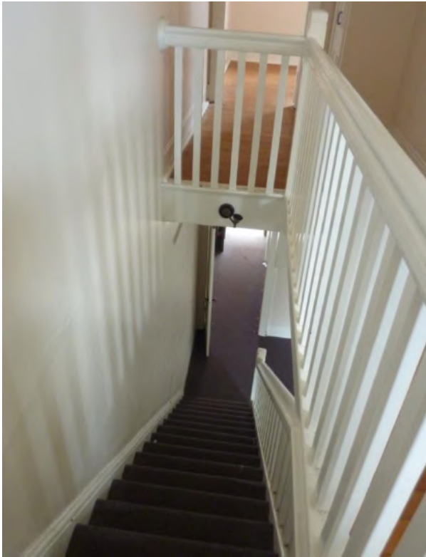
Figure 4.43 Original newel stair in the upper flat (Flat 56A) between the first and second floors. It has a closed string, simple square balusters and newel posts and moulded handrail. (Source: GML 2015)
