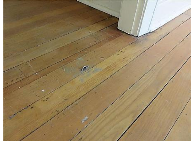
Figure 16.51 Timber floors to the second floor, with oiled finish. Metal keeper in doorway is not significant and can be removed—56C / 46–56 Gloucester Street. (source: GML Heritage, July 2016)
