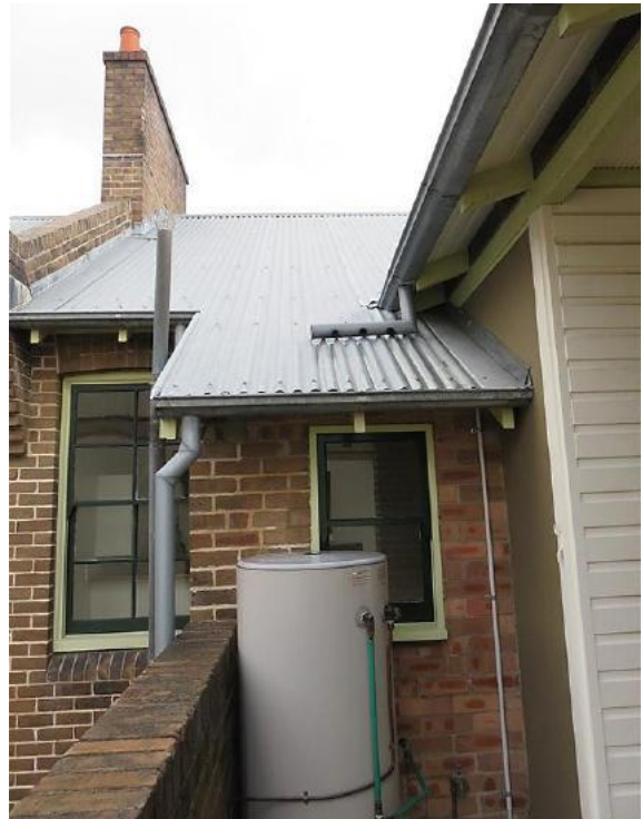
Figure 12.17 Detail of the roofline of flat 54C, showing the open rafters, corrugated metal roof and chimney with terracotta chimney pots—54C / 46–56 Gloucester Street. (Source: GML Heritage, July 2016)
