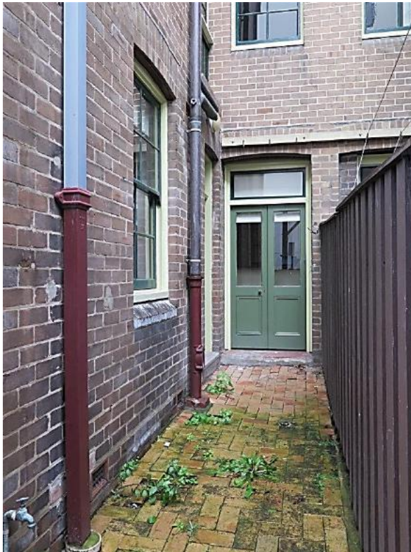
Figure 9.36 Paved rear yard (space E.2) showing rear façade and service pipes, part of reconstructed laundry hoist and later double doors—54 / 46–56 Gloucester Street. (Source: GML Heritage, July 2016)
