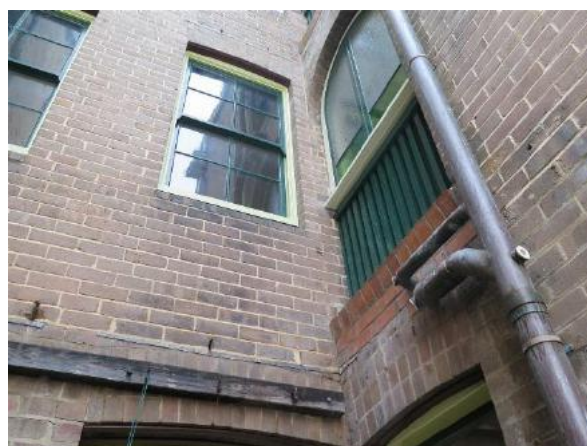
Figure 11.41 Rear wing and rear façade showing copper service pipes and later porch opening infill—54B / 46–56 Gloucester Street. (Source: GML Heritage, July 2016)
