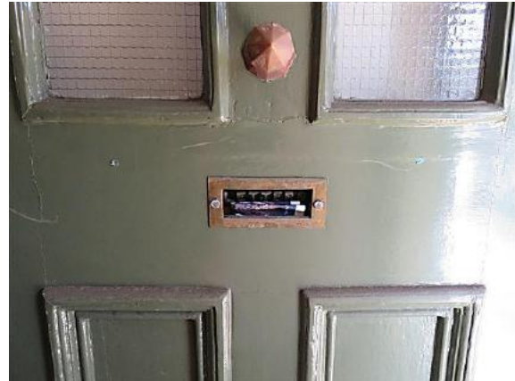
Figure 14.17 Brass door knob and letter flap in front door (not original)—56A / 46–56 Gloucester Street. (Source: GML Heritage, July 2016)
