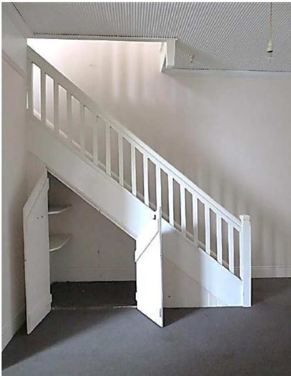
Figure 10.26 Living room (space 1.3) showing original timber stair against south wall, with closed stinger, simple square balusters, moulded handrail and newel posts—54A / 46–56 Gloucester Street. (Source: GML Heritage, July 2016)
