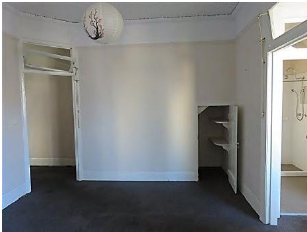
Figure 16.24 Living room (space 1.3) showing the original door frame, with fanlight dislodged from pivot fitting and broken fanlight mechanism. The room has run cement skirtings, picture rail, cornice and ripple iron ceiling. The small door opens to the space under the enclosed stairs—56C / 46–56 Gloucester Street. (Source: GML Heritage, July 2016)
