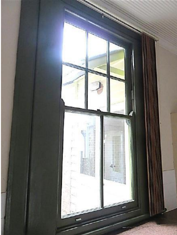
Figure 8.46 Double hung sash window to kitchen (space 2.2), with six lights over two (the window may have been relocated from elsewhere in the building)—52A / 46–56 Gloucester Street. (Source: GML Heritage, July 2016)
