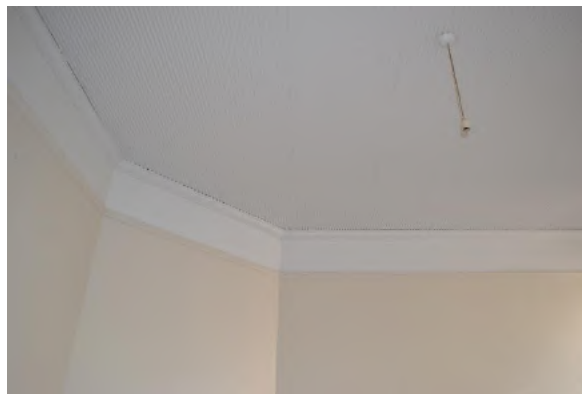
Figure 6.23 Living room (space 1.4) showing corner chimney breast, timber picture rail, cornice and ripple iron ceiling—50A / 46–56 Gloucester Street. (Source: GML Heritage, July 2016)
