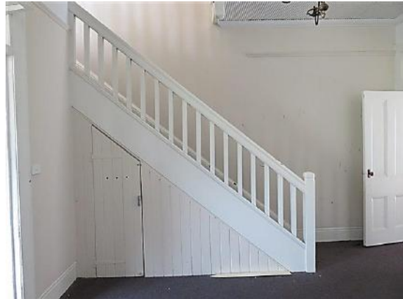
Figure 14.23 Living room (space 1.3) showing original timber stair with closed string, simple square balusters, moulded handrail and newel posts—56A / 46–56 Gloucester Street. (Source: GML Heritage, July 2016)
