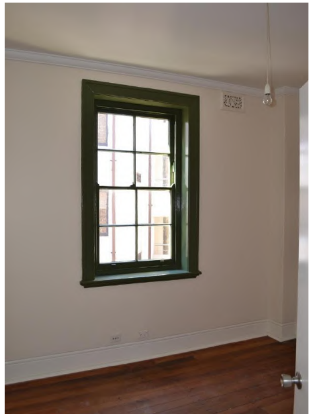
Figure 1.33 Rear bedroom (space G.6) showing timber double hung sash window, timber floor boards, cement rendered skirting and decorative plaster wall vent—46/46–56 Gloucester Street. (Source: GML Heritage, July 2016)
