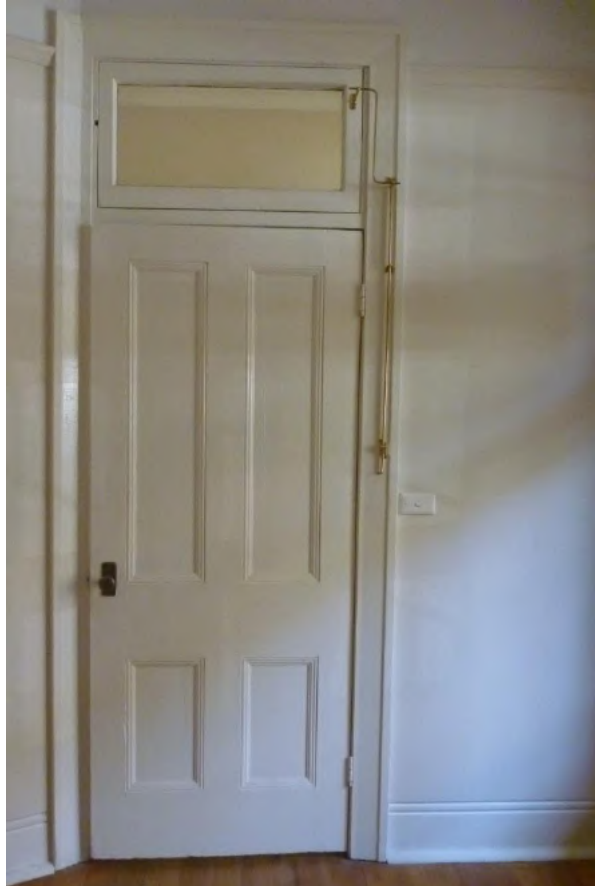
Figure 1.19 Front bedroom (space G.2) showing the timber four panel door with original fanlight—46/46–56 Gloucester Street. (Source: GML Heritage, July 2016)
