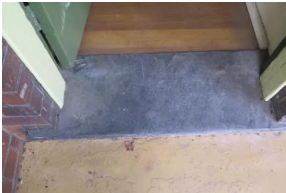
Figure 15.12 Original slate threshold to front door—56B / 46–56 Gloucester Street. (Source: GML Heritage, July 2016)
