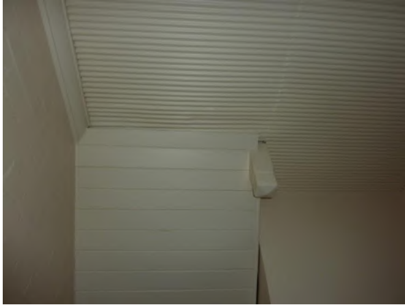
Figure 4.45 Underside of the stair showing the bottom of newel post and timber-boarded soffit (lower ground floor level, Flat 48). Note the ripple iron ceiling and timber cornice. (Source: GML 2015)
