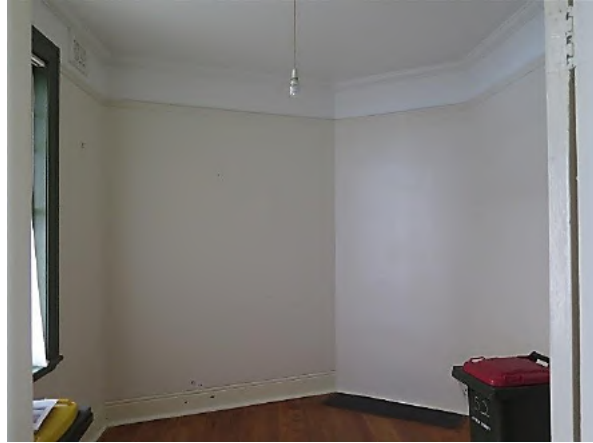
Figure 7.11 Front bedroom (space G.2) showing timber floors, rendered wall finishes, rendered cement skirting, timber picture rail, fibrous plaster cornice and plasterboard ceiling. The corner fire place is blocked up but retains its original concrete hearth—52 / 46–56 Gloucester Street. (Source: GML Heritage, July 2016)
