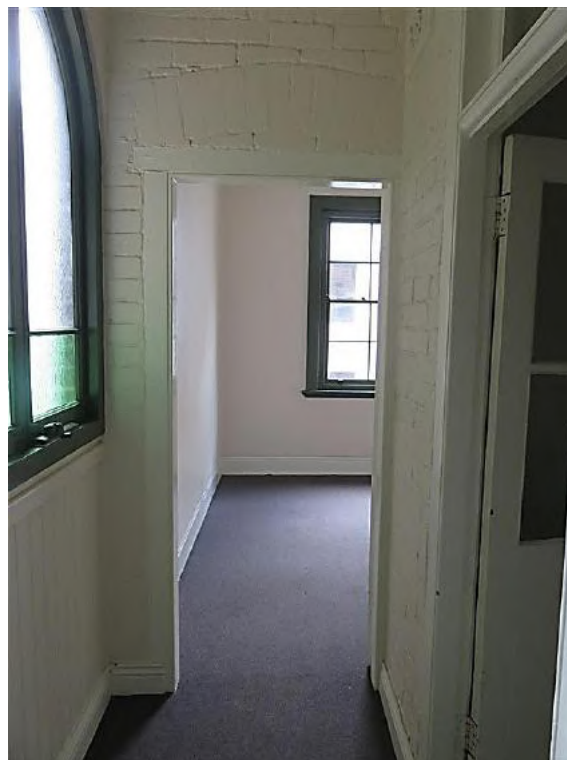
Figure 10.29 Original arched opening to former porch in rear wing (space 1.4), infilled with pair of casement windows and vertical boarded panel below—54A / 46–56 Gloucester Street. (Source: GML Heritage, July 2016)
