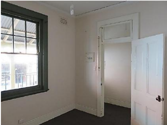
Figure 12.20 Front bedroom (space 1.2) with cement run skirting, timber cornice, ripple iron ceiling, decorative plaster wall vent, original four panel timber door with sunk moulds, original architraves and fanlight over, and original double hung window with original architrave and sill board—54C / 46–56 Gloucester Street. (Source: GML Heritage, July 2016)
