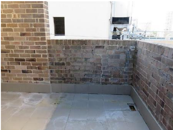
Figure 16.16 Roof terrace (space E.1) showing evidence of the original garbage chute (blocked up) and drain—56C / 46–56 Gloucester Street. (Source: GML Heritage, July 2016)
