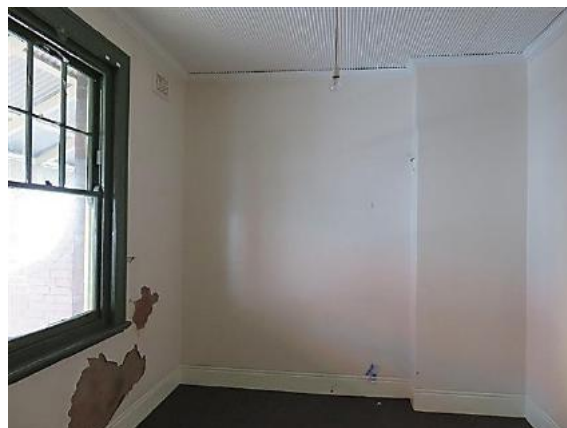
Figure 10.21 Front bedroom (space 1.2) showing timber double hung sash window, cement run skirting, ripple iron ceiling and moulded timber cornice—54A / 46–56 Gloucester Street. (Source: GML Heritage, July 2016)
