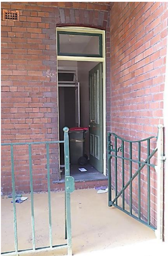
Figure 13.8 Entry to Flat 56 (space E.1) with four-panel timber front door with bolection moulds to bottom timber panels and wired glass to upper panels, and fanlight above. The opening has dark brick surround and arched brick head. A wrought iron fence and gate enclose the front yard located on the verandah—56 / 46–56 Gloucester Street. (Source: GML Heritage, July 2016)
