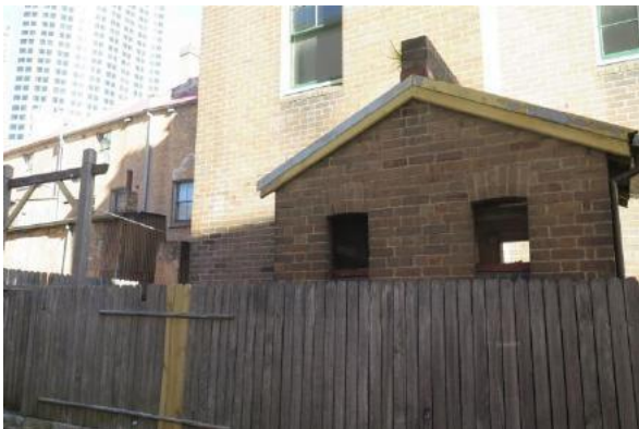
Figure 15.48 Eastern aspect of 56B Gloucester Street, as viewed from Cambridge Street, showing external WC and missing glass in louvres—56B / 46–56 Gloucester Street. (Source: GML Heritage, July 2016)
