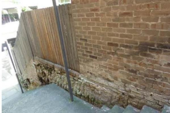
Figure 1.59 Northern boundary of flat 46, showing the sandstone retaining wall stepped up the slope, timber fence and common brick wall to the lower ground of the flat—46/46–56 Gloucester Street. (Source: GML Heritage, July 2016)
