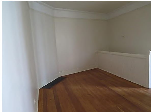
Figure 7.13 Living area (space G.3) showing fireplace blocked up in corner, but retains its concrete hearth. The space has timber floor, cement rendered skirting, timber picture rail, fibrous plaster cornice and plasterboard ceiling. The stair against the eastern wall has a timber boarded balustrade and newel post—52 / 46–56 Gloucester Street. (Source: GML Heritage, July 2016)
