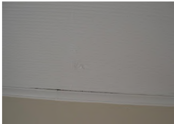
Figure 6.31 Ripple iron ceiling in the rear bedroom—50A / 48–56 Gloucester Street, with moulded timber cornice and remnant gas-light services (space 1.6). (Source: GML Heritage, July 2016)
