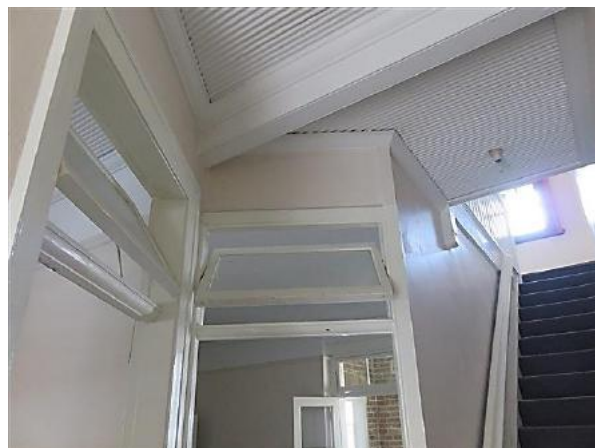
Figure 8.19 Entrance hall (space 1.1) showing the original timber door frames with fanlights above, timber cornices, timber transverse beam and ripple iron ceiling—52A / 46–56 Gloucester Street. (Source: GML Heritage, July 2016)
