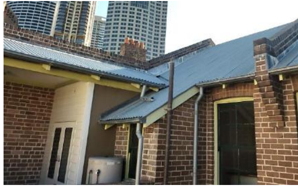
Figure 6.11 Rear elevation —50A / 48–56 Gloucester Street showing corrugated metal roof, party walls and chimneys. (Source: GML Heritage, July 2016)
