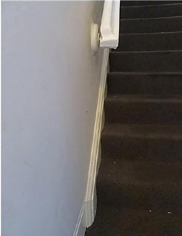
Figure 16.38 Staircase (space 1.7) showing closed moulded timber stringer and timber handrail supported on metal brackets mounted on timber roses fixed to wall—56C / 46–56 Gloucester Street. (Source: GML Heritage, July 2016)
