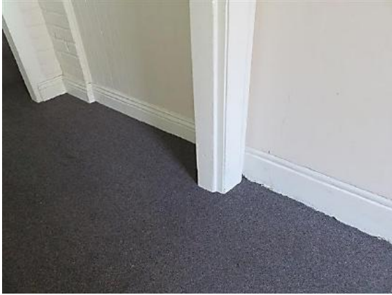
Figure 10.32 Detail of original skirting run in cement on the right and later timber skirting on the left (space 1.4)—54A / 46–56 Gloucester Street. (Source: GML Heritage, July 2016)
