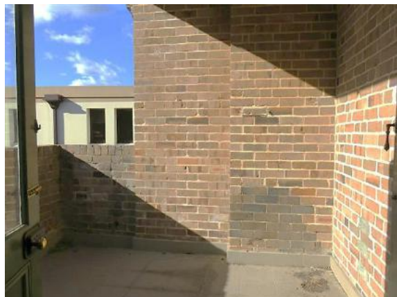
Figure 14.15 Roof terrace (space E.1) showing tiled floor and evidence of the original garbage chute (blocked up) and removal of former laundry copper (under roofed area)—56A / 46–56 Gloucester Street. (Source: GML Heritage, July 2016)
