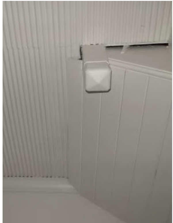
Figure 11.33 The laundry (space LG.3) showing original ripple iron ceiling, timber cornices, and timber pendant newel post—54B / 46–56 Gloucester Street. (Source: GML Heritage, May 2016)
