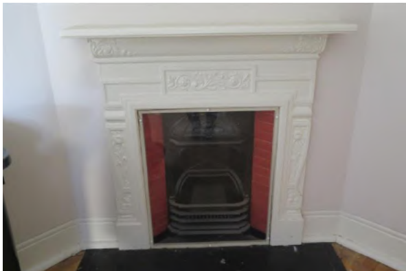
Figure 15.20 Original cast-iron chimney piece and grate in the front bedroom (space G.2). The skirting is run in the wall render—56B / 46–56 Gloucester Street. (Source: GML Heritage, July 2016)
