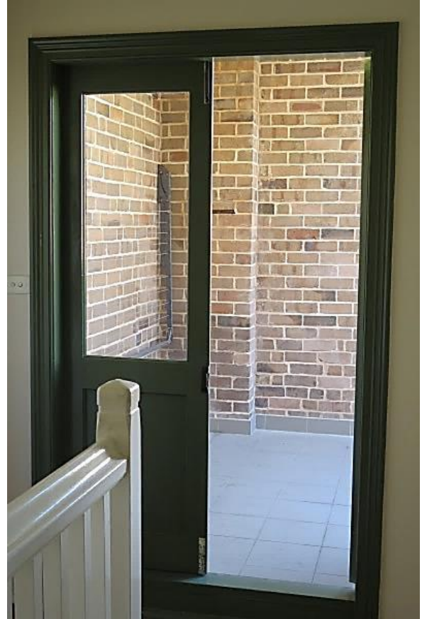
Figure 4.59 Modern French doors to terrace (space E.1) showing modern paving and original brick walls to the enclosed part of the roof terrace—48A / 46–56 Gloucester Street. (Source: GML Heritage, May 2016)
