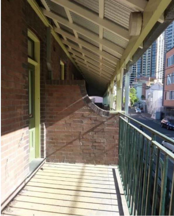
Figure 4.9 Brick dividing wall to upper level verandah (first floor level, Flat 52A). Note the painted concrete slab. (Source: GML 2015)
