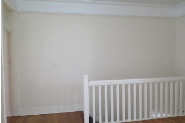
Figure 3.22 The living room (space G.3), showing original cement run skirtings, timber balustrade, newel post and picture rail—48 / 46–56 Gloucester Street. (Source: GML Heritage, May 2016)
