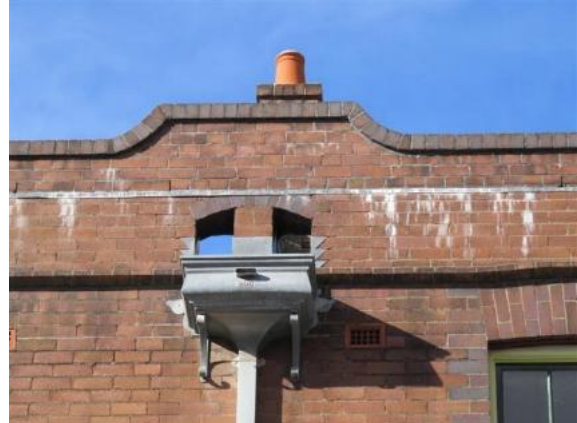
Figure 10.11 Cast rainwater head on front elevation and chimney with terracotta chimney pot over party wall—54A / 46–56 Gloucester Street. (Source: GML Heritage, 2016)
