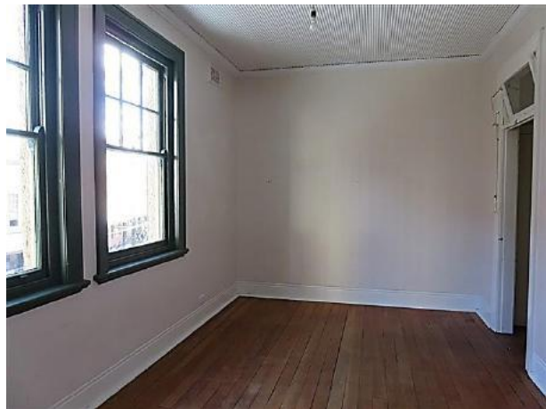
Figure 16.49 Front room on the second floor (space 2.4) showing the original double hung sash windows, cement rendered skirting, ripple iron ceiling and timber cornice—56C / 46–56 Gloucester Street. (Source: GML Heritage, July 2016)
