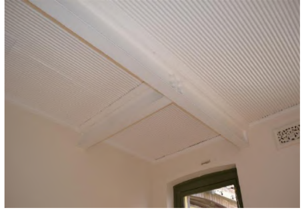
Figure 1.39 Ceiling of the dining room (space LG.1) showing the ripple iron and steel support beams—46/46–56 Gloucester Street. (Source: GML Heritage, July 2016)
