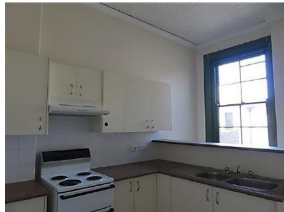
Figure 14.44 Kitchen (space 2.3) showing the original ripple iron ceiling, moulded timber cornice and original double hung window joinery. The fitout is modern—56A / 46–56 Gloucester Street. (Source: GML Heritage, July 2016)
