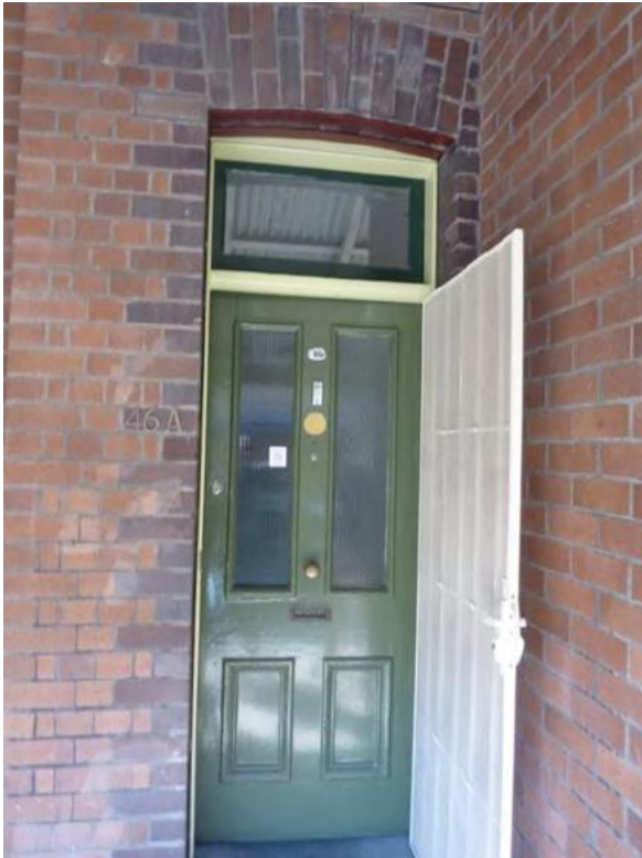
Figure 2.10 Fanlight over the front door showing the contrasting brick surrounds and segmental arch (supported on a metal arch bar) to the opening; also the modern fly screen—46A / 46–56 Gloucester Street. (Source: GML Heritage, November 2015)
