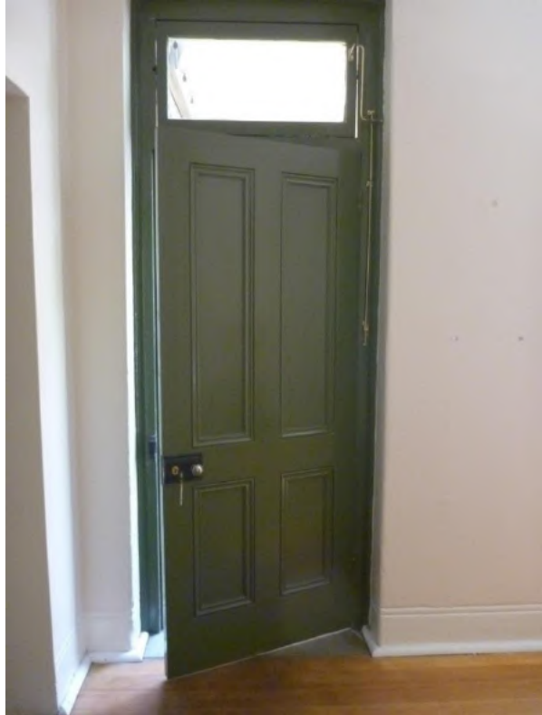
Figure 4.26 Exterior four panel rear main door with external bolection moulding, internal flush moulds and central pivot fanlight in flat 46. (Source: GML Heritage, May 2016)
