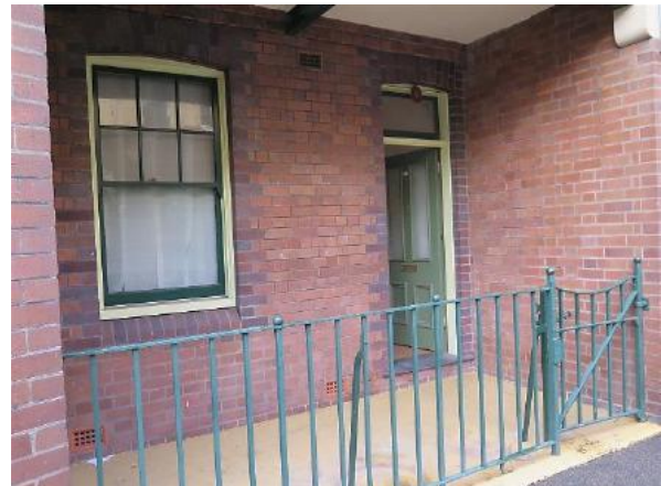
Figure 7.7 Front porch (space E.1) showing external brick walls, timber entry door with fanlight, wrought iron fence and gate, double-hung window with chamfered brick sill—52 / 46–56 Gloucester Street (Source: GML Heritage, July 2016)
