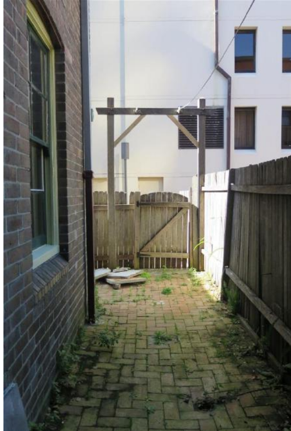
Figure 15.47 Rear yard with brick paving (space E.2), timber fencing, downpipe, external double hung sash window and reconstructed laundry hoist—56B / 46–56 Gloucester Street. (Source: GML Heritage, July 2016)
