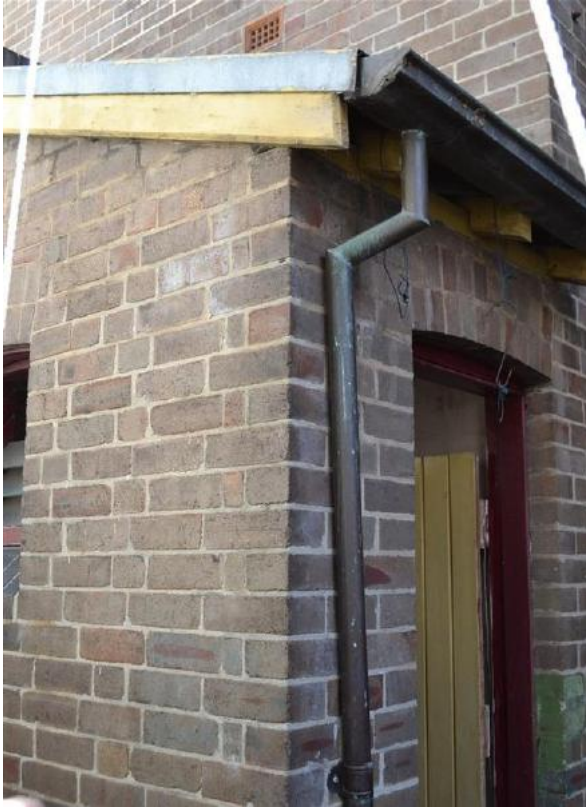
Figure 5.42 Former external WC (space E.3) showing, exposed rafter eaves, brick walls, brick arched doorway and timber boarded door—50 / 46–56 Gloucester Street. (Source: GML Heritage, June 2016)
