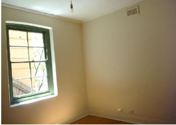
Figure 1.38 Dining room (space LG.1) showing the timber double-hung sash window—46/46–56 Gloucester Street. (Source: GML Heritage, July 2016)
