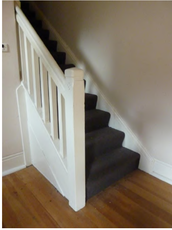
Figure 4.44 The original stair at the lower ground floor level with closed string, simple square balusters and newel posts, moulded handrail and vertical boarding below (Flat 56B). (Source: GML 2015)
