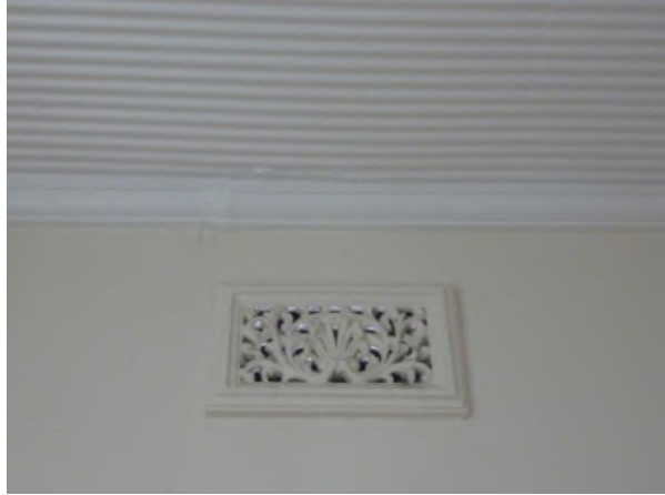
Figure 4.58 Typical decorative plaster scroll pattern vent (Flat 50). (Source: GML 2015)
