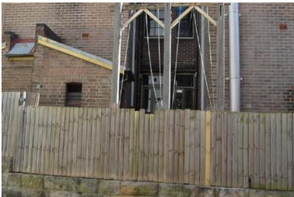
Figure 5.44 Exterior walls in common brick, timber fence and squared rock faced perimeter retaining wall. Rear wing looking west—50 / 46–56 Gloucester Street (Source: GML Heritage, June)
