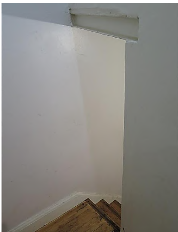
Figure 7.24 Repaired original stairs, original cement rendered and plastered brick walls, and original steel beam over the stair—52 / 46–56 Gloucester Street. (Source: GML Heritage, June 2016)
