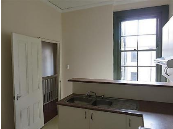
Figure 12.42 Kitchen (space 2.3) showing the original timber double hung window and relocated door—54C / 46–56 Gloucester Street. (Source: GML Heritage, July 2016)
