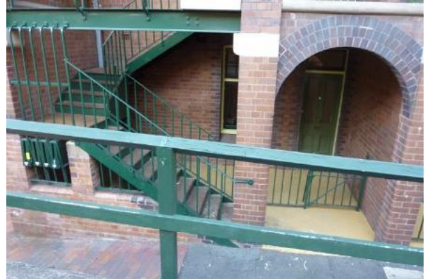
Figure 1.7 Front verandah looking down from Gloucester Street—46/46–56 Gloucester Street, showing the eastern stair access (common property) to the upper floor verandah and contrasting brick arch and sandstone bolster supporting the steelwork—46/46–56 Gloucester Street. (Source: GML Heritage, November 2015)
