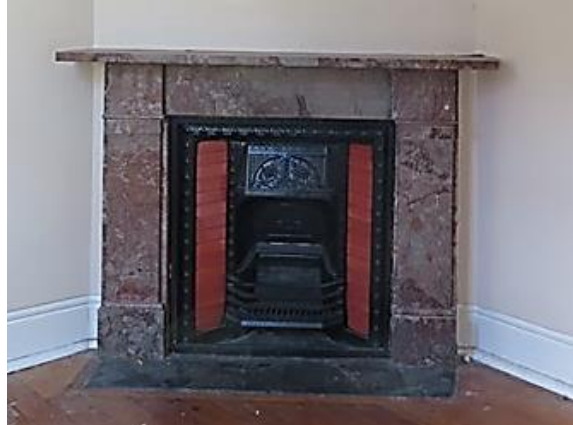
Figure 14.48 Fireplace in the front room on second floor (space 2.4) with early cast iron grate with tiled sides, and red marble chimney piece—56A / 46–56 Gloucester Street. (Source: GML Heritage, July 2016)
