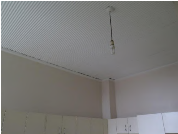
Figure 11.32 Original ripple iron ceiling in kitchen and modern light fixture (space LG.2)—54B / 46–56 Gloucester Street. (Source: GML Heritage, July 2016)
