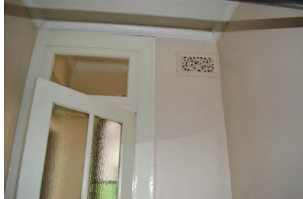
Figure 5.27 Bathroom (space G.5) showing the fanlight above the door, decorative plaster wall vent and plasterboard ceiling—50 / 46–56 Gloucester Street. (Source: GML Heritage, June 2016)
