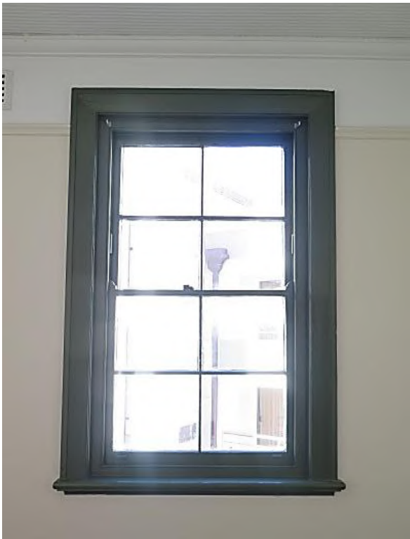
Figure 4.40 Timber double-hung sash window, sillboard, architrave and sash frame in the rear bedroom (space 1.6)—48A / 46–56 Gloucester Street. (Source: GML Heritage, May 2016)
