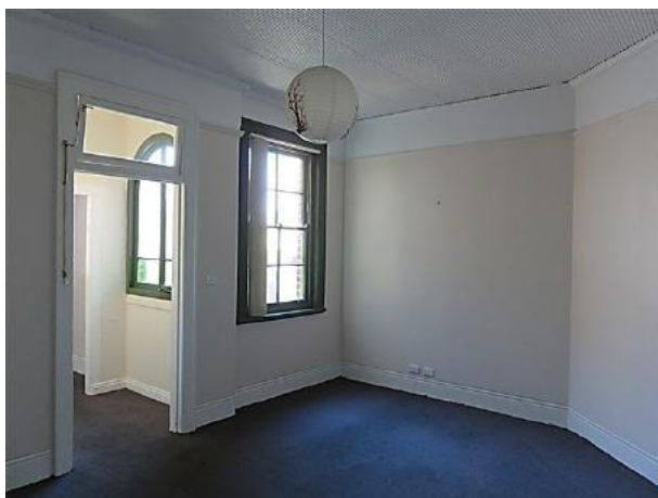
Figure 16.26 Living room (space 1.3) showing the ripple iron ceiling, moulded timber picture rail and cornice, and original double-hung sash window with original architrave, sill board and moulding. The fireplace has been removed, hearth remains under the carpet—56C / 46–56 Gloucester Street. (Source: GML Heritage, July 2016)
