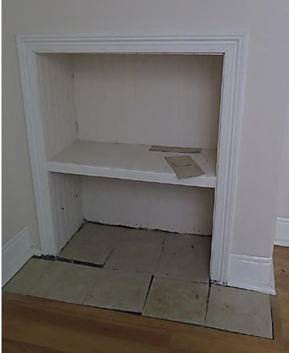
Figure 13.28 Fireplace in the dining room (space LG.1) with 1980s boarding, shelf and architrave—56 / 46–56 Gloucester Street. (Source: GML Heritage, June 2016)
