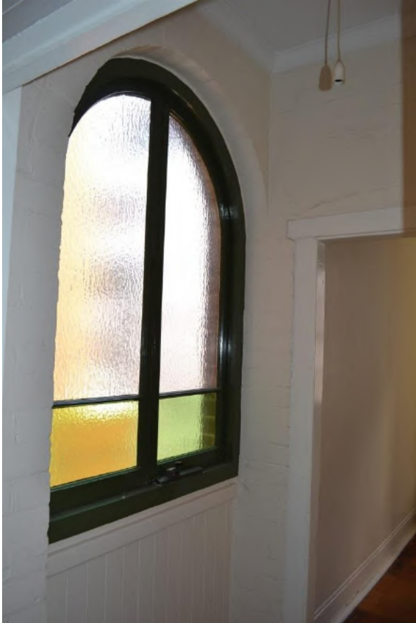
Figure 1.26 Infilled former rear porch opening (space G.4). The original arched opening has been infilled with vertical boarding and casement windows—46/46–56 Gloucester Street. (Source: GML Heritage, July 2016)
