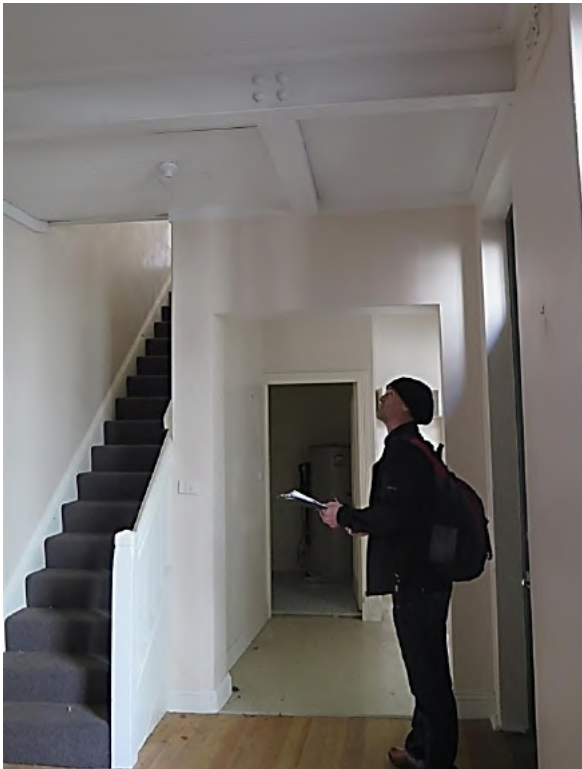
Figure 13.26 Stair descends into dining area (space LG.1). Original steel beams support the walls above. The ceiling is ripple iron—56 / 46—56 Gloucester Street (Source: GML Heritage, July 2016).
