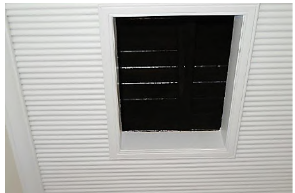
Figure 4.45 Stair hall (space 2.1) showing original ripple iron ceiling, open access to roof space and original roof hatch surround—48A / 46–56 Gloucester Street. (Source: GML Heritage, May 2016)
