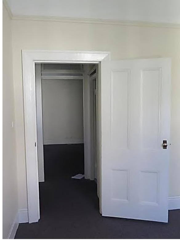
Figure 4.39 Original four-panel sunk moulded timber door in the rear bedroom (space 1.6), original architrave and moulded timber picture rail—48A / 46–56 Gloucester Street. (Source: GML Heritage, May 2016)
