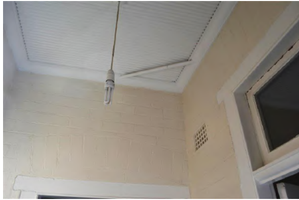
Figure 2.30 Original ripple iron ceiling and original door frames with brick arched heads above (space 1.4)—46A/46–56 Gloucester Street. (Source: GML: Heritage, July 2016)
