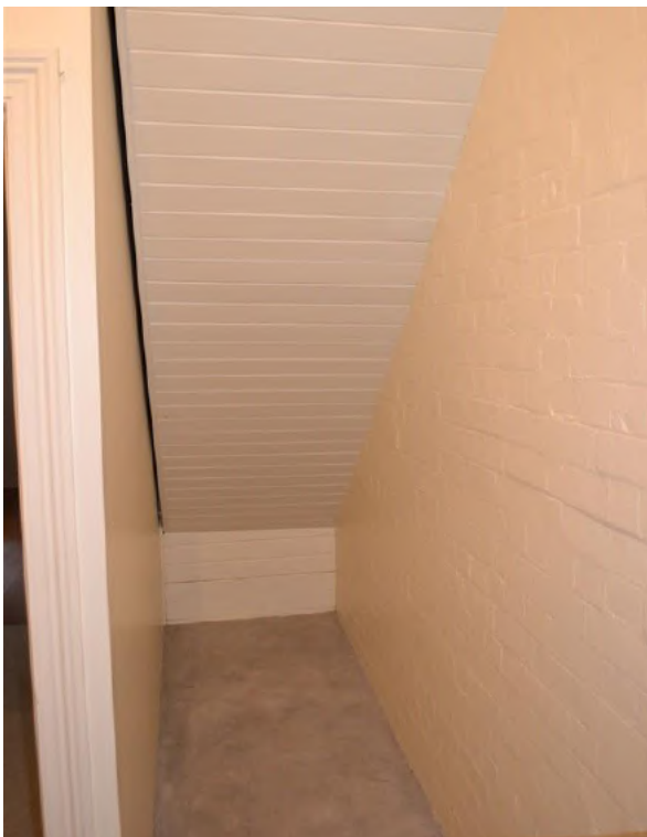
Figure 5.40 Laundry (space LG.3) showing the T&G soffit to the stair and original painted brick walls—50 / 46–56 Gloucester Street. (Source: GML Heritage, June 2016)
