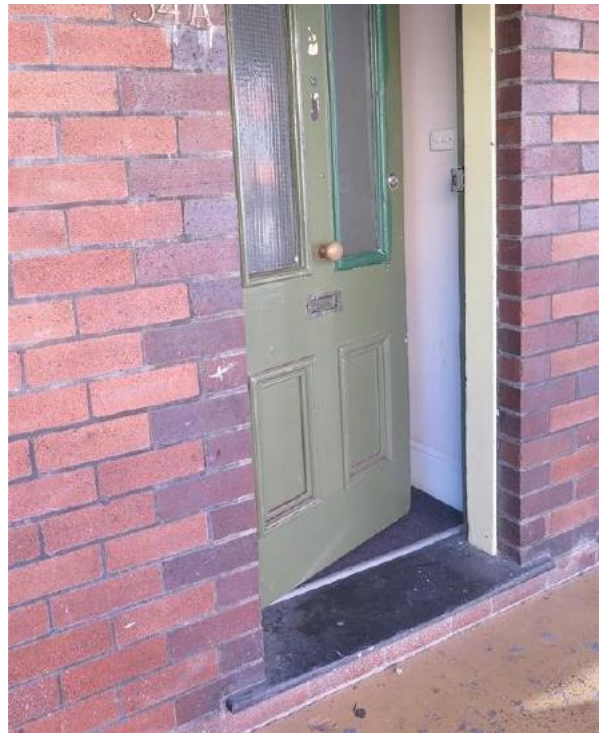
Figure 4.8 Four-panelled doors with bolelection moulding (first floor level, Flat 54A). Note slate threshold to front doors. (Source: GML 2016)
