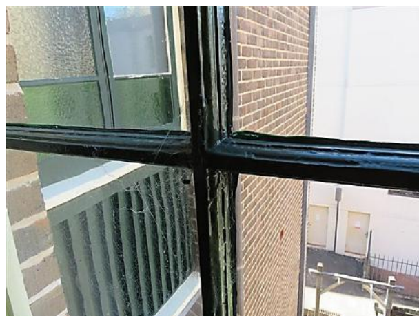
Figure 16.27 Glazing bar detail of window in living room (space 1.3). The balustrade element below the window infill to the arched opening of the former rear porch is visible through the window—56C / 46–56 Gloucester Street. (Source: GML Heritage, July 2016)
