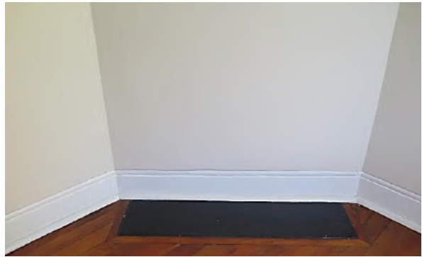
Figure 4.57 Original corner fireplace (blocked off and rendered and skirted over to match adjacent) with concrete hearth (space 2.4)—48A / 46–56 Gloucester Street. (Source: GML Heritage, May 2016)
