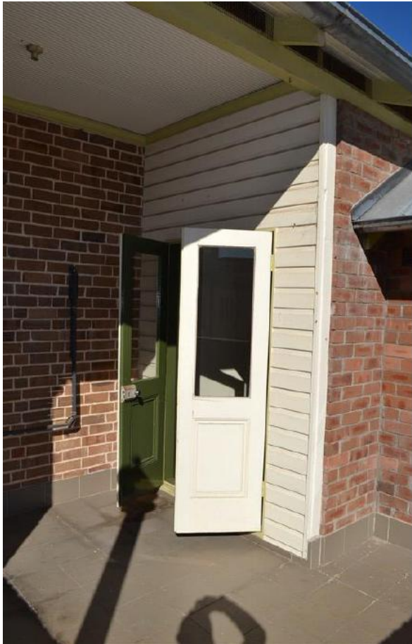
Figure 2.14 Roof terrace (space E.1) showing the modern half-glazed timber doors and recent weatherboard wall—46A/46–56 Gloucester Street. (Source: GML Heritage, July 2016)
