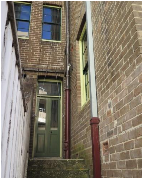
Figure 3.52 Exterior, rear wing showing common brickwork, concrete steps, original cast iron and modern steel/copper downpipes/service pipes, and terracotta wall vents (space E.2)—48 / 46–56 Gloucester Street. (Source: GML Heritage, May 2016)
