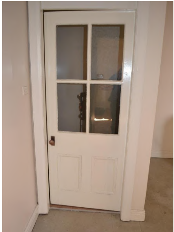
Figure 1.45 half-glazed timber door to laundry (space LG.3)—46/46–56 Gloucester Street. (Source: GML Heritage, July 2016)
