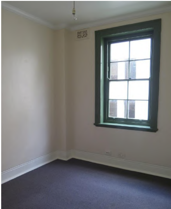
Figure 11.24 Rear bedroom (space G.6) showing modern carpeted floor (over original timber), original cement rendered skirtings, cornice, decorated wall vent and timber double-hung sash window—54B / 46–56 Gloucester Street. (Source: GML Heritage, July 2016)
