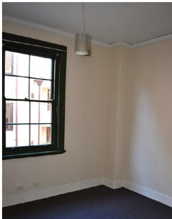
Figure 2.34 Rear bedroom (space 1.6) showing the original double hung window with original architrave, sill board and moulding, moulded timber picture. Chimney flue from flat below in corner of space—46A / 46–56 Gloucester Street. (Source: GML Heritage, July 2016)
