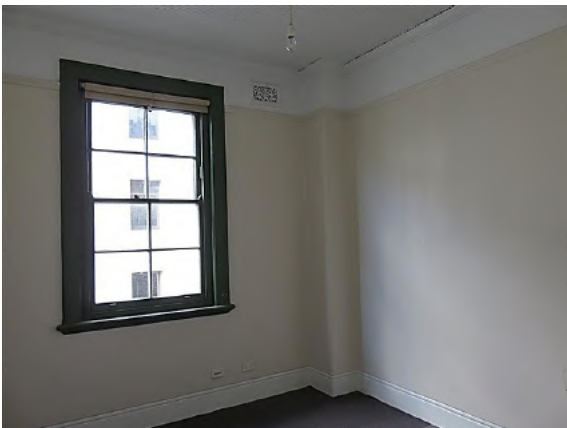
Figure 14.31 Rear bedroom (space 1.6) showing the original double hung window with original architrave, sill board and moulding, moulded timber picture rail and decorative plaster wall vent. Chimney flue from flat below in corner of space—56A / 46–56 Gloucester Street. (Source: GML Heritage, July 2016)
