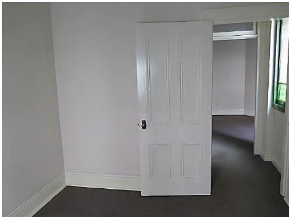
Figure 9.20 Rear bedroom (space G.6) showing cement rendered skirting and original four-panel sunk moulded timber door and architraves—54 / 46–56 Gloucester Street. (Source: GML Heritage, July 2016)
