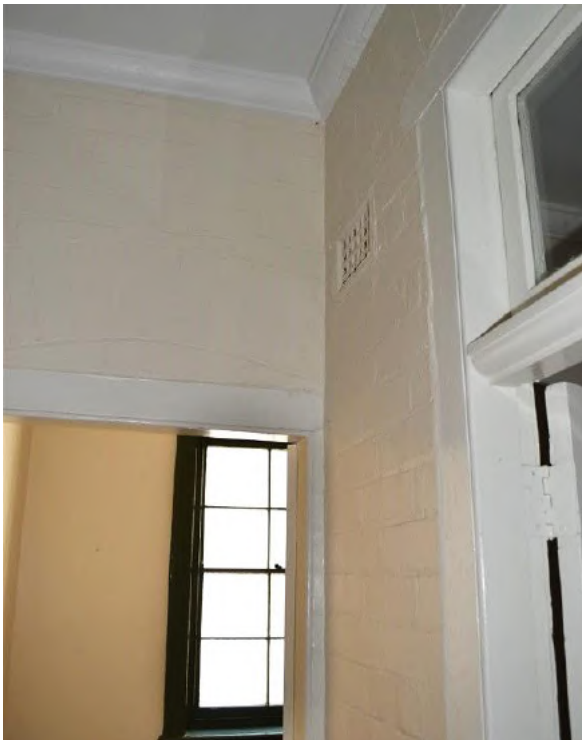
Figure 5.24 Infilled former porch (space G.4), showing the brick head above doorway to the bedroom (space G.6) and the fanlight to the bathroom (space G.5)—50 / 46-56 Gloucester Street (Source: GML Heritage, June 2016).
