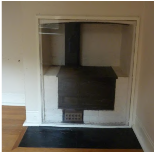
Figure 4.52 The cast-iron cooking range in the fireplace at the lower ground floor level (former kitchen, Flat 56B). Note the range is covered by a perspex screen. (Source: GML 2015)
