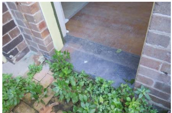
Figure 15.45 Painted concrete threshold to rear door—56B / 46–56 Gloucester Street. (Source: GML Heritage, July 2016)
