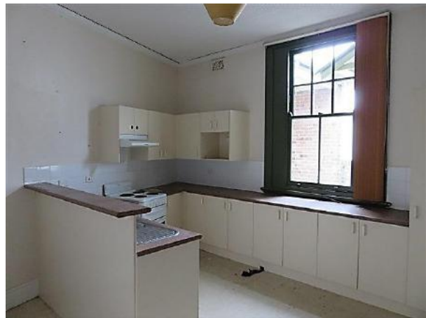
Figure 8.45 Kitchen (space 2.3) showing modern fitout and ripple iron ceiling with moulded timber cornice. Window matches others in the block but may have been relocated—52A / 46–56 Gloucester Street. (Source: GML Heritage, July 2016)
