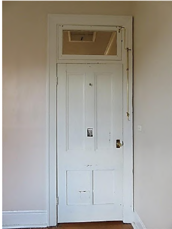
Figure 14.46 Four panel door and fanlight to space 2.4, showing bottom panels replaced and original architrave. Original cement run skirting with timber quad mould—56A / 46–56 Gloucester Street. (Source: GML Heritage, July 2016)
