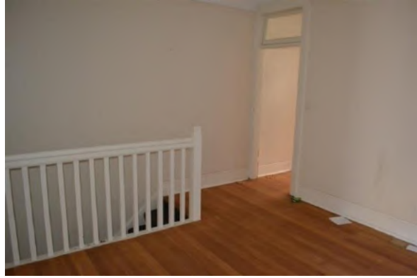
Figure 5.19 The living room (space G.3), showing cement run skirtings, timber balustrade and original timber door frame with fanlight to the entry hall (space G.1)—50 / 46–56 Gloucester Street. (Source: GML Heritage, June 2016)
