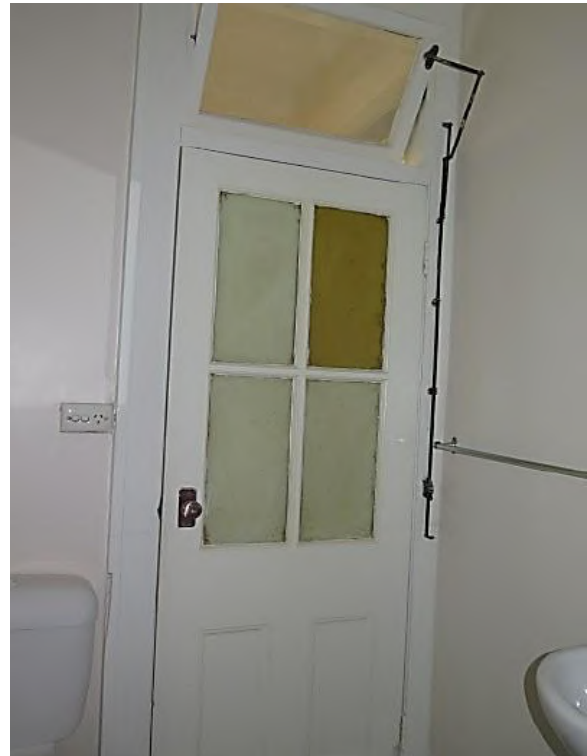
Figure 4.37 Bathroom (space 1.5) showing modern fit-out and original part glazed panel door with fanlight above and original (?) mechanism—48A / 46–56 Gloucester Street. (Source: GML Heritage, May 2016)
