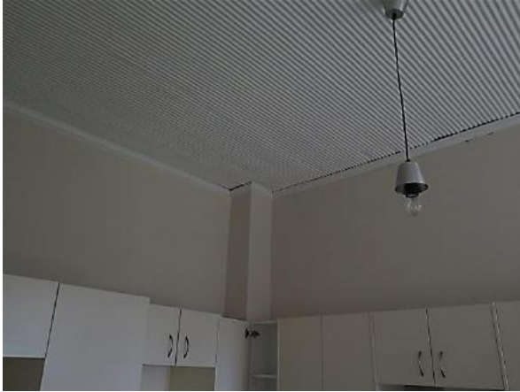
Figure 9.30 Original ripple iron ceiling in kitchen and modern light fixture (space LG.2)—54 / 46–56 Gloucester Street. (Source: GML Heritage, July 2016)
