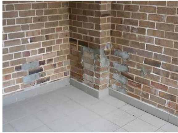
Figure 12.15 Roof terrace (space E.1) showing evidence of removal of the former laundry copper—54C / 46–56 Gloucester Street. (Source: GML Heritage, July 2016)
