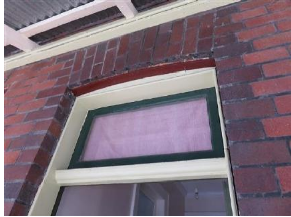
Figure 14.7 Fanlight over the front door showing the contrasting brick surround and segmental arch (supported on a metal arch bar) to the opening—56A / 46–56 Gloucester Street. (Source: GML Heritage, July 2016)
