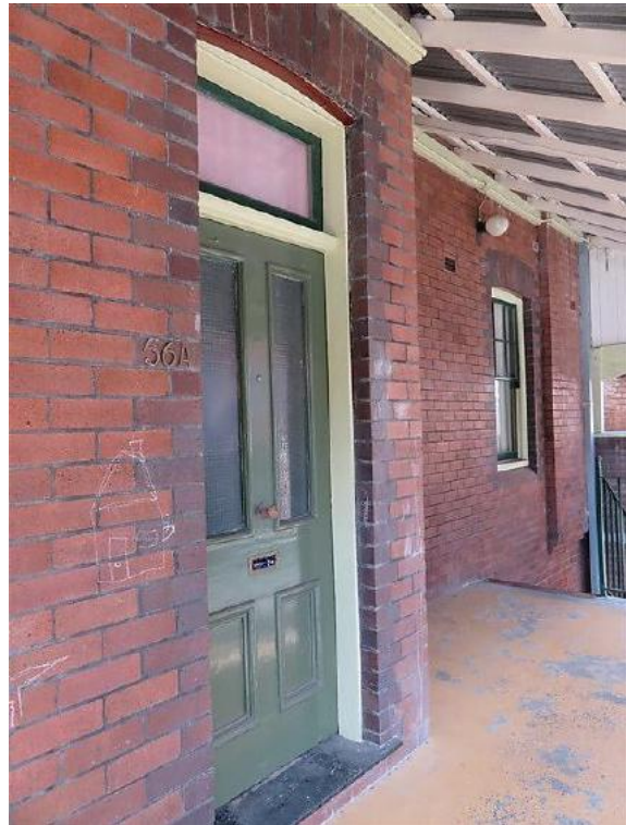
Figure 14.9 Four-panel entrance door with bolection moulds, wired glass to upper panels, slate threshold and fanlight over—56A / 46–56 Gloucester Street. (source: GML Heritage, July 2016)
