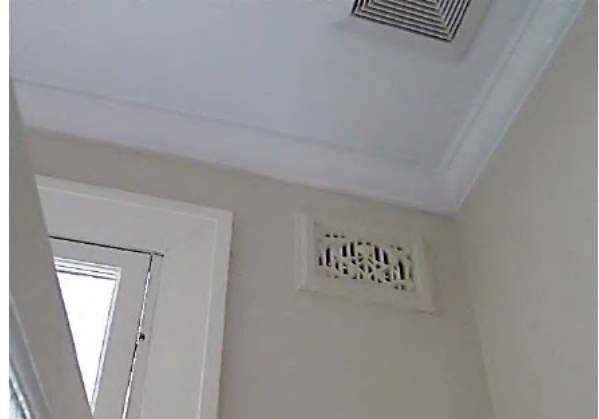
Figure 9.19 Bathroom (space 1.5) showing the plaster ceiling, timber cornice and decorative plaster wall vent—54 / 46–56 Gloucester Street. (Source: GML Heritage, July 2016)
