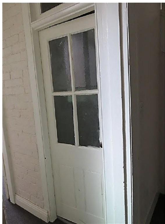
Figure 10.31 Original half glazed door to bathroom (space 1.5) showing obscured glass and bead flush panels. The transom detail over the door is original. The timber skirting is late twentieth century—54A / 46–56 Gloucester Street. (Source: GML Heritage, July 2016)
