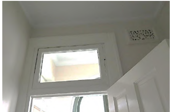
Figure 13.23 Fanlight over door and decorative plaster wall vent in the bathroom (space G.5). The panel door to the bathroom (space G.5) is a modern reproduction—56 / 46–56 Gloucester Street. (Source: GML Heritage, July 2016)
