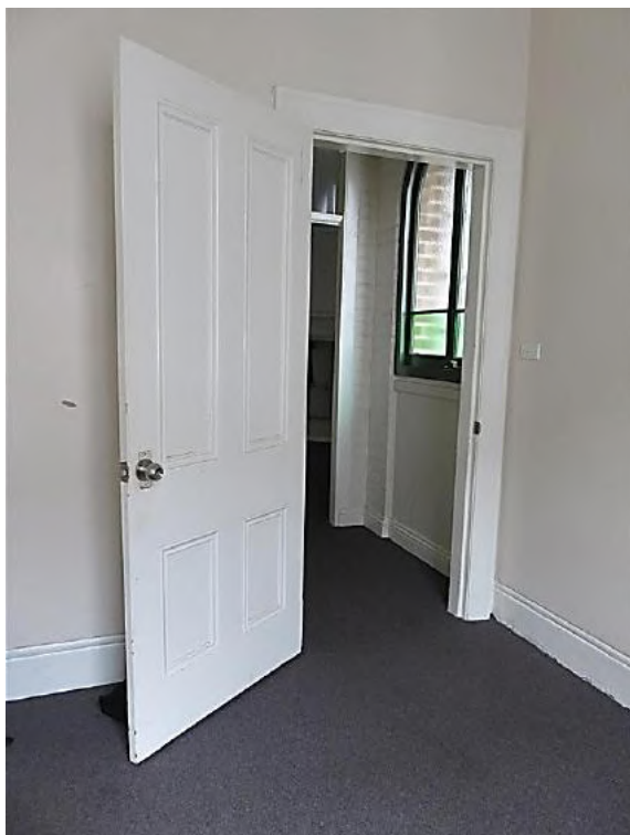
Figure 10.36 Rear bedroom (space 1.6) showing original doorframe and cement rendered skirtings—54A / 46–56 Gloucester Street. (Source: GML Heritage, July 2016)
