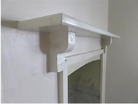
Figure 10.24 Detail of fireplace recess (cast iron range has been removed)—54A / 46–56 Gloucester Street. (Source: GML Heritage, July 2016)
