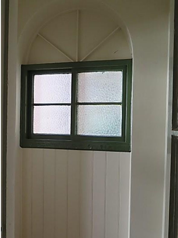
Figure 3.26 Infilled former rear porch opening (space G.4), with horizontal sliding sash window and modern T&G boarding below—48 / 46–56 Gloucester Street. (Source: GML Heritage, May 2016)
