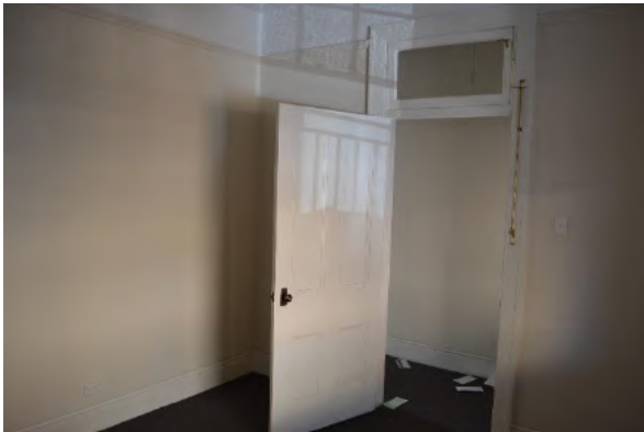
Figure 6.20 Front bedroom (space 1.2)—50A / 48–56 Gloucester Street, with cement rendered skirting, picture rail and original four-panel timber door with sunk moulds, original architrave and fanlight over. (Source: GML Heritage, July 2016)
