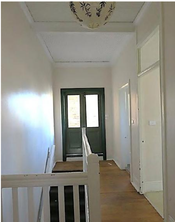
Figure 16.40 Upper stair hall (space 2.1) showing ceiling beam over space, ripple iron ceiling and timber cornice, half glazed timber doors to roof terrace (recent), and original timber frame to kitchen door on right—56C / 46–56 Gloucester Street. (Source: GML Heritage, July 2016)
