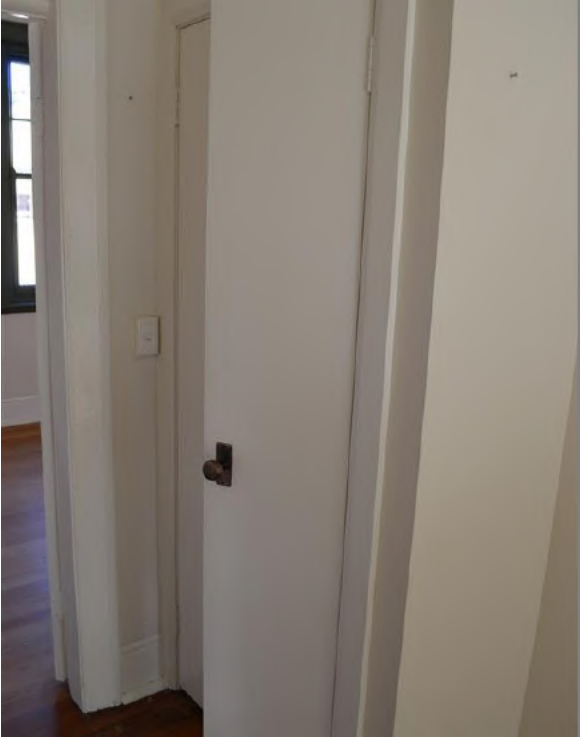
Figure 2.41 Modern cupboard built into the second floor landing (space 2.1) with paneled timber doors—46A/46–56 Gloucester Street. (Source: GML Heritage, July 2016)
