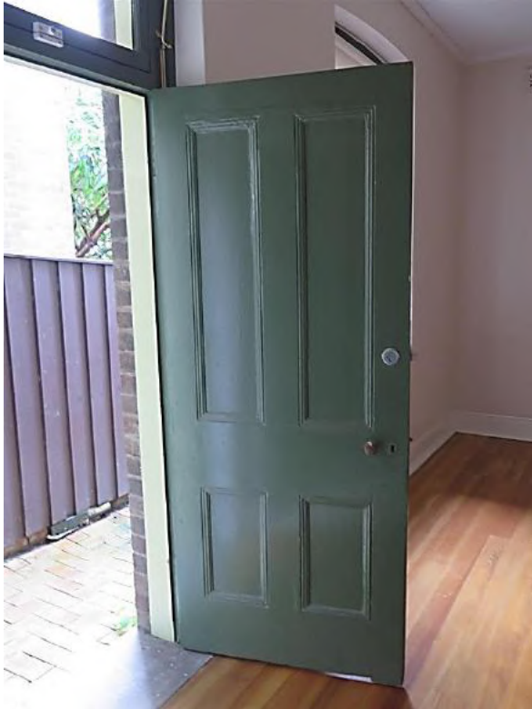
Figure 9.26 Four panel sunk-moulded external door on lower ground-floor level (space LG.1)—54 / 46–56 Gloucester Street. (Source: GML Heritage, July 2016)
