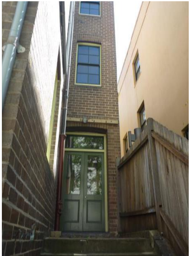
Figure 4.12 The rear elevation of Flat 46, showing French doors added to earlier opening in the 1988 restoration, and original four-paned double-hung sash windows. (Source: GML, 2015)
