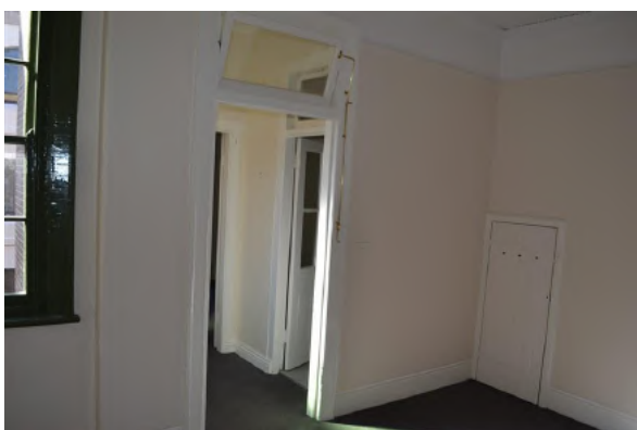
Figure 2.27 Living room (space 1.3) showing original doorframe and fanlight leading to spaces 1.4-1.6, cement run skirting and the cupboard under the stairs—46A/46–56 Gloucester Street. (Source: GML Heritage, July 2016)
