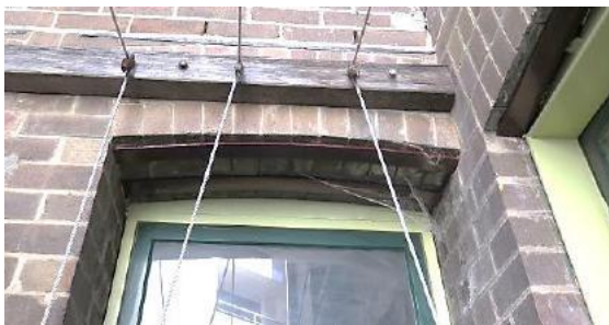
Figure 3.56 Brick arch and iron lintel bar over the rear door fanlight showing laundry hoist fixings above—48 / 46–56 Gloucester Street. (Source: GML Heritage, May 2016)
