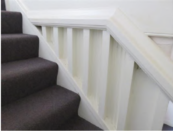
Figure 12.34 Detail of stair balustrade showing ripple iron cladding to outer face enclosing bathroom (space 1.5)—54C / 46–56 Gloucester Street. (Source: GML Heritage, July 2016)
