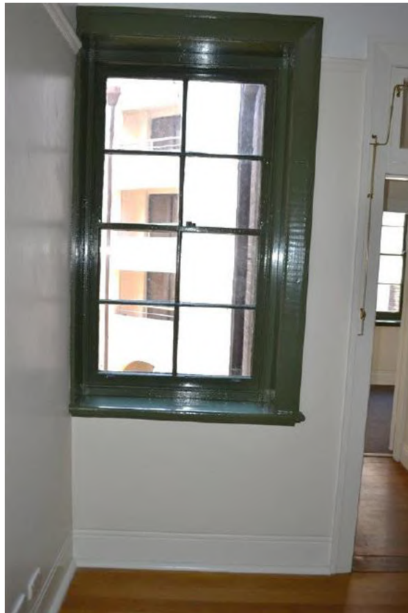
Figure 5.21 Timber double-hung sash window in the living room (space G.3)—50 / 46–56 Gloucester Street. (Source: GML Heritage, June 2016)
