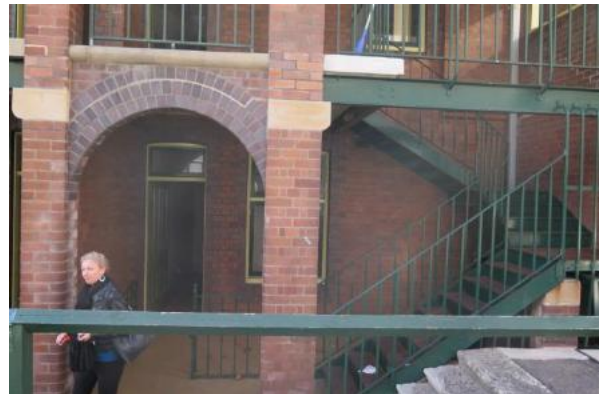
Figure 15.13 Detail of exterior staircase to first floor at the southern end of the building. Sandstone bolsters supporting the steelwork—56B / 46–56 Gloucester Street. (Source: GML Heritage, July 2016)
