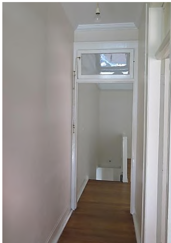
Figure 3.15 The entry (space G.1) showing timber floor, cement run skirtings, timber cornice and timber door frame with fanlight to the living room (space G.3)—48 / 46–56 Gloucester Street. (Source: GML Heritage, May 2016)
