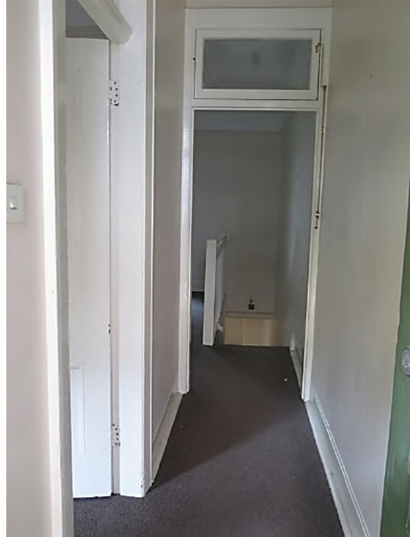
Figure 9.11 The entry (space G.1) showing modern carpeting over timber floors, cement run skirtings, and timber door frame with fanlight to the living room (space G.3)—54 / 46–56 Gloucester Street. (Source: GML Heritage, July 2016)
