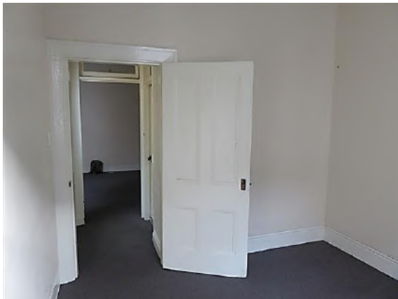
Figure 12.32 Rear bedroom (space 1.6) showing the original four panel timber door with its original architraves, and cement rendered skirtings—54C / 46–56 Gloucester Street. (Source: GML Heritage, July 2016)
