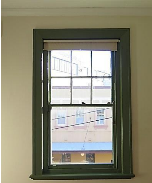
Figure 4.58 Original timber double-hung sash window in dining room (space 2.4)—48A / 46–56 Gloucester Street. (Source: GML Heritage, May 2016)
