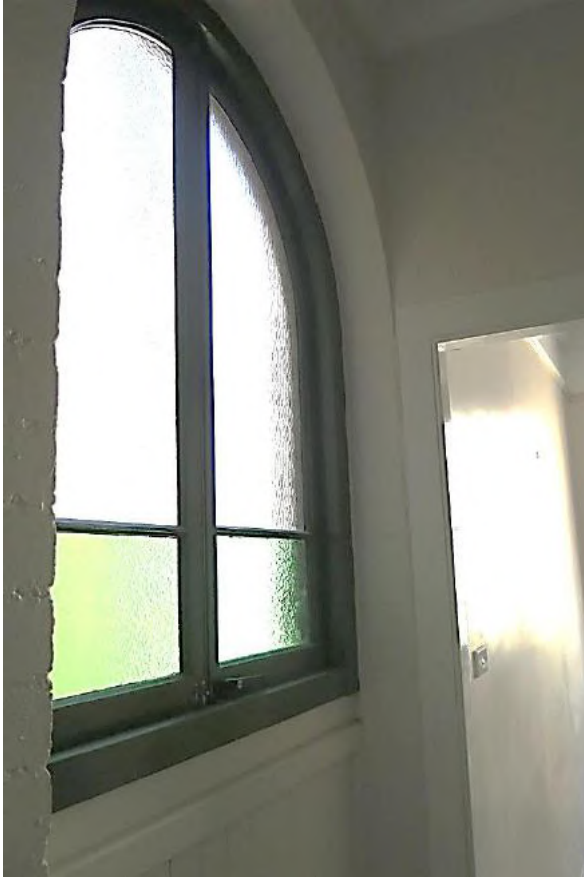
Figure 13.20 Infill to arched opening of former rear porch (space G.4) consisting of casement windows with textured and coloured glass, and modern T&G boarding below—56 / 46–56 Gloucester Street. (Source: GML Heritage, July 2016)
