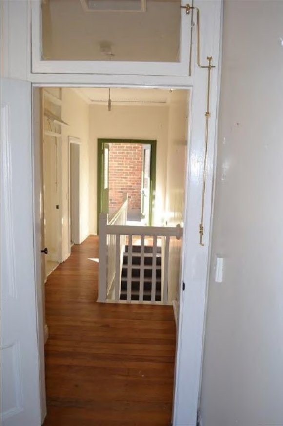
Figure 2.49 Original (?) doorway to the dining room (space 2.4) with fanlight and opening mechanism above—46A / 46–56 Gloucester Street. (Source: GML Heritage, July 2016)
