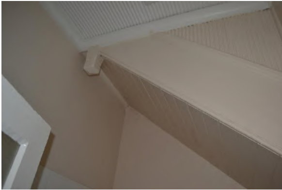
Figure 6.28 Bathroom (space 1.5)—50A / 48–56 Gloucester Street showing modern fit out, v-jointed timber stair soffit with ripple iron to ceiling and side of stair above the string. (Source: GML Heritage, July 2016)
