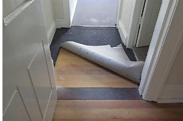
Figure 13.21 Original timber threshold to doorway from living room (space G.3) to rear porch (space G.4). The half glazed door between space G.3 and G.4 is a modern reproduction. The timber floor of the porch has been raised—56 / 46–56 Gloucester Street (Source: GML Heritage, July 2016)
