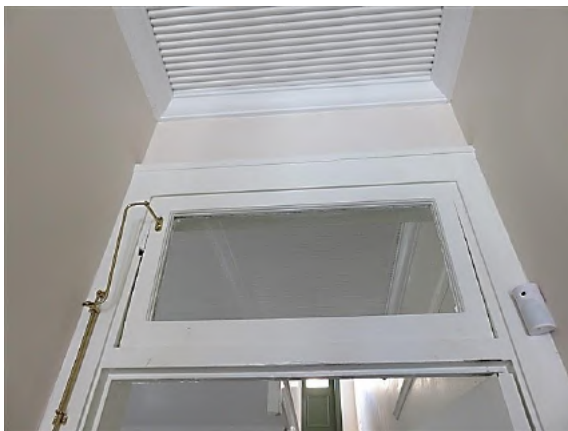
Figure 14.18 Typical detail of original internal fanlight, ripple iron ceiling and moulded timber cornice—door between spaces 1.1 and 1.3—56A / 46–56 Gloucester Street. (Source: GML Heritage, July 2016)
