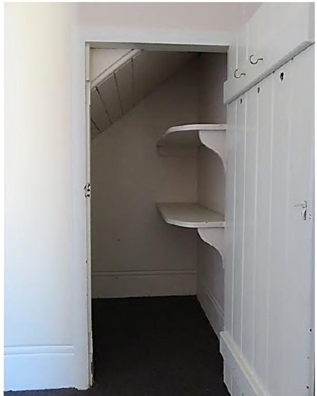
Figure 16.25 Cupboard under the stairs in the living room (space 1.3) with timber shelves, showing the v-jointed timber board soffit to the stair and ledged and sheeted door to the cupboard with air holes drilled in it—56C / 46–56 Gloucester Street. (Source: GML Heritage, July 2016)
