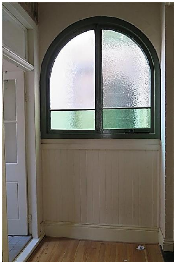
Figure 7.15 The arched opening of the former porch (space G.4) is infilled with a pair of casement windows and vertical timber boarding. (Source: GML Heritage, July 2016)
