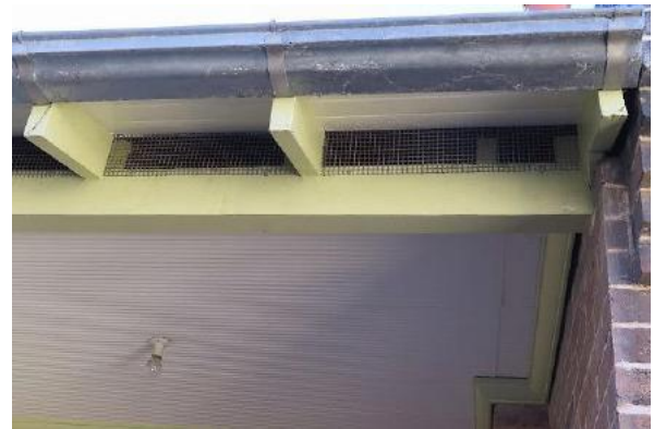
Figure 4.13 Exposed rafter of eaves to the rear wing at roof terrace level showing modern galvanised gutters and original ripple iron ceiling and rafters with timber cornice under roof (space E.2). 48A / 46–56 Gloucester Street. (Source: GML Heritage, May 2016)
