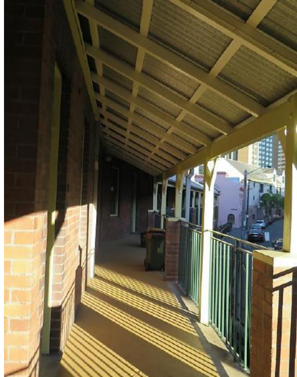
Figure 4.7 Underside of the verandah roof (common property), with original wrought iron balustrade, timber structure, brick pier and concrete verandah floor slab—48A / 46–56 Gloucester Street. (Source: GML Heritage, May 2016)
