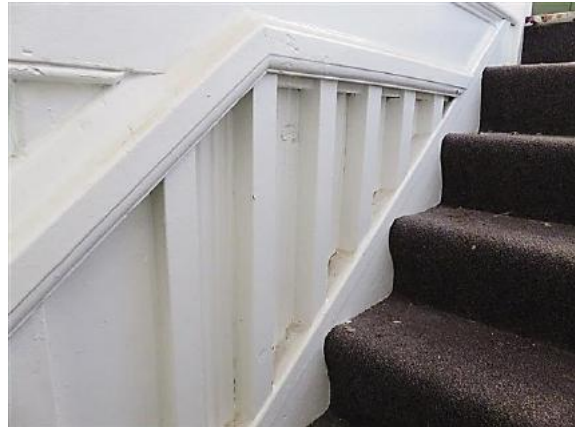
Figure 14.34 Ripple iron cladding to outer face of balustrade enclosing bathroom (space 1.5)—56A / 46–56 Gloucester Street. (Source: GML Heritage, July 2016)
