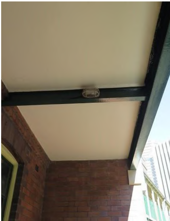
Figure 3.8 The ceiling of the front yard, showing steel structural I-beam, trimmer and concrete verandah floor slab—48 / 46–56 Gloucester Street. (Source: GML Heritage, May 2016)
