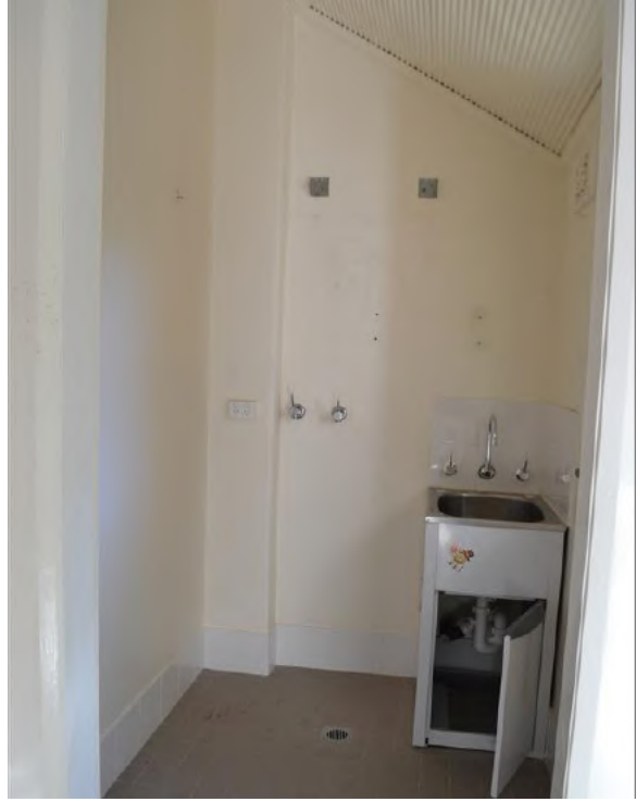
Figure 2.42 Laundry (space 2.2) showing original raked ripple iron ceiling—46A/46–56 Gloucester Street. (Source: GML Heritage, July 2016)
