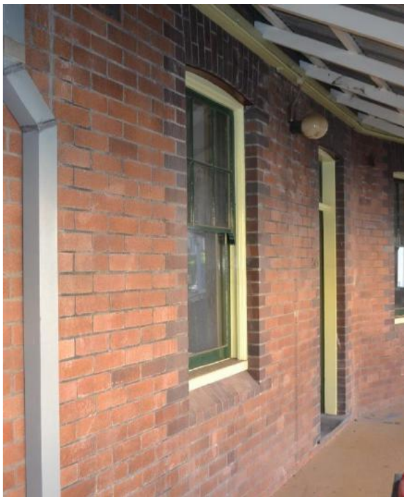
Figure 6.8 Front façade of flat 50A showing face brick external wall with contrasting brick surround to window and door openings and chamfered brick window sill—50A / 48–56 Gloucester Street. (Source: GML Heritage, July 2016)
