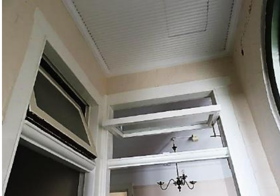
Figure 14.27 Original ripple iron ceiling and original door frames with brick arched heads above the fanlights (space 1.4)—56A / 46–56 Gloucester Street. (Source: GML: Heritage, July 2016)
