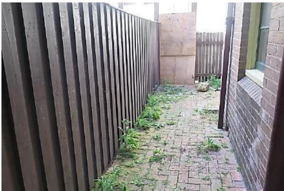
Figure 13.38 Brick paved rear yard and modern timber lapped and capped fencing (space E.2) —56 / 46–56 Gloucester Street. (Source: GML Heritage, June 2016)
