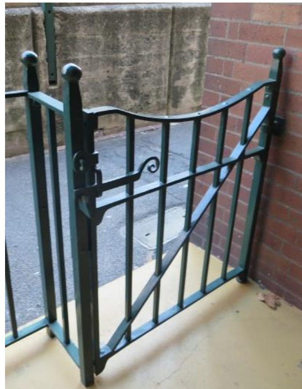
Figure 3.9 The original wrought iron gate with latch and latch plate—48 / 46–56 Gloucester Street. (Source: GML Heritage, May 2016)
