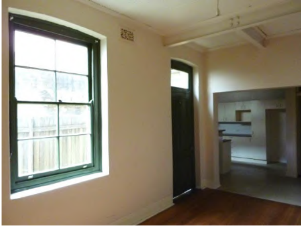
Figure 15.38 Original double-hung timber window, four panelled door with external beaded panels, with fanlight over in the dining room (space LG.1)—56B / 46–56 Gloucester Street. (Source: GML Heritage 2015)
