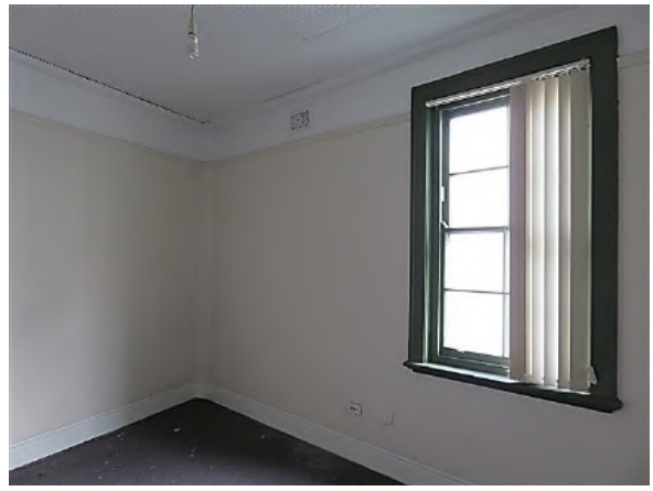
Figure 8.37 Rear bedroom (space 1.6) showing original double hung sash window and ripple iron ceiling with cement skirtings and carpeted timber floor—52A / 46–56 Gloucester Street. (Source: GML Heritage, July 2016)
