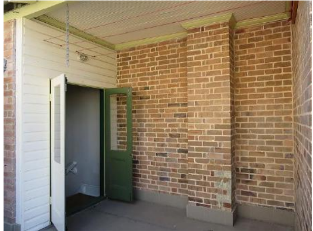
Figure 16.15 Roof over terrace (space E.1) showing the ripple iron ceiling, timber cornice. Patching of brickwork provides evidence of former laundry copper which has been removed—56C / 46–56 Gloucester Street. (Source: GML Heritage, July 2016)
