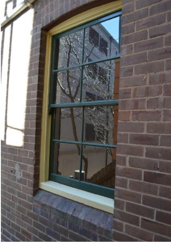
Figure 1.50 External timber double-hung sash window with brick arch and chamfered brick sill—46/46–56 Gloucester Street. (Source: GML Heritage, July 2016)
