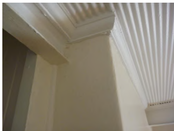
Figure 4.56 Ripple iron ceiling and cornice detail, typical of lower ground, first and second floor levels (Flat 46). (Source: GML 2015)
