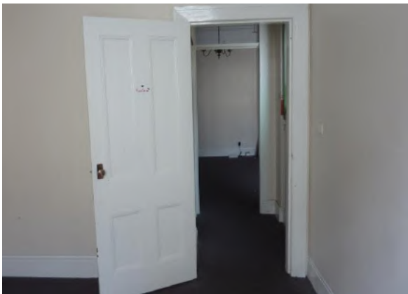
Figure 6.30 Original timber four-panel door to the rear bedroom (space 1.6)—50A / 46–56 Gloucester Street. (Source: GML Heritage, July 2016)
