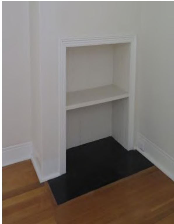
Figure 3.37 The original fireplace with original concrete hearth, later boarded out and fitted with modern shelving (space LG.1)—48 / 46–56 Gloucester Street. (Source: GML Heritage, May 2016)
