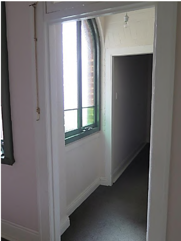
Figure 9.16 Infilled former rear porch opening (space G.4), with unrendered painted brick walls, arched modern casement window and modern T&G boarding below—54 / 46–56 Gloucester Street. (Source: GML Heritage, July 2016)
