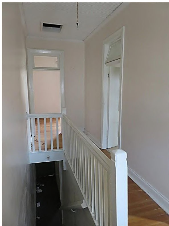
Figure 8.41 Second floor landing (space 2.1) showing timber floors, balustrade, square newel post, moulded handrail, ripple iron ceiling and cement skirting—52A / 46–56 Gloucester Street. (Source: GML Heritage, July 2016)
