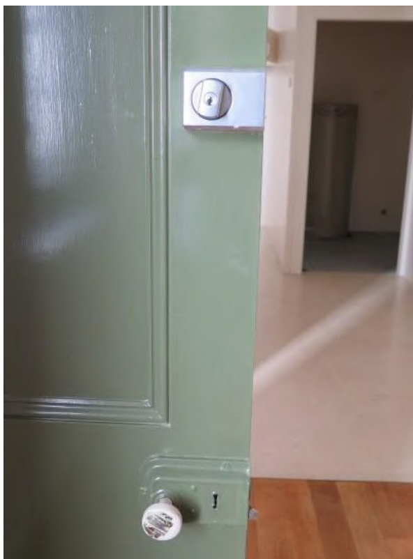
Figure 3.40 Modern/reproduction door fittings on the rear external door in dining room (space LG.1)—48 / 46–56 Gloucester Street. (Source: GML Heritage, May 2016)
