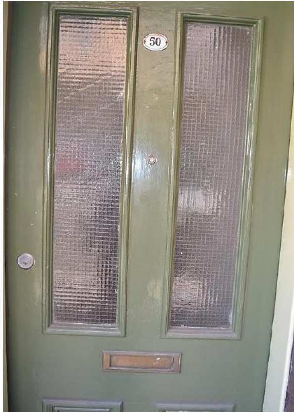
Figure 5.11 Four panel front door with bolection moulds to bottom panels and wired glass to top panels with original letter slot—50 / 46–56 Gloucester Street. (Source: GML Heritage, June 2016)
