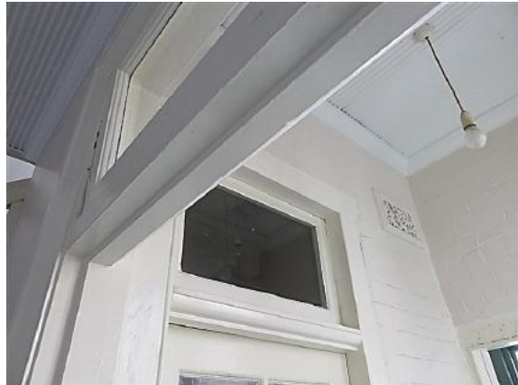
Figure 12.29 Original door frames, showing original transom and fanlight detail. Space 1.4 (the former porch) has painted brick walls and brick arched heads above the door openings. The space has a ripple iron ceiling with moulded timber cornice—54C / 46–56 Gloucester Street. (Source: GML Heritage, July 2016)
