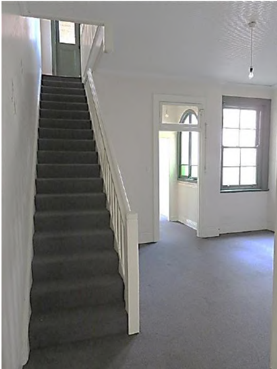
Figure 12.36 Original timber stair rising to second floor. The bottom of the newel post projects below the ceiling—54C / 46–56 Gloucester Street. (Source: GML Heritage, July 2016)
