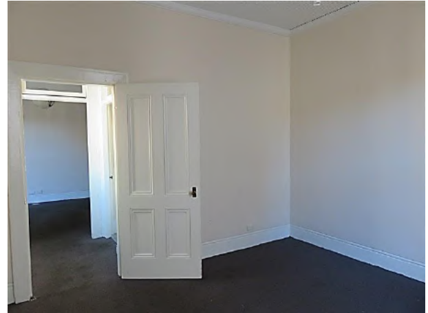
Figure 16.35 Rear bedroom (space 1.6) showing cement rendered skirtings and four panel door (reproduction) and original architrave—56C / 46–56 Gloucester Street. (Source: GML Heritage, July 2016)
