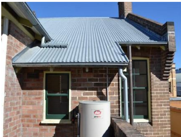
Figure 2.17 Rear elevation of Flat 46A showing corrugated metal roof and guttering—46A/46–56 Gloucester Street. (Source: GML Heritage, July 2016)
