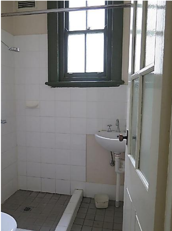
Figure 7.18 The bathroom (space G.5) showing modern tiling and fitout—52 / 46-56 Gloucester Street. The double-hung window with its sillboard and architrave is original (Source: GML Heritage, May 2016)
