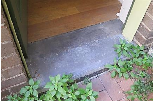
Figure 13.36 Painted concrete threshold to rear door (space LG.1)—56 / 46–56 Gloucester Street. (Source: GML Heritage, July 2016)
