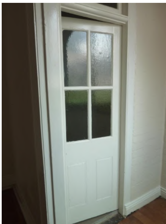
Figure 15.29 Modern half-glazed timber door to the bathroom (space G.5) with modern fit-out—56B / 46–56 Gloucester Street. (Source: GML Heritage, November 2015)
