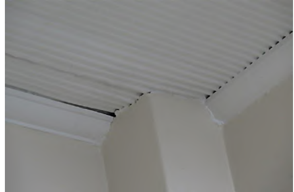
Figure 13.33 Kitchen ceiling (space LG.2) showing ripple iron ceiling with timber cornices around top of chimney flue—56 / 46–56 Gloucester Street. (Source: GML Heritage, July 2016)
