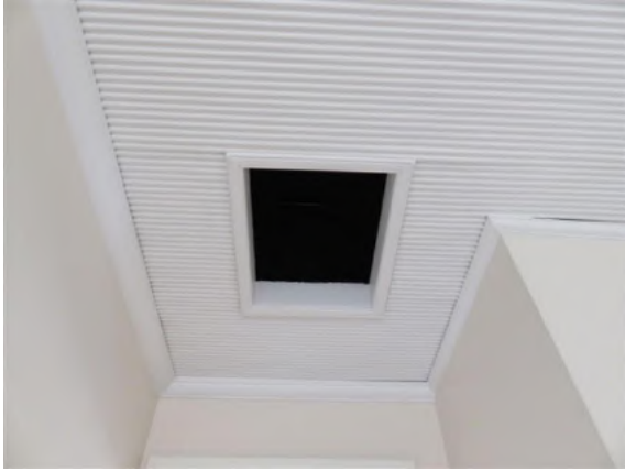
Figure 10.40 Second floor landing ceiling (space 2.1) showing roof hatch and architrave with ripple iron ceiling—54A / 46–56 Gloucester Street—54A / 46–56 Gloucester Street. (Source: GML Heritage, July 2016)
