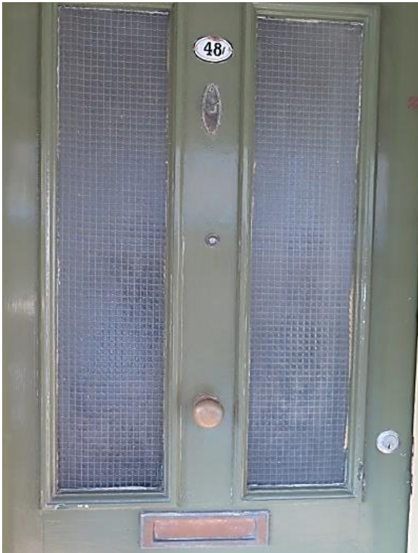
Figure 4.20 Original door knob, letter slot, bell twist and enamel number plate on front door—48A / 46–56 Gloucester Street. (Source: GML Heritage, May 2016)
