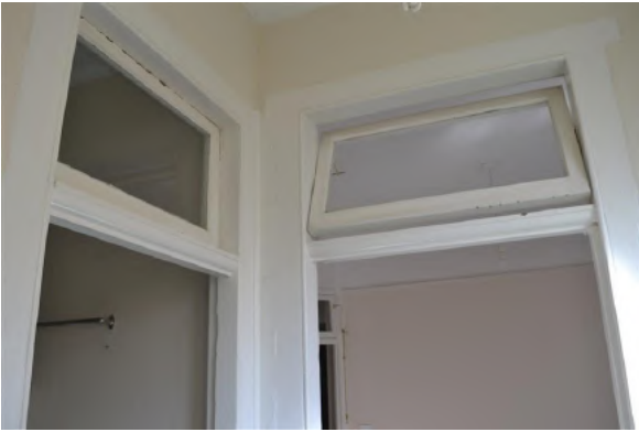
Figure 2.29 Original fanlights above doorway opening to bathroom (space 1.5) and living room (space 1.3) from the former porch (space 1.4)—46A/46–56 Gloucester Street. (Source: GML Heritage, July 2016)
