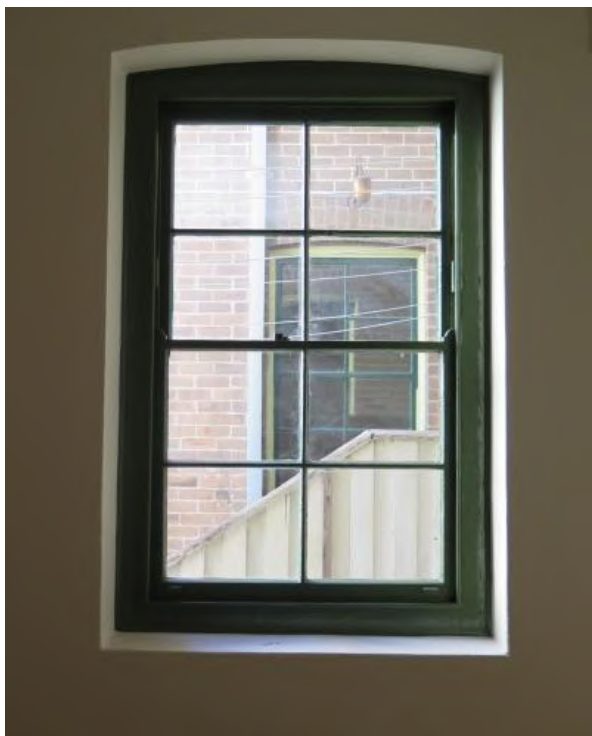
Figure 3.38 Four-over-four timber double-hung sash window in the dining room (space LG.1)—48 / 46–56 Gloucester Street. (Source: GML Heritage, May 2016)
