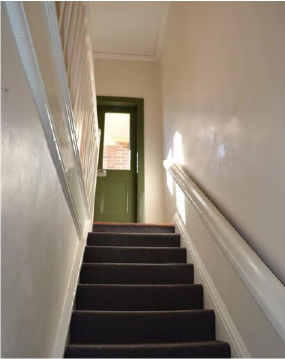
Figure 2.37 Staircase (space 1.7) showing the moulded timber handrail and carpeted treads—46A/46–56 Gloucester Street. (Source: GML Heritage, July 2016)
