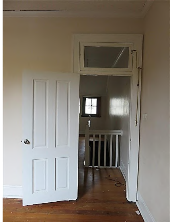
Figure 8.51 Four panel door and fanlight to space 2.4 with original architraves and original cement rendered skirting with timber quad mould—52A / 46–56 Gloucester Street. (Source: GML Heritage, July 2016)
