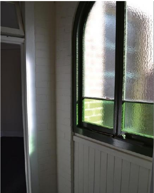
Figure 2.31 Original arched opening to former porch in rear wing (space 1.4), infilled with pair of casement windows and vertical boarded panel below—46A / 46–56 Gloucester Street. (Source: GML Heritage, July 2016)
