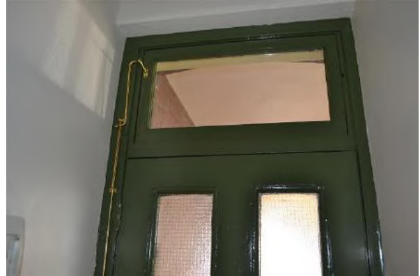
Figure 1.15 Original fanlight and reproduction fanlight mechanism to front door—46/46–56 Gloucester Street. (Source: GML Heritage, July 2016)
