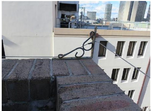
Figure 16.17 Top of brick balustrade around roof terrace (space E.1) showing decorative metal bracket for the clothesline—56C / 46–56 Gloucester Street. (Source: GML Heritage, July 2016)
