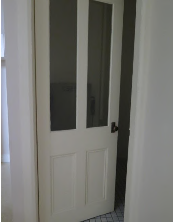
Figure 11.34 Entry to laundry (space LG.3) showing part glazed timber panel door—54B / 46–56 Gloucester Street. (Source: GML Heritage, July 2016)
