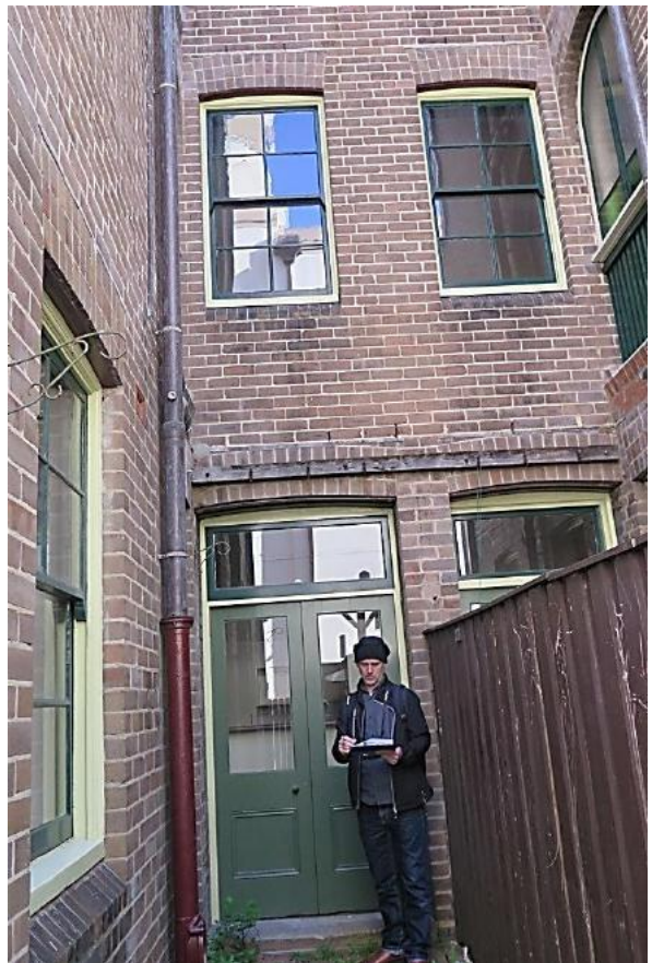
Figure 13.39 Exterior elevation (from space E.2) showing service pipes from flat above, part of reconstructed laundry hoist and later double doors to kitchen (space LG.2)—56 / 46–56 Gloucester Street. (Source: GML Heritage, June 2016)
