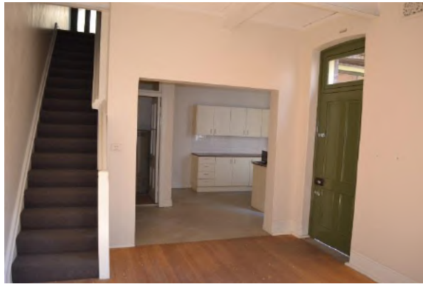
Figure 1.37 Lower ground floor level, showing the original timber stair, large opening cut through to kitchen (space LG.2) and enclosure to create a laundry under the stairs c1988 (space LG.3)—46/46–56 Gloucester Street. (Source: GML Heritage, July 2016)
