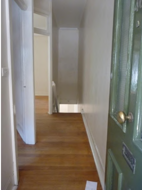
Figure 1.14 Entry (space G.1) showing timber floor cement run skirting and timber door frames to the living room (space G.3) — 46/46–56 Gloucester Street. (Source: GML Heritage, July 2016)
