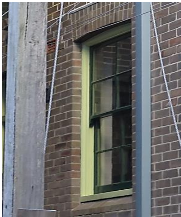
Figure 3.57 Triple brick arched head (typical detail to the 46-56 Gloucester Street flats) and typical chamfered brick window sill to the exterior rear wing of the flat—48 / 46–56 Gloucester Street. (Source: GML Heritage, May 2016)
