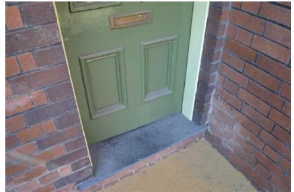
Figure 5.9 Slate threshold and dark brick surround to the front door—50 / 46–56 Gloucester Street. (Source: GML Heritage, June 2016)
