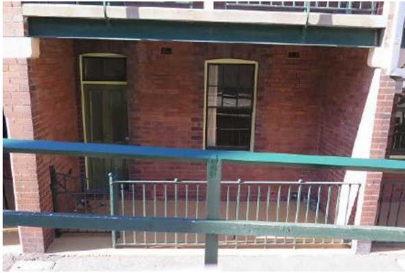
Figure 3.6 The front façade—48 / 46–56 Gloucester Street—showing external walls, projecting party walls with sandstone bolsters, wrought iron fence with square pales, wrought iron gate and the front yard (space E.1). (Source: GML Heritage, May 2016)
