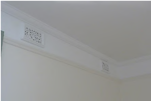
Figure 1.20 Front bedroom (space G.2) showing detail of timber picture rail, decorative plaster wall vent and plasterboard ceiling—46/46–56 Gloucester Street. (Source: GML Heritage, July 2016)
