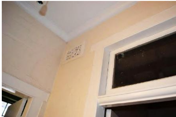
Figure 1.29 Infilled former porch opening (space G.4) showing the arched brick heads above door, decorative plaster wall vent and plaster ceiling—46/46–56 Gloucester Street. (Source: GML Heritage, July 2016)
