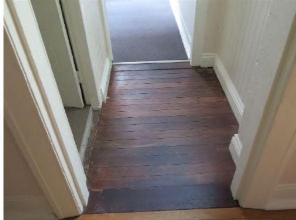
Figure 11.19 The raised timber floor of the former rear porch (space G.4) with original timber thresholds—54B / 46–56 Gloucester Street. (Source: GML Heritage, July 2016)
