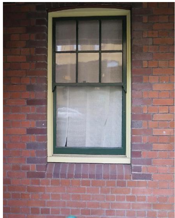
Figure 7.9 Detail of western elevation to Flat 52 at ground floor level, showing double hung sash window, chamfered sill and dark brick surround—52 / 46–56 Gloucester Street (Source: GML Heritage, July 2016)
