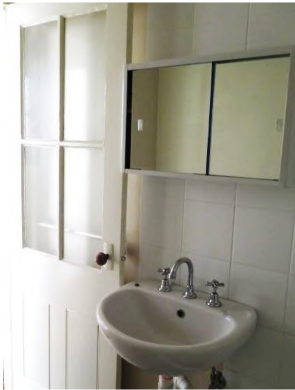
Figure 3.29 The bathroom (space G.5) showing modern fitout and original part glazed panel door. Fanlight over door matches all others in the flat (refer to Figure 3.24)—48 / 46–56 Gloucester Street. (Source: GML Heritage, May 2016)
