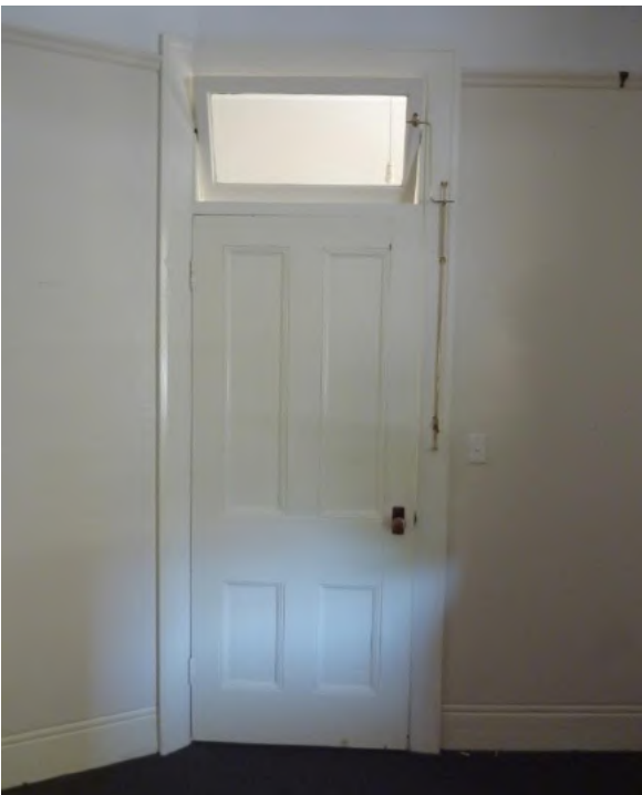
Figure 2.21 Front bedroom (space 1.2) with cement rendered skirting, picture rail and original four panel timber door with sunk moulds, original architrave and fanlight over—46A/46–56 Gloucester Street. (Source: GML Heritage, November 2015)
