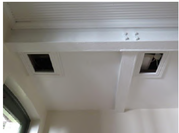
Figure 3.33 Exposed original steel transverse I-beam and trimmer in the dining room (space LG.1) showing ripple iron ceiling with fibrous plaster cornice and later ceiling and access to services void—48 / 46–56 Gloucester Street. (Source: GML Heritage, May 2016)
