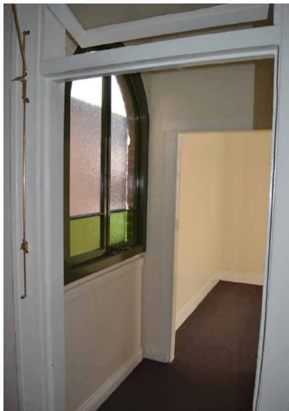
Figure 6.25 Original arched opening to former porch in rear wing (space 1.4) —50A / 48–56 Gloucester Street, infilled with pair of casement windows and vertical boarded panel below. Also shows original door frame and architrave between spaces 1.3 and 1.4, and original fanlight above. (Source: GML Heritage, July 2016)
