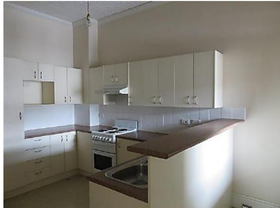
Figure 10.43 Kitchen (space 2.3) showing late twentieth century fitout, original ripple iron ceiling and timber cornice. A chimney flue rises in the northwest corner—54A / 46–56 Gloucester Street. (Source: GML Heritage, July 2016)
