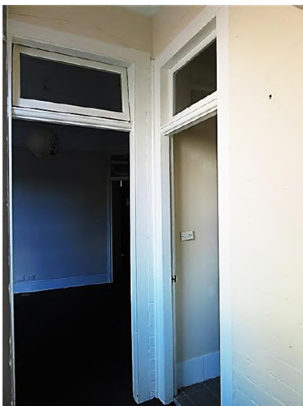
Figure 16.28 The original timber door frames with central pivot fanlights over open into space 1.4 (former porch). Walls are painted brickwork. Arched brick heads are visible over the door openings—56C / 46–56 Gloucester Street. (Source: GML Heritage, July 2016)
