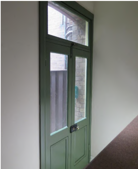
Figure 11.36 Modern half-glazed double French doors from the kitchen (space LG.2) to the rear yard—54B / 46–56 Gloucester Street. (Source: GML Heritage, July 2016)
