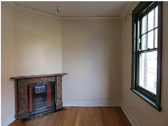
Figure 12.44 Front room on the second floor (space 2.4) showing the fireplace, timber double hung window, cement run skirting, ripple iron ceiling and moulded timber cornice—54C / 46–56 Gloucester Street. (Source: GML Heritage, July 2016)
