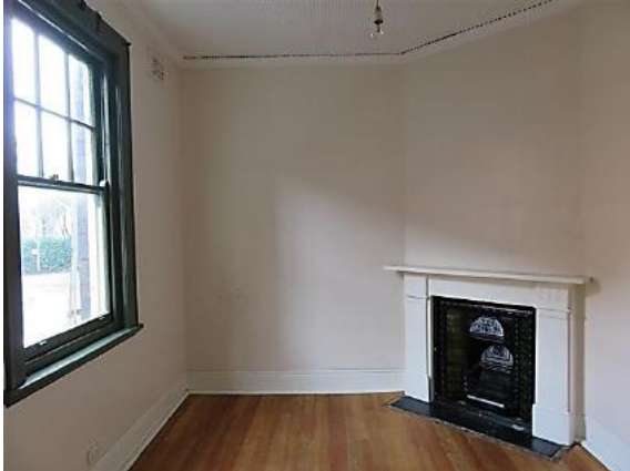
Figure 10.48 Front room on the second floor (space 2.4) showing the original double hung window, fireplace, timber floor, cement run skirting, timber cornice and ripple iron ceiling—54A / 46–56 Gloucester Street. (Source: GML Heritage, July 2016)
