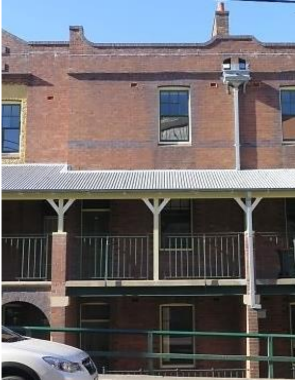
Figure 4.6 Overall façade of 48 and 48A Gloucester Street, showing front verandah (common property), shared guttering and downpipe, brick parapet and brick chimney on the boundary with 50 and 50A Gloucester Street. (Source: GML Heritage, May 2016)
