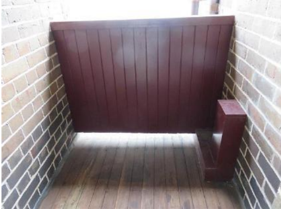
Figure 10.16 Vertical timber V-jointed boarding to balcony balustrade (space 2.3)—54A / 46–56 Gloucester Street. (Source: GML Heritage, July 2016)
