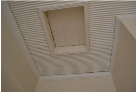
Figure 6.34 Ceiling of space 2.1 showing original roof hatch, timber cornice and ripple iron ceiling—50A / 46–56 Gloucester Street. (Source: GML Heritage, July 2016)
