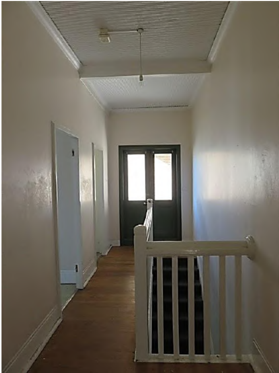
Figure 14.37 Second floor landing (space 2.1) looking east showing timber balustrade with moulded handrail, square balusters and chamfered top to newel posts, cement rendered skirting and half glazed timber doors to the roof terrace—56A / 46–56 Gloucester Street. (Source: GML Heritage, July 2016)
