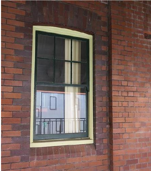
Figure 16.10 Front façade of flat 56C showing face brick external wall with contrasting brick surround to window, arched brick head and chamfered brick window sill—56C / 46–56 Gloucester Street. (Source: GML Heritage, July 2016)
