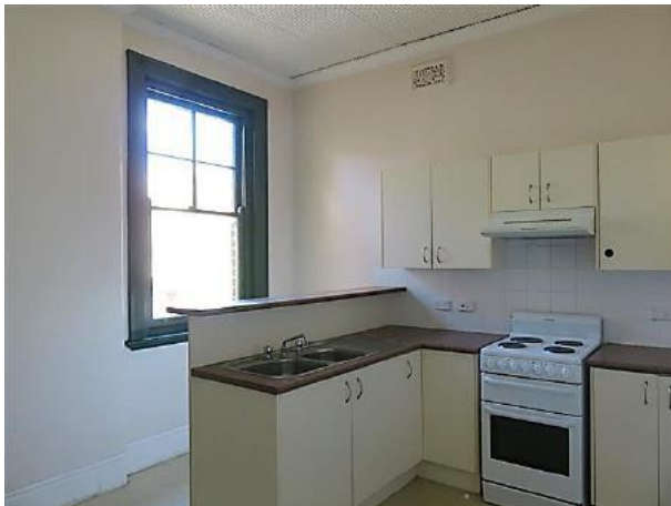
Figure 16.44 Kitchen (space 2.3) showing original window with architrave, sill board and moulding, cement run skirting, timber cornice and ripple iron ceiling—56C / 46–56 Gloucester Street. (Source: GML Heritage, July 2016)
