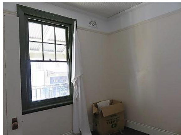
Figure 14.19 Front bedroom (space 1.2) showing timber double hung sash window, moulded timber picture rail and ripple iron ceiling with moulded timber cornice—56A / 46–56 Gloucester Street. (Source: GML Heritage, July 2016)
