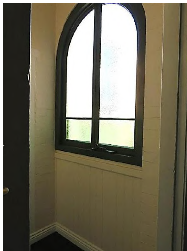
Figure 16.29 Original arched opening to former porch in rear wing (space 1.4), infilled with pair of casement windows and vertical boarded panel below. The space has a moulded timber skirting (not original)—56C / 46–56 Gloucester Street. (Source: GML Heritage, July 2016)
