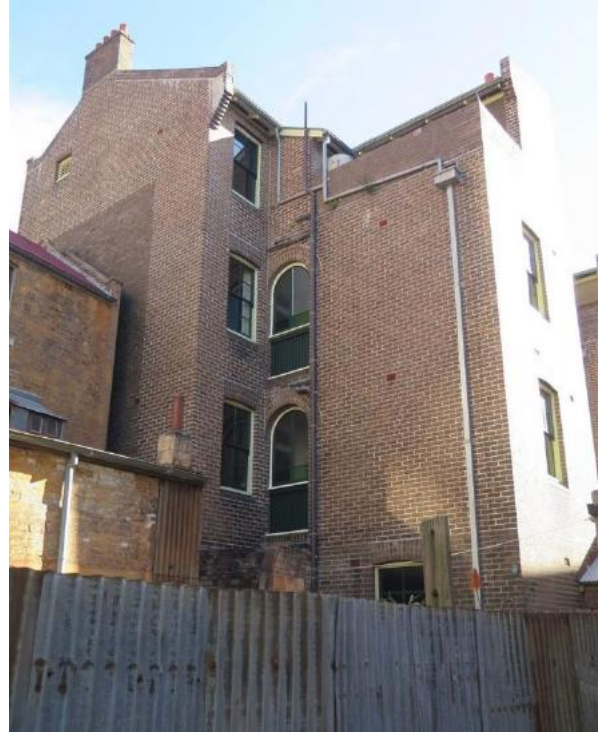
Figure 15.51 Southeastern rear elevation of Flat 56B showing rear porch window infill—56B / 46–56 Gloucester Street. (Source: GML Heritage, July 2016)
