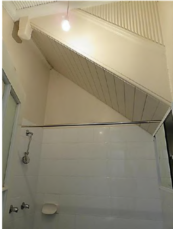
Figure 14.30 Bathroom (space 1.5) showing modern fit out, v-jointed timber stair soffit with ripple iron to ceiling and side of stair above the string—56A / 46–56 Gloucester Street. (Source: GML Heritage, July 2016)
