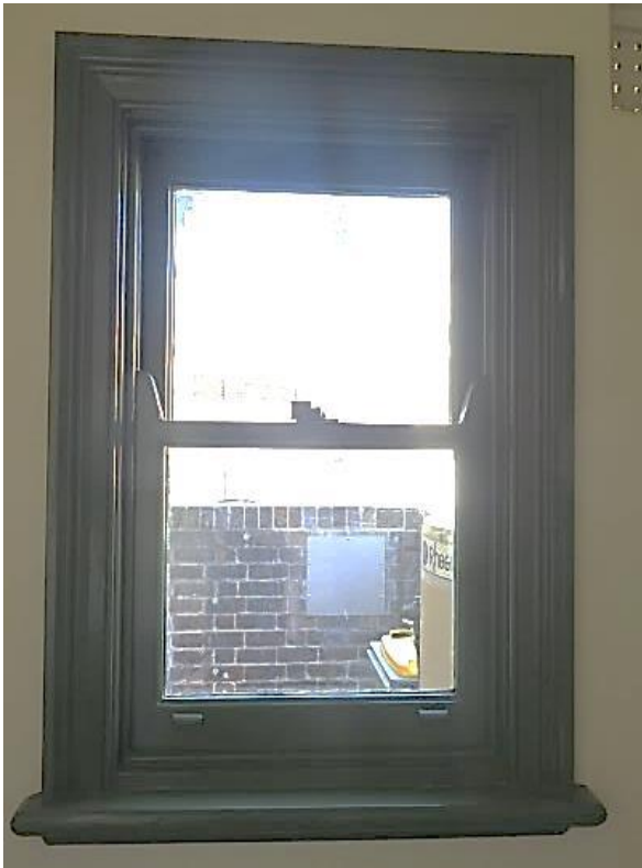
Figure 4.48 Timber spiral balance sash window in laundry (space 2.2)—48A / 46–56 Gloucester Street. (Source: GML Heritage, May 2016)
