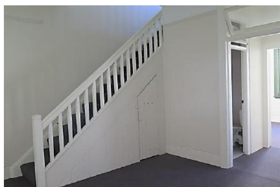
Figure 4.29 Living room (space 1.3)—48A / 46–56 Gloucester Street, showing timber balustrade and original T&G timber boarded stairs and ledged and sheeted door. (Source: GML Heritage, May 2016)
