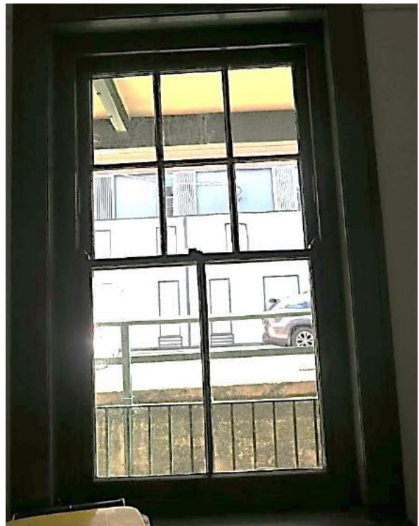
Figure 13.17 Timber double-hung sash window, architrave and sill board in front bedroom (space G.2)—56 / 46-56 Gloucester Street. (Source: GML Heritage, July 2016)
