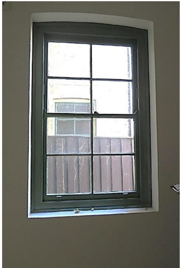
Figure 13.31 original timber double hung sash window (space LG.1)—56 / 46–56 Gloucester Street. (Source: GML Heritage, July 2016)
