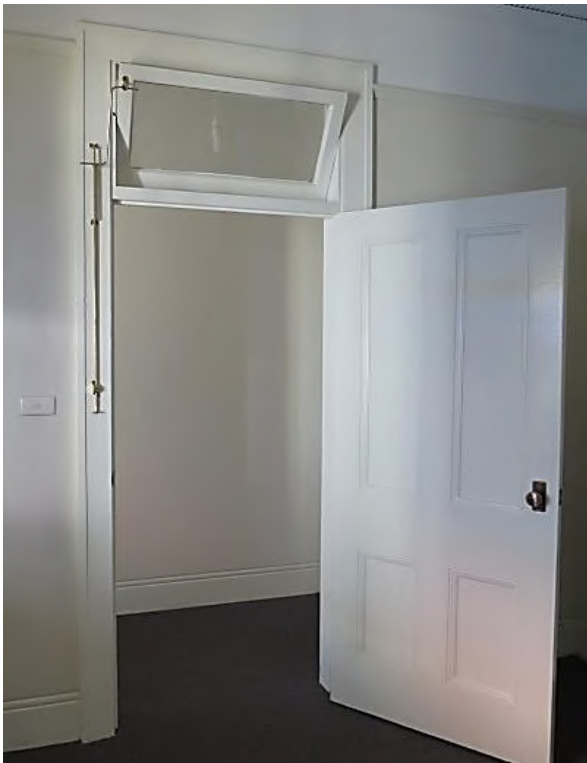
Figure 4.24 Four-panel timber door with fanlight above and reproduction mechanism between front bedroom (space 1.2) and entry (space 1.1)—48A / 46–56 Gloucester Street. (Source: GML Heritage, May 2015)
