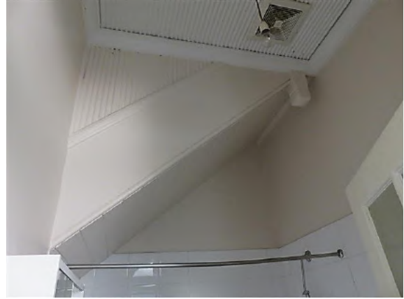
Figure 12.31 Bathroom (space 1.5) showing soffit of the stair lined with v-jointed timber boarding beneath and ripple iron to the ceiling and side of stair above the stringer. The bottom of the stair newel post projects below the stair—54C / 46–56 Gloucester Street. (Source: GML Heritage, July 2016)
