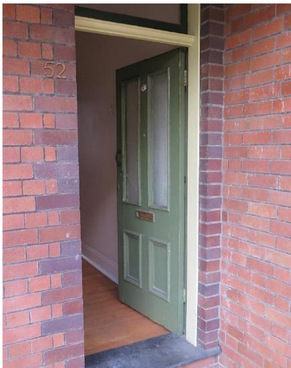
Figure 7.8 The four-panel front door with bolection moulds to bottom panels and wired glass to top panels, fanlight above, dark brick surround, number plate and slate threshold—52 / 46–56 Gloucester Street (Source: GML Heritage, July 2016)
