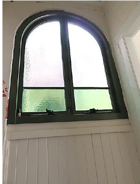
Figure 14.26 Original arched opening to former porch in rear wing (space 1.4), infilled with pair of casement windows and vertical boarded panel below—56A / 46–56 Gloucester Street. (Source: GML Heritage, July 2016)
