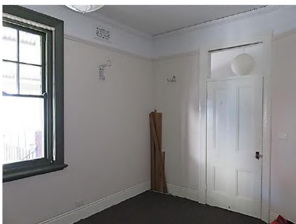
Figure 16.20 Front bedroom (space 1.2) showing the cement rendered skirting, picture rail, cornice and ripple iron ceiling, as well as decorative plaster wall vent, timber double-hung sash window with original architrave, sill board and moulding and original four panel door. The fanlight over has been removed, but the architraves have been retained—56C / 46–56 Gloucester Street. (Source: GML Heritage, July 2016)
