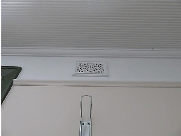
Figure 16.22 Front bedroom (space 1.2) showing moulded timber picture rail, cornice, ripple iron ceiling and decorative plaster wall vent—56C / 46–56 Gloucester Street. (Source: GML Heritage, July 2016)
