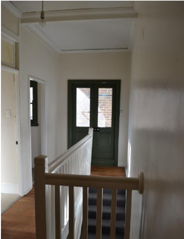
Figure 6.36 Second floor landing (space 2.1)—50A / 48–56 Gloucester Street looking east showing ripple iron ceiling and transverse I-beam, original timber balustrade with moulded handrail, newel posts, door frame to the kitchen, and later architrave to the laundry and half glazed timber doors to the roof terrace. (Source: GML Heritage, July 2016)
