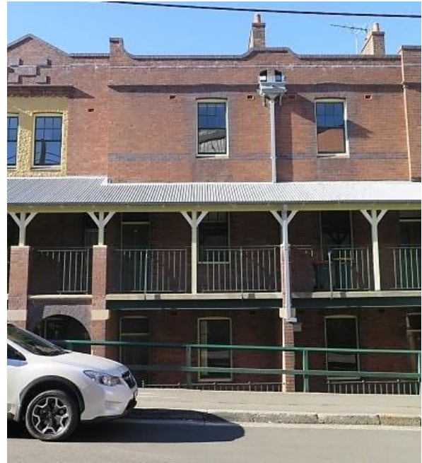
Figure 3.7 Overall façade of 48 and 48A / 46–56 Gloucester Street, showing the shared front verandah, shared guttering, and brick chimney at the ridge line over the boundary with 50 and 50A Gloucester Street. (Source: GML Heritage, May 2016)
