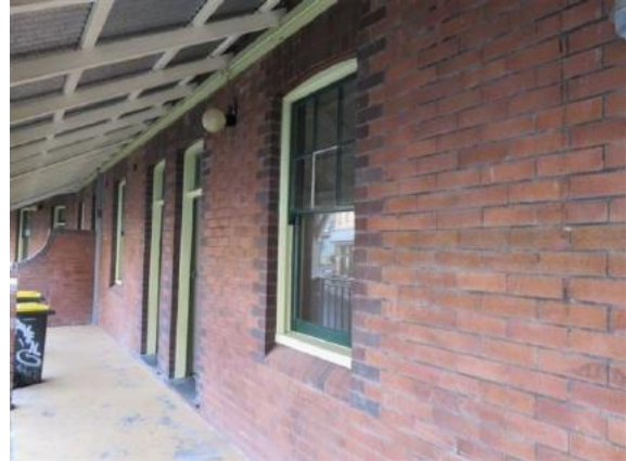
Figure 12.7 Front facades of flats 54A and 54C showing face brick external walls with contrasting brick surround to window and door openings—54C / 46–56 Gloucester Street. (Source: GML Heritage, July 2016)
