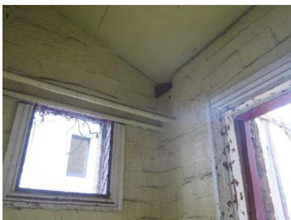
Figure 11.40 Interior of WC showing rendered painted brick (space E.3)—54B / 46–56 Gloucester Street. (Source: GML Heritage, July 2016)
