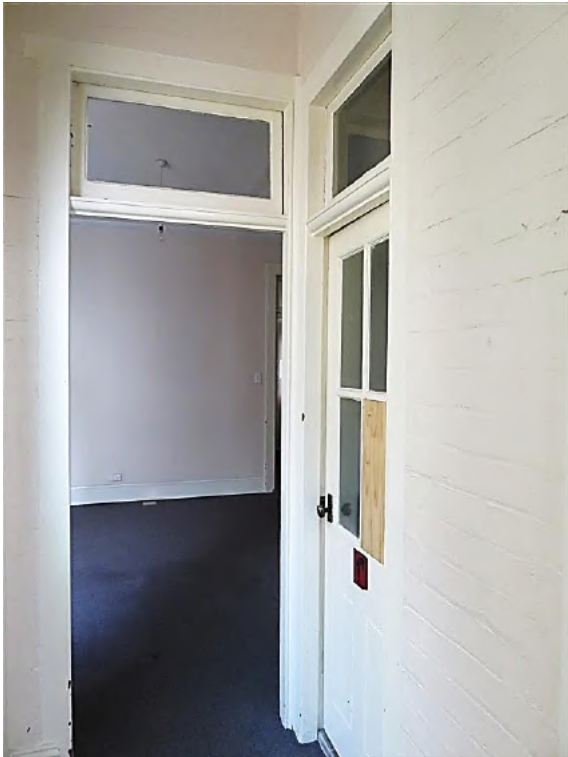
Figure 12.28 Original door frames with original fanlights and brick heads above (space 1.4). The half glazed door to the bathroom (space 1.5) is original. The door to space 1.3 is missing—54C / 46–56 Gloucester Street. (Source: GML Heritage, July 2016)
