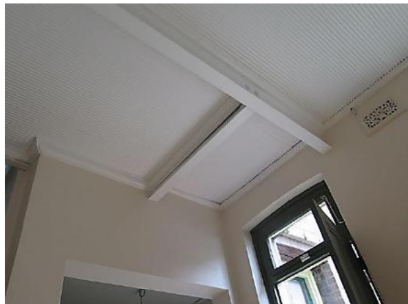
Figure 9.25 Steel beams supporting walls above and ripple iron ceiling (space LG.1)—54 / 46–56 Gloucester Street. (Source: GML Heritage, July 2016)
