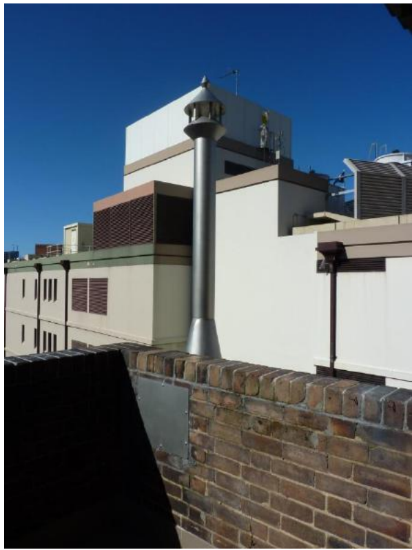
Figure 4.20 The solid brick balustrade to the roof terrace showing the cover over opening to reconstructed garbage chute (Flat 46A). (Source: GML 2015)
