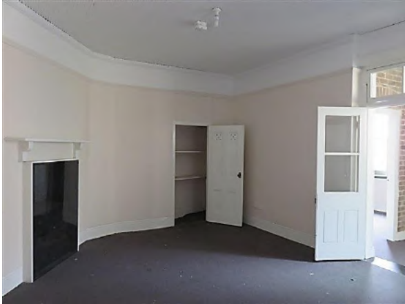
Figure 8.22 Living room (space 1.3) showing the ripple iron ceiling with moulded timber cornice, moulded timber picture rail and cement rendered skirting, original mantel shelf and cupboard—52A / 46–56 Gloucester Street. (Source: GML Heritage, July 2016)
