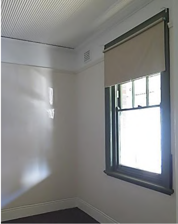
Figure 4.22 Front bedroom (space 1.2)—48A / 46–56 Gloucester Street, showing cement run skirtings, timber cornice, timber picture rail, wall vent and ripple iron ceiling. (Source: GML Heritage, May 2016)
