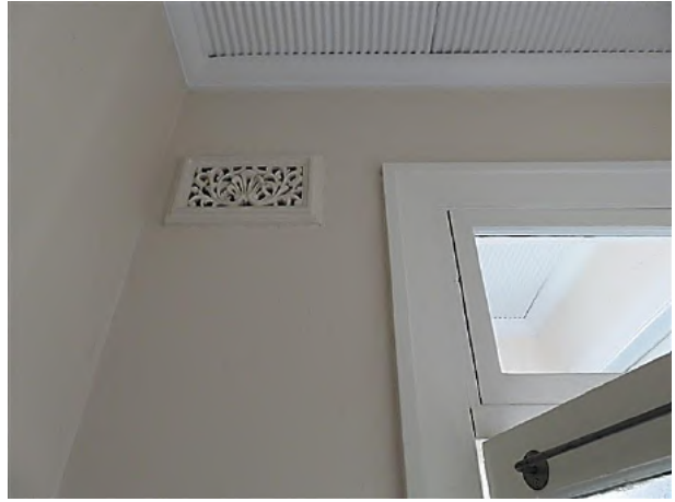
Figure 16.31 Decorative plaster wall vent in the bathroom (space 1.5)—56C / 46–56 Gloucester Street. (Source: GML Heritage, July 2016)
