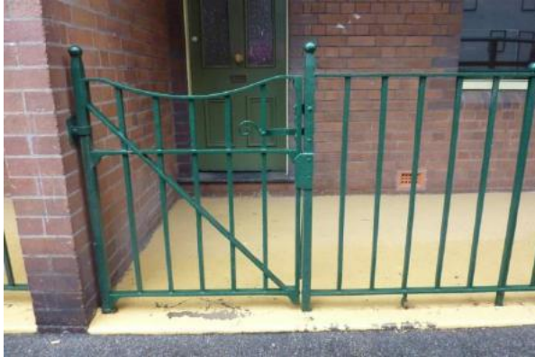
Figure 4.5 Detail of the wrought iron balustrade and gate to Flat 48, with original gate latch, at ground floor flat level on Gloucester Street. (Source: GML 2015).
