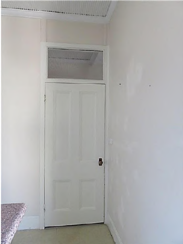
Figure 16.46 Original door in light weight concrete wall and original four panel door (space 2.3). Fanlight is missing—56C / 46–56 Gloucester Street. (Source: GML Heritage, July 2016)
