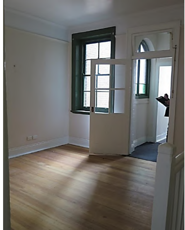
Figure 13.19 Living room (space G.3)—56 / 46–56 Gloucester Street, showing cement run skirtings, timber flooring, picture rail, and timber double-hung sash window and half-glazed timber door to rear porch (space G.4). (Source: GML Heritage, July 2016)
