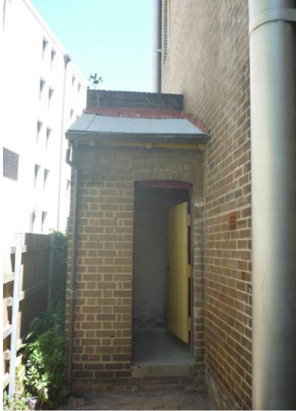
Figure 1.51 External WC or store in common brick (space E.3) with skillion roof and timber door with brick arch above—46/46–56 Gloucester Street. (Source: GML Heritage, July 2016)
