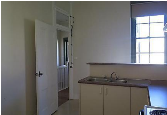
Figure 4.52 Kitchen (space 2.3) showing modern fit-out and original four-panel sunk moulded door —48A / 46–56 Gloucester Street. (Source: GML Heritage, May 2016)
