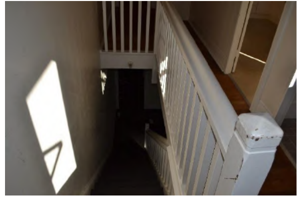
Figure 6.33 Timber balustrade and newel post to the hall/landing (space 2.1)—50A / 48–56 Gloucester Street. (Source: GML Heritage, July 2016)
