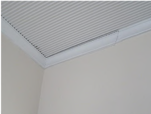
Figure 16.36 Ripple iron ceiling and moulded timber cornice in south-west corner of the rear bedroom (space 1.6)—56C / 46–56 Gloucester Street. (Source: GML Heritage, July 2016)
