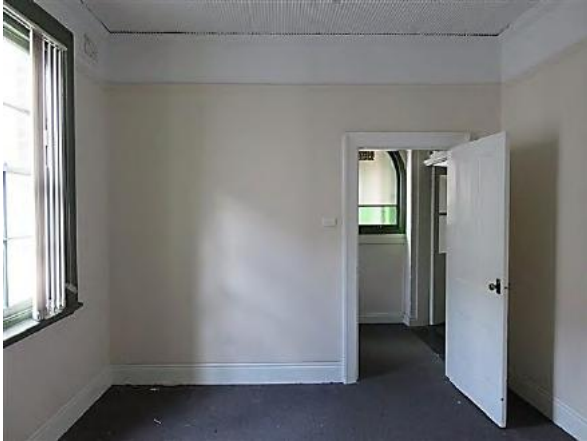
Figure 8.38 Rear bedroom (space 1.6) showing the four panel timber door, moulded timber picture rail and cement rendered skirting—52A / 46–56 Gloucester Street. (Source: GML Heritage, July 2016)
