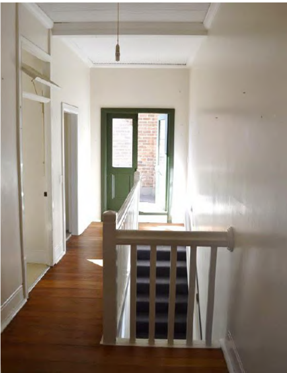
Figure 2.39 Second floor landing (space 2.1) looking east showing timber balustrade with moulded handrail, square balusters and chamfered top to newel posts, cement rendered skirting and half glazed timber doors to the roof terrace—46A/46–56 Gloucester Street. (Source: GML Heritage, July 2016)
