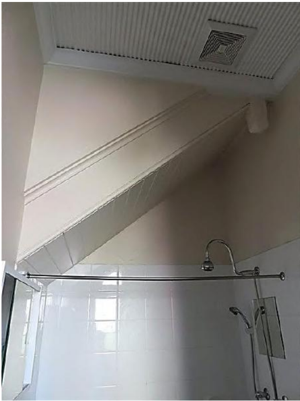
Figure 16.32 Bathroom (space 1.5) showing modern fit out, expressed stair stringer and bottom of newel post protruding through ceiling, v-jointed timber stair soffit and ripple iron ceiling with timber cornice—56C / 46–56 Gloucester Street. (Source: GML Heritage, July 2016)
