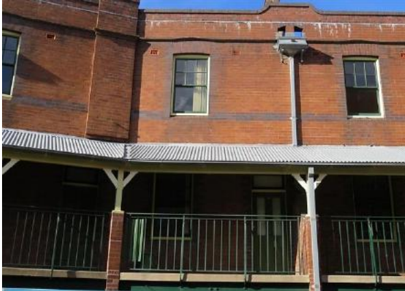
Figure 8.6 Western façade of flat 52A / 46–56 Gloucester Street, as viewed from Gloucester Street. Showing the common verandah, balustrade, face brick walls with dark brick banding and projecting string, curved parapet and timber double hung sash window to the upper floor. (Source: GML Heritage, July 2016).
