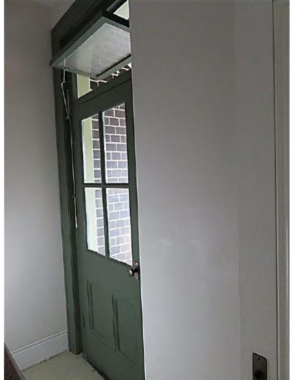
Figure 10.45 Original half glazed timber door leading onto balcony from kitchen (space 2.3), with four glass panes above two timber panels with sunk moulds and with fanlight over—54A / 46–56 Gloucester Street. (Source: GML Heritage, July 2016)
