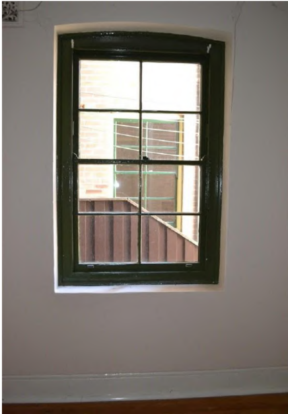
Figure 5.34 Dining room (space LG.1) showing the cement run skirting and timber double hung sash window—50 / 46–56 Gloucester Street. (Source: GML Heritage, June 2016)
