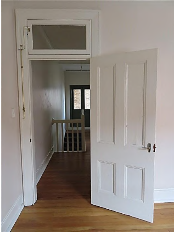
Figure 12.46 Front room on the second floor (space 2.4) showing the original four panel timber door with fanlight above with fanlight opener. The door furniture has been replaced—54C / 46–56 Gloucester Street. (Source: GML Heritage, July 2016)
