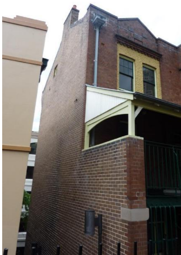
Figure 2.7 Northern façade of flat 46A showing the brick chimney stacks with terracotta pots, timber boarded gable to the verandah, and timber louvre in the main roof gable—46A/46–56 Gloucester Street. (Source: GML Heritage, November 2015)
