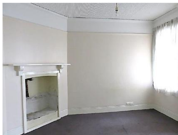
Figure 10.23 Living room (space 1.3) showing cement run skirting, ripple iron ceiling, moulded timber cornice, timber picture rail and original fireplace with mantel shelf supported on curved brackets—54A / 46–56 Gloucester Street. (Source: GML Heritage, July 2016)
