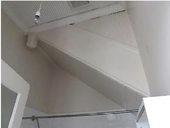
Figure 10.34 Bathroom (Space 1.5) showing v-jointed timber stair soffit with ripple iron to ceiling and side of the stair above the string—54A / 46–56 Gloucester Street. (Source: GML Heritage, July 2016)
