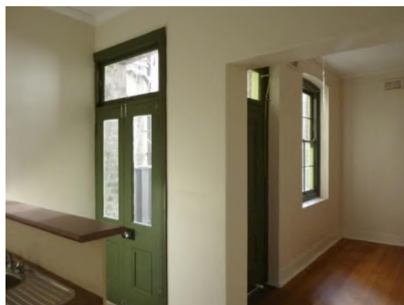
Figure 5.33 Dining room (space LG.1) and kitchen (Space LG.2) showing the double-hung sash window to the dining room and the two four panel doors with fanlights above to the rear yard (space E.2)—50 / 46–56 Gloucester Street. (Source: GML Heritage, June 2016)
