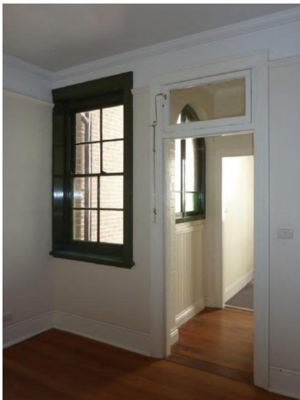
Figure 4.37 Looking into the former porch from the main living room (ground floor level, Flat 50). The original arched opening has been infilled with vertical boarding and casement windows. The main room has a cement rendered skirting, picture rail and cornice. The window and door opening have original timber architraves. (Source: GML 2015)
