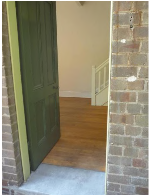
Figure 1.49 Concrete threshold to dining room door (space LG.1)—46/46–56 Gloucester Street. (Source: GML Heritage, July 2016)
