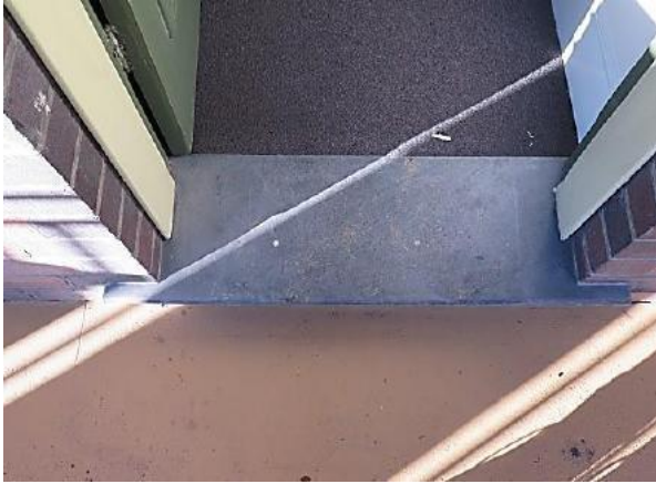
Figure 4.18 Original slate threshold to front door—48A / 46–56 Gloucester Street. (Source: GML Heritage, May 2016)
