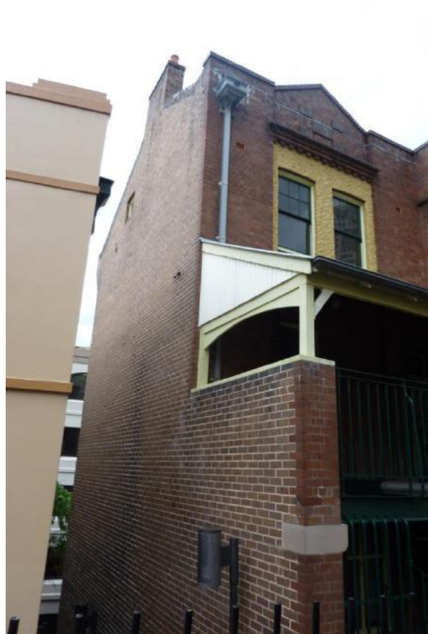
Figure 4.2 Detail of timber boarding and curved valence to northern end of the front verandah. A timber louvre ventilates the roof space over Flat 46A. (Source: GML 2015).
