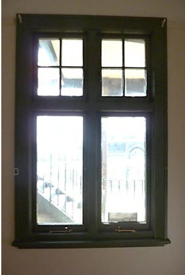
Figure 15.18 Front bedroom (space G.2) showing the casement window—56B / 46–56 Gloucester Street, (Source: GML Heritage, November 2015)
