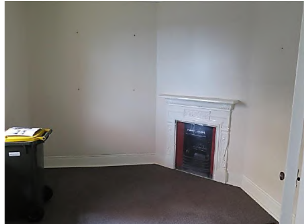
Figure 9.13 Front bedroom (space G.2) showing modern carpeting over timber floors, rendered wall finishes, rendered cement skirting and original cast iron chimney piece and grate—54 / 46–56 Gloucester Street. (Source: GML Heritage, July 2016)
