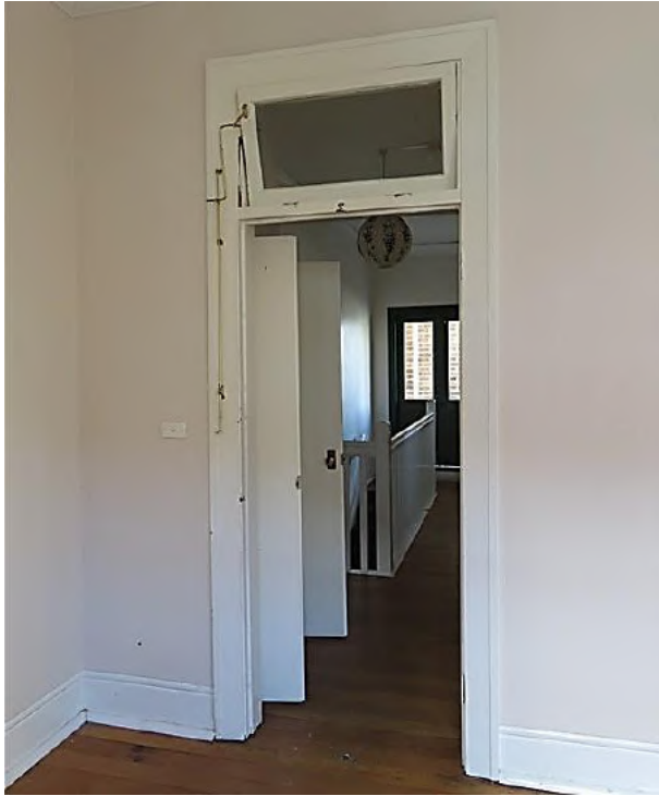
Figure 16.50 Original door frame, fanlight and architrave (door is missing) (space 2.4)—56C / 46–56 Gloucester Street. (Source: GML Heritage, July 2016)
