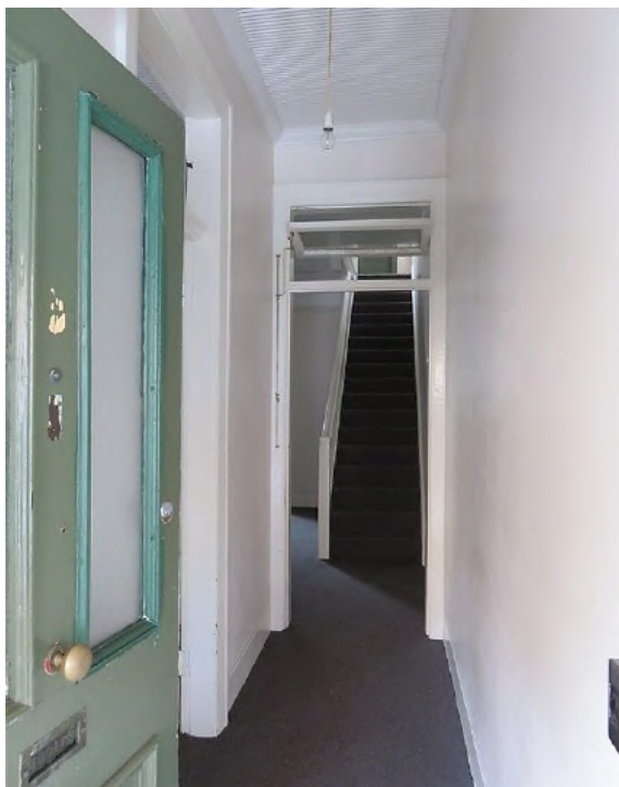
Figure 10.20 Entrance hall (space 1.1) showing the ripple iron ceiling with moulded timber cornice and cement rendered skirting. The doors opening to spaces 1.2 and 1.3 have their original fanlights—54A / 46–56 Gloucester Street. (Source: GML Heritage, July 2016)
