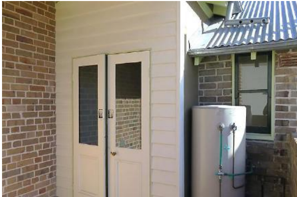
Figure 6.14 Rear wall opening onto the roof terrace—50A / 48–56 Gloucester Street (space E.1), showing recent weatherboard wall, pair of half glazed doors and rendered finish to stair hall wall. The window is also recent, replacing a previous door (Source: GML Heritage, July 2016)
