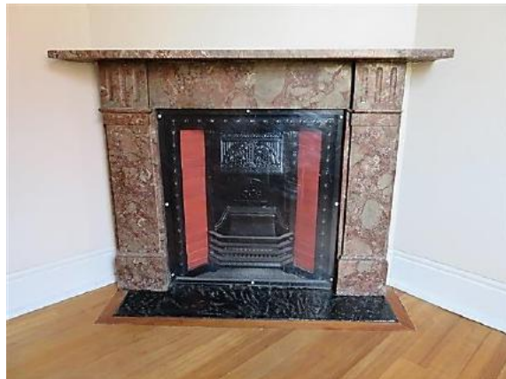
Figure 12.45 Fireplace (space 2.4) with marble chimney piece and cast iron grate with tiled sides and concrete hearth—54C / 46–56 Gloucester Street. (Source: GML Heritage, July 2016)
