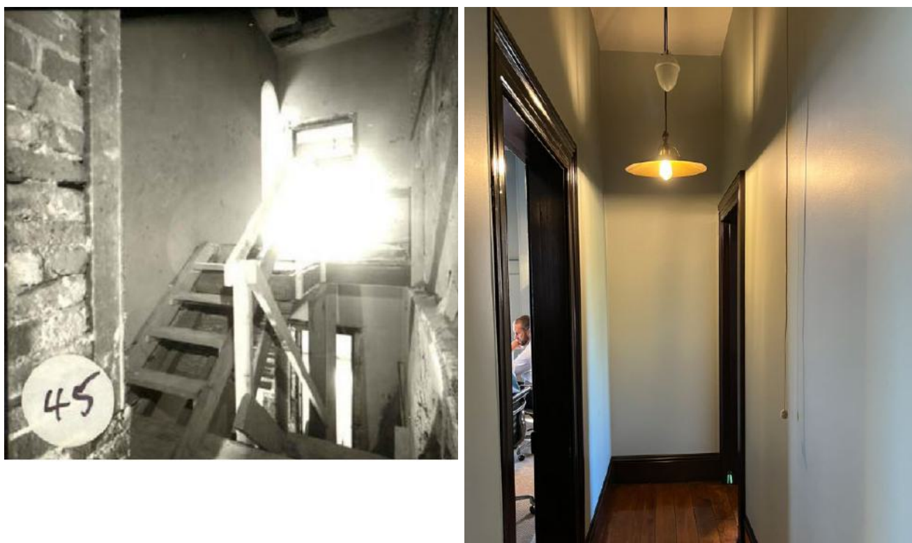
Figure 145: Room 2.3 looking west, 1995. (Source: PMNSW image 45, as reproduced in the 2015 CMP, p 128)
