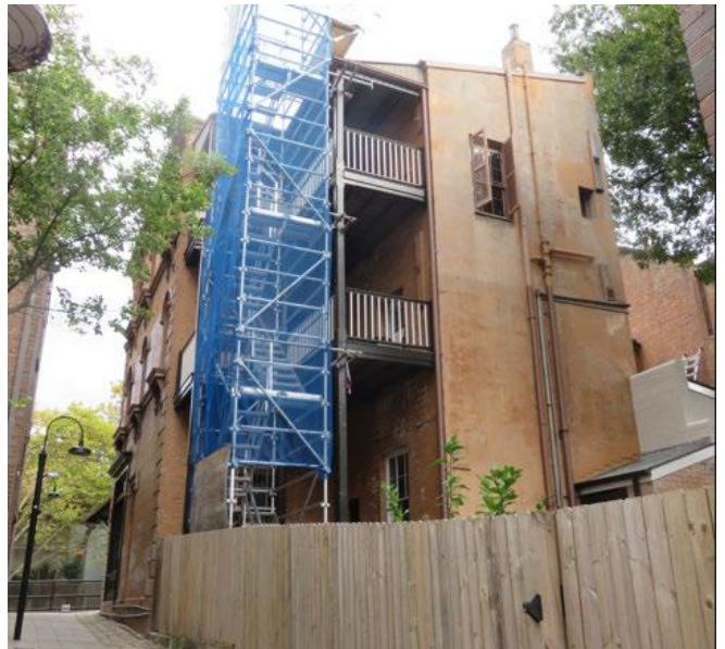
Figure 64: View 4, looking west along Long's Lane towards the rear of the building
