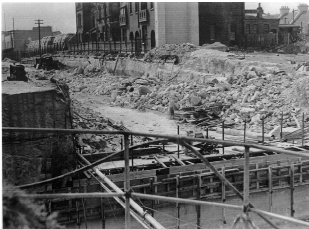
Figure 46: The lowering of Cumberland to allow the construction of the Cahill Expressway overpass over Cumberland Street, 1958. Source: SHFA
