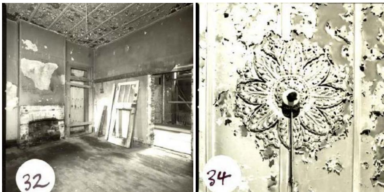
Figure 107: looking south-west in 1995. (Source: PMNSW image 32, as reproduced in the 2015 CMP, p 119)
