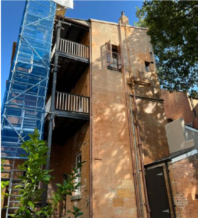
Figure 77: Rear (east) elevation of the rear wing. The wall is rendered with ashlar markings but there are no decorative mouldings.
