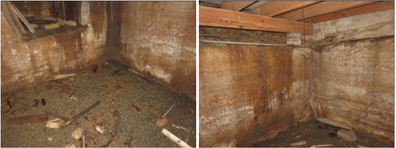
Figure 91: North-eastern corner of the basement, with cut sandstone walls. The framing of the false ceiling, supported on brick piers built off the stone, can be seen.
