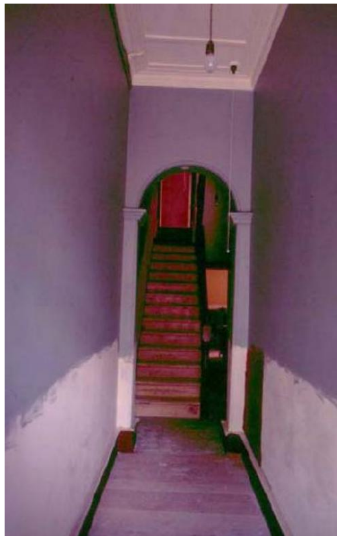
Figure 101: Looking east across room G.2 in 1997, with conservation works underway. (Source: PMNSW image 189148, as reproduced in the 2015 CMP, p 117)
