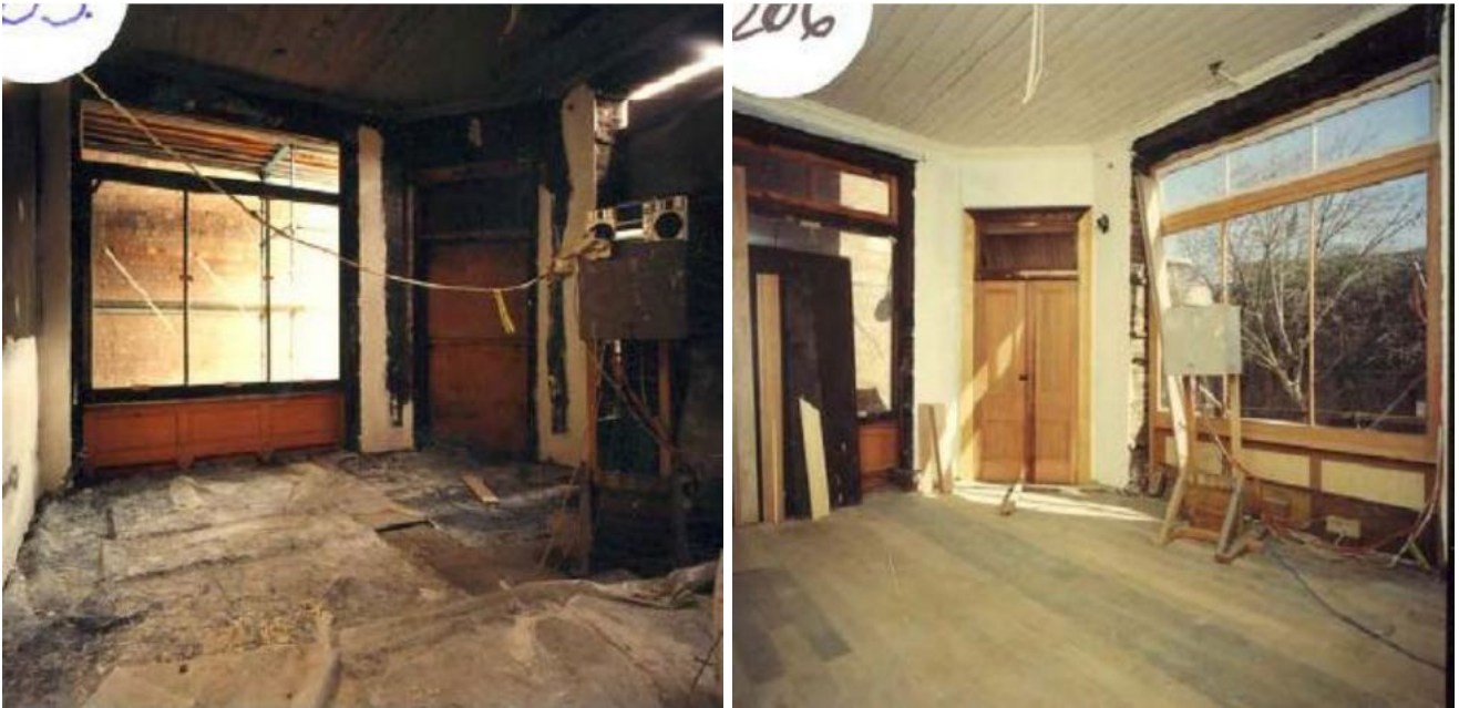
Figure 99: Looking south across room G.1 in 1997, with conservation works underway. (Source: PMNSW image 163, as reproduced in the 2015 CMP, p 115)
