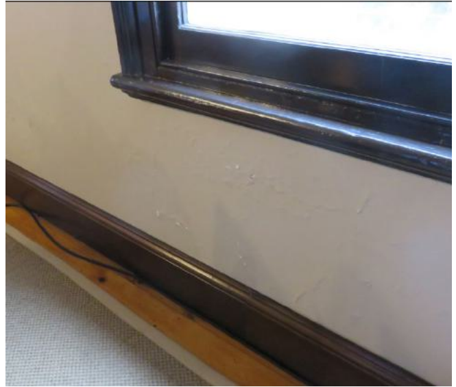
Figure 121: Evidence of damp below the northern-most window in room 1.1, 2024.
