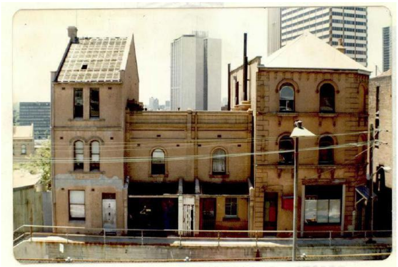
Figure 52: Nos. 130-136 Cumberland Street from the 1979 Condition Report. Source: SHFA
