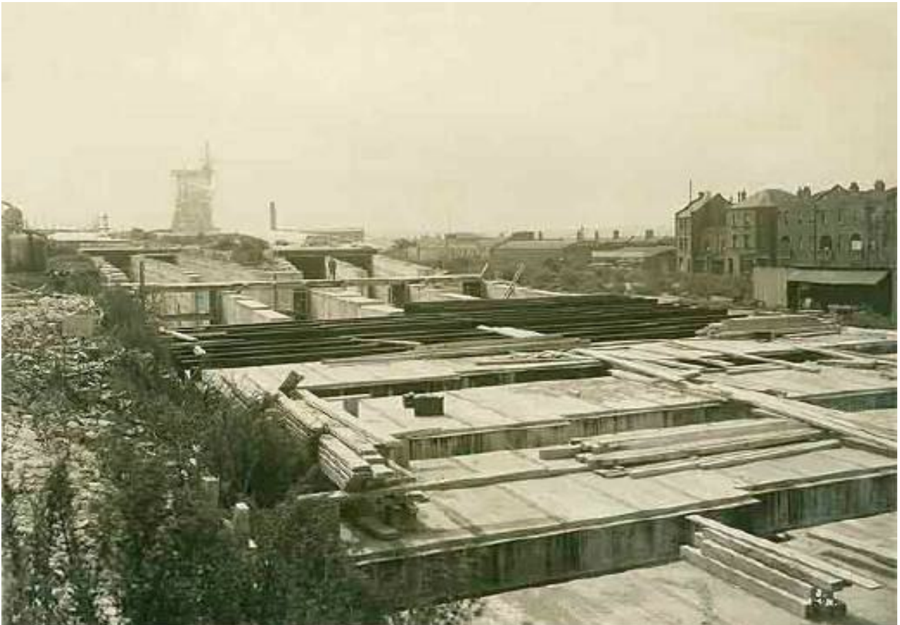
Figure 42: Construction of the southern approach to the Sydney Harbour Bridge (Bradfield Highway) was well underway by April 1930 when a photograph was taken showing the group of buildings in Cumberland Street in the distance. Source: State Records Series 12685 Sydney Harbour Bridge photographs
