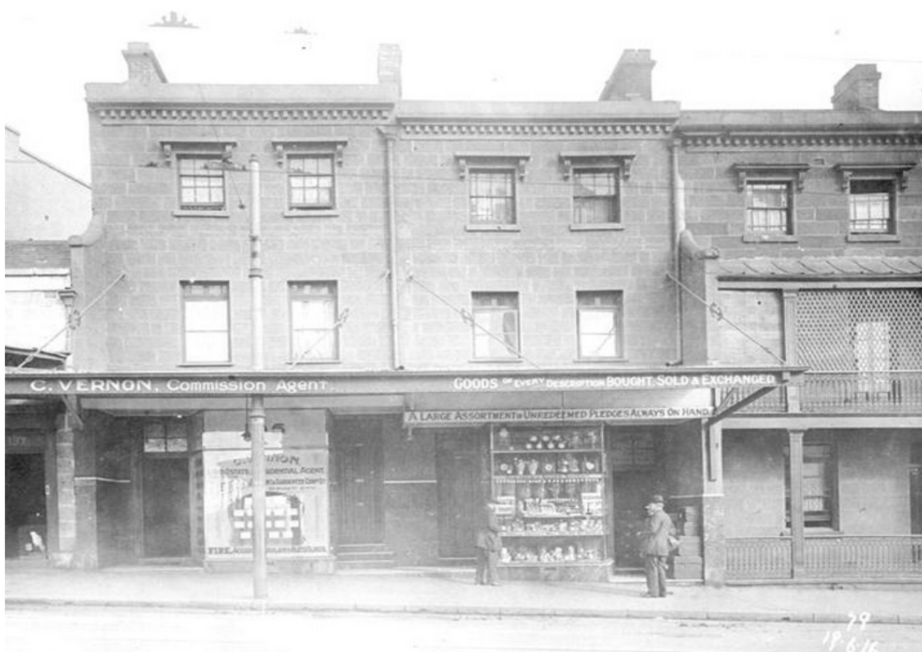
Figure 164: Pair of shops at 191-195 William Street Source: SCC Demolition Books
