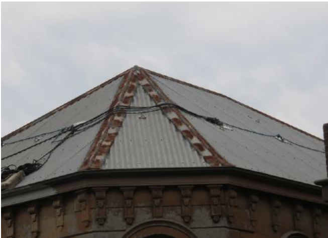
Figure 83: Detail of the main roof, showing the rust affected galvanized steel cappings. The ropes indicate that the roof harness system is in use.
