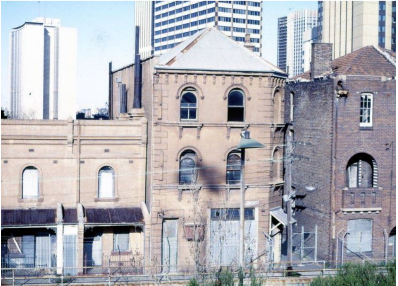
Figure 26: View east from Sydney Harbour Bridge of terrace houses, 130-138 and 140-142 Cumberland Street, The Rocks, with Longs Lane between them, 1983. All are derelict, with corrugated iron on ground floor windows, and wire mesh fence with barbed wire around them. Source: City of Sydney Archives
