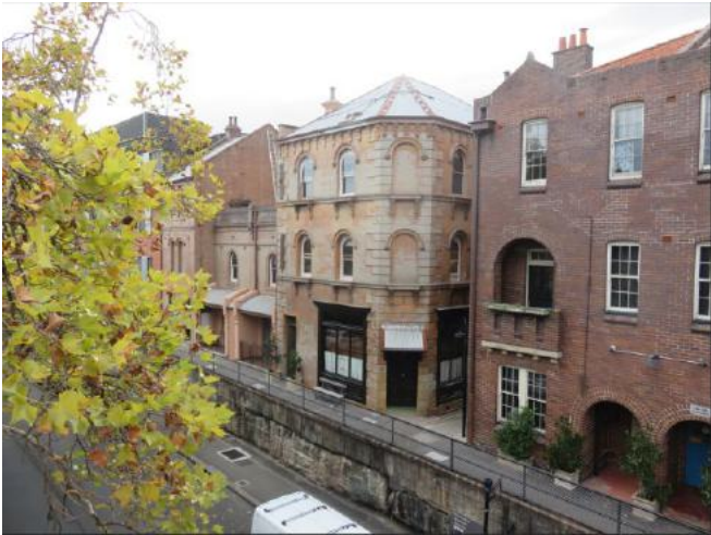
Figure 65: View 1, from the Cahill Expressway overpass
