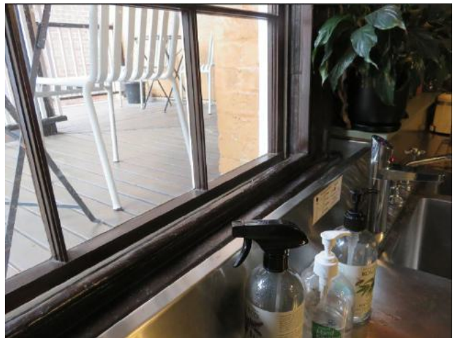
Figure 134: Detail of the careful detailing of the splashback of the contemporary bench unit and the windowsill.
