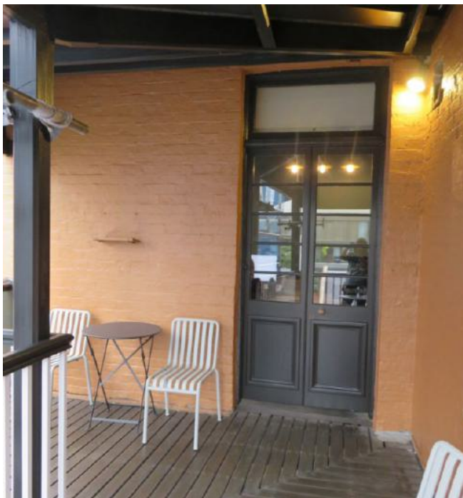
Figure 79: Level 2 east wall of the main part of the building with French doors opening onto the reconstructed veranda. The wall paint is in good condition on the upper floors.
