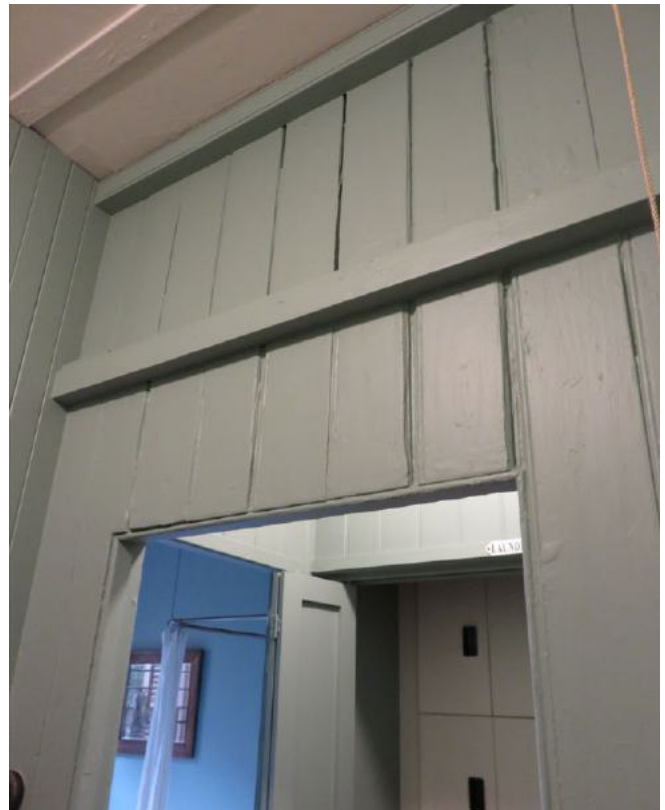
Figure 158: Detail of the wall that divides room 2.5 and extends to separate rooms 2.6 and 2.7. The fabric of this wall suggests it dates from the early to mid-20th century.
