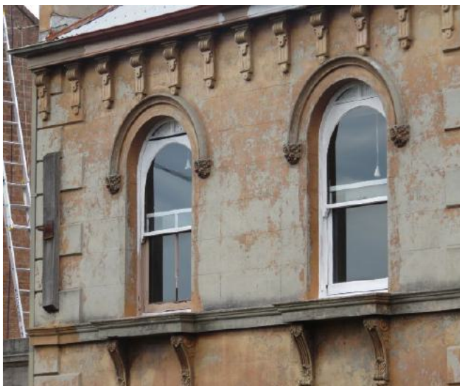
Figure 71: Second floor arched windows. The perforated panels above the top sash are typical of all of the building's double-hung windows. To the left of the windows is one of the timber structural bracings that exist on all elevations.
