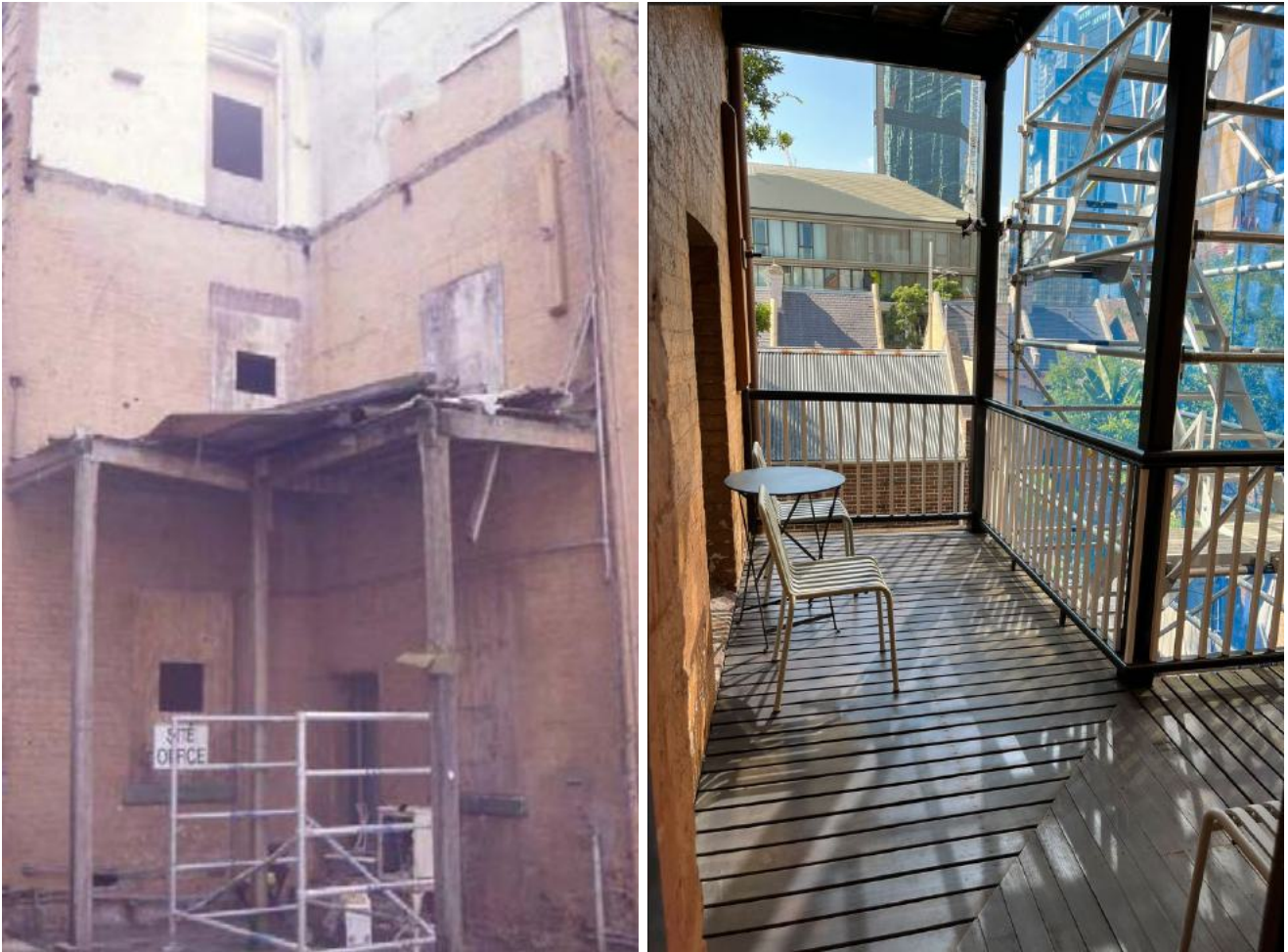
Figure 131: Remnants of rear verandah being demolished, 1996. (Source: PMNSW image 188808_CU_19-11, as reproduced in the 2015 CMP, p 124)
