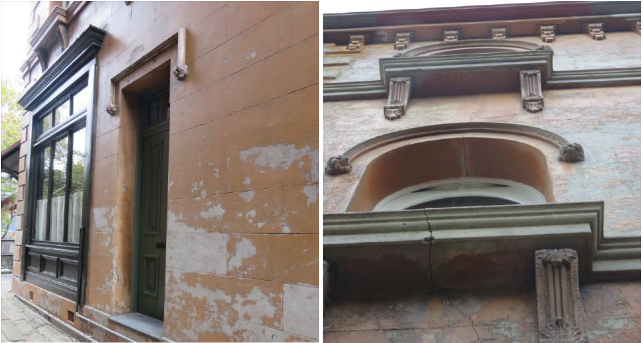
Figure 75: Detail of the Long's Lane (south) elevation showing the original shopfront and parlour door which is no longer operable.
