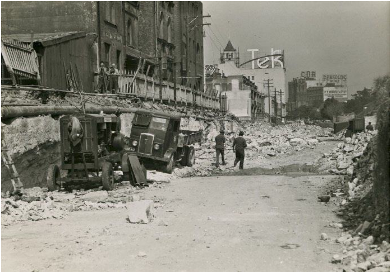
Figure 23: 1855 view of construction works for the Cahill Expressway south along Cumberland St to the Surviving Longs Lane Terraces in the upper left. Source: City of Sydney Archives
