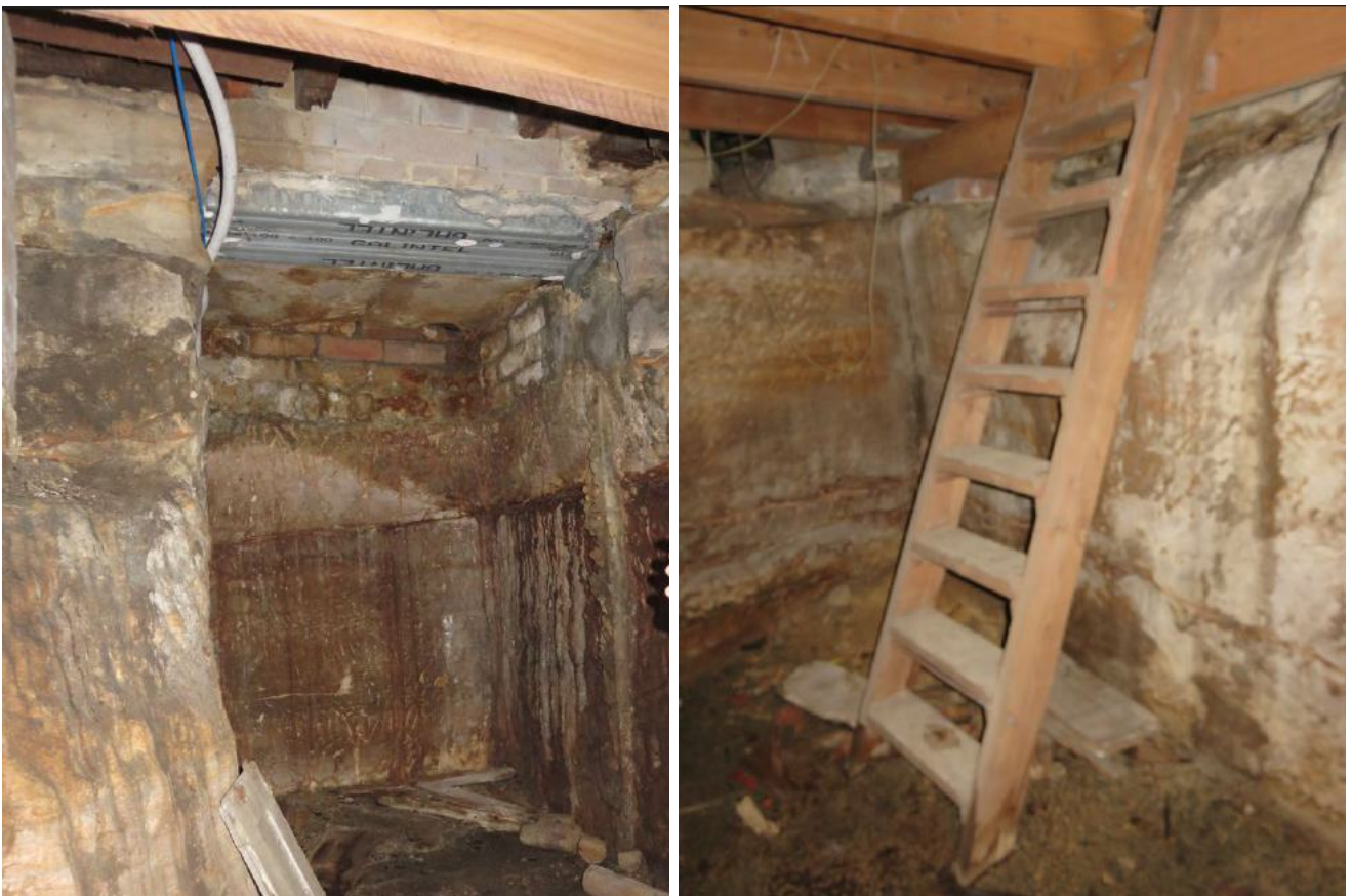
Figure 93: The delivery chute in the western wall.
