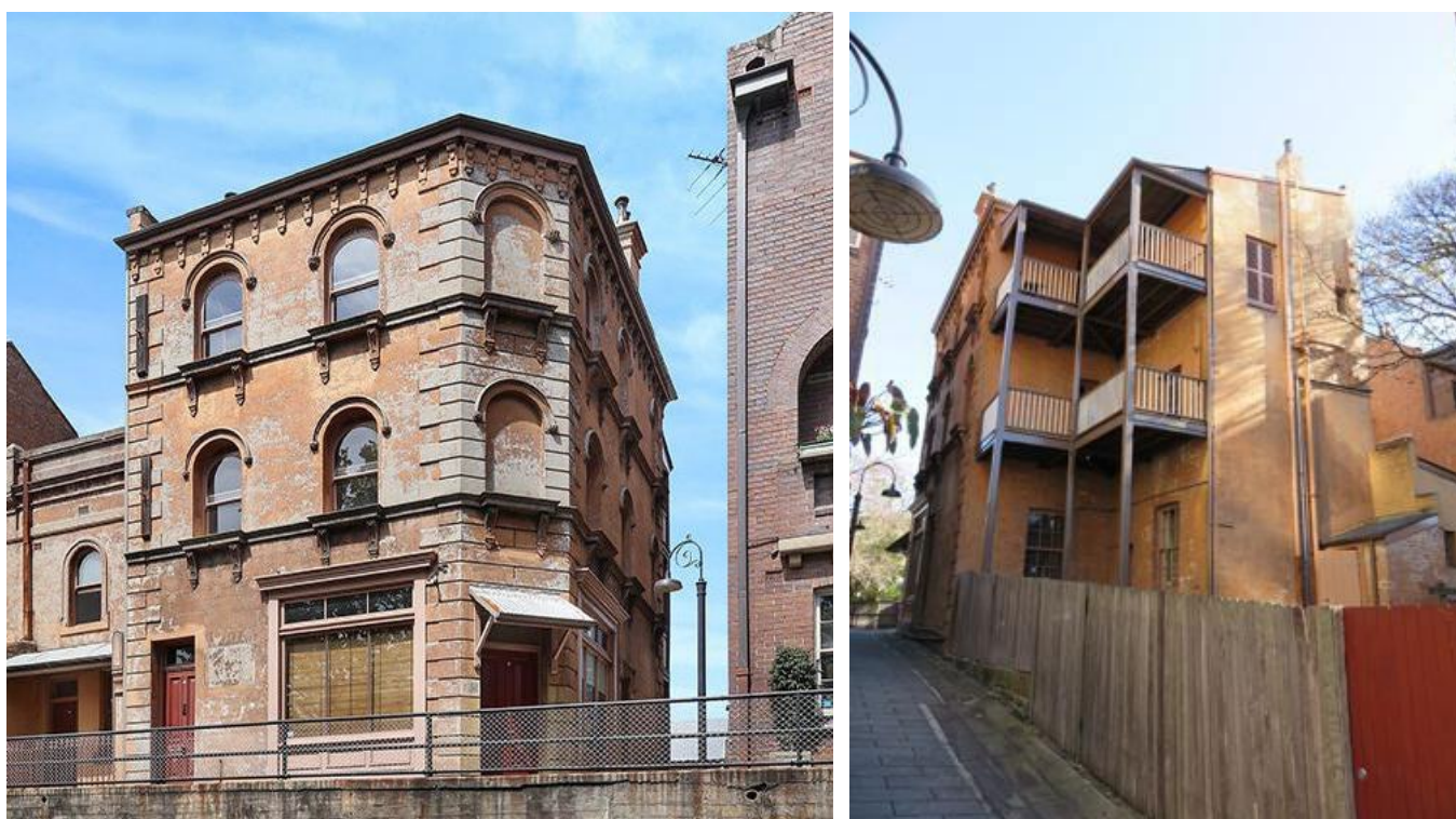
Figure 4 and Figure 5: 136-138 Cumberland Street, front and rear elevation, showing the subject property. Source: PMNSW
