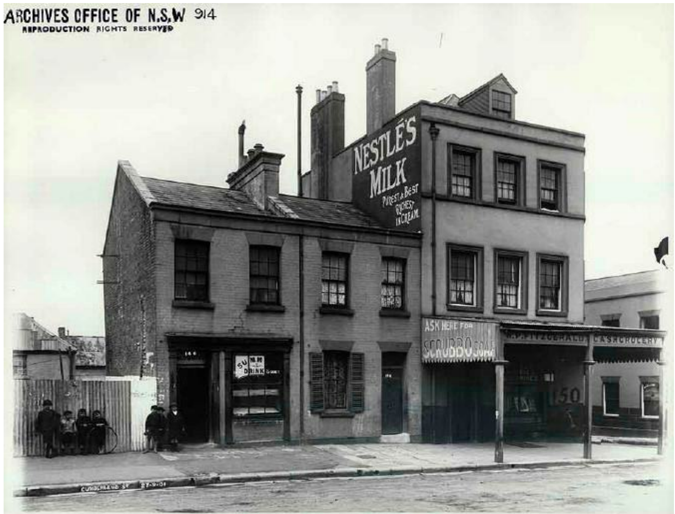
Figure 40: View of W. P. Fitzgerald's original three-storey Cash Grocery at No 150 Cumberland Street and Nos. 146-148 (two-storey) taken in September 1901 prior to his relocation to No. 136-138 Cumberland Street. Source: State Records series 4481 image
