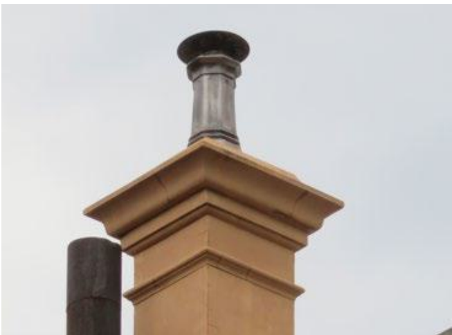
Figure 81: One of the two rendered chimneys with decorative mouldings and glazed ceramic chimney pot.
