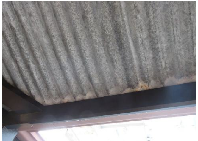
Figure 83: Detail of the main roof, showing the rust affected galvanized steel cappings. The ropes indicate that the roof harness system is in use.
