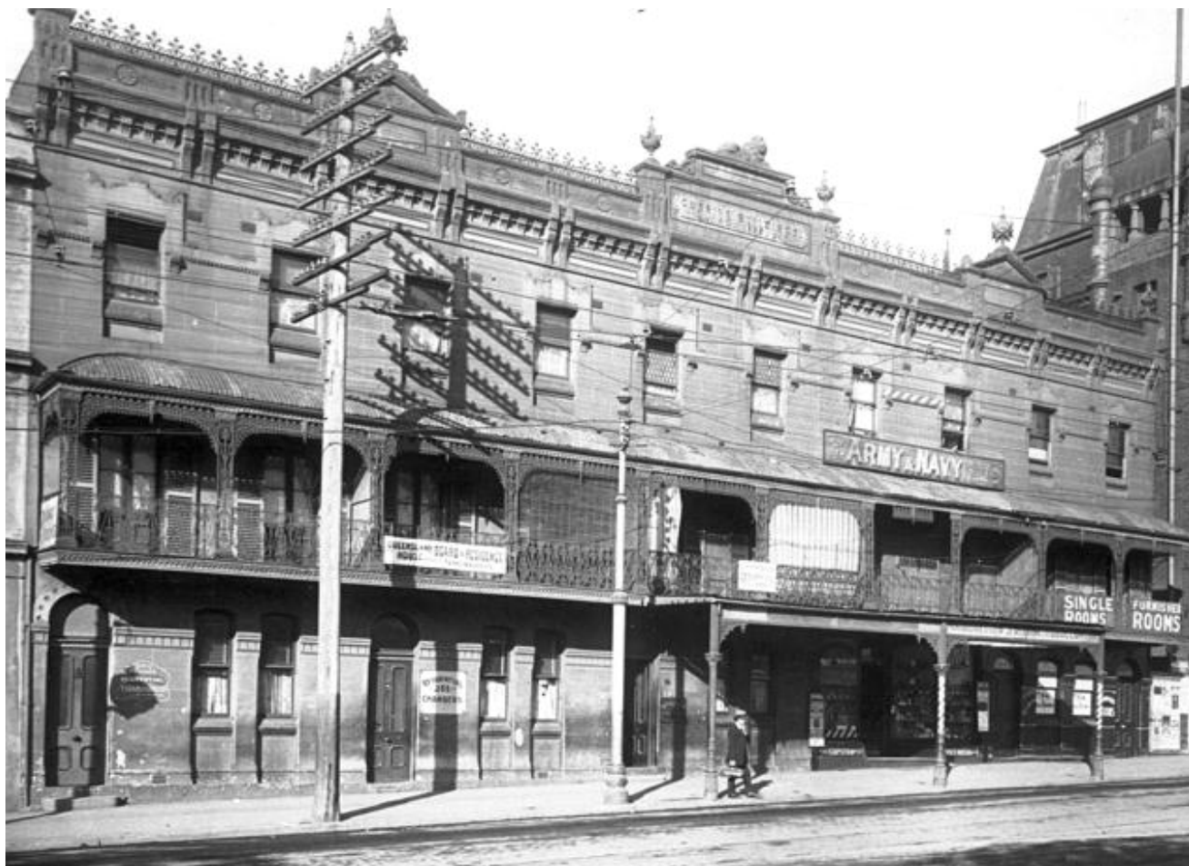
Figure 178: Guerin's Building, 286-292 Elizabeth Street part of which was occupied as a boarding house. Source: SCC Demolition books
