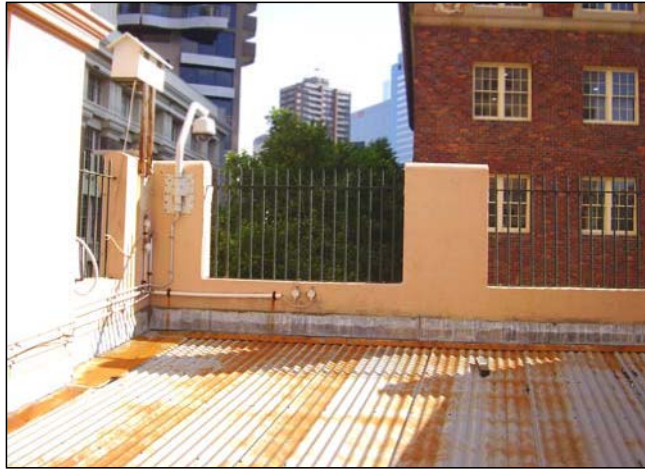
Figure 3.84 View of the south eastern roof and parapet.
