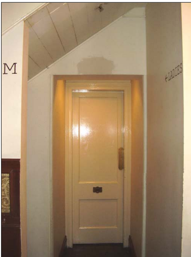
Figure 3.49 The stair soffit has been lined with timber boards and the alcove also accommodates an ATM. The rear yard of No. 10 was infilled and space amalgamated with the rear ground floor room to create service areas in the late 1980s and converted to the ladies' WC as part of the early 1990s works. Some patching is evident above the door.
