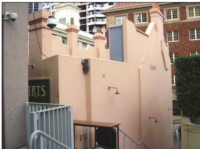
Figure 3.25 The western façade and roofline from the central open courtyard between the buildings and its immediate neighbours. The roof retains evidence of the former access to the roof of each of the buildings, however, only one (eastern end) stair and access actually remains intact.
