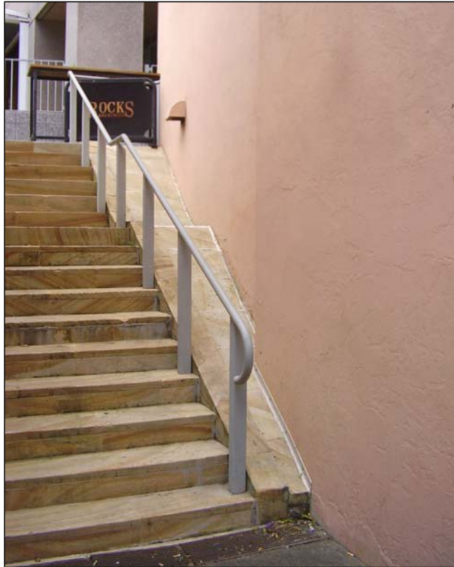
Figure 3.23 A modern stone stair and connection to the internal courtyards and Hotel complex extends along the western façade of the buildings.
