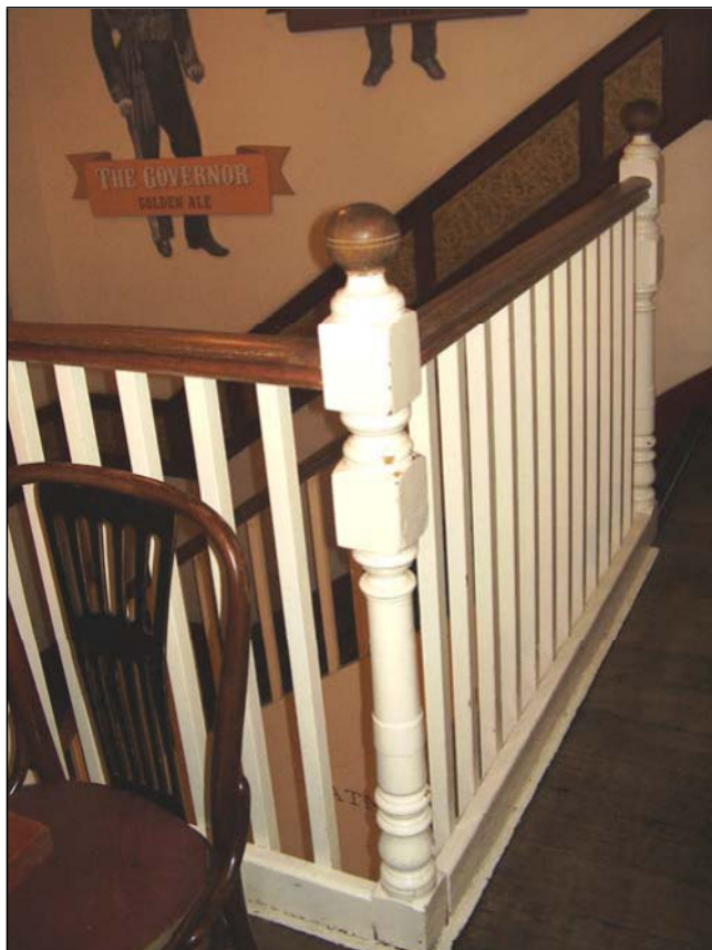
Figure 3.69 The timber balustrade which was added as part of the 1990s works. The stair balustrade has been detailed to match the remaining roof access stair in the north eastern corner of the first floor.
