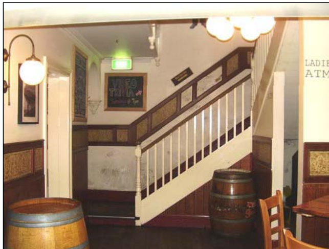
Figure 3.66 The stair located on the western end wall (No. 10) connecting the ground and first floor levels. Note the step and change of floor level at the base of the stair.
