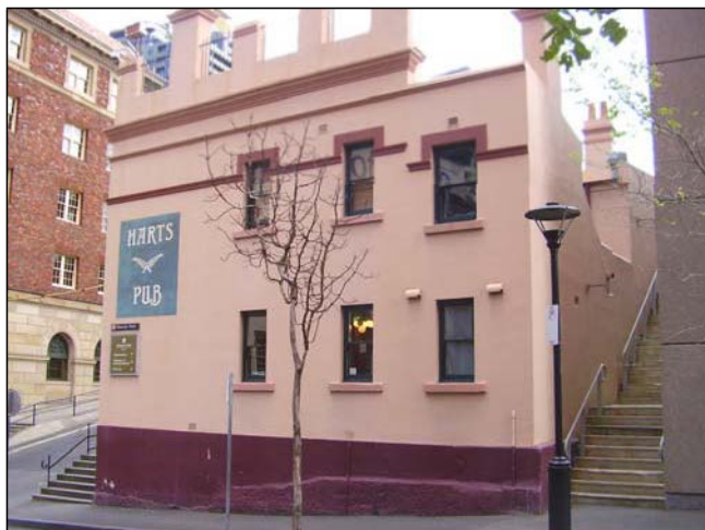
Figure 3.34 The north eastern and eastern facades of the buildings. The eastern end wall is constructed on natural stone base which has been painted.
