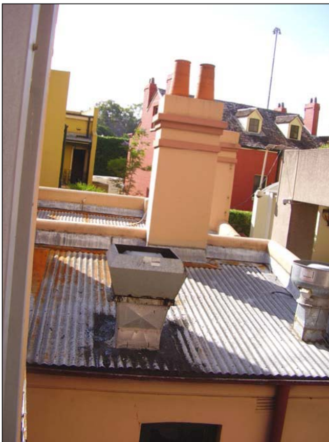
Figure 3.88 The roof over No. 10 and 12.
