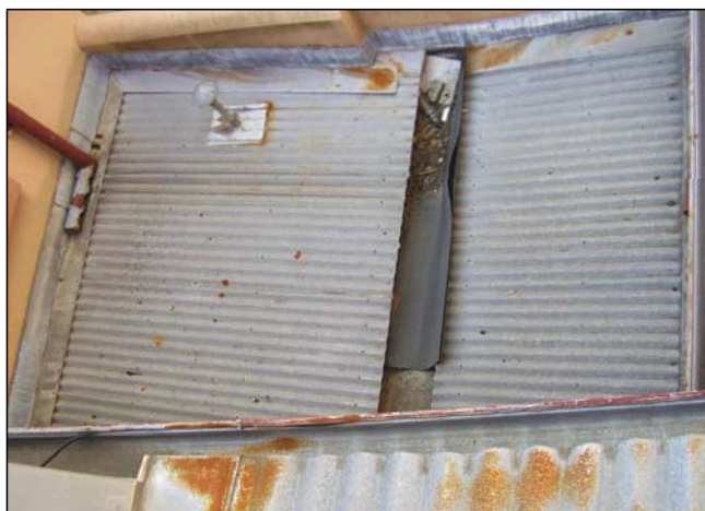
Figure 3.86 The roof over the north eastern section of the buildings (former rear wing and infilled yard of No. 14).
