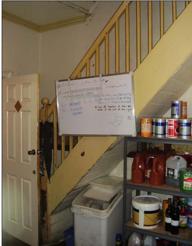
Figure 3.82 The room retains the one remaining stair to the roof.
