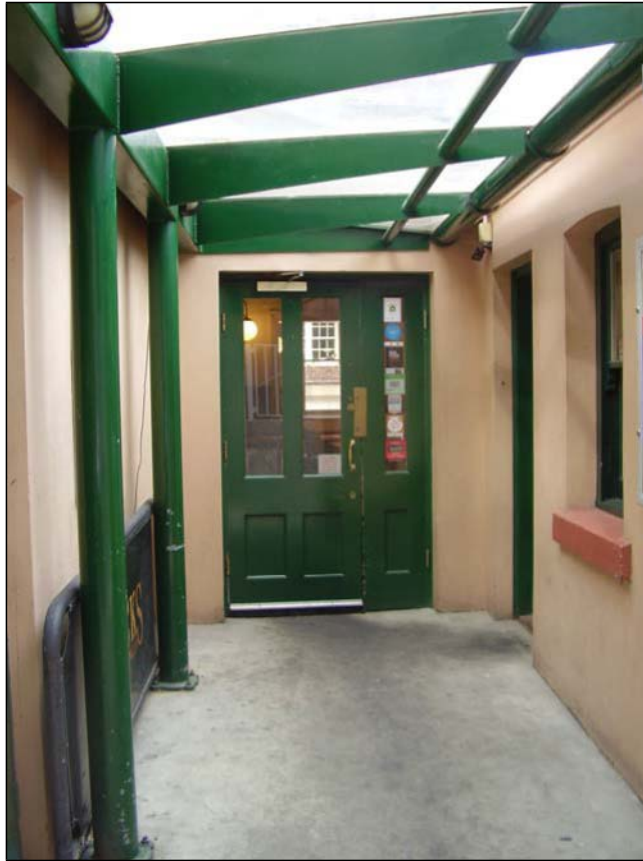
Figure 3.30 The access between the pub and courtyard. The doorways were created as part of the 1990s works. The former rear wing has an office (door at right) which is simply finished with skylight over.
