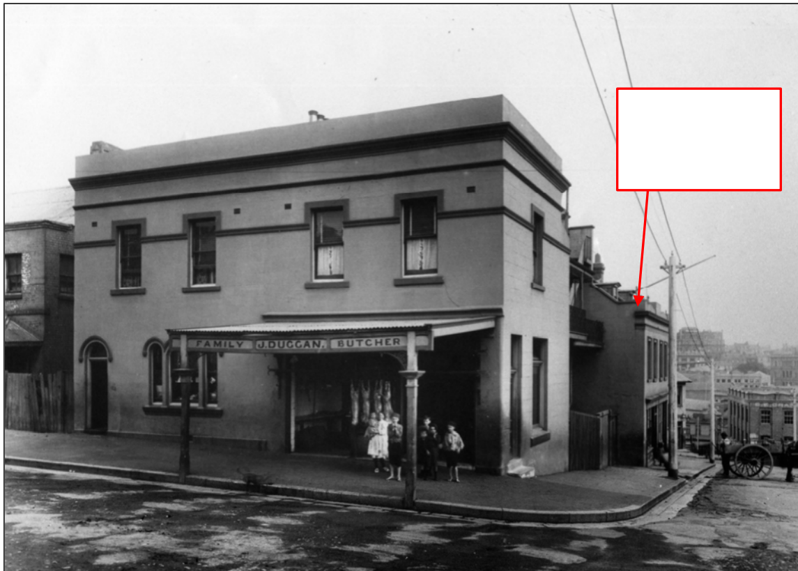
Figure 2.14 Photograph dating from around the turn of the century, looking east along Essex Street from Cumberland Street. Harts Buildings are not visible, however, the building demolished to make way for Gloucester Lane, Nos. 6-8 Essex Street is evident. (Source: Foreshore Authority Archives, 32688 CD 110)
