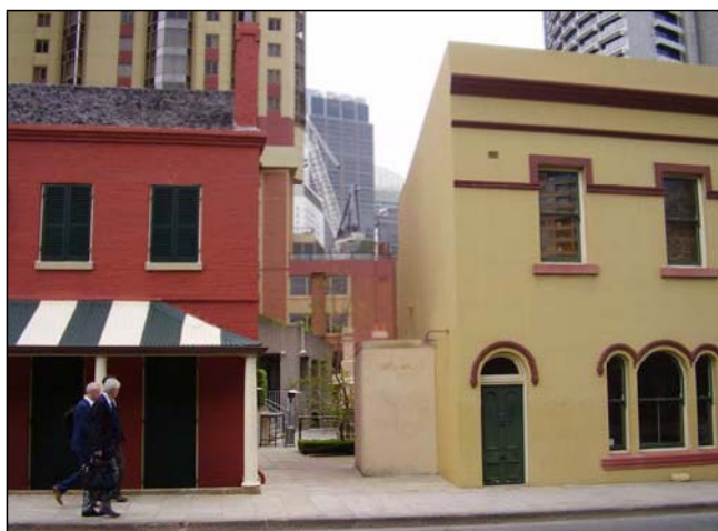
Figure 3.13 The Butchery Buildings also feature rendered wall planes with rendered string courses and moulded cornices to the front of the buildings which is constructed to the Cumberland and Essex Street alignment. An open public walkway separated the buildings from Lilyvale, No. 176 Cumberland Street.
