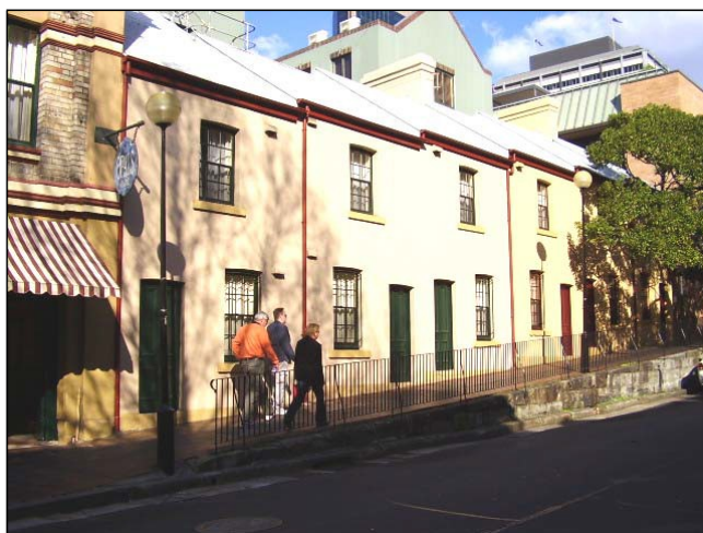
Figure 4.7 Nos. 42-52 Harrington Street, have similarly been constructed to follow the grade of the street.
