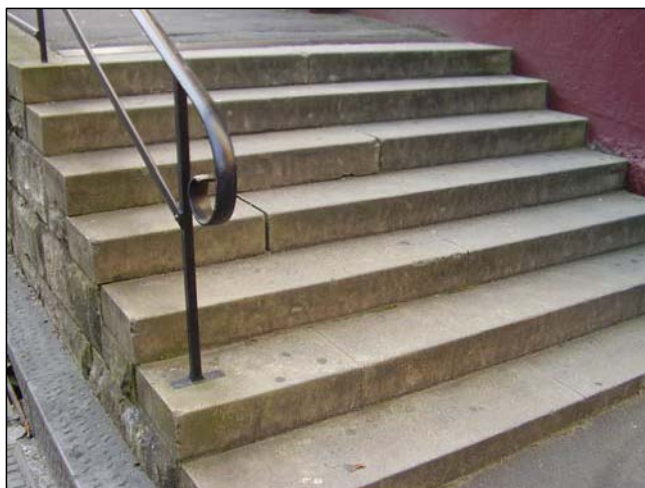
Figure 3.39 A sandstone stair is located in front of No. 14 Essex Street, near the corner of Gloucester Street. The street level and pedestrian footpath in front of the buildings were altered prior to 1988 and were formalised as part of the overall redevelopment of the precinct in the late 1980s, early 1990s. It is assumed that the stone treads date from the early 1990s works to the area.
