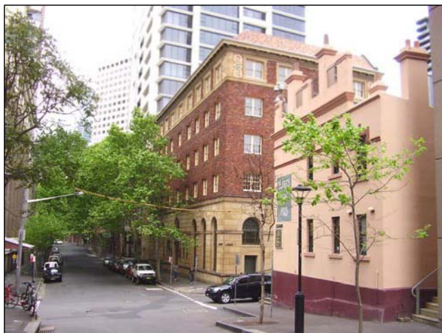
Figure 3.7 Science House, located opposite the subject buildings, is constructed in the Inter-war Commercial Palazzo style and features stone base and details and textured face brick façade with terracotta tile clad roof.
