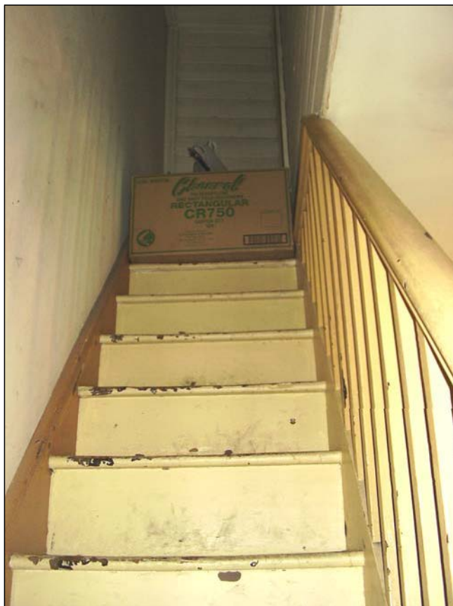
Figure 3.83 The stair is narrow with simple painted timber treads and risers and balustrade. The ceiling and soffit are lined with timber boards. A ledged and sheeted door is located on the upper landing.
