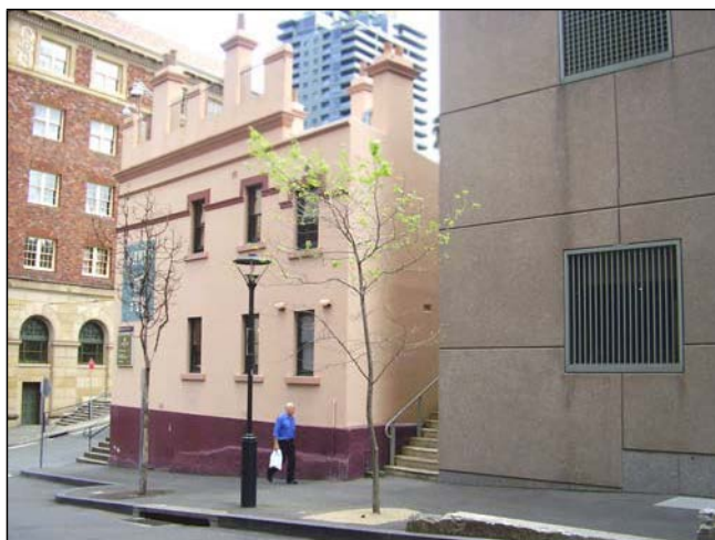
Figure 3.36 The eastern end wall is constructed directly to the Gloucester Street frontage.
