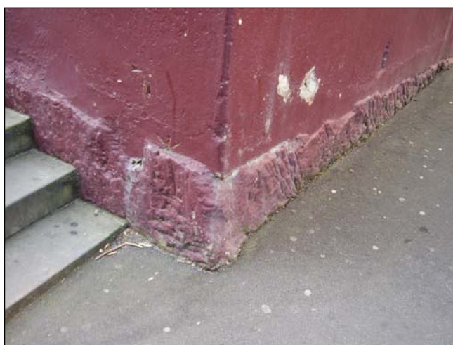
Figure 3.38 The base of the buildings on the corner of Essex and Gloucester Street has been constructed directly onto the rock ledges that gave the area its name.
