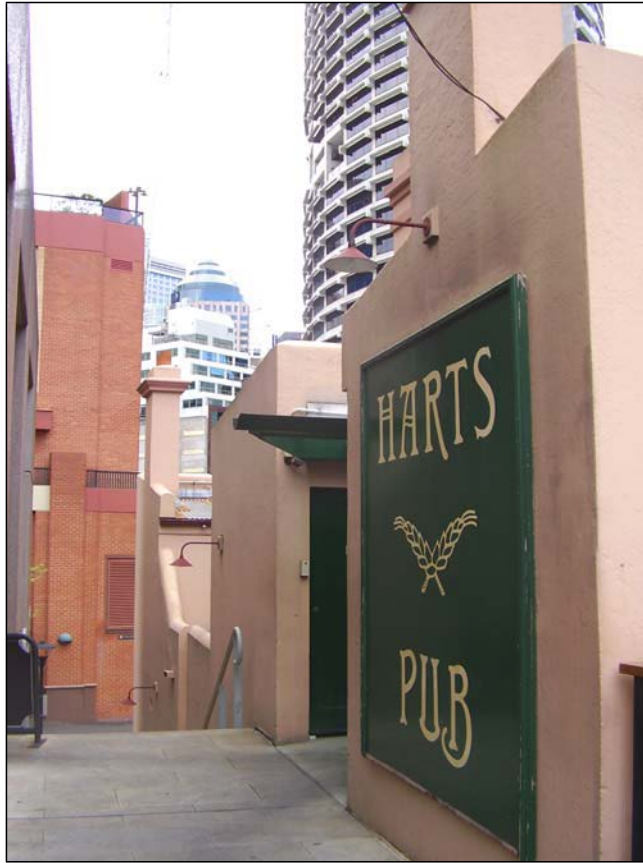
Figure 3.28 The rear facades of the buildings. A painted sign as been fixed to the western end wall. Lamps and services have also generally been added to the facades. It is assumed as part of the early 1990s works.
