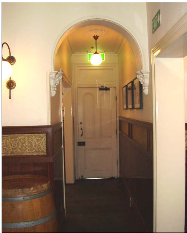
Figure 3.58 The entry of No. 12 which also retains the hall arch and a strong sense of the earlier layout of the buildings.
