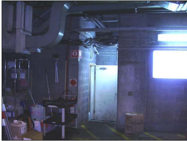
Figure 3.54 The shared basement service area and store under the hotel that is accessed by the Harts Buildings via the staircase at the rear of 12 Essex Street.
