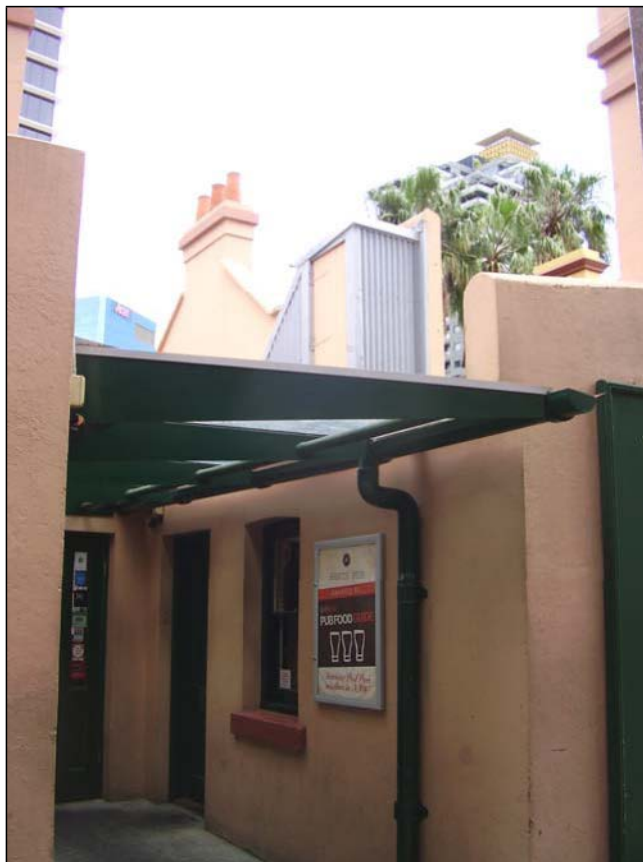
Figure 3.29 The access to the courtyard and pub now has a modern steel awning added as part of the 1990s works. The former rear yard (below) was covered over in c. 1988, however, the slab was added to create the access to the shared courtyard between 1990 and 1992. The rear upper room (at right) is only externally accessed and is used as an office.
