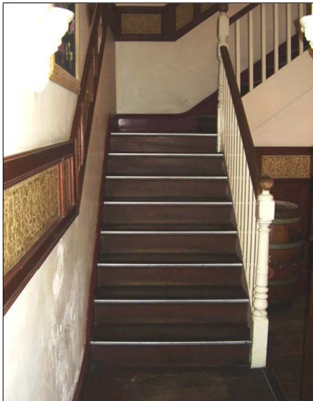
Figure 3.67 The stair was constructed as part of the 1990s works and has timber treads and risers and balustrade.
