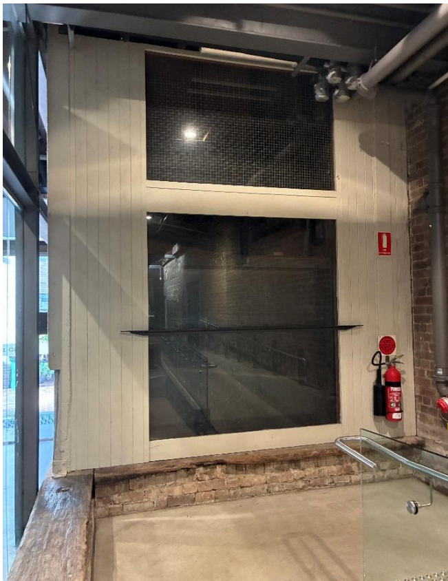
Figure 95: Modern glazed panel on the western side on the ground floor. (Source: PMNSW 2026)
