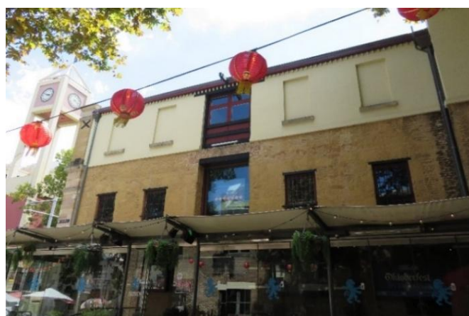
Figure 108: Argyle Stores—southern portion of east elevation, Playfair Street.
