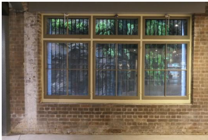
Figure 70: Original timber-framed windows along the western façade.
