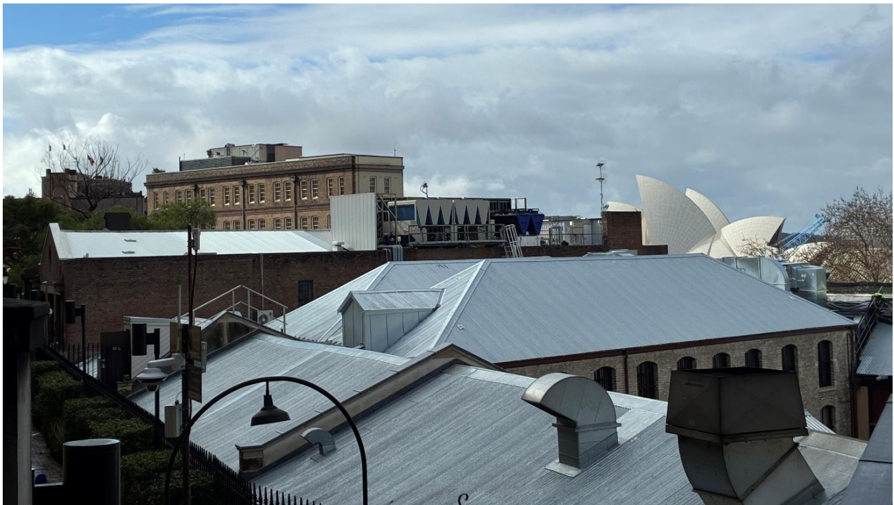
Figure 60: Roof of Cleland Bond Store (left) as viewed from Argyle Bridge, looking northeast. (Source: PMNSW 2026)
