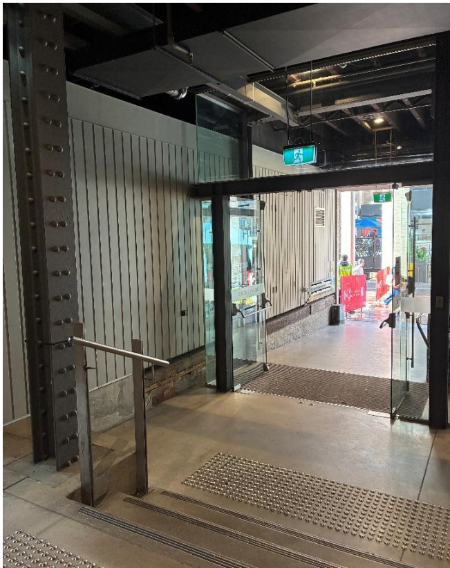
Figure 93: Looking northeast to the removed life north of the entrance off Playfair street. (Source: PMNSW 2026)
