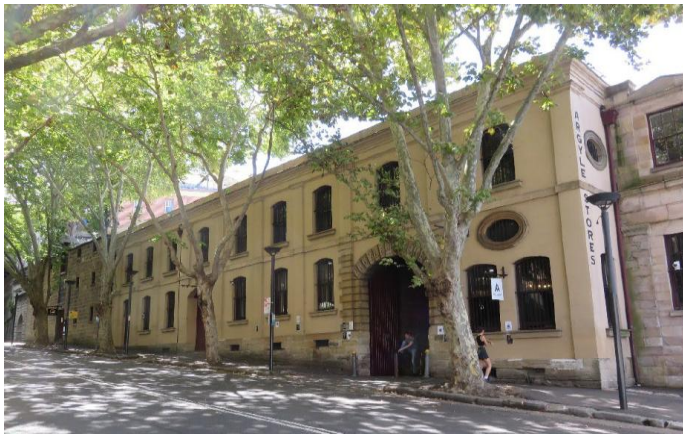
Figure 109: Western and central portions of the main south elevation of the Argyle Stores.
