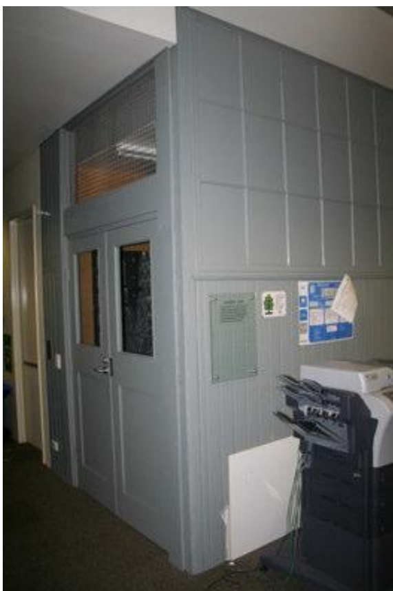
Figure 120: Timber panelled shaft of goods lift, Former Bushells Building. (Source: Tanner Architects, 2008).
