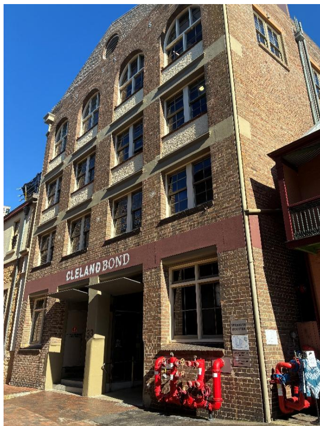
Figure 48: View 6 — northeast front façade corner, looking southwest from Playfair Street. (Source: PMNSW 2026)
