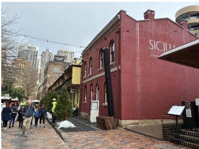
Figure 47: View 5 — looking southwest along Playfair Street with Cleland Bond Store visible over Playfair Street Terraces. (Source: PMNSW 2026)
