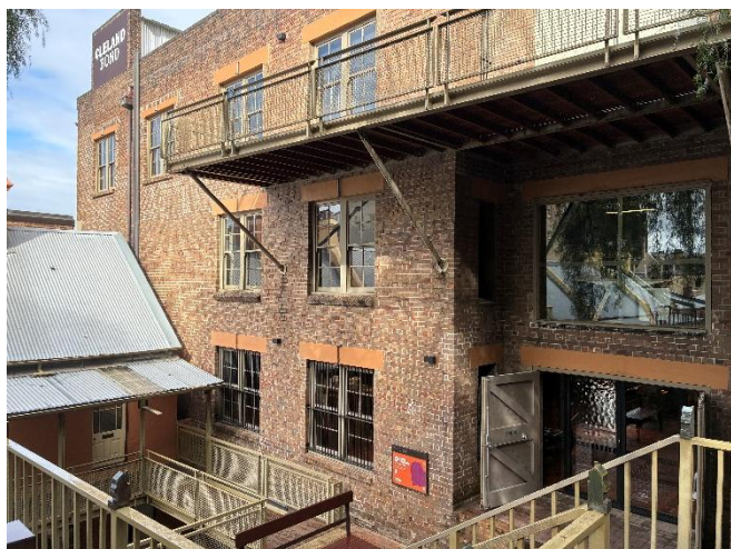
Figure 56: North elevation, looking southwest. (Source: PMNSW 2026)
