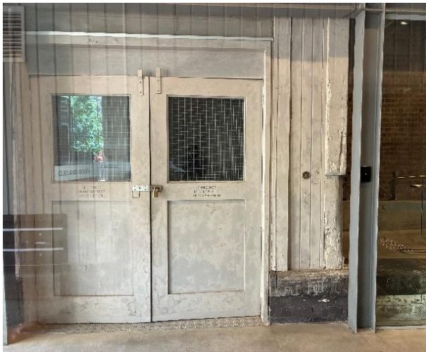
Figure 63: Original timber goods lift near the entryway, looking north. The timber clad shaft and lift car have been modified. (Source: PMNSW 2026)
