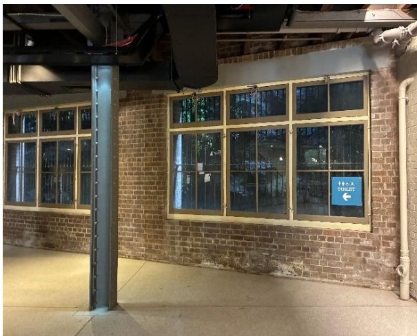
Figure 69: View to the western wall, looking southwest. (Source: PMNSW 2026)
