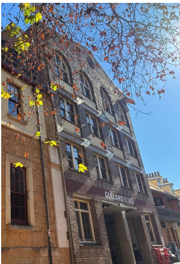
Figure 49: View 7 — oblique view of front façade looking northwest from Playfair Street. (Source: PMNSW 2026)
