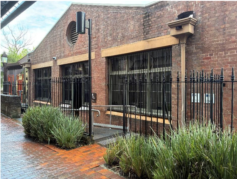
Figure 54: West elevation, rear facade on Gloucester Walk. (Source: PMNSW 2026)
