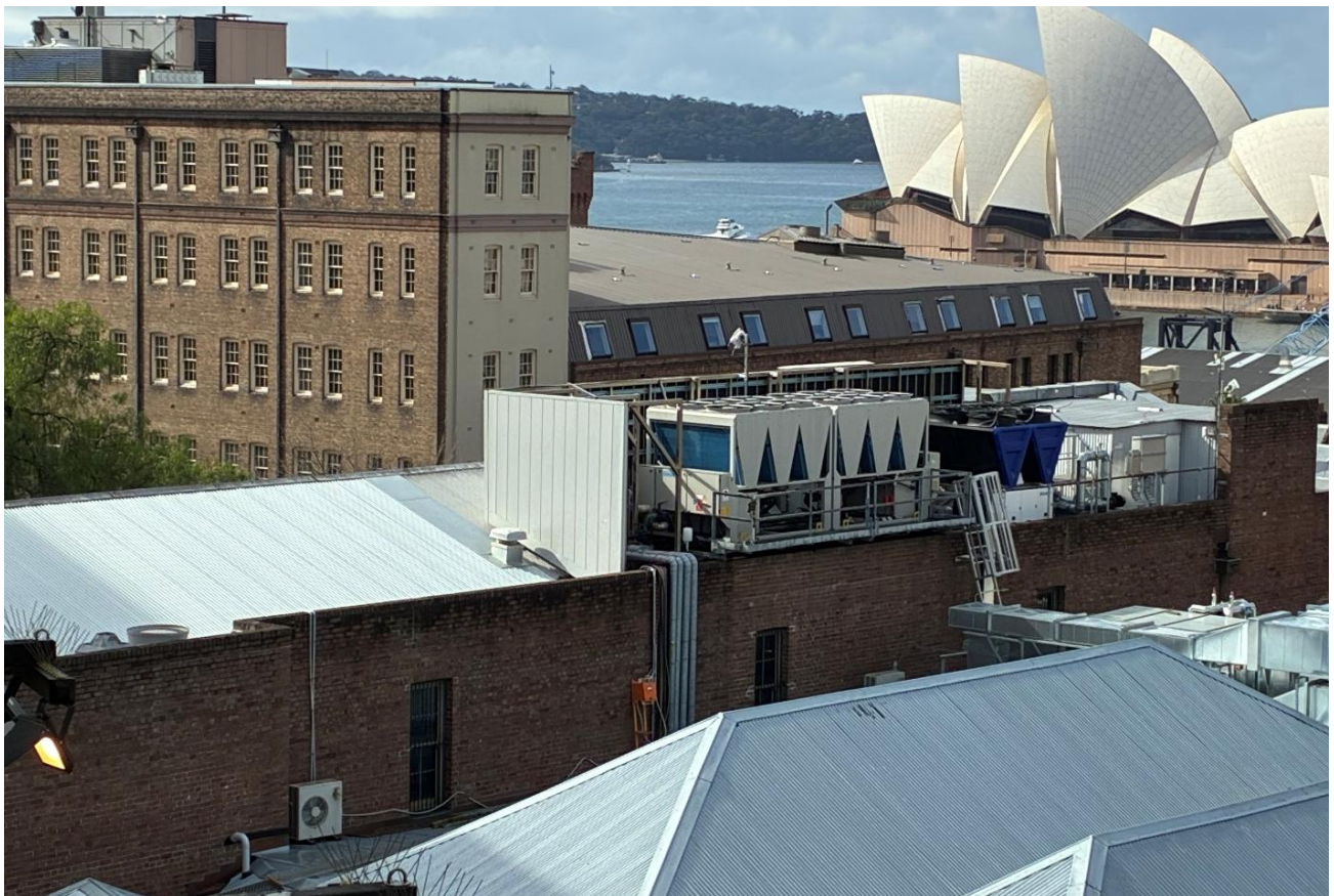
Figure 61: Roof of Cleland Bond Store (left) as viewed from Glenmore Hotel, looking northeast. (Source: PMNSW 2026)
