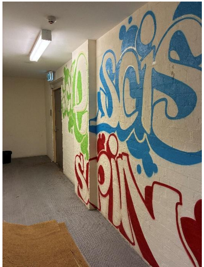
Figure 80: Level 2 — view of the isolated fire passage along the northern wall. Note graffiti. (Source: PMNSW 2026)
