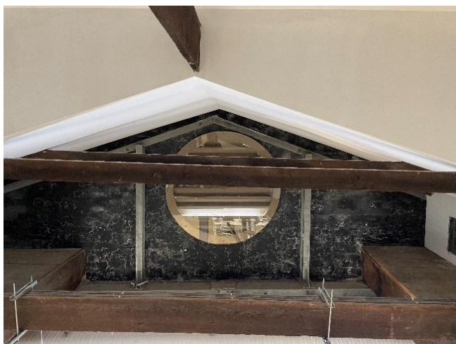
Figure 89: View of timber vent to the primary elevation, looking east.
