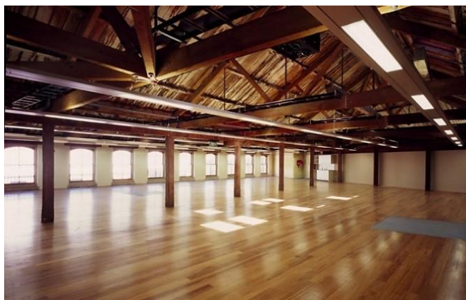
Figure 33: Level 3 of the north wing of the Argyle Stores following the 2005 refurbishment works. (Source: TKD Architects webpage, https://www.tkda.com.au/projects/argyle-and-cleland-bond-stores/ )
