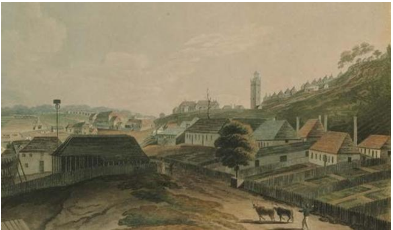
Figure 15: Extract from Edward Dayes' view of Sydney Cove showing the small buildings erected on the ridge above the hospital c.1802. Source: ML V1/1802/1
