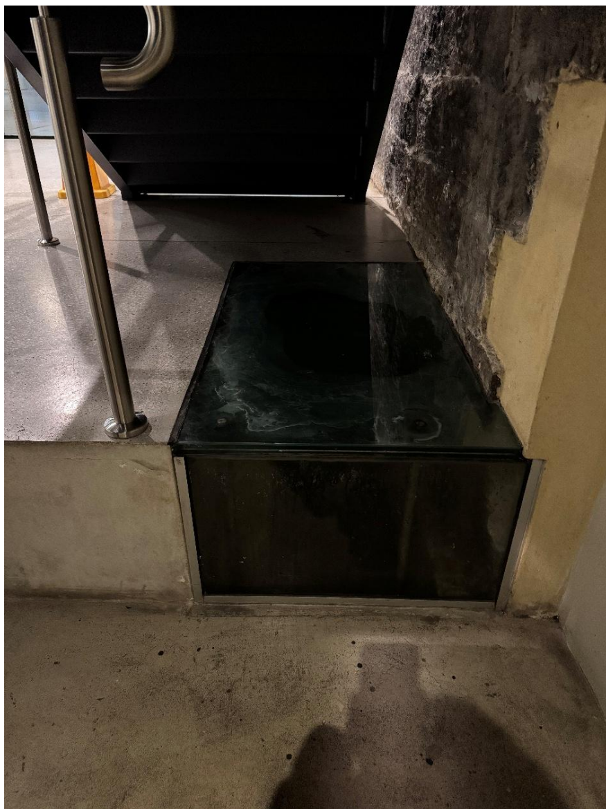
Figure 32: Glass-covered sandstone box drain below curved staircase, associated with part of the Argyle Stores erected by Unwin in c1828's Stores. (Source: PMNSW 2026)
