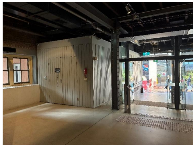
Figure 92: Looking northeast to the removed life north of the entrance off Playfair street. (Source: PMNSW 2026)
