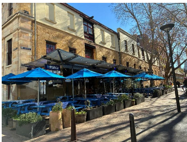
Figure 50: View 8 — looking north along Playfair Street. Argyle Stores is prominent on the corner and Cleland Bond Store is concealed behind the tree at the rear of the photo. (Source: PMNSW 2026)
