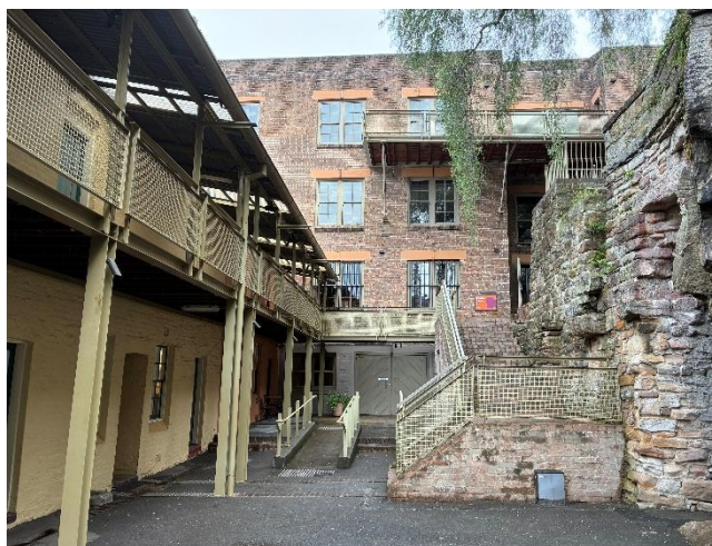
Figure 46: View 4 — looking south from ground level at the north façade of Cleland Bond Store. (Source: PMNSW 2026)
