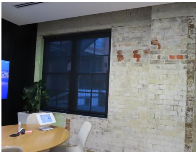
Figure 82: View of the southern brick wall.
