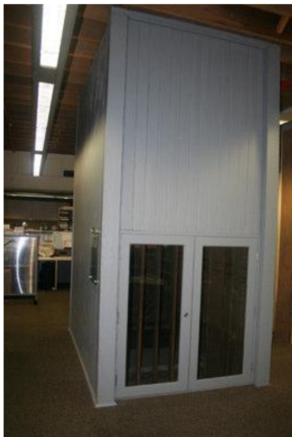
Figure 119: Wooden tea chest elevator, Former Bushells Building. (Source: Tanner Architects, 2008).
