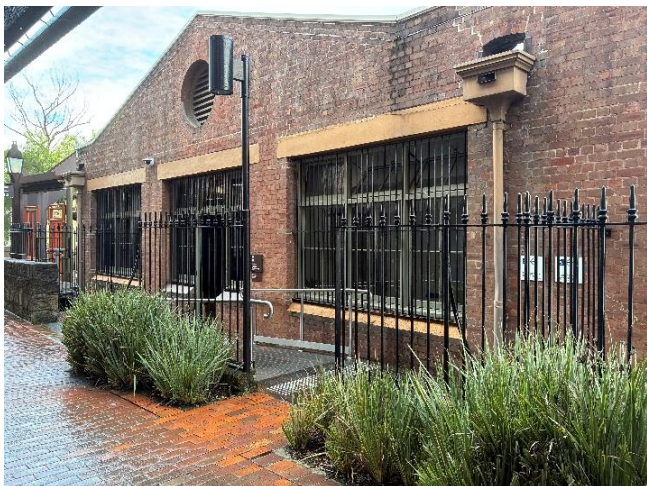
Figure 43: View 1 — looking northeast towards Cleland Bond Store from Gloucester Walk. (Source: PMNSW 2026)
