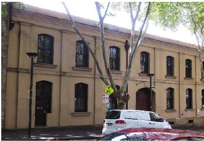
Figure 111: South wing — west end of south elevation
