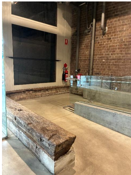
Figure 66: View of the low wall to the southeastern corner. (Source: PMNSW 2026)
