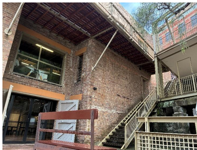
Figure 57: North elevation, looking southwest. (Source: PMNSW 2026)
