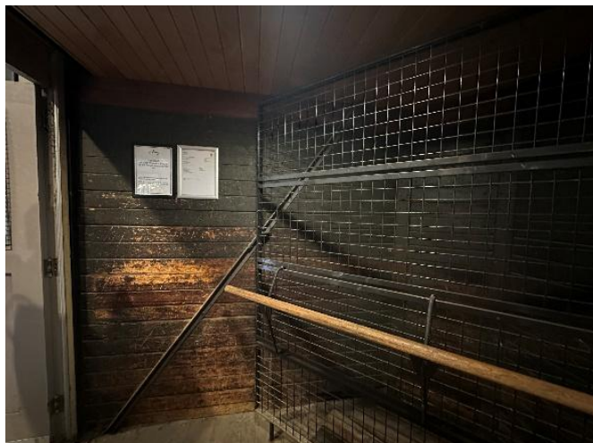
Figure 98: The original timber lift car with modern metal screen.
