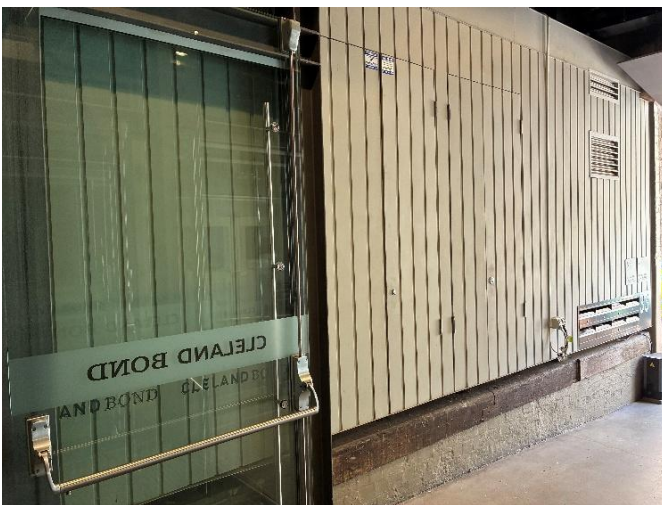
Figure 91: Looking northeast to removed lift to the north of the entrance off Playfair street. (Source: PMNSW 2026)
