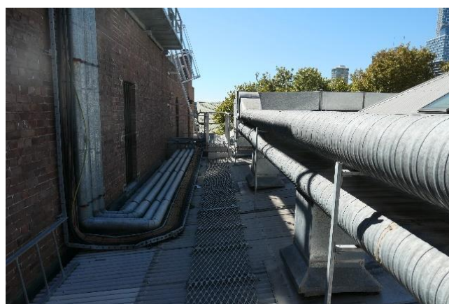
Figure 59: South elevation, looking northeast. The shared brick wall is visible in the background, and the Argyle Stores metal roof is visible in the foreground.
