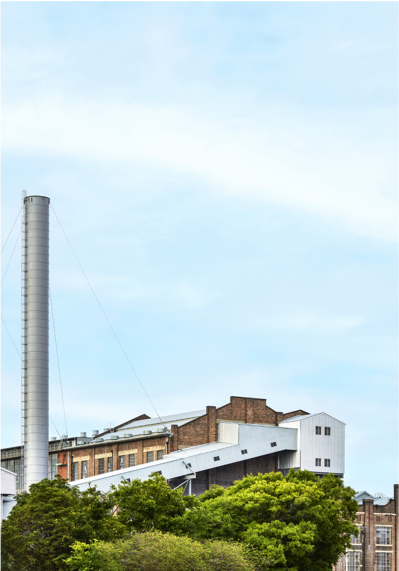
Figure 3.2.4 View of the White Bay Power Station north elevation over the canopy, 2024 (courtesy of Toby Peet).
