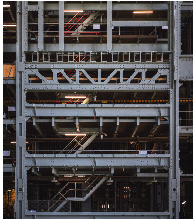
Figure 6.6.18 No. 1 Boiler and walkways, 2023 (courtesy of Toby Peet).
