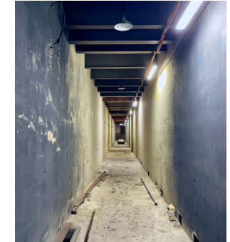
Figure 4.2.8 Switch House Level 1-North, 2023 (courtesy of Chris Bennett: Evolving Picture).
