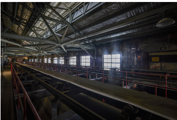
Figure 6.6.22 The Conveyor Level of the Boiler House, 2023 (courtesy of Toby Peet).
