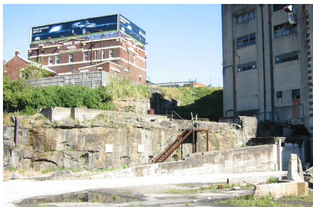
Figure 2.7.92 White Bay Hotel from South Yard, Administration and Staff Accommodation on right, 2002 (Design 5 – Architects)
