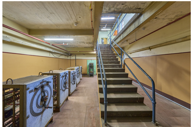
Figure 4.2.42 The Rheostat Room in the Control Room Building, 2024 (courtesy of Chris Bennett: Evolving Picture).
