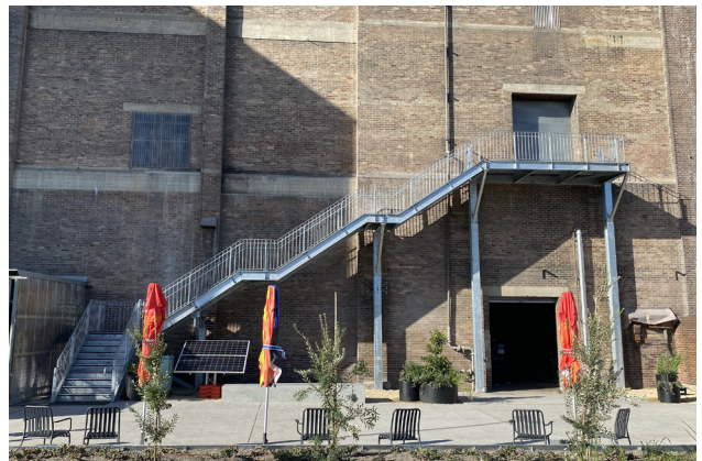
Figure 6.10.2 New stairs constructed on the north end of the Boiler House as part of the 2022-24 works, 2024 (Design 5 – Architects).
