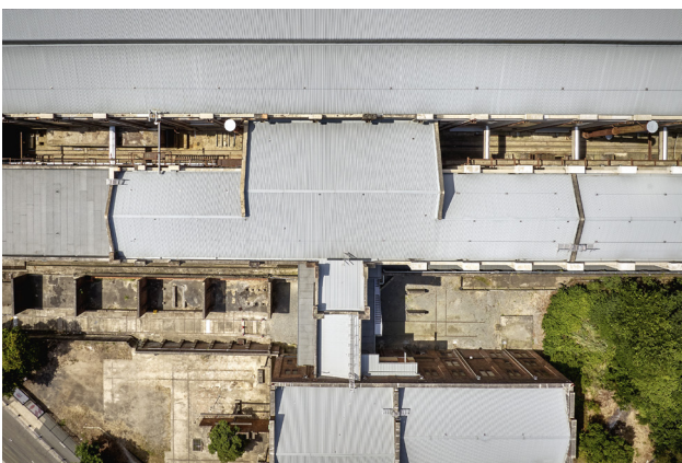
Figure 6.10.4 Corrugated steel roofs that were replaced as part of the 2022–24 remediation works, 2024 (courtesy of Toby Peet).
