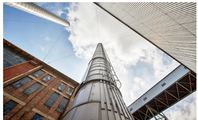
Figure 6.6.16 Chimney Stacks located between the Coal Handling Shed and Boiler House, 2024 (courtesy of Toby Peet).
