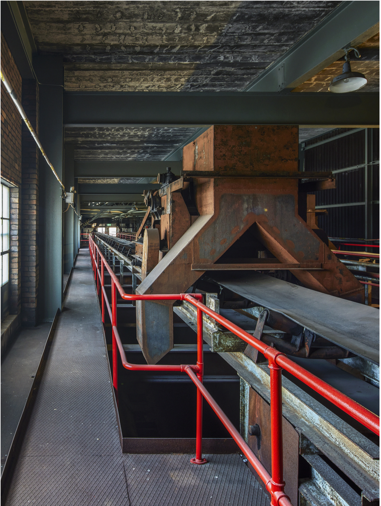
Figure 4.2.49 Conveyor Level in the Boiler House, 2023 (courtesy of Toby Peet).
