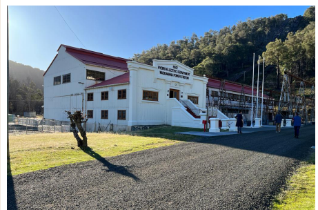
Figure 2.8.9 Waddamana Power Station ‘A’, 2023 (Alan Croker, Design 5 – Architects).
