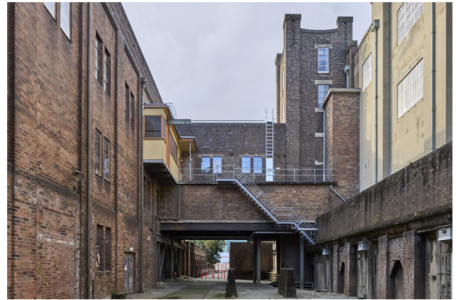
Figure 5.10.4 The link building between the Switch House and the Control Room Building, 2024 (courtesy of Chris Bennett: Evolving Picture).
