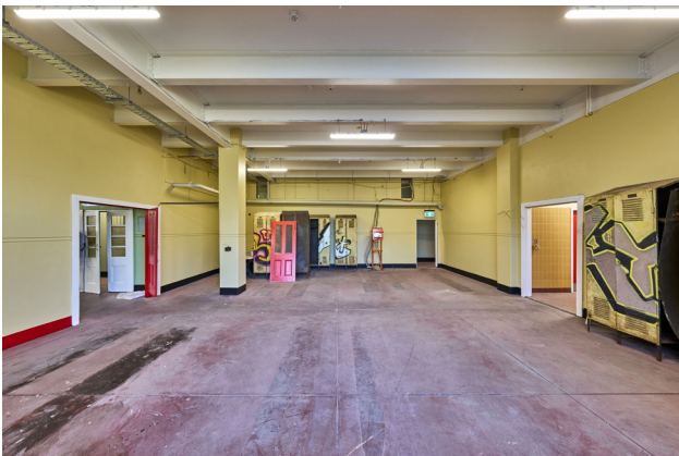
Figure 6.6.36 Level 2 Locker Room with extant lockers, 2024 (courtesy of Chris Bennett: Evolving Picture).
