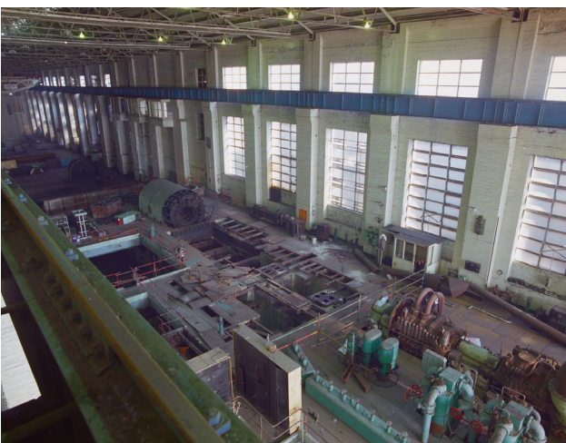
Figure 2.7.57 The Turbine Hall during the decommissioning of the power station, c. 1990s (courtesy of the ECNSW Archives, CN7.0021-J).
