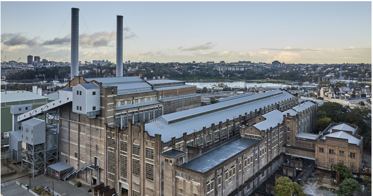
Figure 1.5.2 Aerial view of White Bay Power Station, 2024 (courtesy of Chris Bennett: Evolving Picture)
