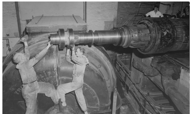
Figure 2.770 White Bay Power Station workers assembling the second turbo-alternator rotor, 1956 (courtesy of the ECNSW Archives, 00979D).
