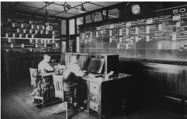
Figure 2.7.36 White Bay Power Station Trouble Room, 1930 (courtesy of the NSW State Rail Authority records, State Archives Collection, 26180, 235/41, 363/39).
