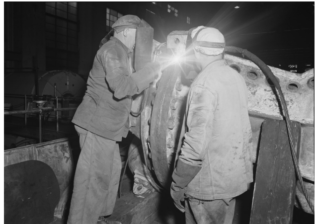
Figure 3.5.9 Workers welding a crack in a turbine cover, 1958 (courtesy of the State Archives of NSW, NRS-20347-1-001774_A).
