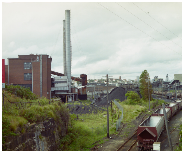
Figure 2.7.55 White Bay Power Station in 1986 (courtesy of NSW State Archives, NRS-20347-1_cn70012_Q).
