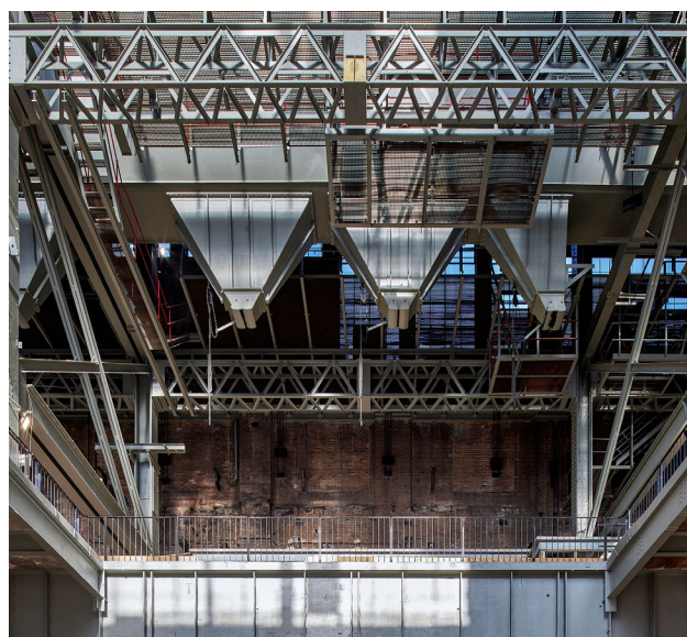
Figure 3.6.1 Boiler House hopper chutes, 2024 (courtesy of Toby Peet)
