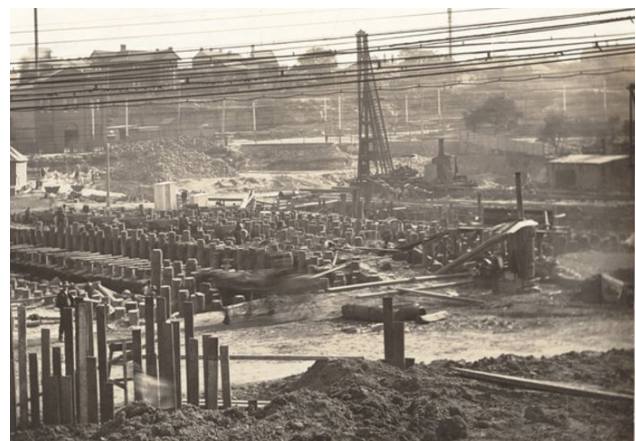
Figure 2.7.20 Boiler Room piling during construction at White Bay, 1912 (courtesy of NSW State Archives, NRS-17420-2-4-363/003).
