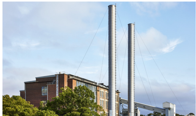
Figure 3.2.23 Chimney Stacks, 2024 (courtesy of Toby Peet).
