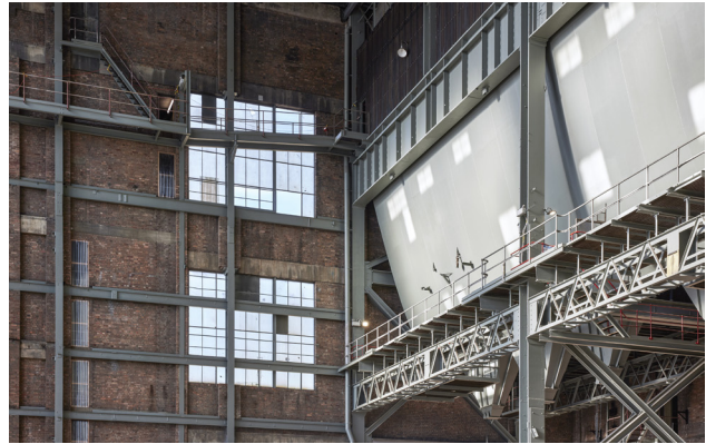
Figure 6.16.4 Painted structure and machinery of the Boiler House, 2024 (courtesy of Toby Peet).
