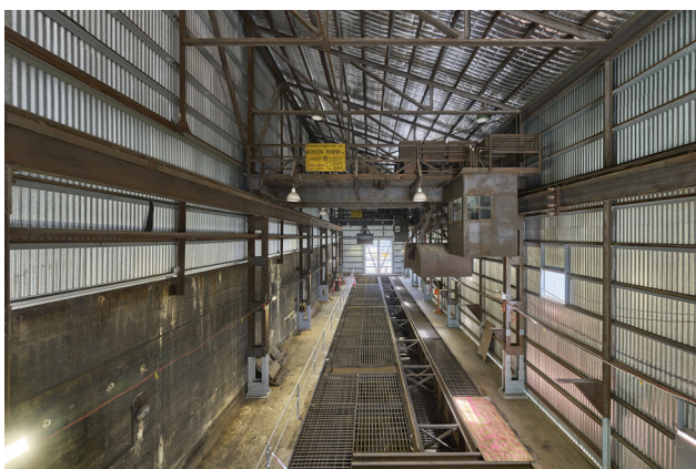
Figure 2.2.29 Coal Handling Shed with view of the Capstan, the Two Cranes and Grabs, the Screens, and the Hoppers and Pneumatic Feed Gates underneath, 2023 (courtesy of Chris Bennett: Evolving Picture).
