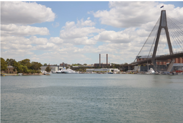
Figure 6.5.2 View of the power station across Blackwattle Bay, 2015.
