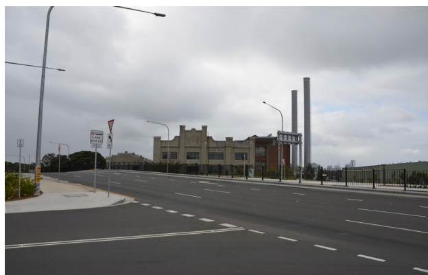
Figure 3.2.18 Southern Elevation, viewed from Victoria Road, July 2024 (Design 5 – Architects).
