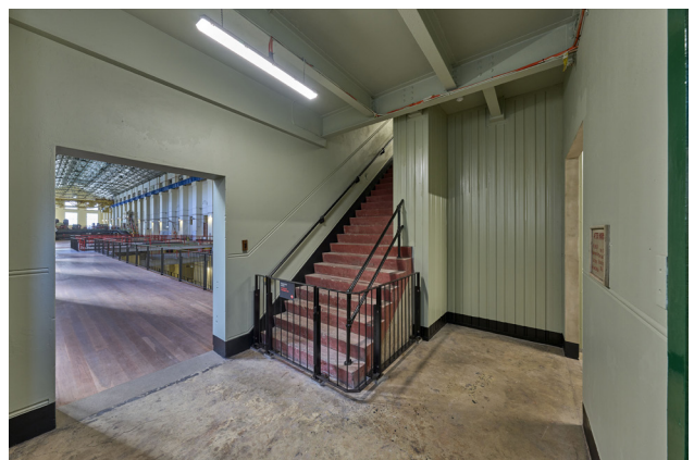
Figure 6.10.7 Administration and Staff Accommodation with new walkway from Turbine Hall and gate, 2024 (courtesy of Chris Bennett: Evolving Picture).
