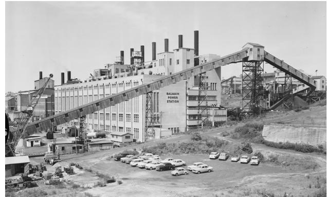
Figure 2.7.18 Balmain Power Station, 1964 (courtesy of NSW State Records, NRS-20347-1-44-4755).
