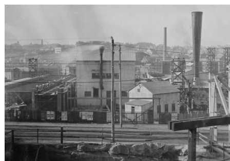
Figure 2.7.97 White Bay Power Station during Turbine Hall construction, 1913 (courtesy of Powerhouse Museum Archive).
