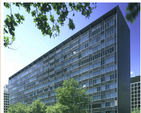
Figure 2.8.43 MLC Building west facade (courtesy of Bates Smart).140
