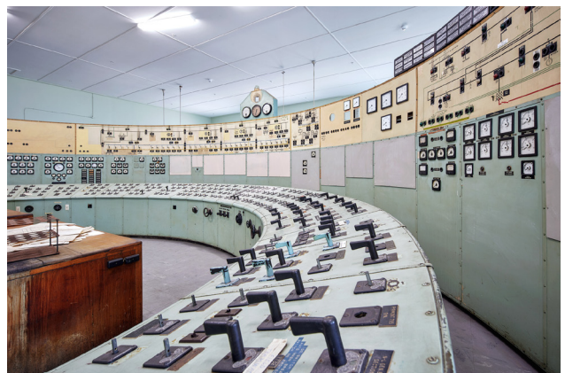
Figure 4.2.44 The 1948 Control Room, 2024 (courtesy of Toby Peet).
