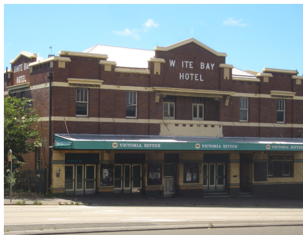
Figure 2.7.95 White Bay Hotel front view, 26 January 2008 (courtesy of J Bar, available through Wikimedia Commons, file: White Bay Hotel.jpg).
