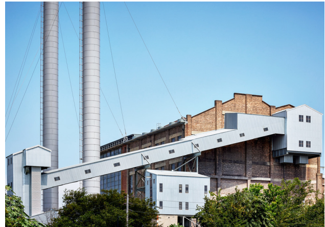
Figure 2.2.1 North elevation of White Bay Power Station, March 2024 (courtesy of Toby Peet).
