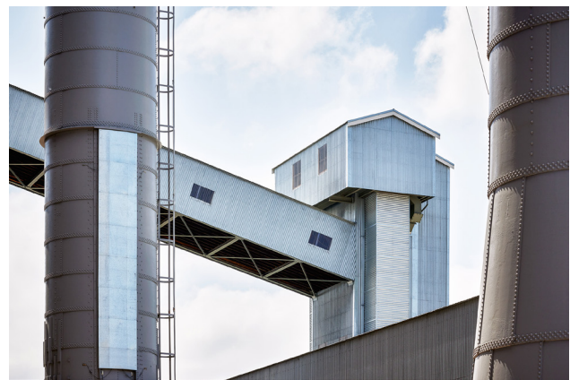
Figure 6.6.13 The tower of the Coal Handling Shed, the External Conveyor, and the Chimney Stacks, 2024 (courtesy of Toby Peet).
