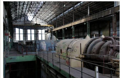
Figure 2.8.17 East Perth Power Station Turbine Hall, 2020 (courtesy of ABC News: Jacob Kagi). 115
