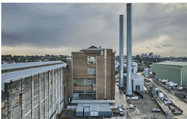
Figure 3.2.16 Southeastern Elevation, July 2024 (courtesy of Chris Bennett: Evolving Picture).
