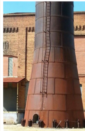
Figure 2.8.40 Base of stack at former steam plant (courtesy of Gabe Janke).
