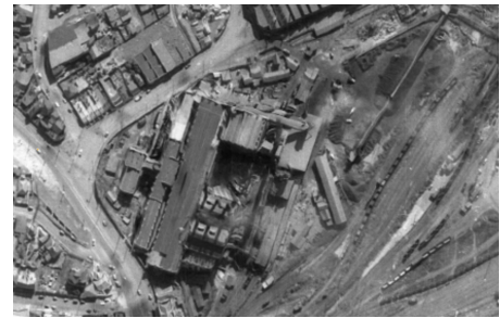
Figure 2.7.105 Aerial View showing construction of the No. 3 Boiler House, 1955 (courtesy of NSW Historical Imagery).
