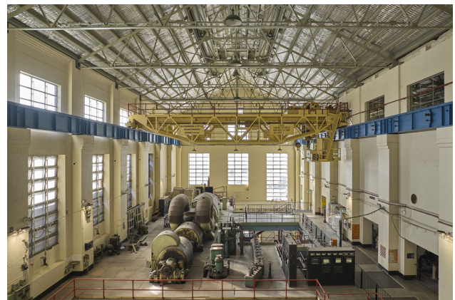
Figure 2.2.17 Turbine Hall South end at Level 2, looking north, 2024 (courtesy of Chris Bennett: Evolving Picture).
