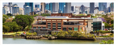
Figure 2.8.7 Brisbane Powerhouse (courtesy of Brisbane City Council).109
