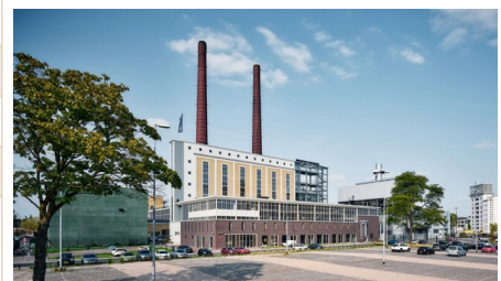
Figure 2.8.28 Innovation Power Station (courtesy of Tycho Merjin).125
