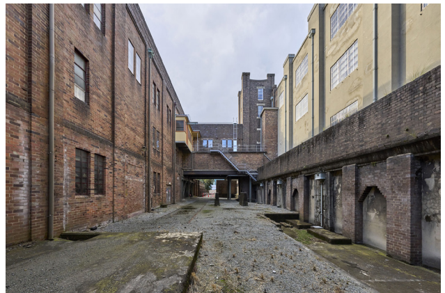
Figure 6.5.27 View looking north from the South West Yard towards the Control Room Bridge, 2024 (courtesy of Chris Bennett: Evolving Picture).
