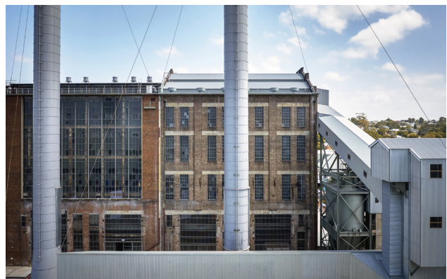
Figure 3.2.24 Boiler House Exterior east facade, March 2024 (courtesy of Toby Peet).
