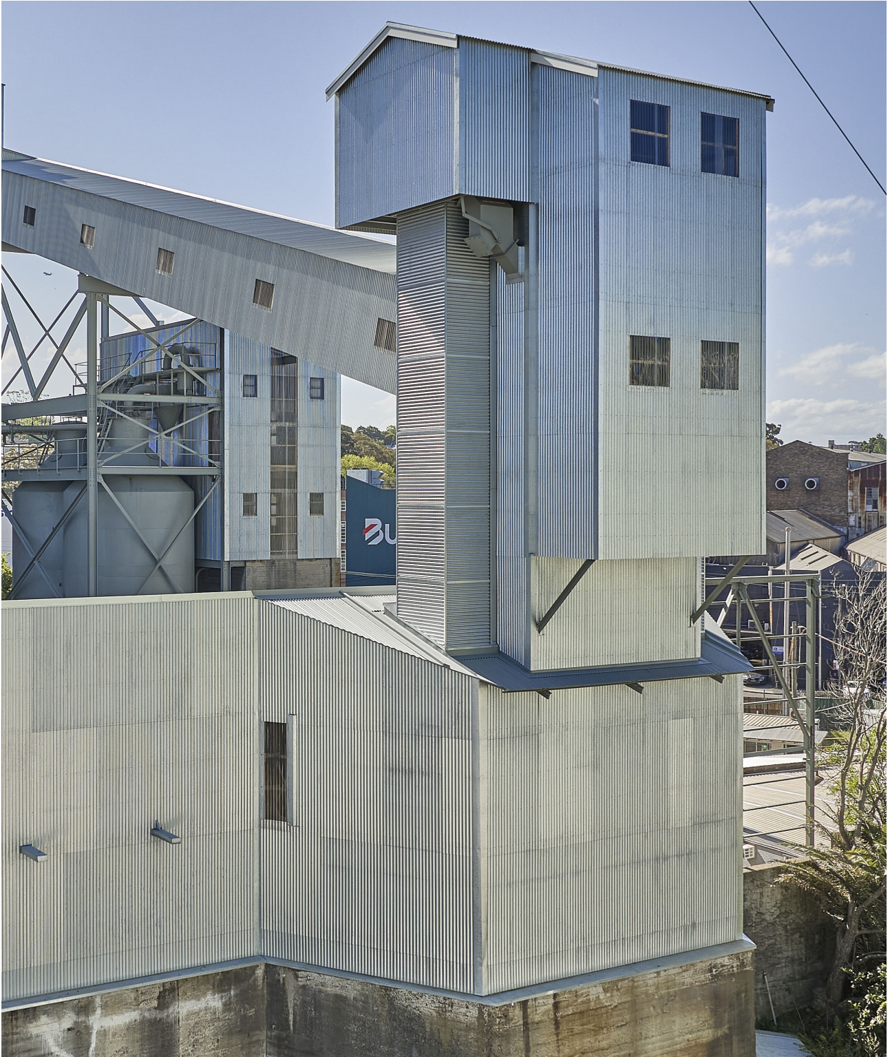
Figure 1.1.1 Coal Handling Shed and External Conveyor, 2024 (courtesy of Chris Bennett: Evolving Picture).
