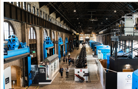
Figure 2.8.33 Niagara Parks Power Station generator floor (courtesy of Niagara Falls Canada).131
