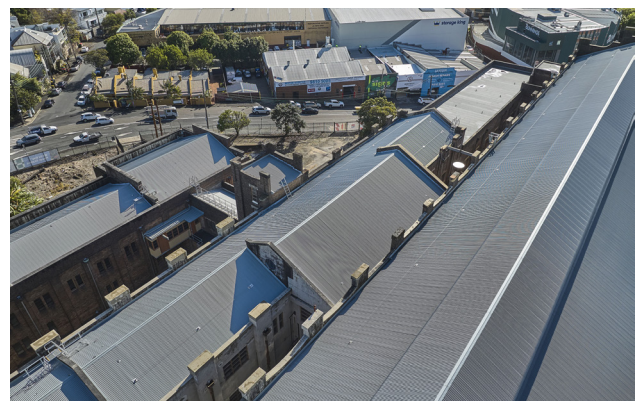
Figure 6.16.11 The corrugated steel and concrete rooftops of the White Bay Power Station, 2024 (courtesy of Chris Bennett: Evolving Picture).
