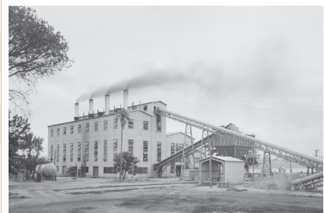
Figure 2.8.6 Maitland Power Station, 1954 (courtesy of the State Archives of NSW, NRS-20347-1-2-241).
