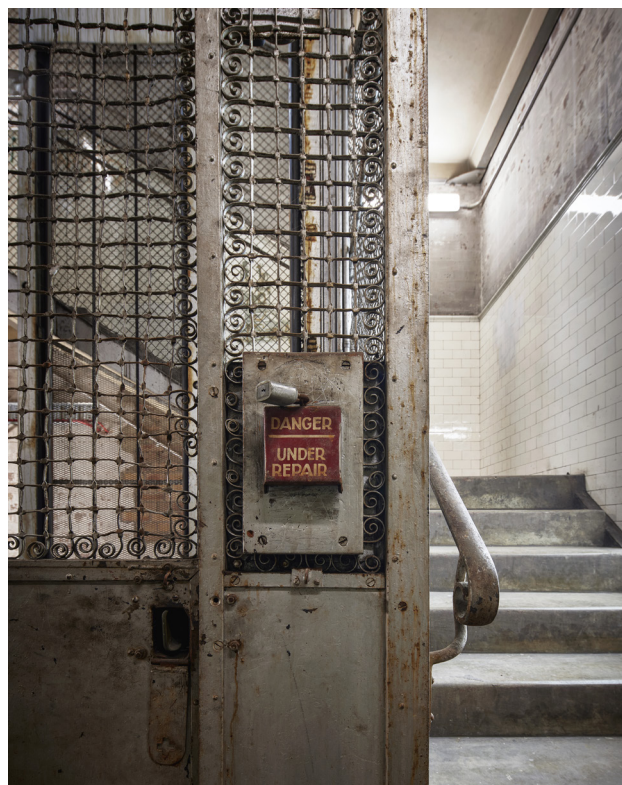
Figure 5.6.1 Lift Shaft of the Switch House, 2024 (courtesy of Toby Peet).
