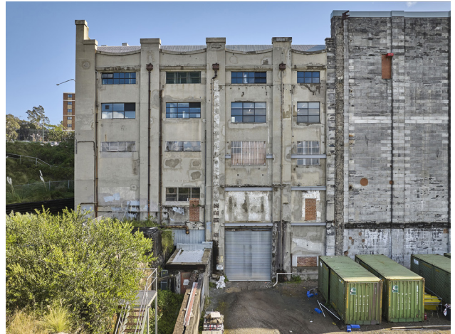
Figure 6.5.25 View of east elevation of Administration and Staff Accommodation, 2024 (courtesy of Chris Bennett, Evolving Picture).
