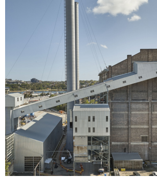
Figure 4.2.1 Coal Conveyor / Chimneys, 2023 (courtesy of Chris Bennett: Evolving Picture).
