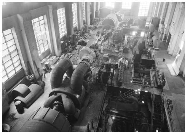
Figure 2.750 No. 2 Turbine Failure, 1958 (courtesy of NSW State Archives Collection, NRS-20347-1-42-1428).
