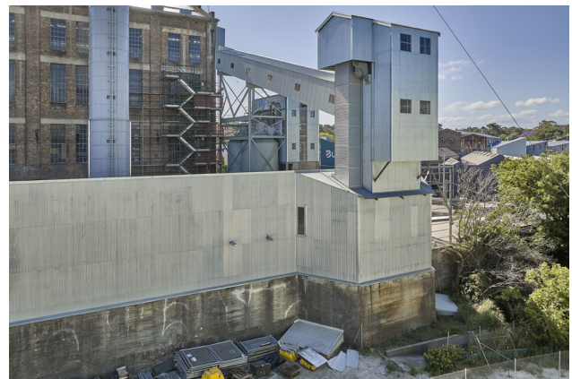
Figure 2.2.4 Coal Handling Shed, Transfer House, and External Conveyor, 2023 (courtesy of Chris Bennett: Evolving Picture).
