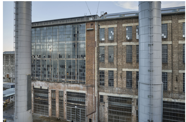
Figure 2.2.10 Boiler House east facade with Chimney Stacks in the foreground, 2024 (courtesy of Chris Bennett: Evolving Picture).
