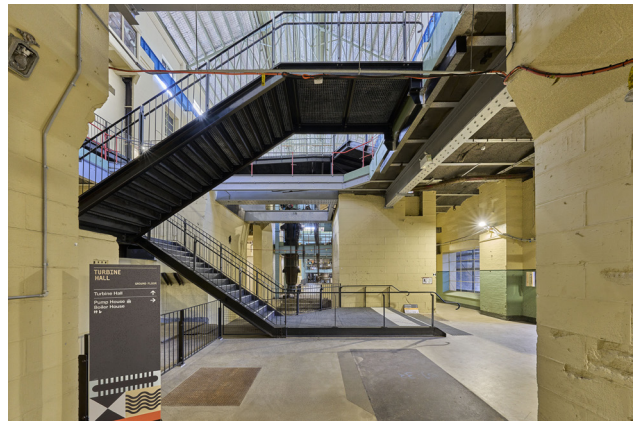
Figure 6.10.6 New stairs installed in the Turbine Hall during the 2022–24 works. The floor has also undergone remediation, 2024 (courtesy of Chris Bennett: Evolving Picture).
