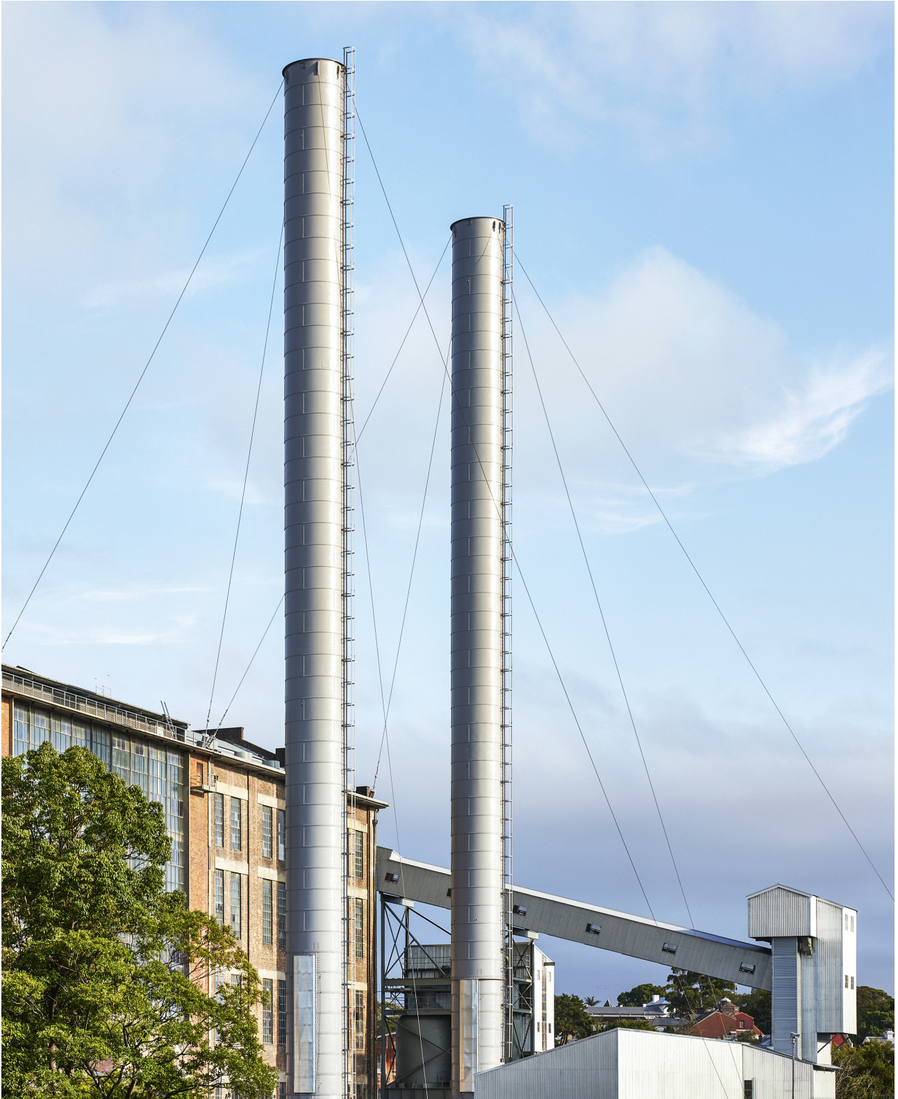
Figure 4.1.1 Chimney Stacks, External Conveyor, and Boiler House looking northwest, 2024 (courtesy of Toby Peet).
