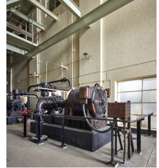
Figure 4.2.4 Pump House Level 2, 2024 (courtesy of Toby Peet).
