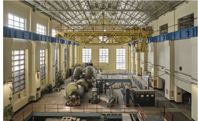
Figure 3.2.29 Turbine Hall Interior looking north, July 2024 (courtesy of Chris Bennett: Evolving Picture).
