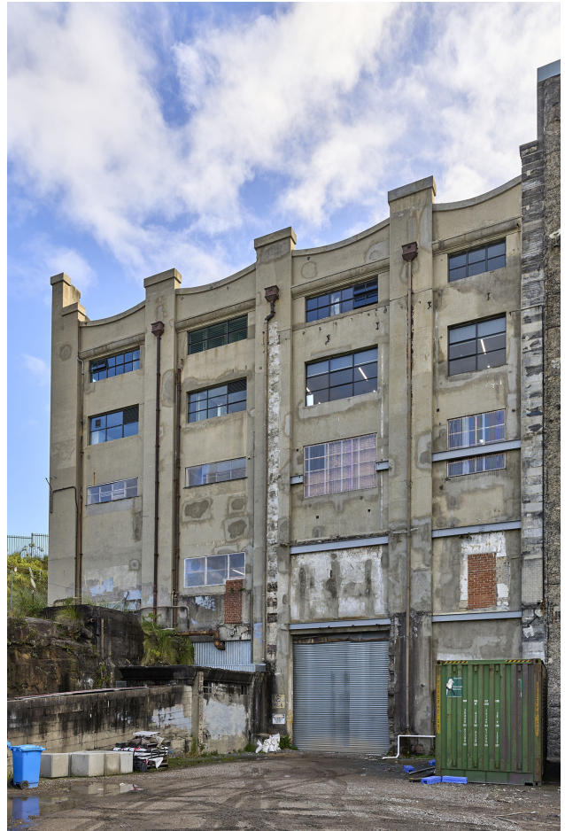
Figure 4.2.33 The eastern facade of the Administration and Staff Accommodation, 2024 (courtesy of Chris Bennett: Evolving Picture).
