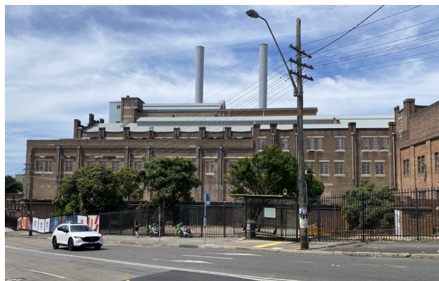
Figure 3.2.17 Western Elevation, viewed from Victoria Road, March 2024 (Design 5 – Architects).
