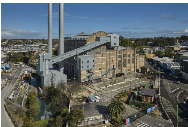
Figure 2.2.27 North Forecourt (middle) and Coal Wash Pit (left), 2024 (courtesy of Chris Bennett: Evolving Picture).
