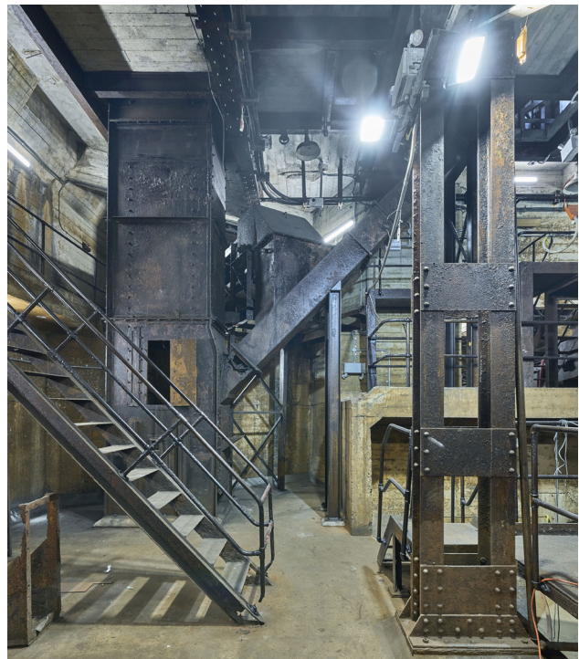
Figure 6.16.6 Basement of the Coal Handling Shed with lead encapsulated machinery, 2023 (courtesy of Chris Bennett: Evolving Picture).
