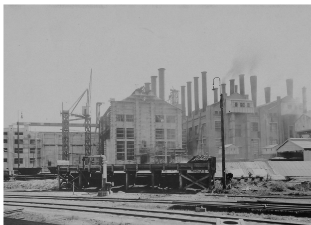
Figure 6.11.1 Boiler House No. 2 under construction, c.1920s (courtesy of State Rail Authority records, State Archives Collection, 0363-011).
