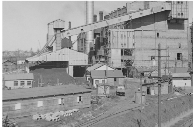
Figure 6.11.3 Dry Coal Store building on the left of the Coal Handling Shed, c.1950 (courtesy of ECNSW Photo Collection, 00906).
