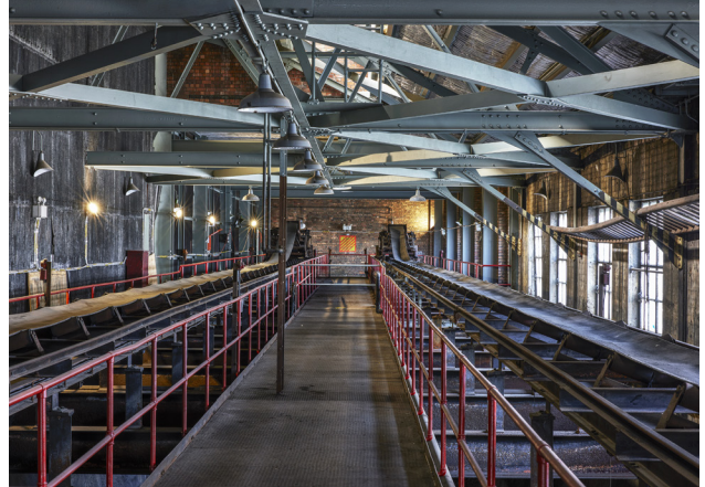
Figure 5.5.3 Conveyor Level of the Boiler House looking north, 2023 (courtesy of Toby Peet)
