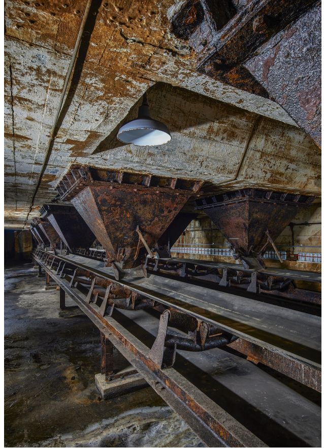
Figure 4.2.20 The Coal Handling Shed basement level, 2023 (courtesy of Toby Peet).
