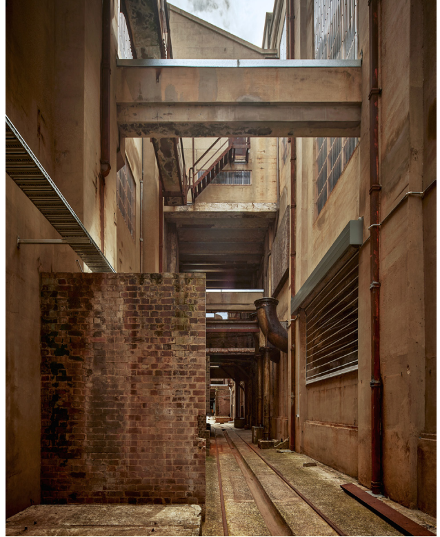
Figure 4.2.38 Transformer Alley looking north, 2024 (courtesy of Toby Peet).
