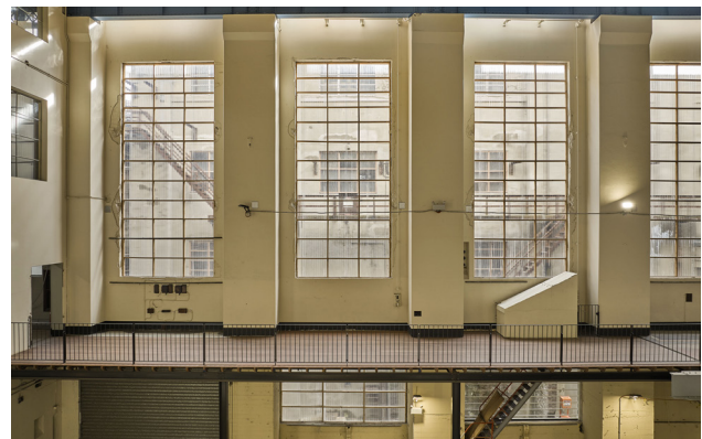
Figure 6.16.2 Corrugated clear polycarbonate coverings to Turbine Hall window openings, 2024 (courtesy of Chris Bennett: Evolving Picture).
