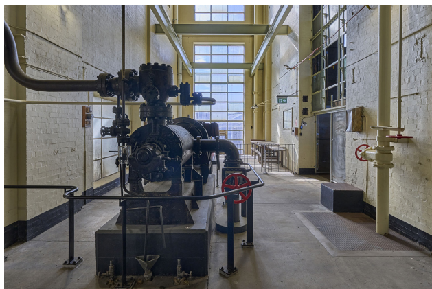
Figure 4.2.28 Pump House looking north, 2024 (courtesy of Chris Bennett: Evolving Picture).
