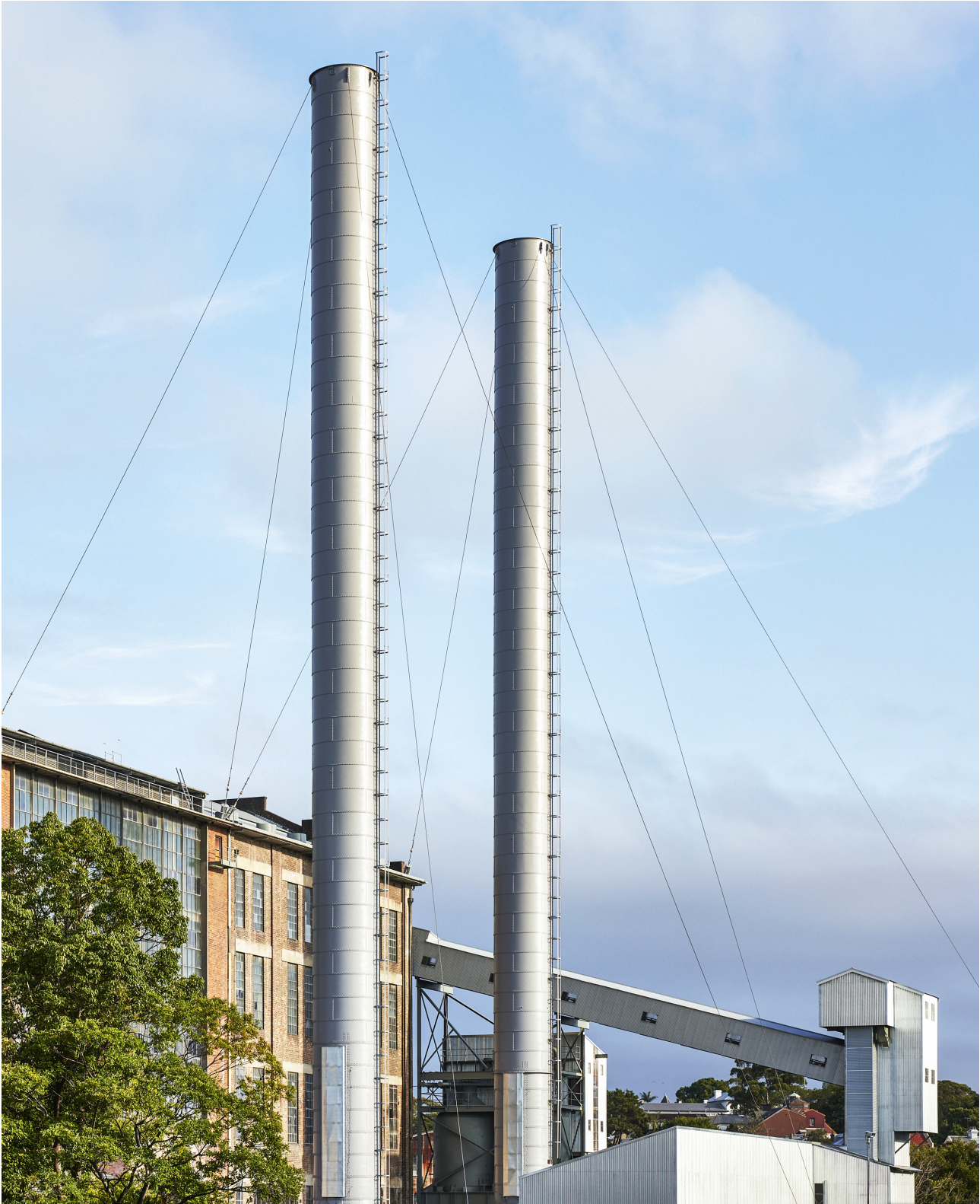
Figure 3.71 Chimney Stacks, External Conveyor, and Boiler House looking northwest, 2024 (courtesy of Toby Peet).
