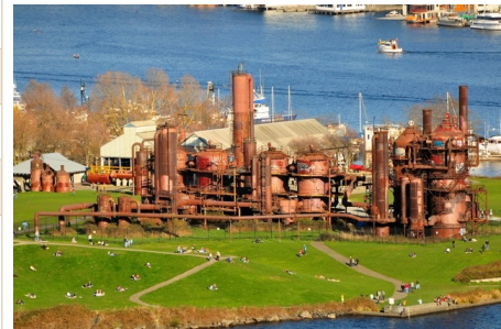
Figure 2.8.22 Gas Works Park, 2010 (courtesy of Tony Cyphert).119
