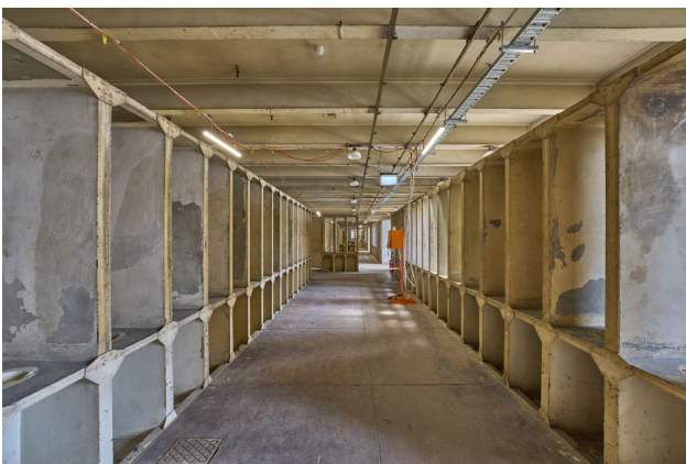
Figure 6.6.43 South section of Level 1 of the Switch House with the concrete housing for the cycle switches, 2023 (courtesy of Chris Bennett: Evolving Picture).
