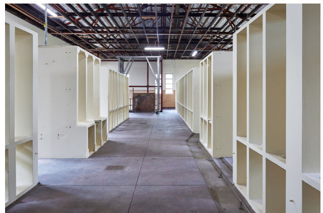
Figure 6.6.53 Level 2 of the 1948 Switch House, 2024 (courtesy of Toby Peet).
