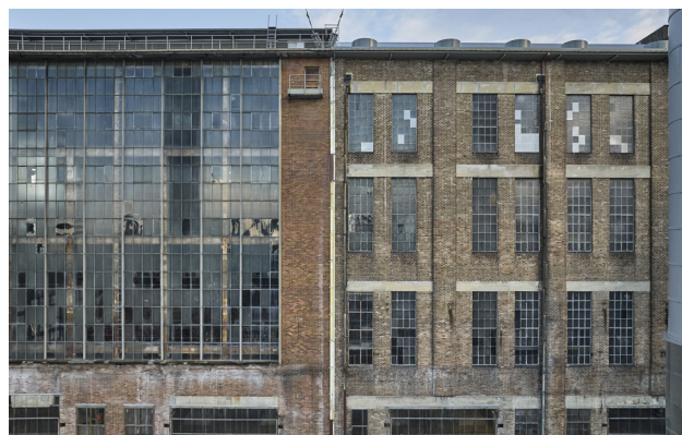
Figure 6.16.10 Windows of the Boiler House east facade, 2024 (courtesy of Chris Bennett: Evolving Picture).
