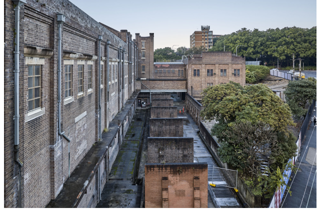
Figure 6.6.54 Transformer Yard looking south, 2024 (courtesy of Chris Bennett).
