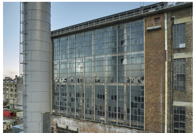
Figure 2.8.41 Boiler House Curtain Wall, east elevation, 2024 (courtesy of Chris Bennett: Evolving Picture).
