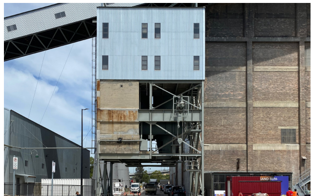
Figure 3.2.22 Ash Handling Tower and north facade of Boiler House, March 2024 (Design 5 – Architects).
