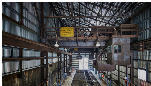
Figure 6.6.11 Coal Handling Shed looking south, 2024 (courtesy of Toby Peet).
