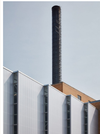
Figure 2.8.36 Stack at Beloit College Powerhouse, 2020 (cropped, courtesy of Dezeen).133
