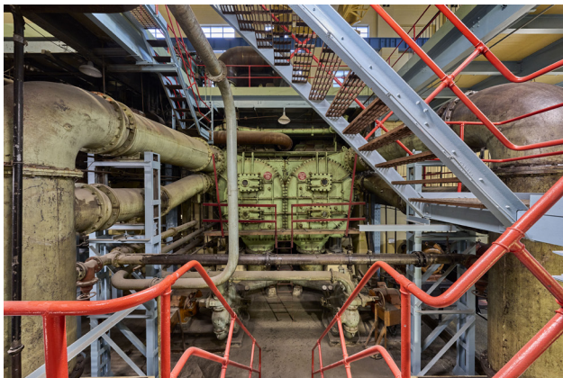
Figure 2.2.31 Turbine Hall Condensers, 2024 (courtesy of Chris Bennett: Evolving Picture).
