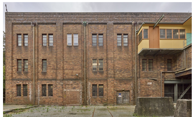
Figure 3.2.34 Control Room, East Elevation, November 2023 (courtesy of Chris Bennett: Evolving Picture).
