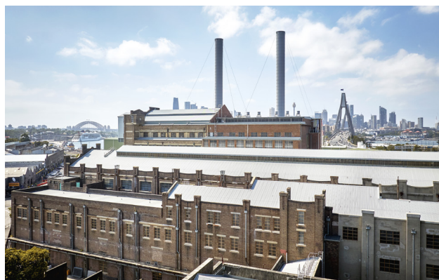
Figure 3.2.26 Turbine Hall / Pump House Exterior, West Elevation, March 2024 (courtesy of Toby Peet).
