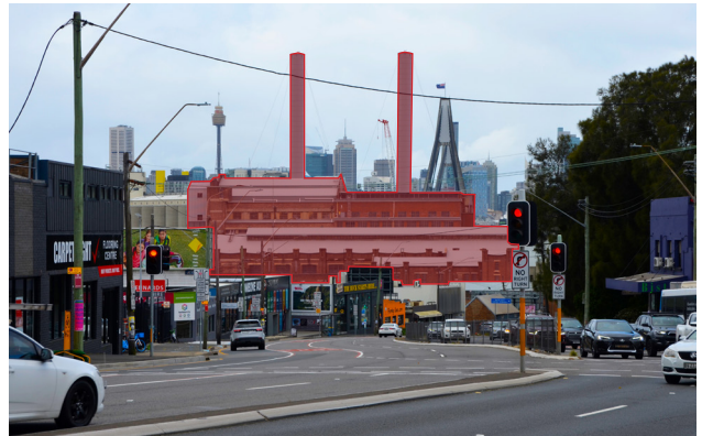
Figure 6.5.13 View of the power station from near the Victoria Road intersection with Gordon Street, 2024.
