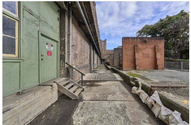
Figure 6.5.26 View looking south along Transformer Yard towards the Control Room Bridge, 2024 (courtesy of Chris Bennett: Evolving Picture).
