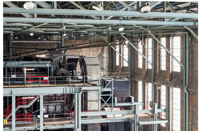
Figure 2.2.11 Ground Level of Coal Handling Shed, 2023 (courtesy of Toby Peet).
