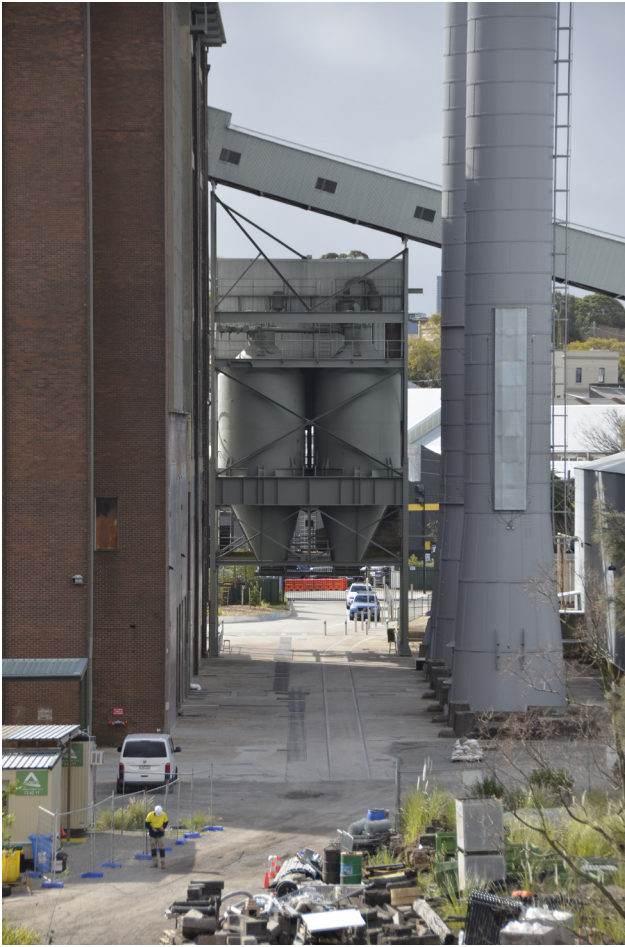
Figure 6.5.23 View looking north along axis of Ash Handling Yard, terminating at the Ash Handling Tower, 2024 (Design 5 - Architects).
