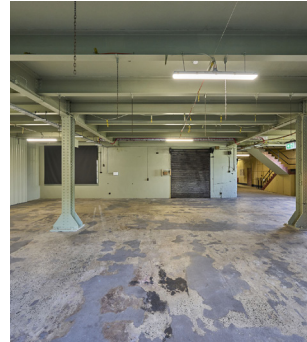
Figure 4.2.5 Administration Building Level 1, 2023 (courtesy of Chris Bennett: Evolving Picture).
