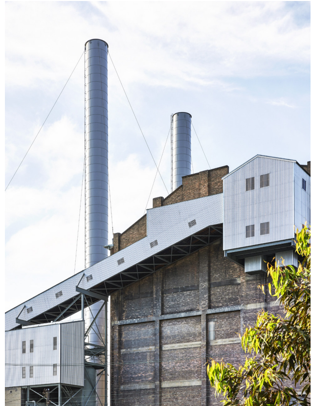
Figure 3.2.19 Ash Handling Tower, Chimney Stacks, and the north facade of the Boiler House, December 2023 (courtesy of Toby Peet).
