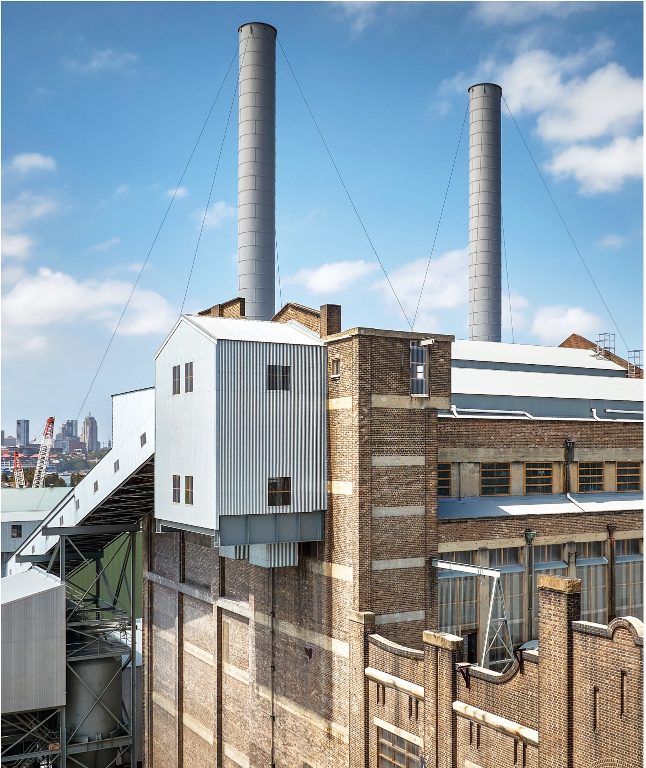
Figure 2.1.1 External Coal Conveyor and Transfer House, March 2024 (courtesy of Toby Peet).
