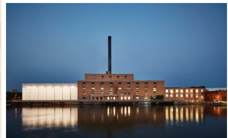
Figure 2.8.24 Beloit College Powerhouse, 2021 (courtesy of Tom Harris, Archdaily).121
