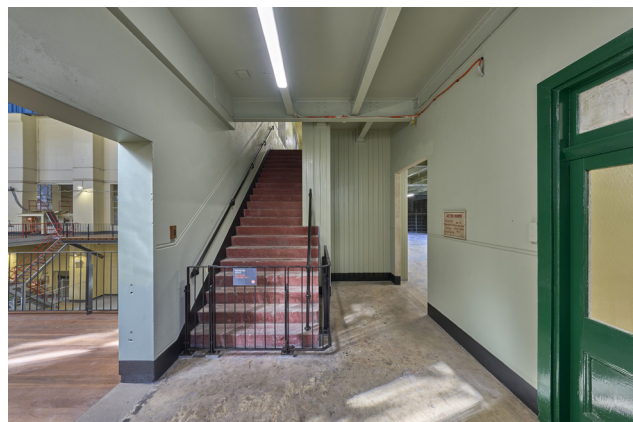
Figure 6.6.41 Existing encased lift shaft on Level 1, 2024 (courtesy of Chris Bennett: Evolving Picture).
