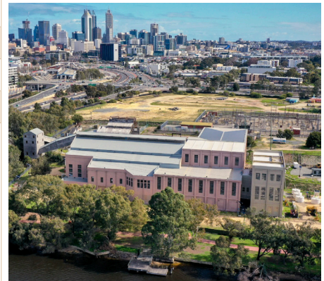
Figure 2.8.16 East Perth Power Station (courtesy of DevelopmentWA). 114
