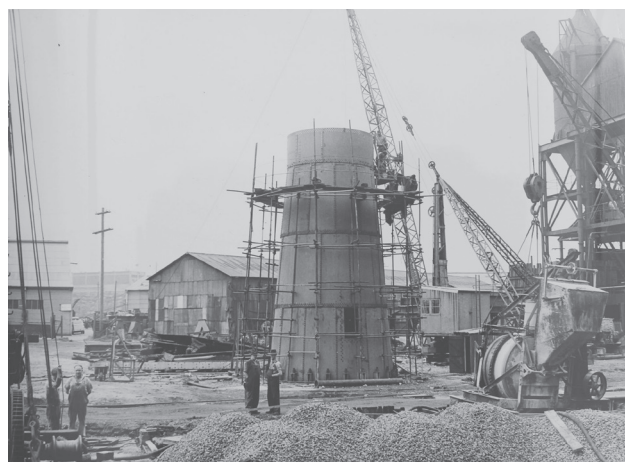
Figure 2.7.40 Construction of the new Chimney Stacks, 1949 (courtesy of the Railways Department, E1391).
