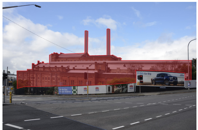
Figure 6.5.14 View of the power station from the intersection of Victoria Road with Robert Street, 2024.
