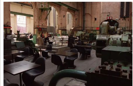
Figure 2.8.31 Turbines and seating inside Wapping Hydraulic Power Station when cafe was active (courtesy of Phil Adams).129
