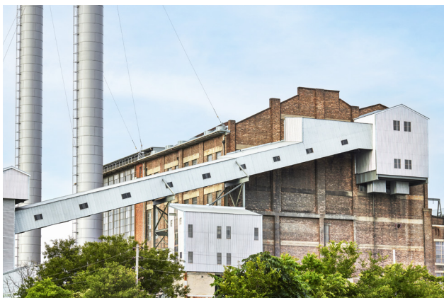
Figure 6.6.1 North Elevation of the White Bay Power Station, 2023 (courtesy of Toby Peet).
