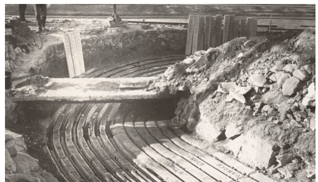
Figure 6.9.1 Cable laying at the White Bay Power Station, 1926 (courtesy of NSW State Archives, NRS-17420-2-4-363/061).
