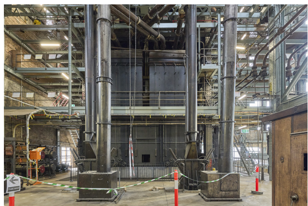
Figure 2.2.30 View of the Chutes from Hopper to Mill, the Pulverised Fuel Feed Pipes, and the No. 1 Boiler in the background, 2023 (courtesy of Chris Bennett: Evolving Picture).
