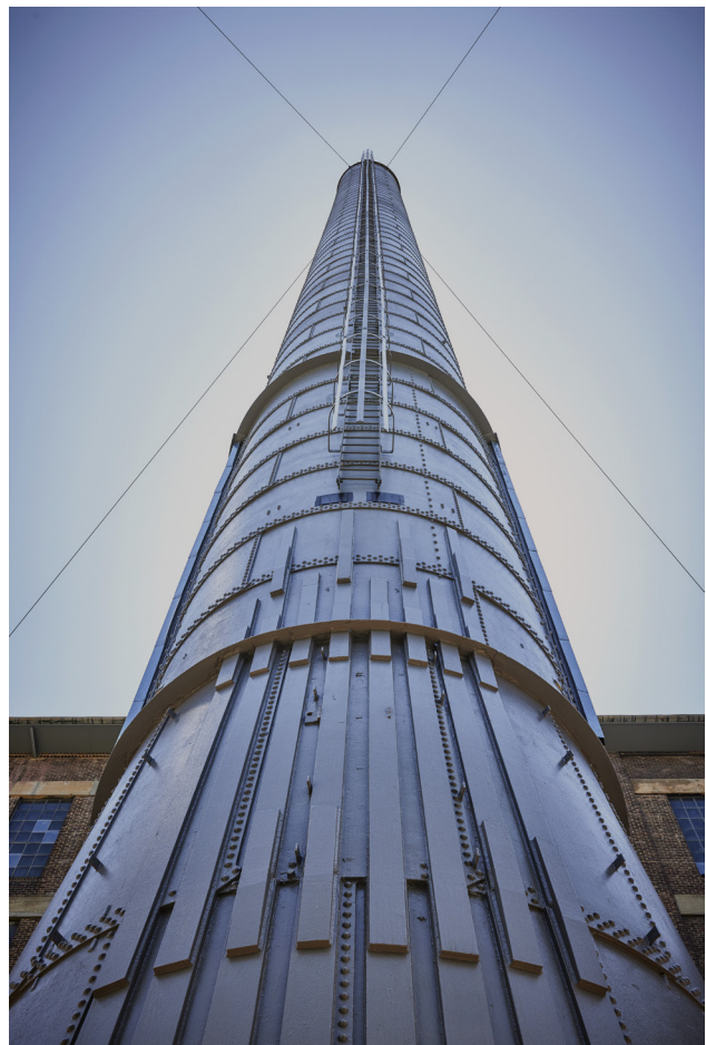
Figure 6.21.1 Chimney Stack of the White Bay Power Station, 2023 (courtesy of Toby Peet).
