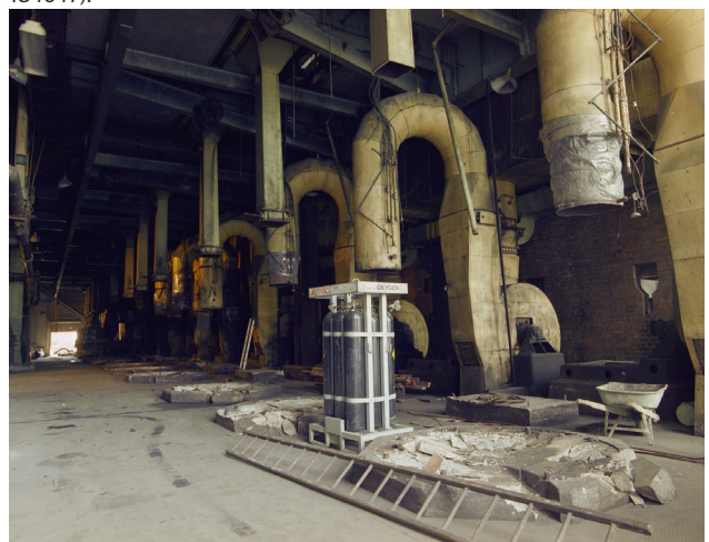
Figure 2.7.59 The Boiler House with removed pulverising mills, 1996 (courtesy of the ECNSW Archives, CN7.0020-T).
