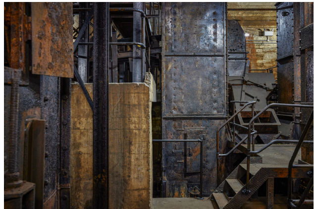
Figure 6.6.3 Coal Elevators in the Basement of the Coal Handling Shed, 2024 (courtesy of Toby Peet).
