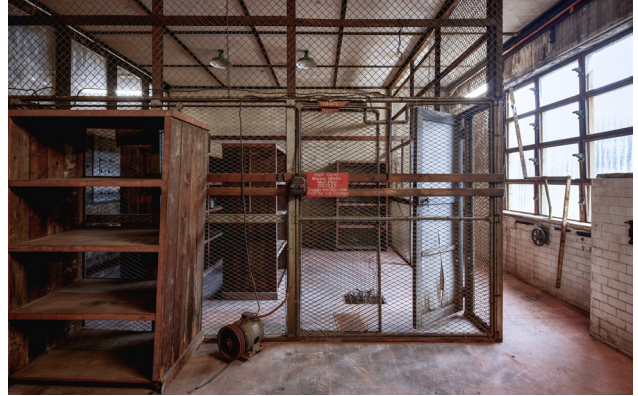
Figure 6.20.1 Storage room in Switch House, 2024 (courtesy of Toby Peet).
