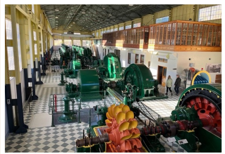
Figure 2.8.10 Waddamana Power Station Turbine Hall, 2023 (Alan Croker, Design 5 – Architects).
