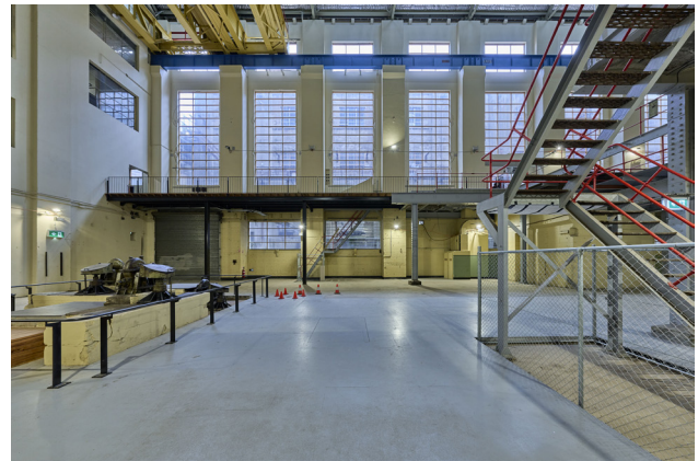
Figure 2.2.16 Turbine Hall south end at ground level, looking west, 2024 (courtesy of Chris Bennett: Evolving Picture).
