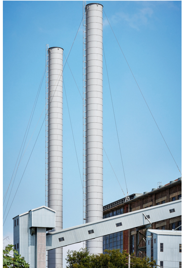
Figure 4.2.47 The Chimney Stacks behind the External Conveyor, 2024 (courtesy of Toby Peet).
