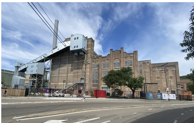
Figure 3.2.15 Northern Elevation, viewed from Robert Street, March 2024 (Design 5 – Architects).
