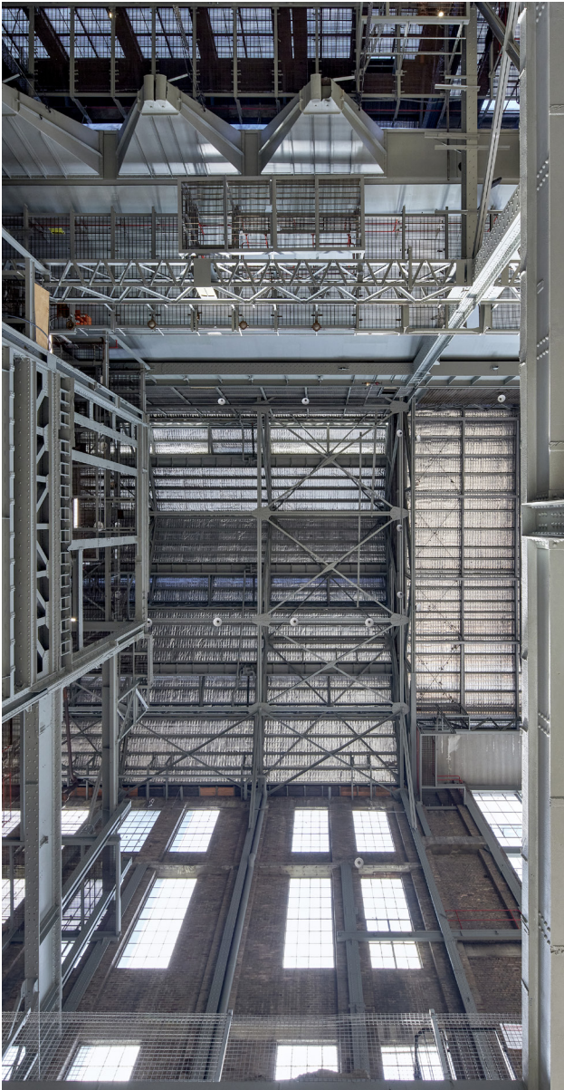
Figure 6.6.21 View of the underside of the Boiler House roof from the ground level through the void of the former Boiler No. 2, 2023 (courtesy of Toby Peet).
