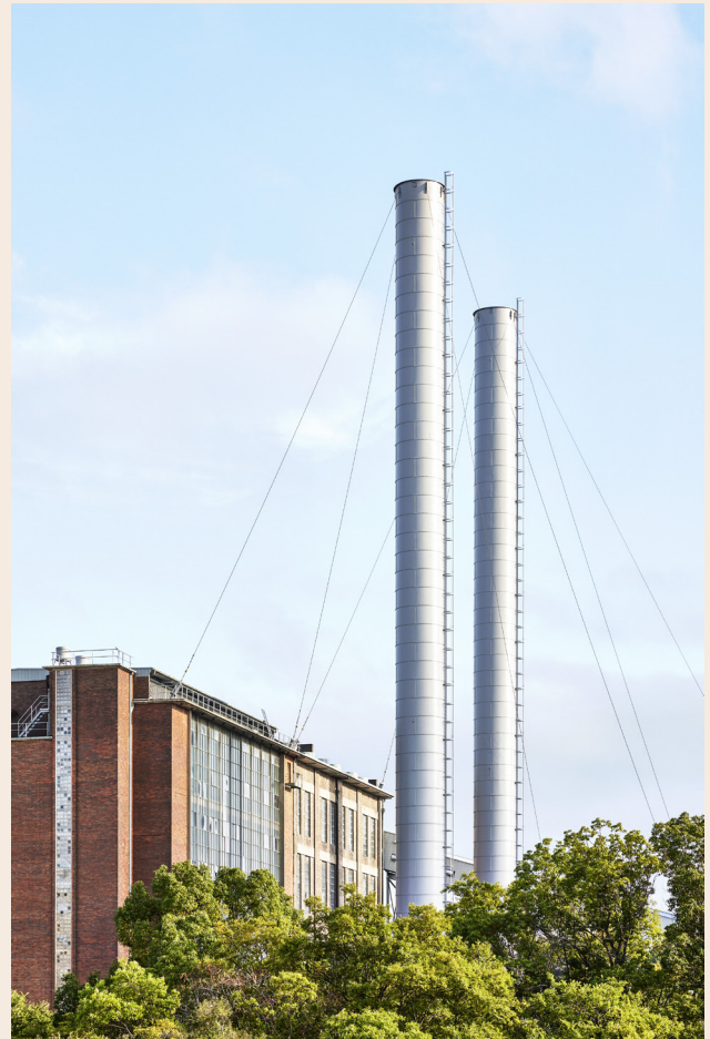
Figure 0.8: White Bay Power Station Chimney Stacks and Boiler House, 2023 (courtesy of Toby Peet).
