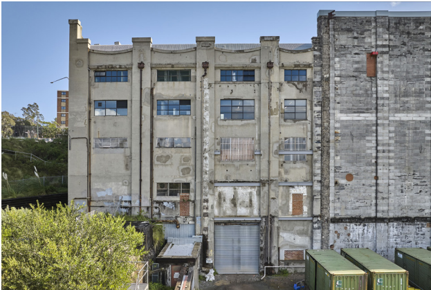
Figure 6.6.34 East facade of the Administration and Staff Accommodation, 2024 (courtesy of Chris Bennett: Evolving Picture).
