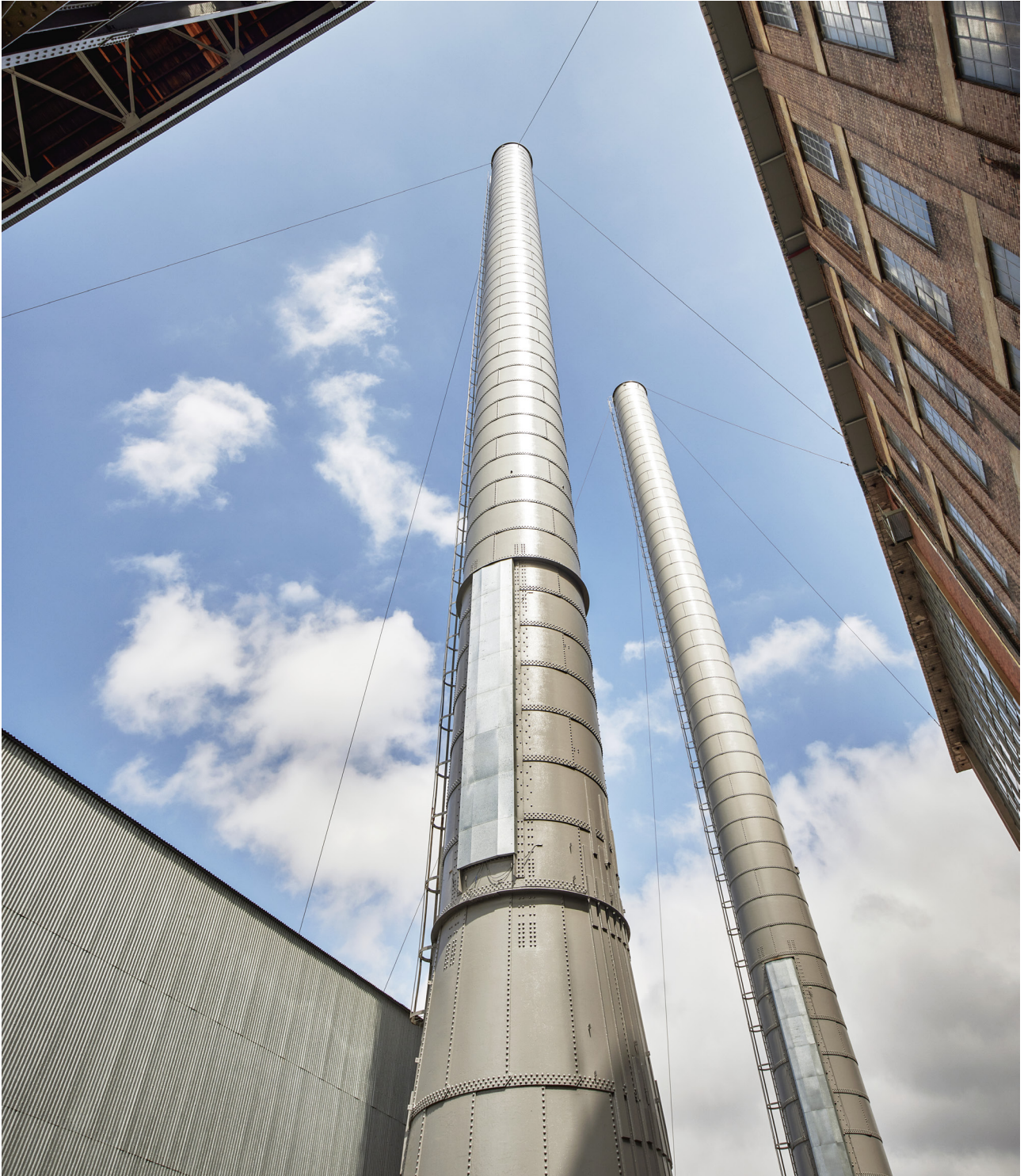
Figure 6.1.1 (left) Chimney Stacks, 2024 (courtesy of Toby Peet).
