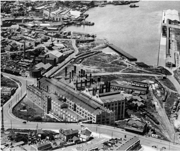
Figure 2.789 Aerial view of the White Bay Power Station, with the Hotel to its right, 1930 (courtesy of City of Sydney Archives, A-00007796, SRC352, 020/020600).
