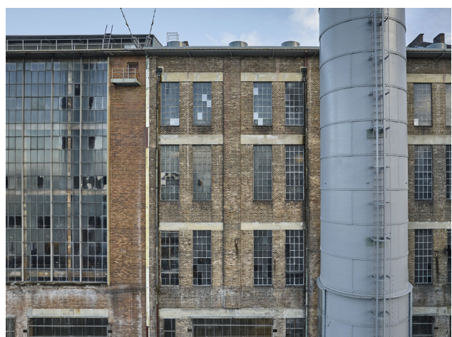
Figure 6.6.17 East facade of the Boiler House with iconic curtain wall on the left, 2023 (courtesy of Chris Bennett: Evolving Picture).
