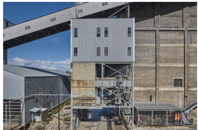
Figure 2.2.8 Ash Handling Tower north elevation, 2024 (courtesy of Chris Bennett: Evolving Picture).
