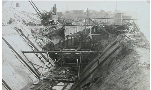
Figure 2.7.26 Excavation of White Bay Power Station Channel, 1912 (courtesy of Powerhouse Collection).
