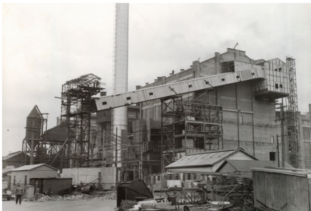
Figure 2.744 Construction of the Coal Handling Shed, External Conveyor, and Ash Handling Tower with one complete Chimney Stack, 1953 (courtesy of Inner West Council archives, BRN: 193659).
