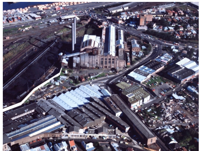
Figure 2.7.58 Aerial view of the decommissioned and closed White Bay Power Station, c. 1995 (courtesy of the Inner West Council Archives, BRN: 184647).
