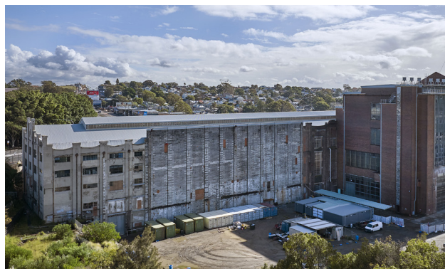
Figure 3.2.27 Turbine Hall / Pump House Exterior, from southeast, July 2024 (courtesy of Chris Bennett: Evolving Picture).
