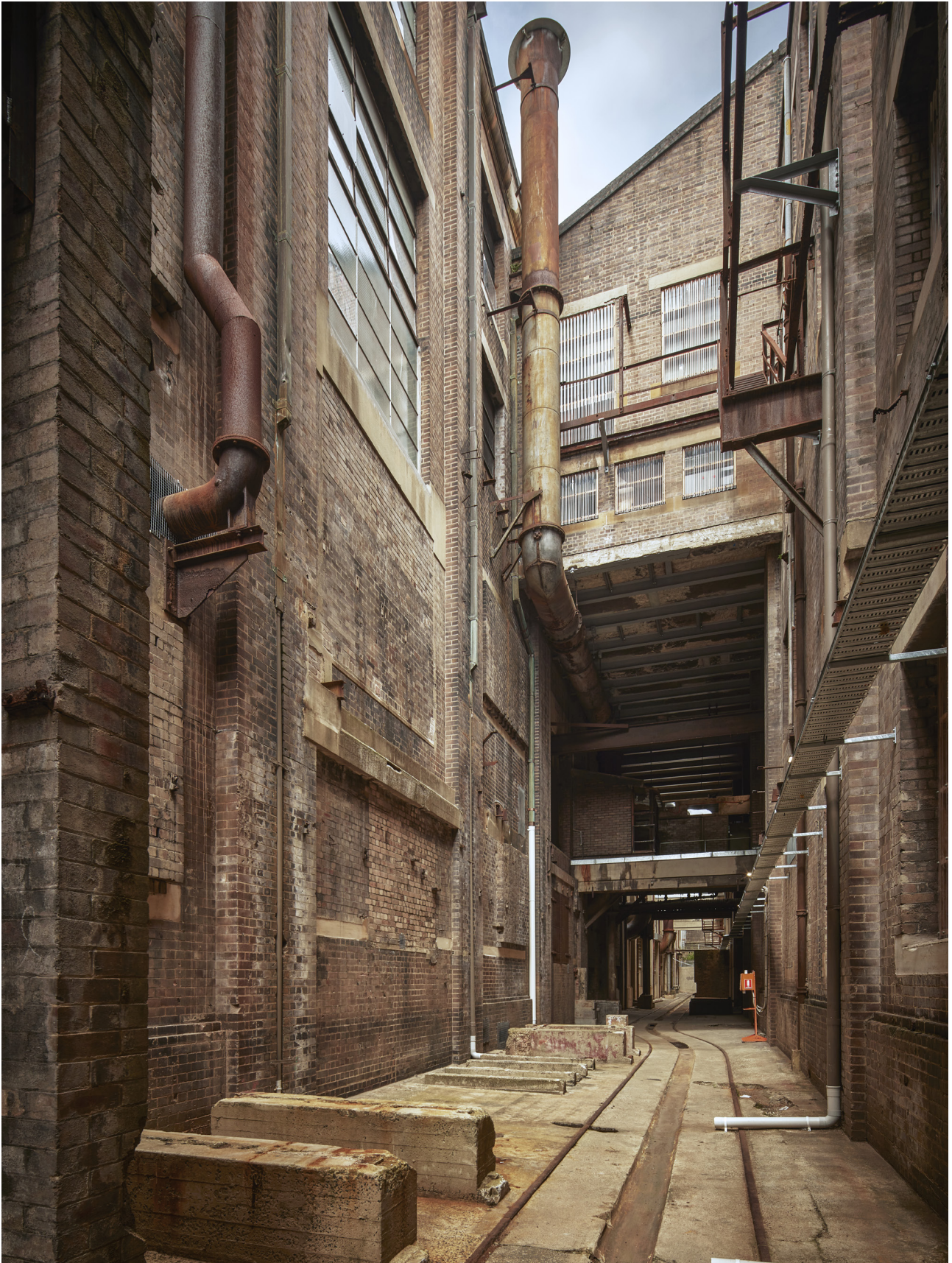
Figure 2.8.46 Transformer Alley looking south, 2024 (courtesy of Toby Peet).
