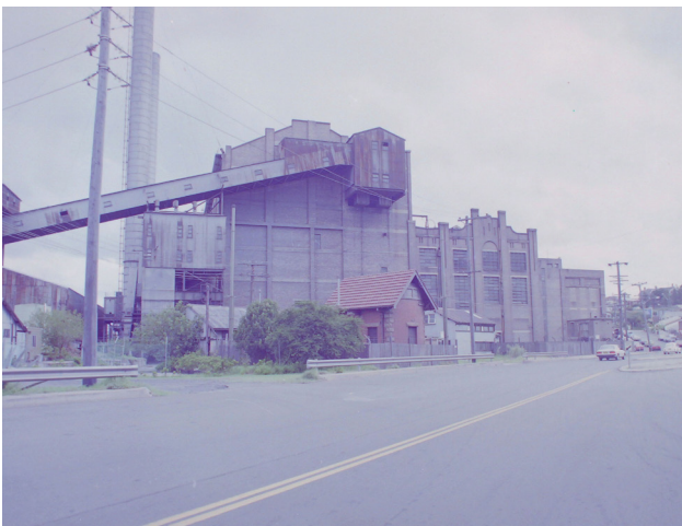
Figure 2.7.56 White Bay Power Station, 1986 (courtesy of the ECNSW Archives, CN7.0012-1D).
