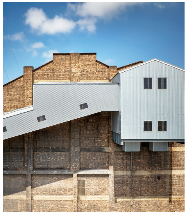
Figure 6.16.9 The External Conveyor, Transfer House and brickwork of the north facade of the Boiler House, 2024 (courtesy of Toby Peet).
