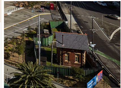
Sewage Pumping Station No. 7, 2024 (courtesy of Chris Bennett: Evolving Picture)
