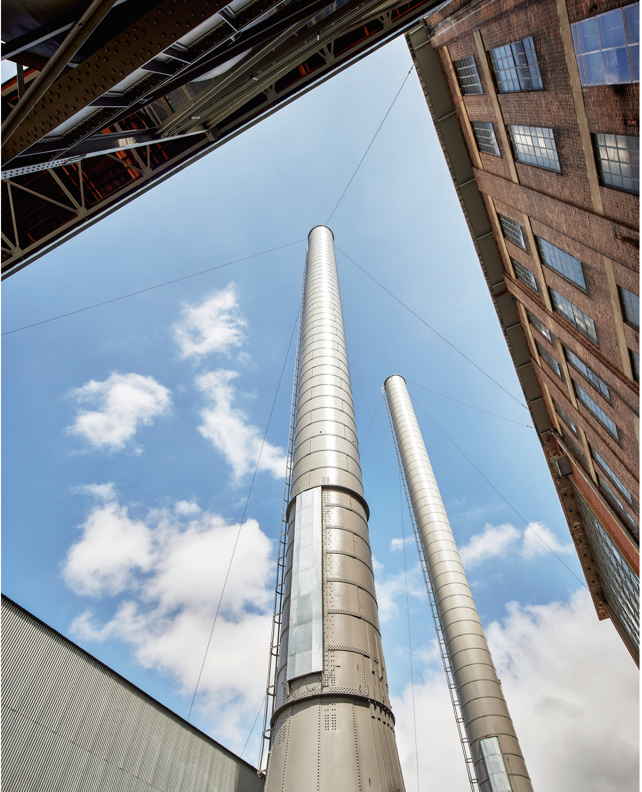
Figure 9.1 Chimney Stacks, 2024 (courtesy of Toby Peet)
