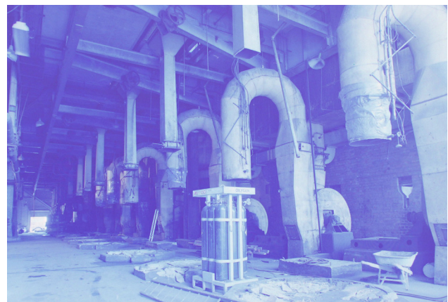
Figure 3.5 Boiler House decommissioning, 1996 (courtesy of ECNSW Archive)
