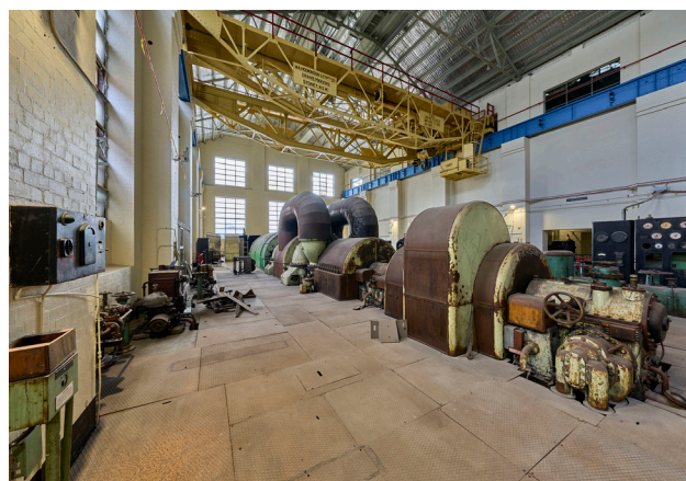
Figure 5.8 Level 2 extant Parsons Turbo-Alternator Set, 2024 (courtesy of Chris Bennett: Evolving Picture)
