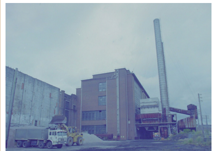
View north of Boiler House, precipitators and Chimney Stacks, 1994 (courtesy of ECNSW Archive, CN7.0016-F)
