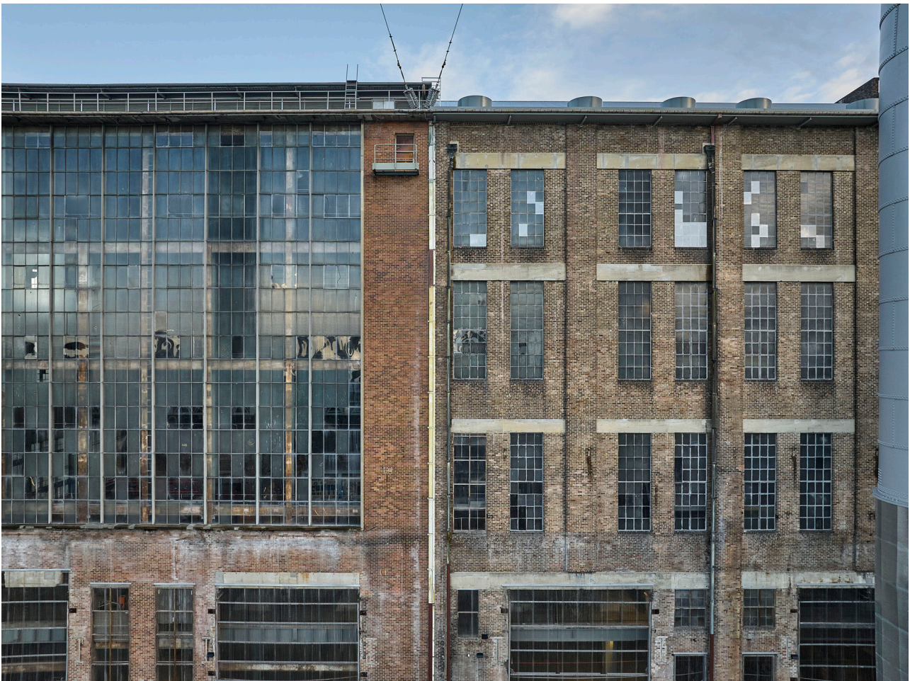
Figure 3.12 Boiler House East Elevation, 2024 (courtesy of Chris Bennett: Evolving Picture)
