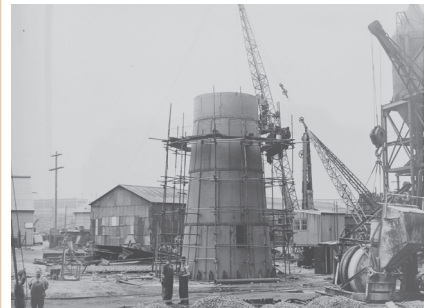
Chimney Stack during construction, 1949 (courtesy of Railways Department Archives, A5115; E1391)
