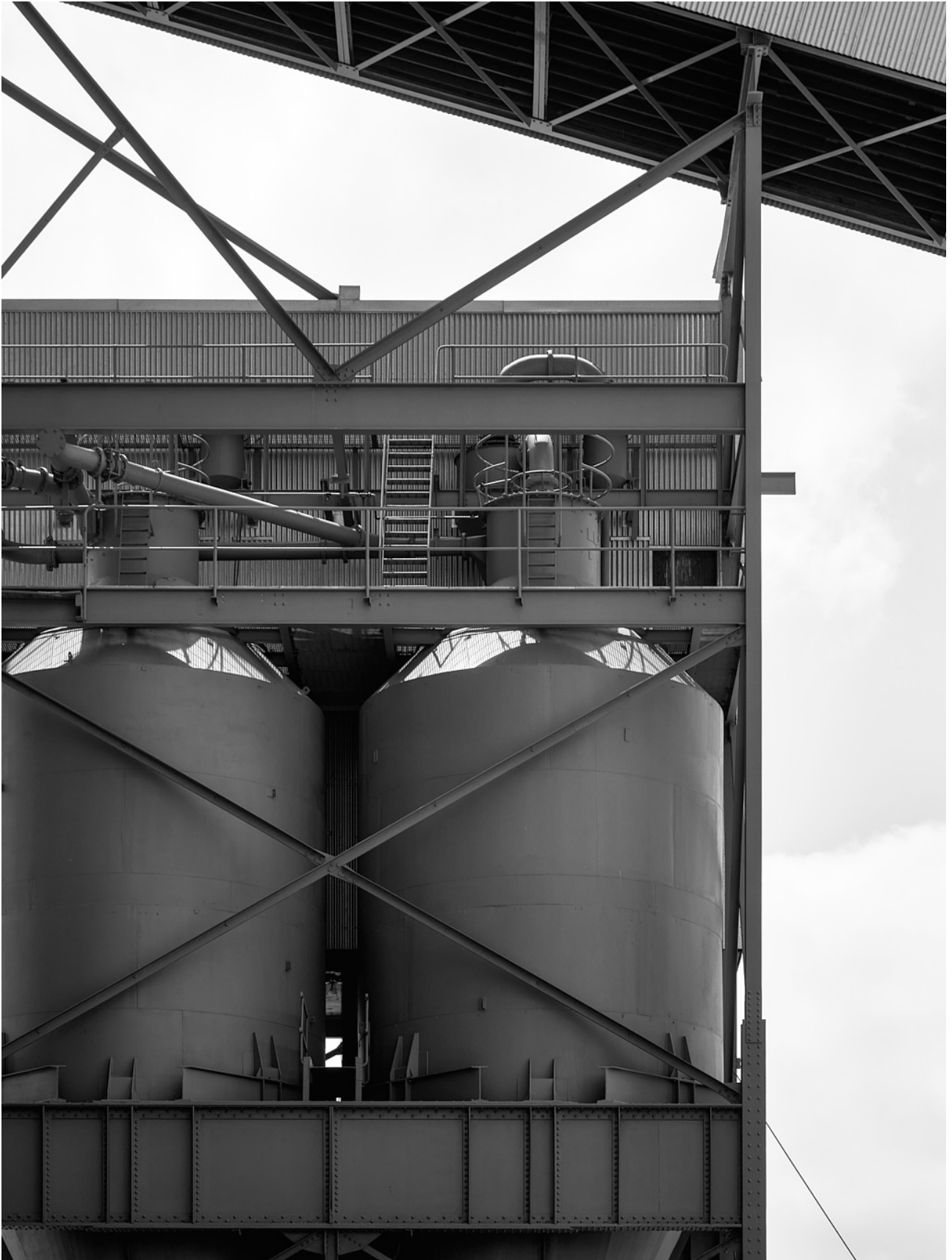
Figure 2.8 Ash Handling Tower Drums, 2024 (courtesy of Toby Peet), cropped
