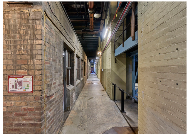
Figure 4.5 Pump House north, Ground Floor, 2024 (courtesy of Chris Bennett: Evolving Picture)
