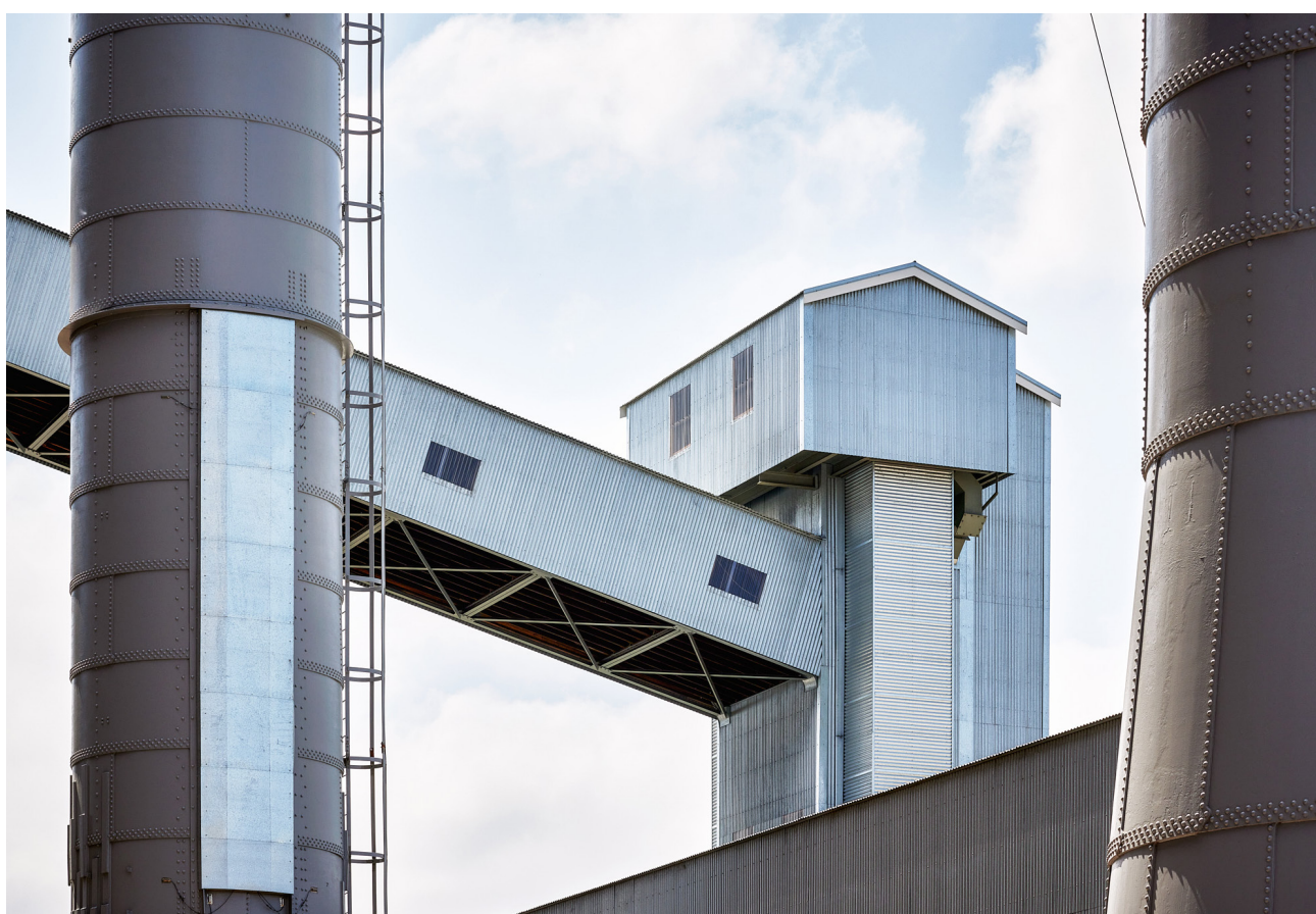
Figure 1.11 Coal Handling Shed from South, 2024 (courtesy of Toby Peet)
