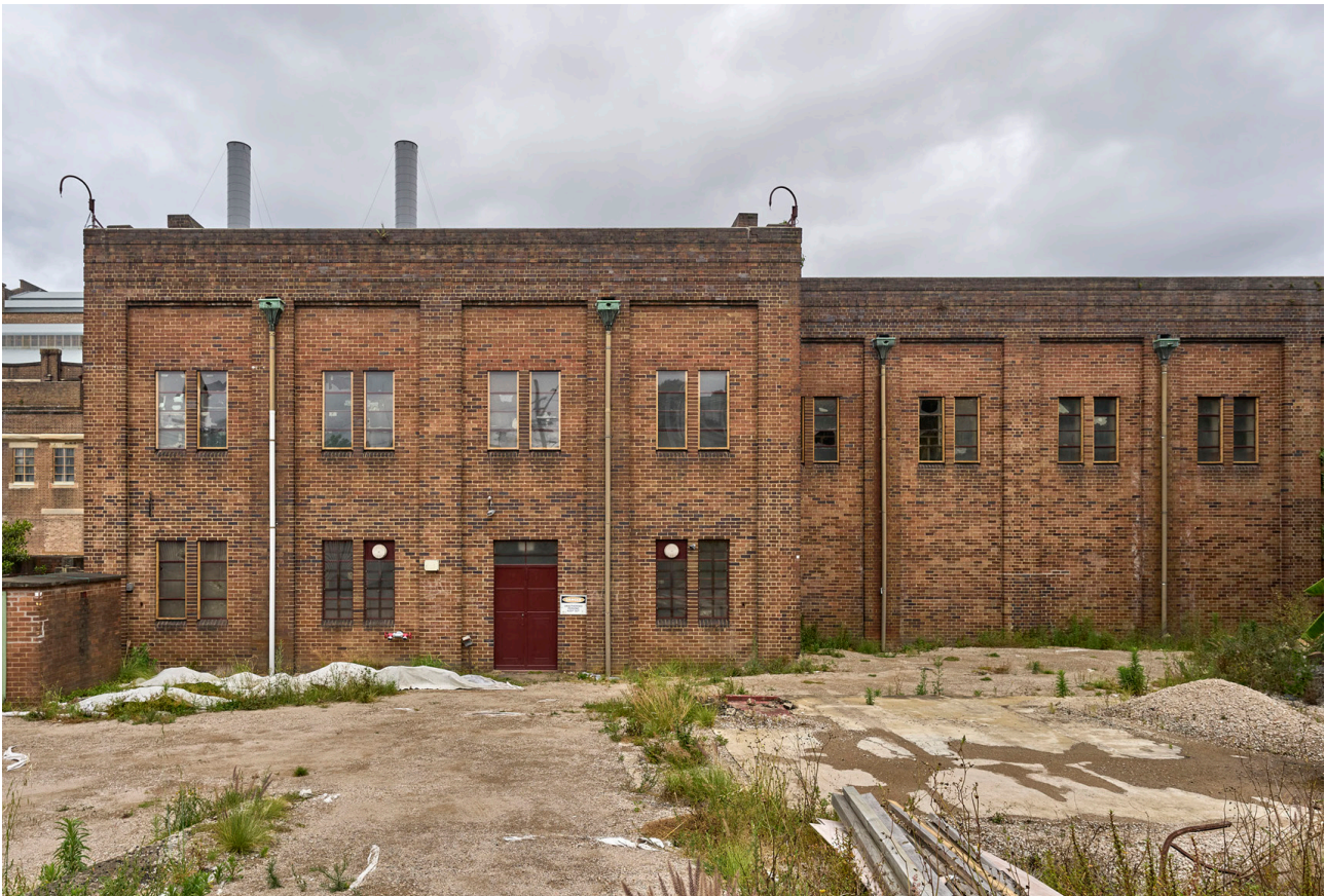
Figure 8.13 Control Room West Elevation, 2024 (courtesy of Chris Bennett: Evolving Picture)
