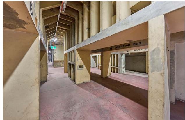
Figure 7.7 Switch House Level 1 Bus Floor, 2024 (courtesy of Chris Bennett: Evolving Picture)
