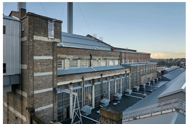
Figure 3.9 Boiler House Western Elevation, 2024 (courtesy of Chris Bennett: Evolving Picture)
