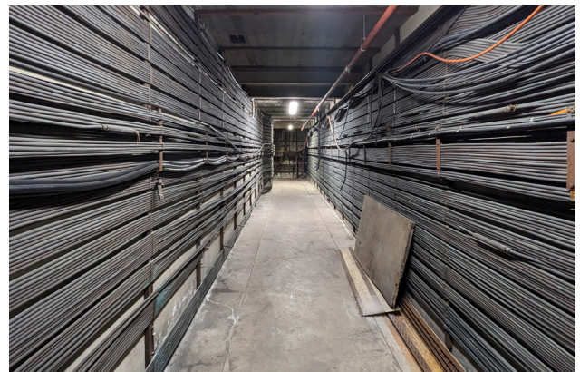
Figure 8.6 First Floor Cable Corridor, 2024 (Design 5 - Architects)
