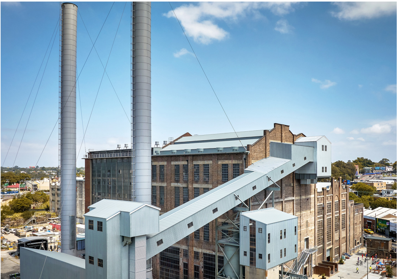
Figure 1.9 Coal Handling Shed connecting to Transfer House with External Conveyor, 2024 (courtesy of Toby Peet)
