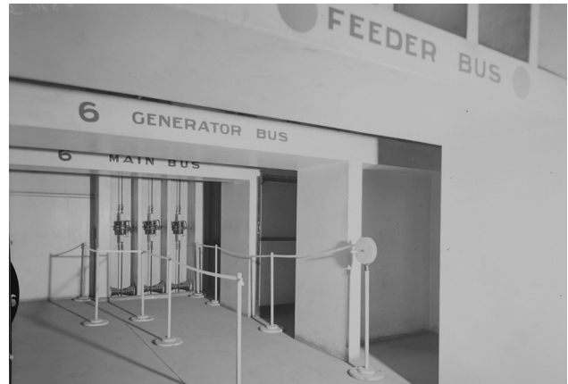
Figure 7.6 Switch House Level 1 Bus Floor, 1964 (courtesy of ECNSW Archive, 05370D)
