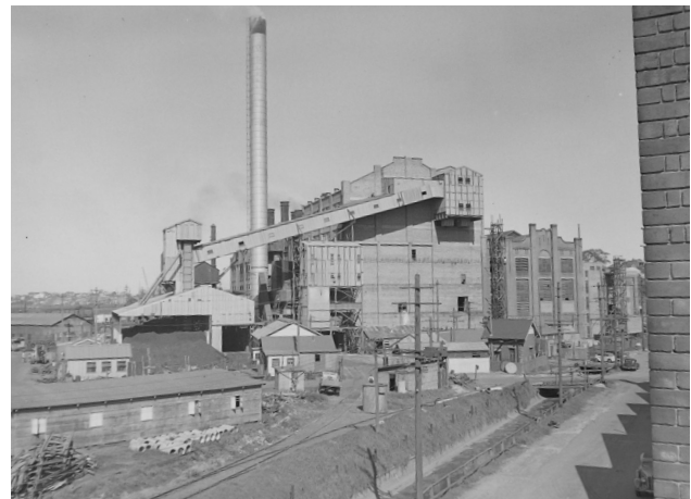
Figure 2.5 Northern Elevation of White Bay Power Station, c.1955 (courtesy of ECNSW Archive), angle adjusted.
