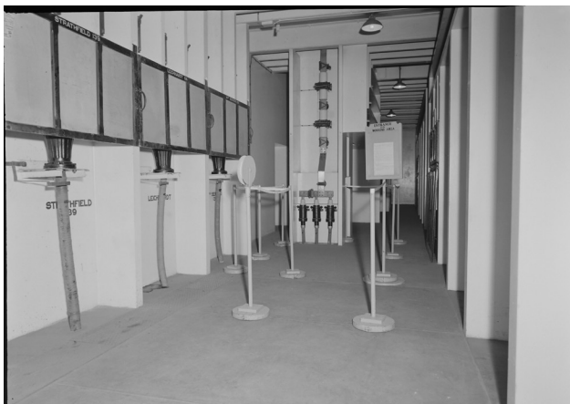
Figure 8.7 First Floor Bus Floor (CS1.2) with white taping method, 1958 (courtesy of ECNSW Archive, 02360C)
