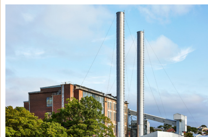
The pair of Chimney Stacks as seen from the south, 2024 (courtesy of Toby Peet)
