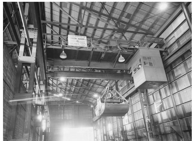
Figure 1.8 Crane and control cabin in operation, 1957 (courtesy of NSW State Archives, NRS-20347-1_001324).
