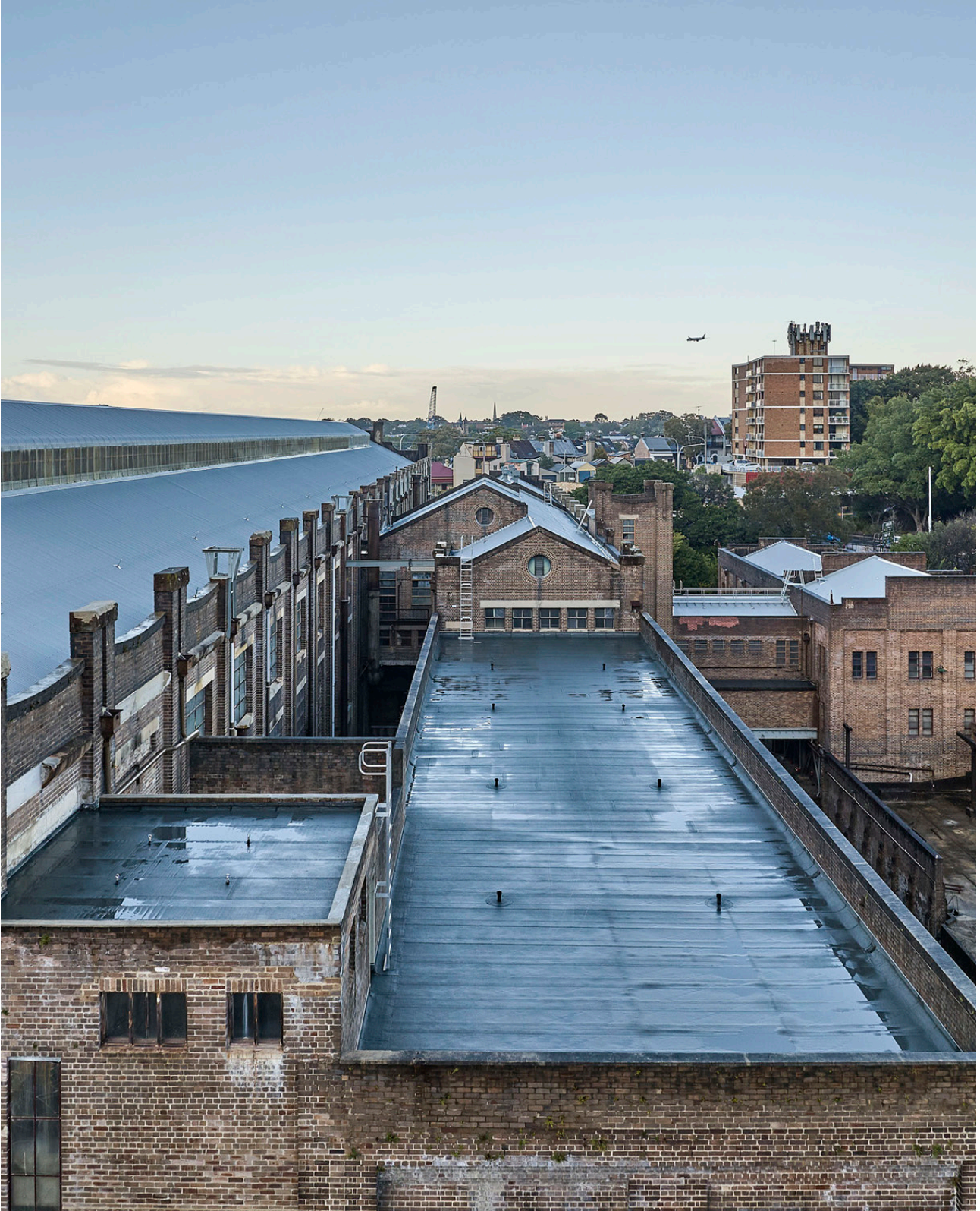
Figure 7.1 Switch House Roof from North, 2024 (courtesy of Chris Bennett: Evolving Picture)
