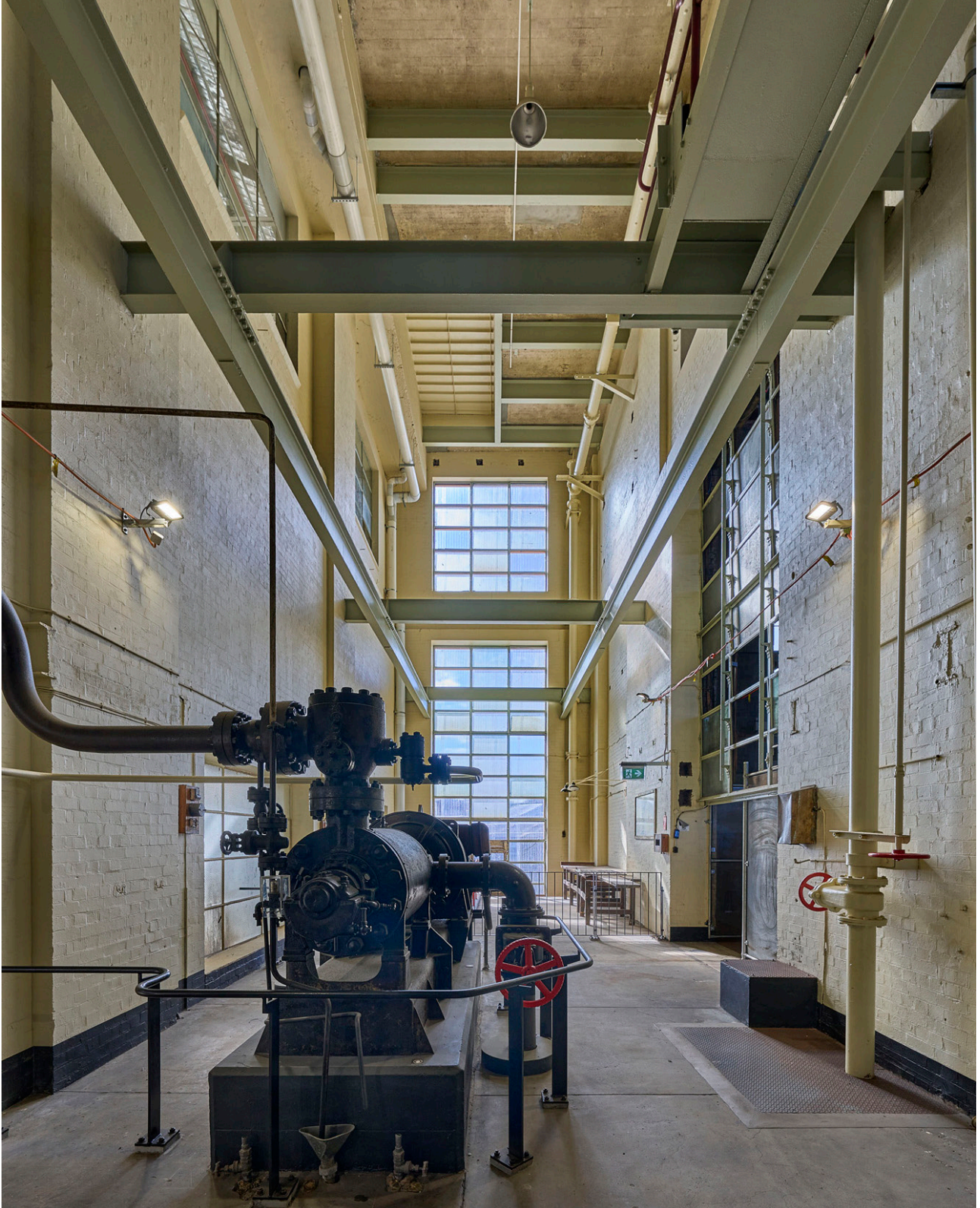
Figure 4.1 Pump House Internal, facing north, 2024 (courtesch of Chris Bennett: Evolving Picture)
