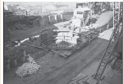
Chimney Stack base, 1957 (courtesy of NSW State Archives, NRS 20347-1-001210_B)
