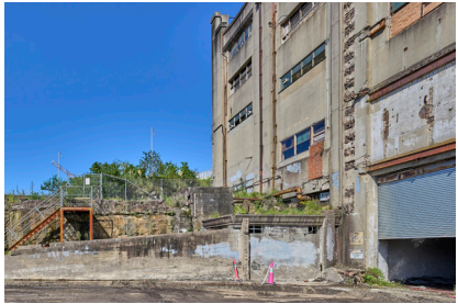
Terraced layers of the Mid & Upper South Yards viewed from the (lower) South Yard, 2022 (courtesy of Chris Bennett: Evolving Picture)
