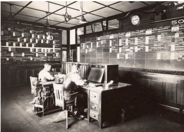
Figure 7.14 Trouble Room on Level 3 (SH 3.12), 1930 (courtesy of ECNSW Archive, 0363-069)
