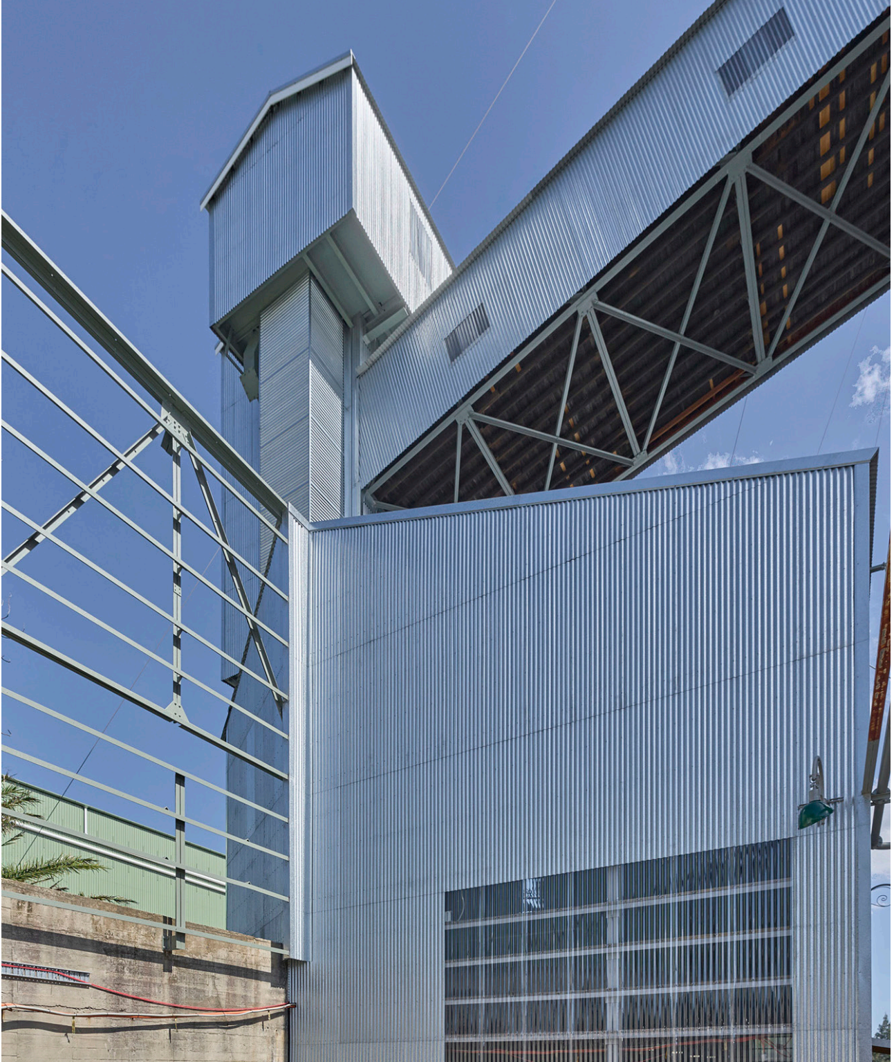
Figure 1.1 The Coal Handling Shed, 2024 (Chris Bennett: Evolving Picture).
