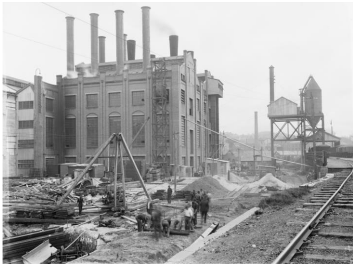
Fig 34: 1924 – Site of No 2 Boiler House, and Turbine Hall/ Pumphouse construction. Foreground shows excavation to bedrock in vicinity of former Padstow House (State Library NSW, FL382932)
