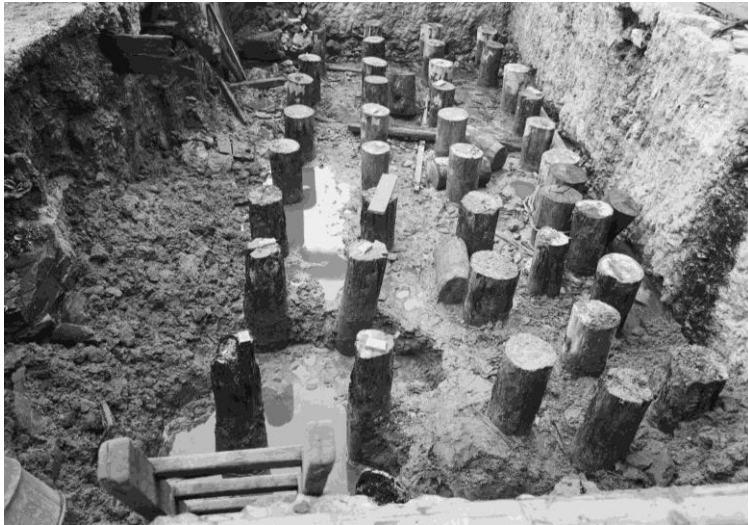
Fig 52: Timber pile foundations for new Boiler House, February 1956. (NSW Archives, NRS-20347-1 674)
