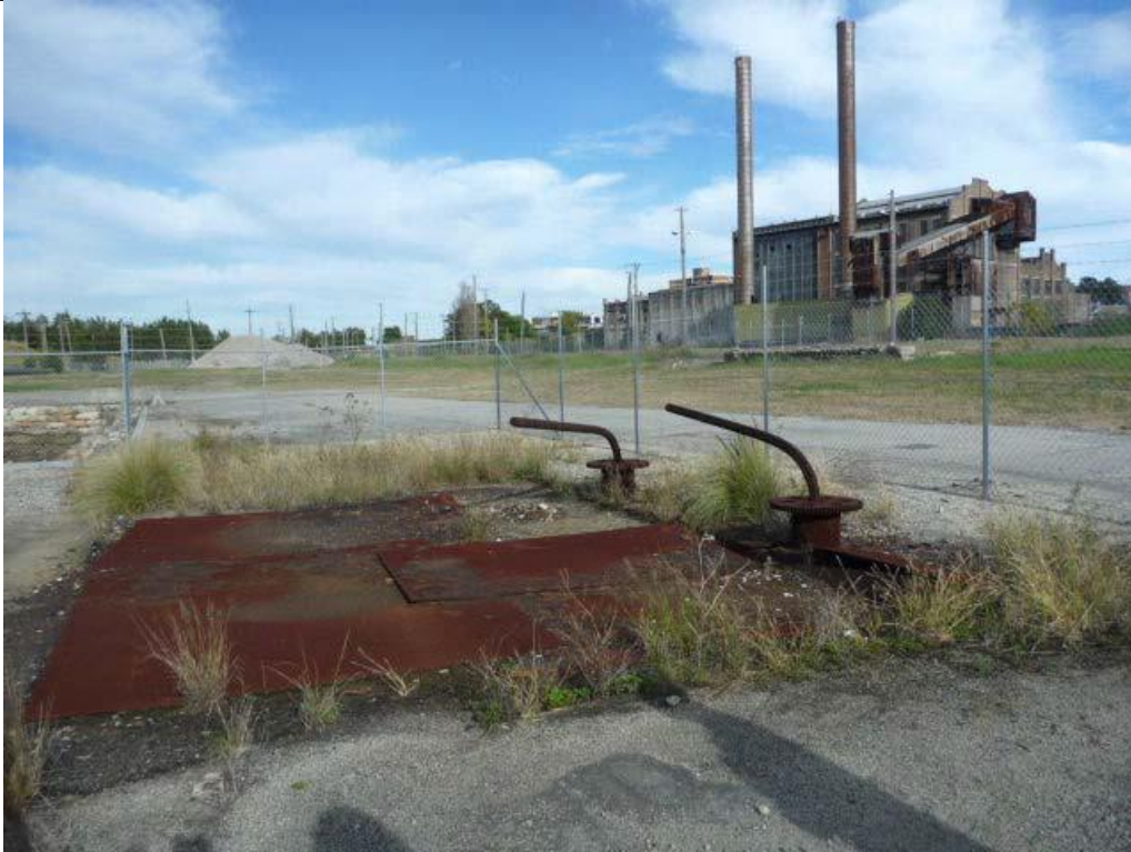
Caption: Site of conduit Entry at White Bay
