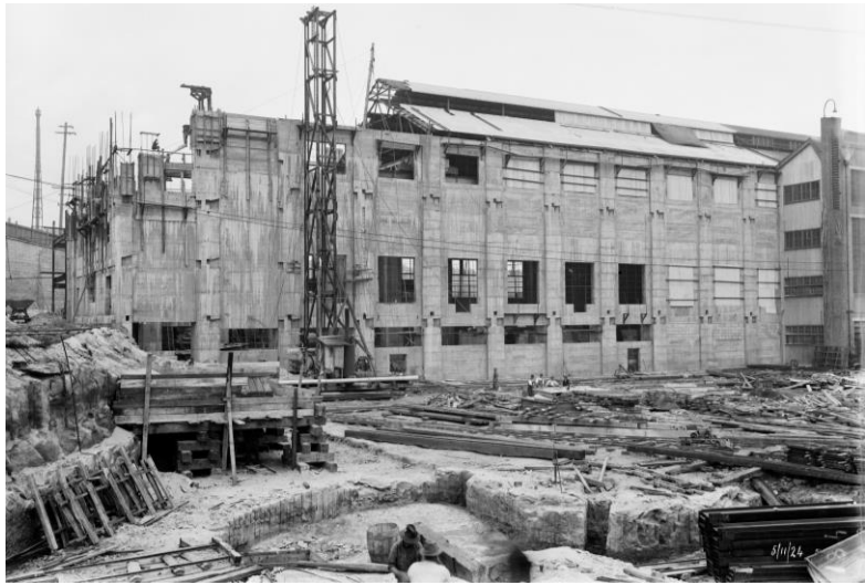
Fig 34: 1924 – Site of No 2 Boiler House, and Turbine Hall/ Pumphouse construction. Foreground shows excavation to bedrock in vicinity of former Padstow House (State Library NSW, FL382932)
