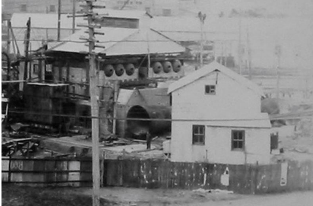
Fig 13: 1912 – The Temporary Boiler House under construction, showing six horizontal boilers in place prior to chimney construction. NSW Archives.
