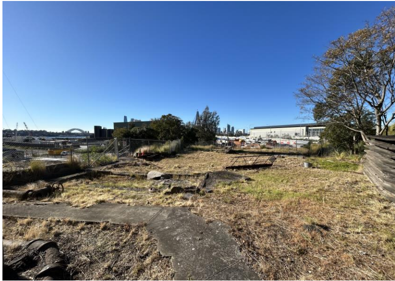
Fig 47: 2025 - South Yard foundations of staff buildings shown in Plan 10 and Figs 49a/b. Lower right shows the bricked-in window in the Administration Building that formerly provided server access between the Canteen and the staff dining room. The timber Canteen had been suspended over the void (shown) and was demolished in c2010 when it became structurally unsound.
