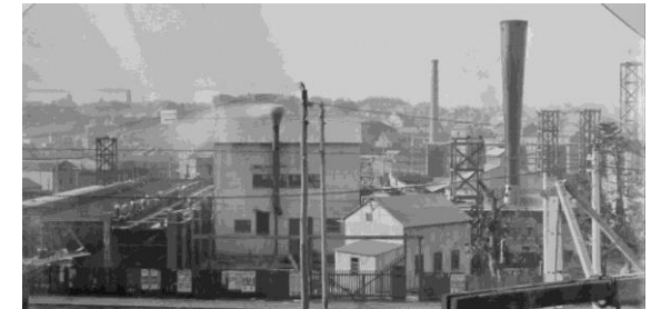
Fig 15: 1913 – The Temporary Power Station: On the left is the Switch House and Transformer Alley, with Turbine Hall west wall.
