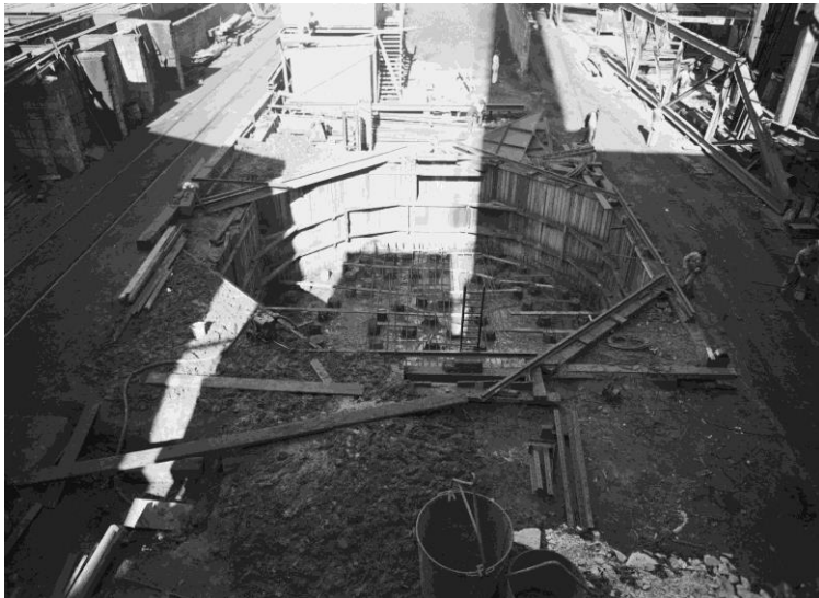
Fig 53: Chimney foundation construction (timber piles), 1957. (NSW Archives, NRS-20347-1 1210 E)
