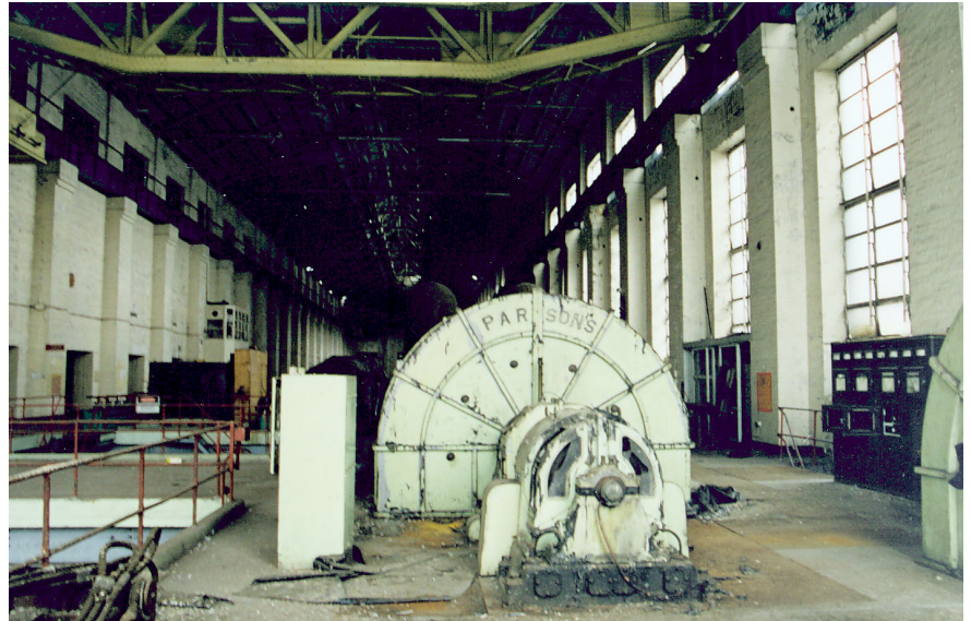
Figure 3.4 View northwards of the Turbine Hall. The Parsons turbo-alternator is located in the centre of this view.
