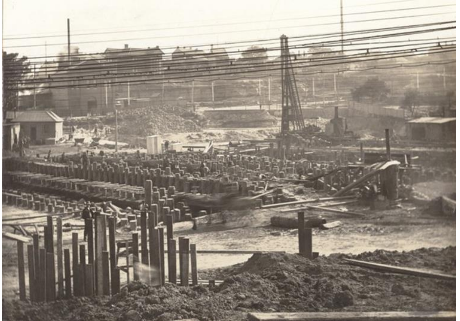
Fig 12: 1912 – Timber pile foundations for the Turbine Hall, Switch House and Boiler House, looking west to Crescent Street and Weston Road. (Archives NSW FL1783437)
