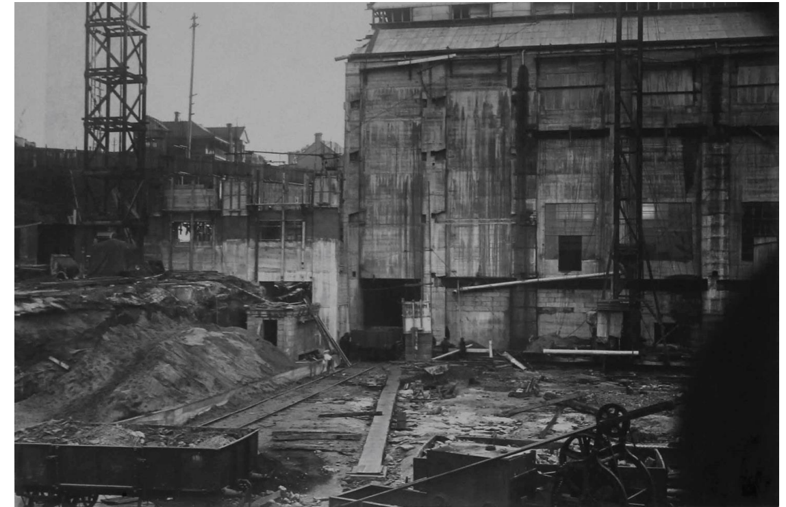
Fig 38: 1925 – Construction on the site of No 2 Boiler House. See also Figs 29, 31. (Former Railway Dept Archives 0363-045)
