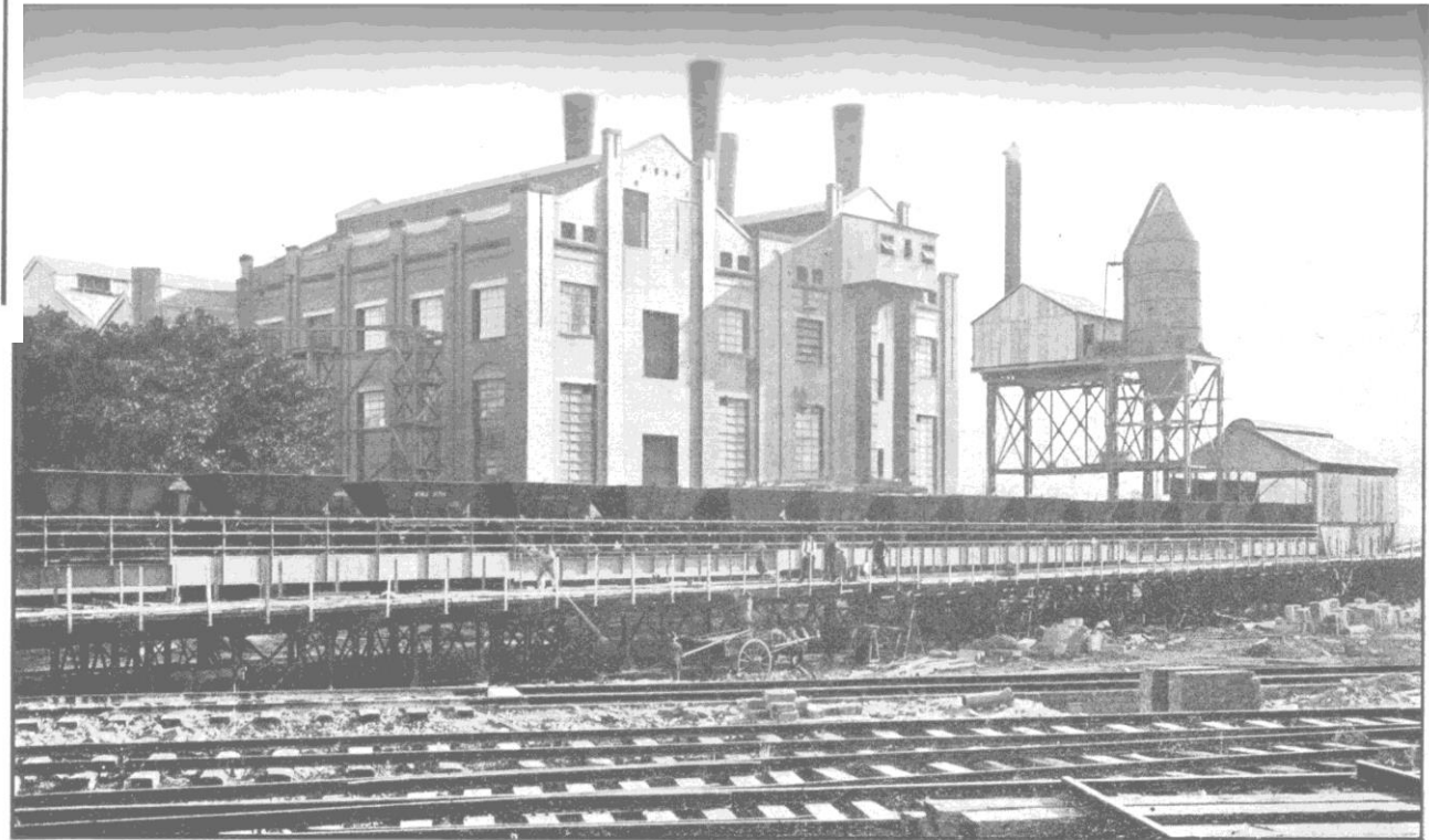
White Bay Power House (showing Elevated Railway Tracks for Coaling).
