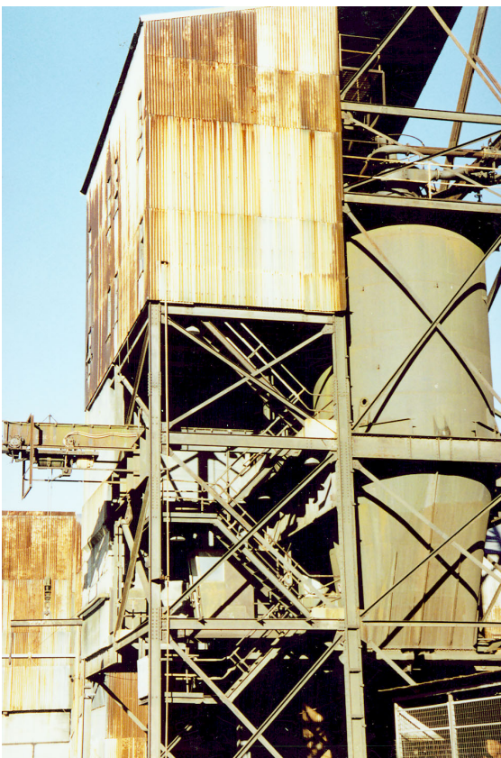
Figure 3.11 The Ash Tower, viewed from the east side, is the only substantial remnant of the Ash handling system.
